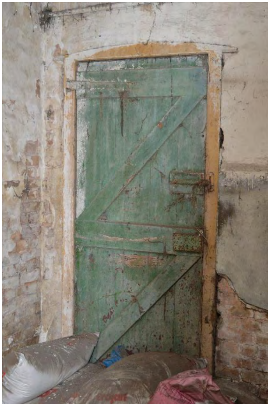
Plate 10: Building B, west unit, typical door design, facing north (40)
