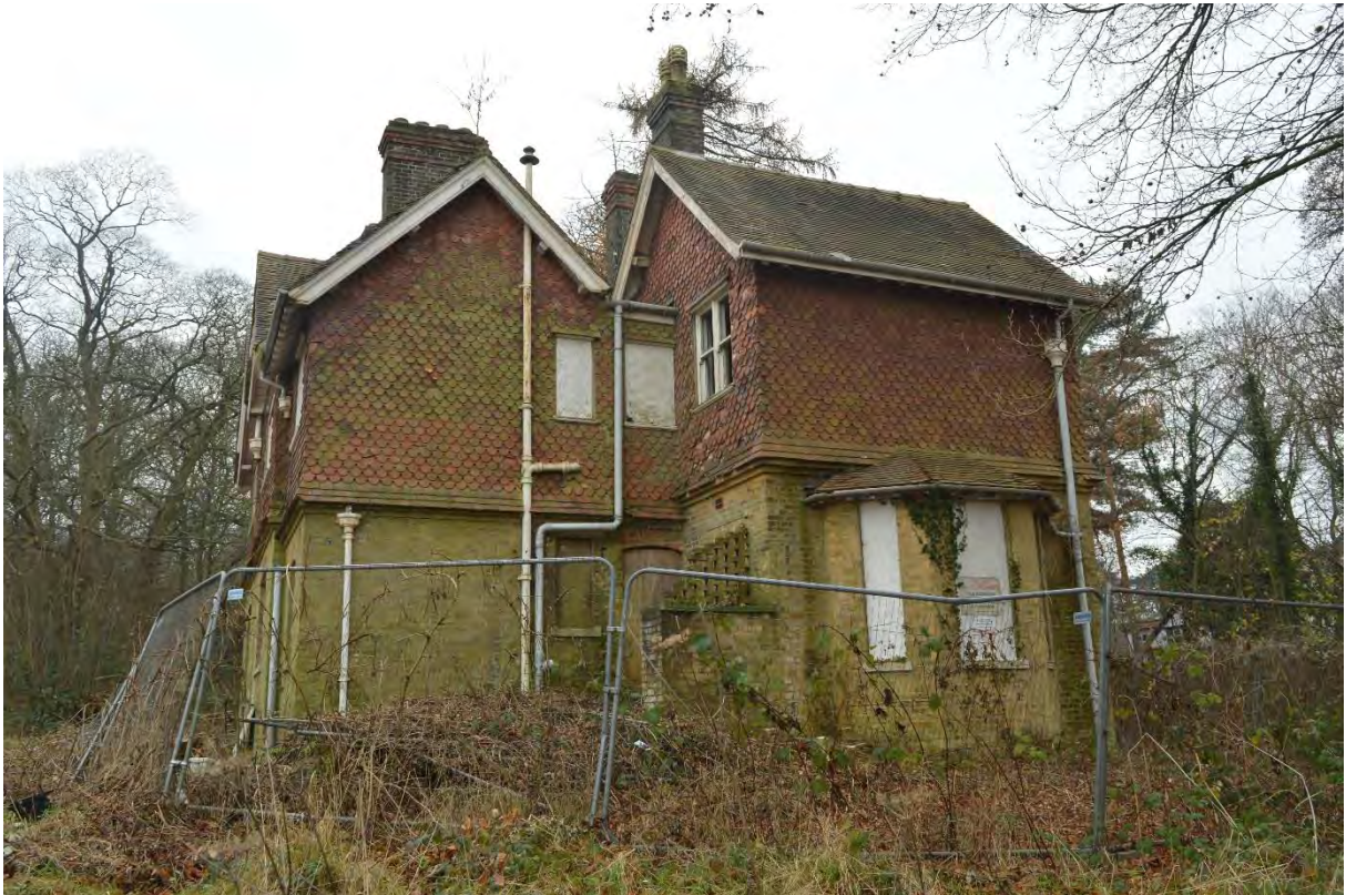
Plate 57: South Lodge, north elevation, facing south (324)
