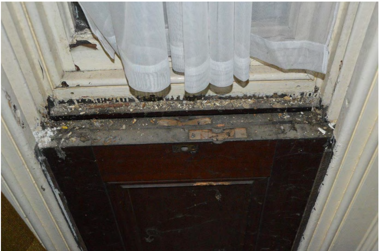
Plate 64: South Lodge, ground floor, Flat 1, Room 3 bay window shutters, facing south (419)
