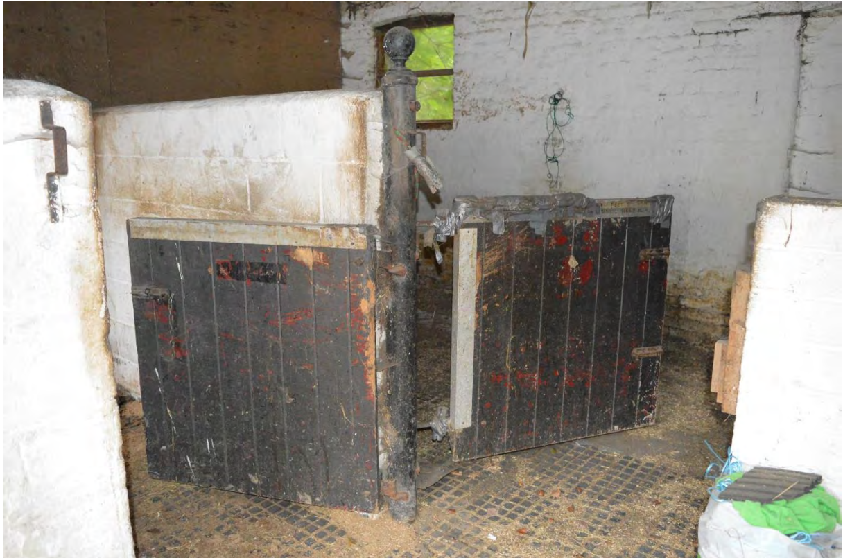
Plate 31: Building F, west unit, end stable enclosures, facing south-east (134)
