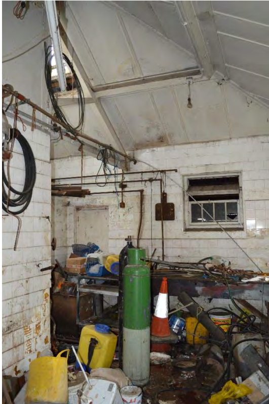
Plate 37: Building G, south unit, southern workshop, facing north-east (94)
