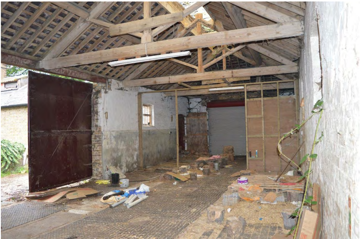
Plate 30: Building F, east unit interior, facing north-east (148)
