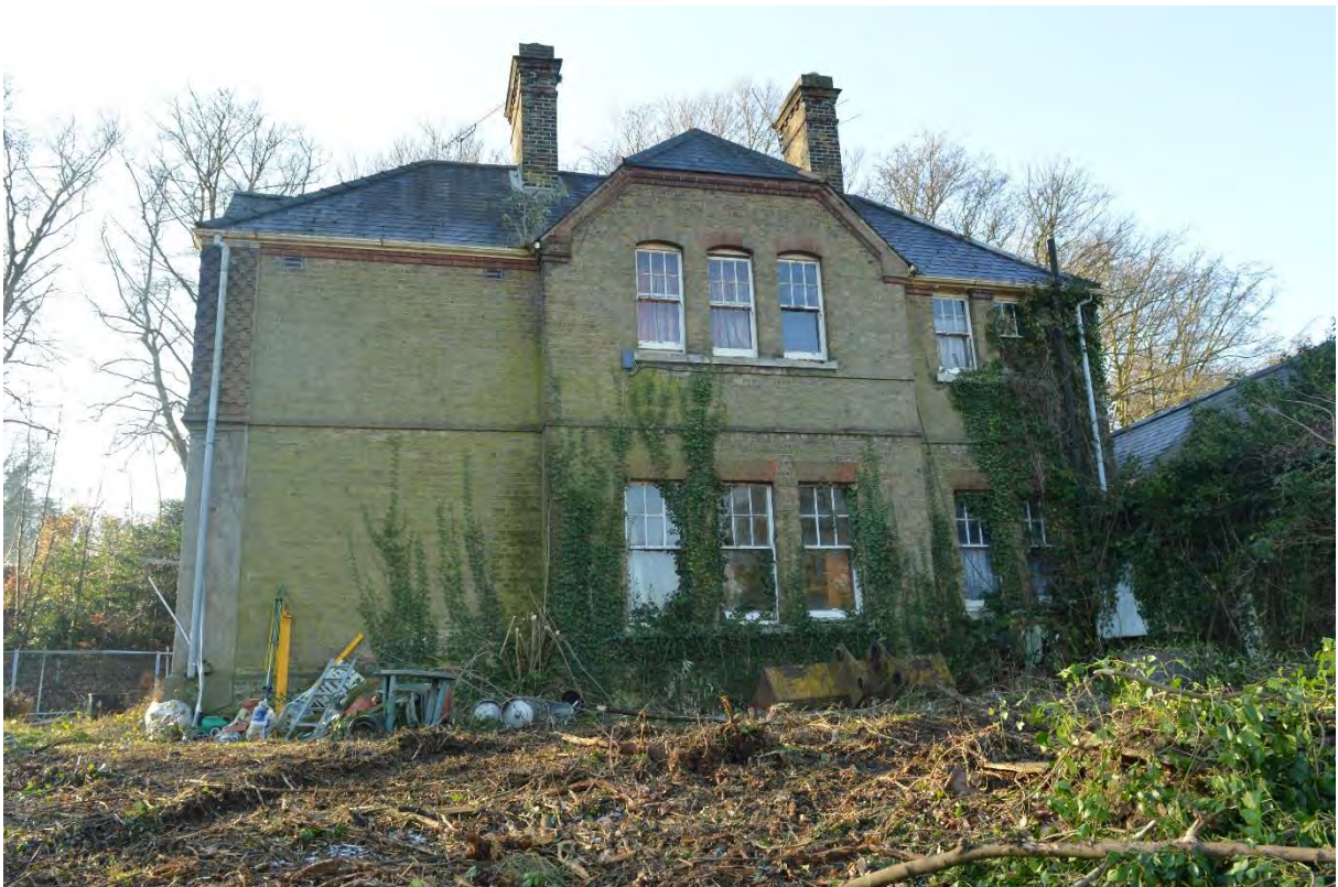
Plate 40: Farmhouse, east elevation, facing south-west (204)
