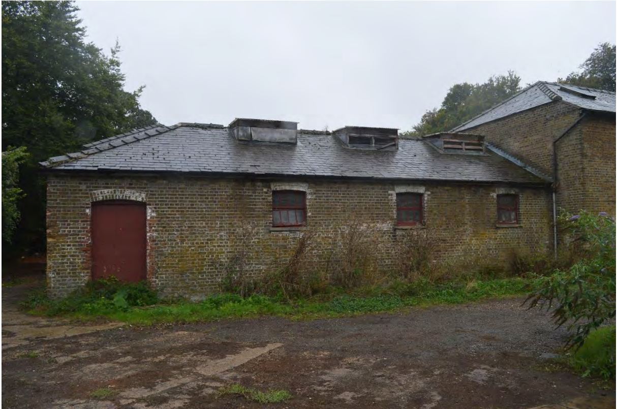
Plate 7: Building B, typical door and window arrangement, facing north-east (31)
