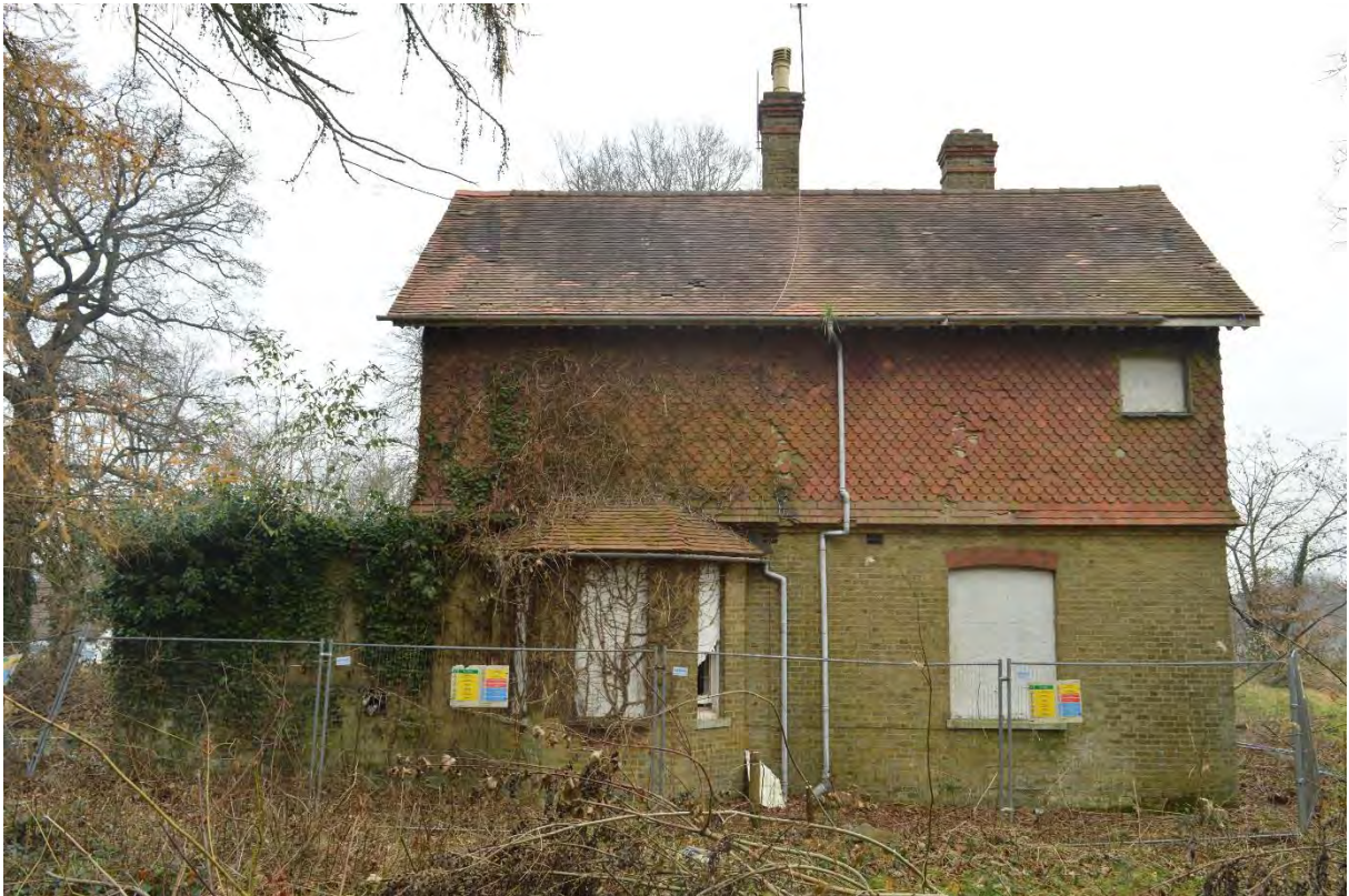
Plate 55: South Lodge, south elevation, facing north (335)
