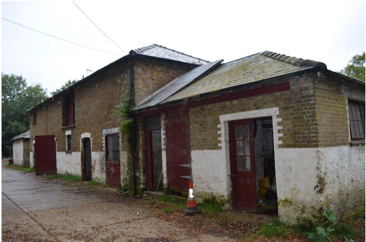
Plate 32: Building G, west elevation, facing north-east (81)
