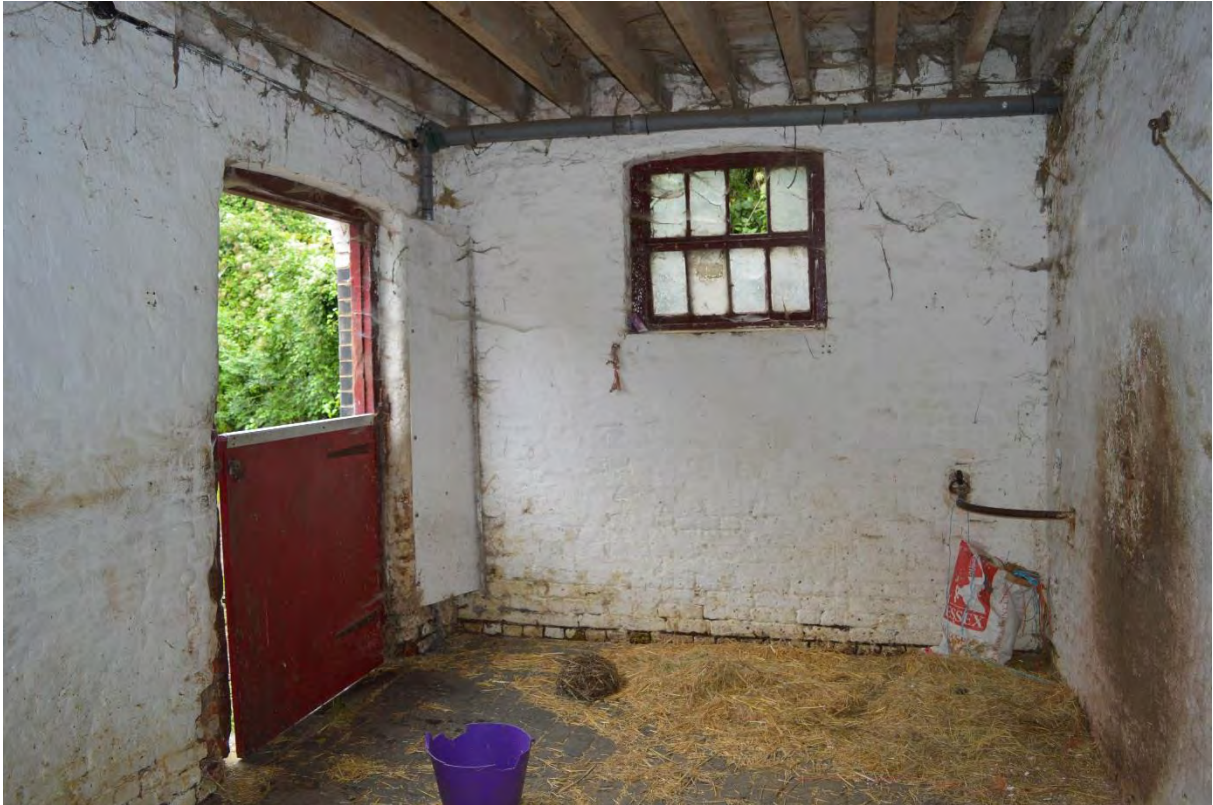
Plate 21: Building D, north unit, Bay 1, facing east (107)
