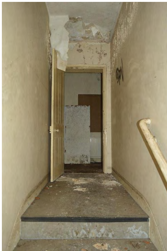
Plate 50: Farmhouse, first floor, staircase, facing north-east (281)
