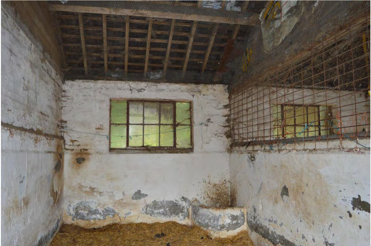
Plate 5: Building A, Bay 9, facing west (13)
