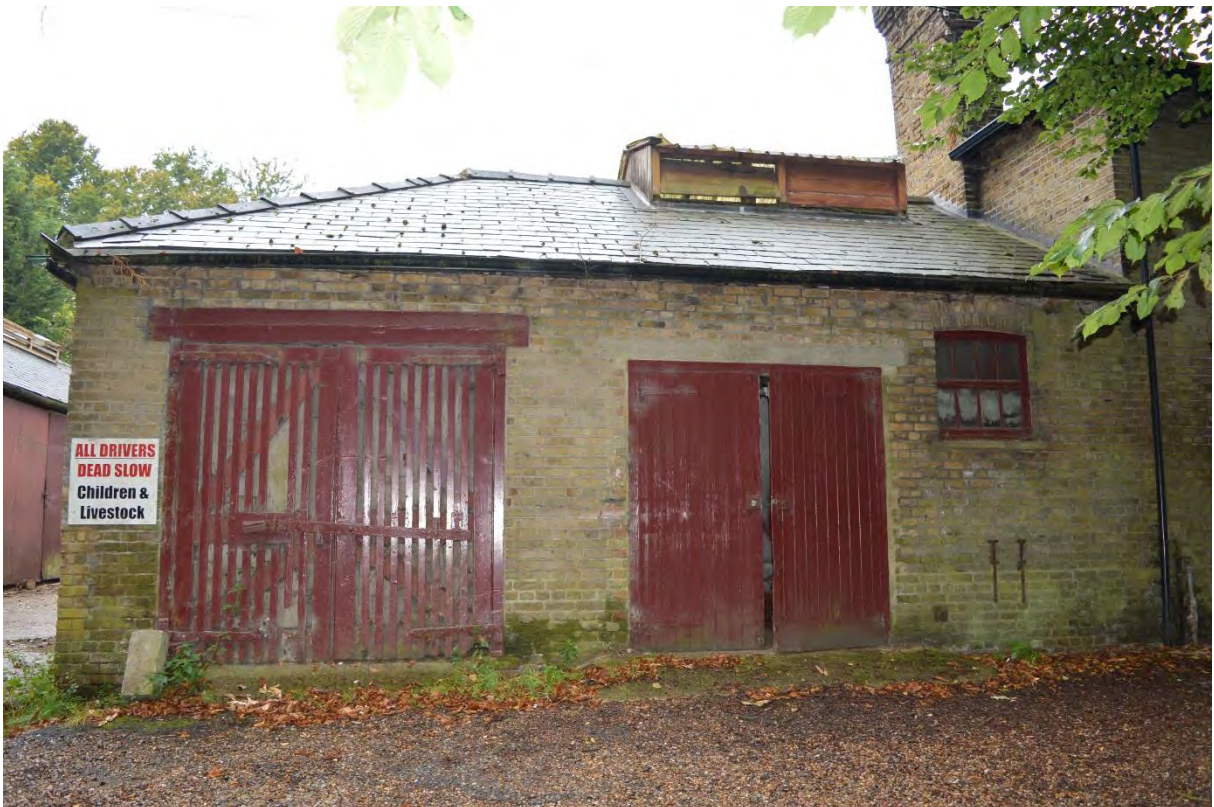
Plate 20: Building D, south unit, east elevation, facing north-west (102)
