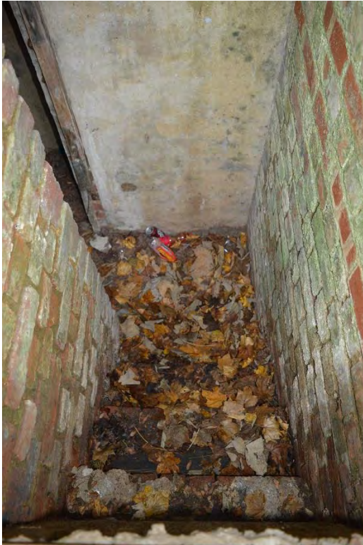
Plate 73: Entrance passage within the air-raid shelter, facing south (356)
