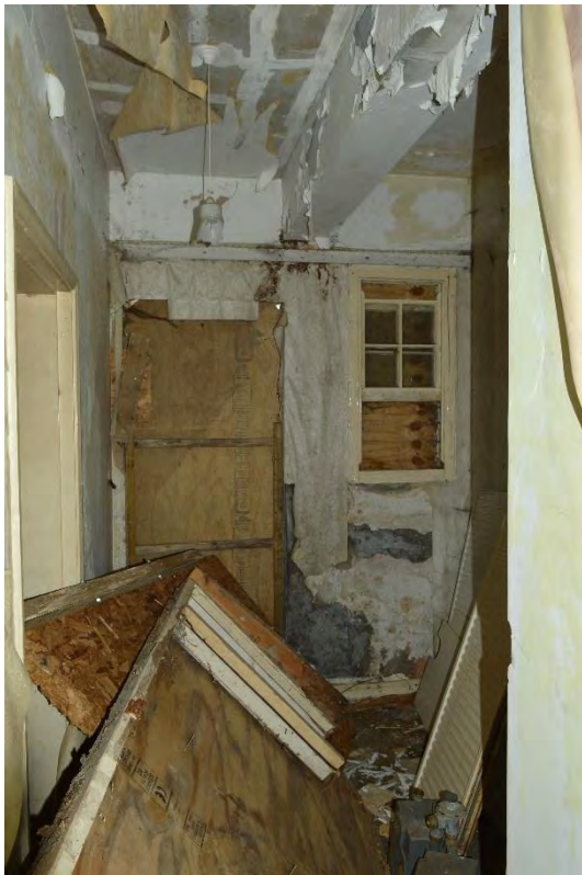
Plate 66: South Lodge, ground floor, Flat 2, inner hall, facing north (399)
