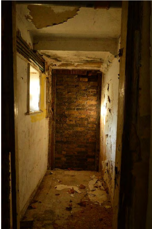
Plate 45: Farmhouse, ground floor, Room 4 under-stair passage, facing north-west (250)
