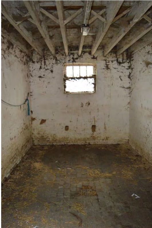
Plate 33: Building G, north unit, Bay 1, facing east (83)
