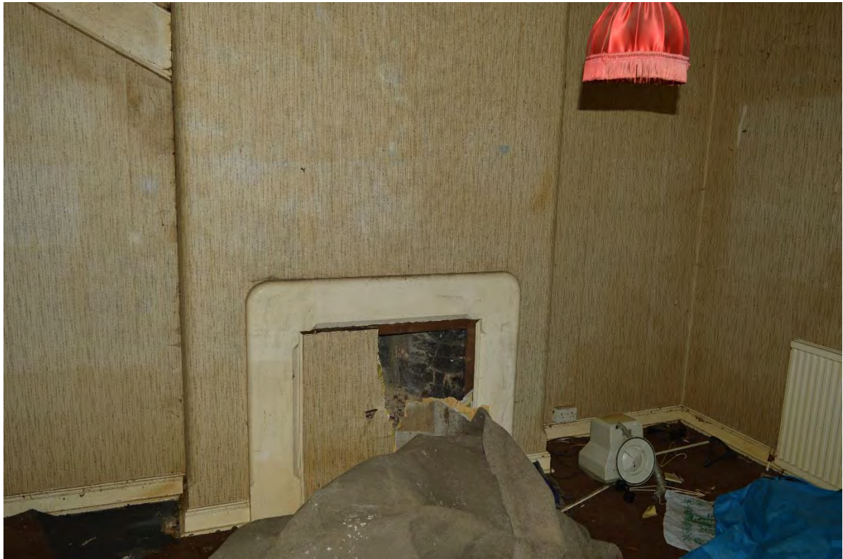
Plate 51: Farmhouse, first floor, Room 11 showing fireplace, facing north-west (286)
