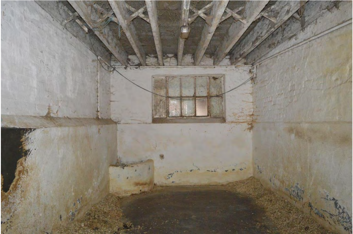
Plate 35: Building G, north unit, Bay 5, facing east (91)
