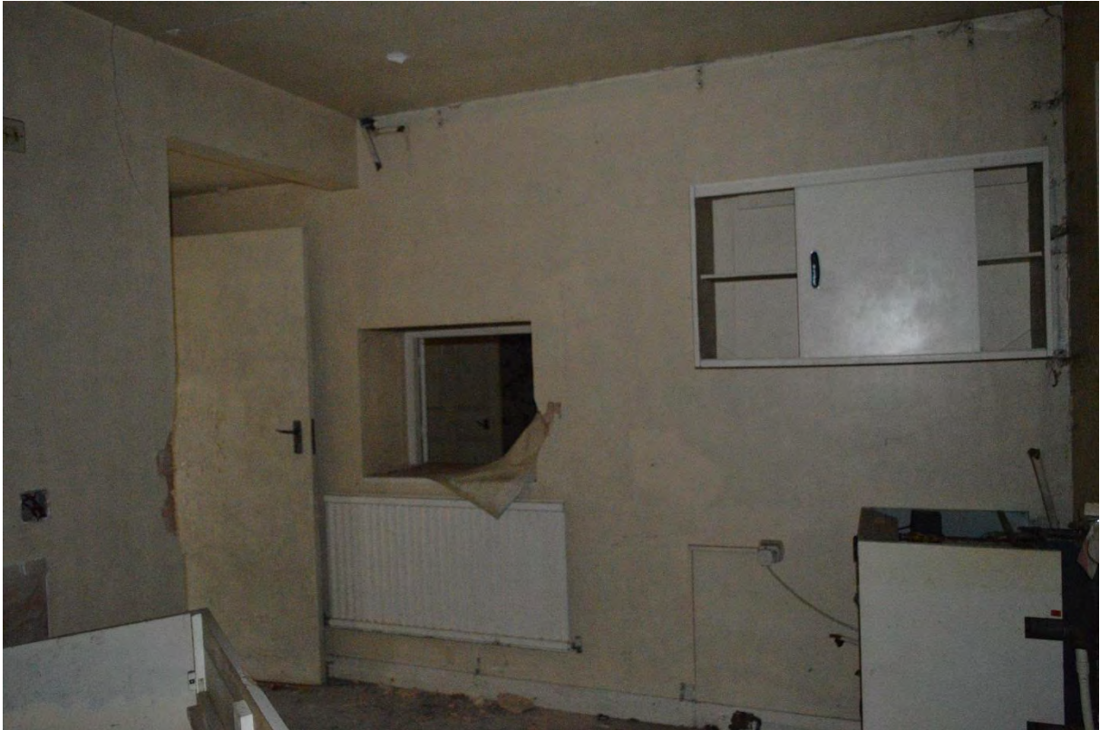
Plate 59: South Lodge, ground floor, Flat 1, western extension, Room 2, facing north-east (366)
