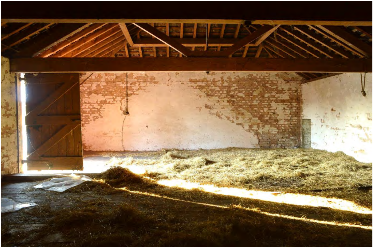
Plate 12: Building B, central unit, first floor hay loft, facing south-west (189)
