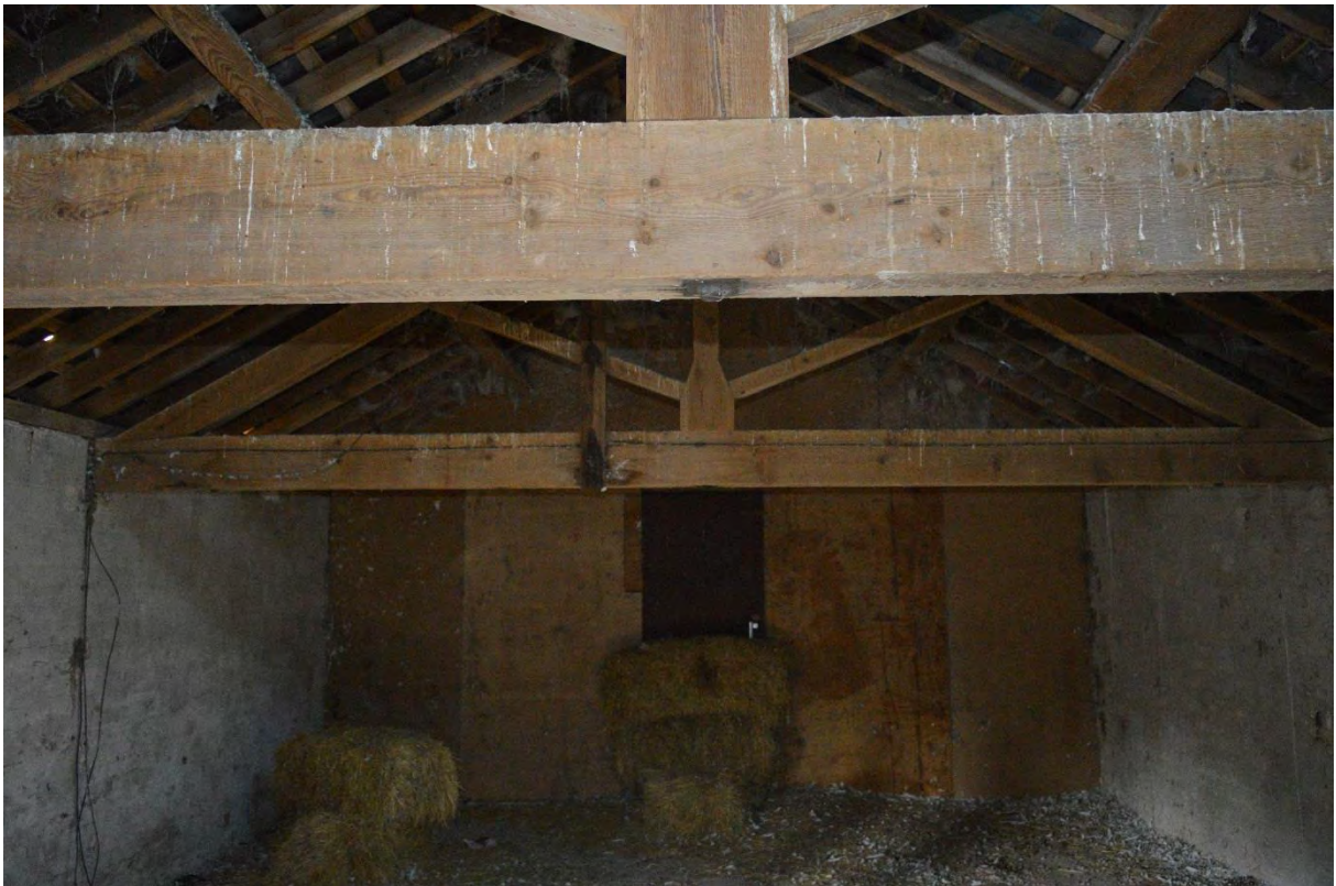
Plate 36: Building G, north unit, first floor level hay loft, facing north (186)
