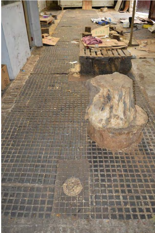
Plate 29: Building F, east unit floor divisions and redundant footings, facing east (146)
