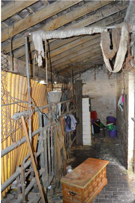
Plate 17: Building C, east end interior, facing north (75)
