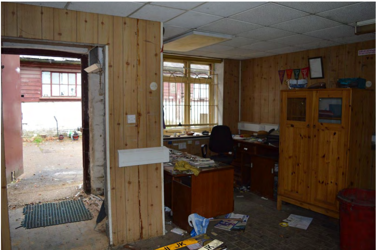
Plate 34: Building G, north unit, Bay 2 office conversion, facing north-west (87)
