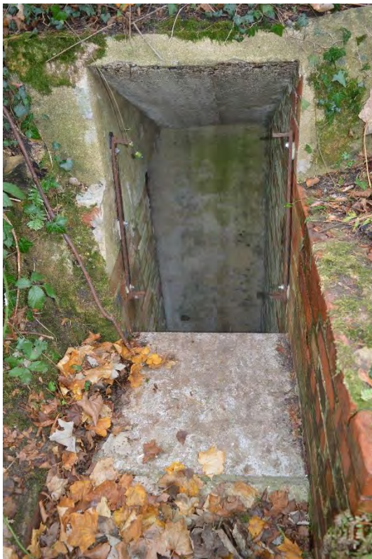
Plate 72: Principal northern entrance of the air-raid shelter, facing south (355)
