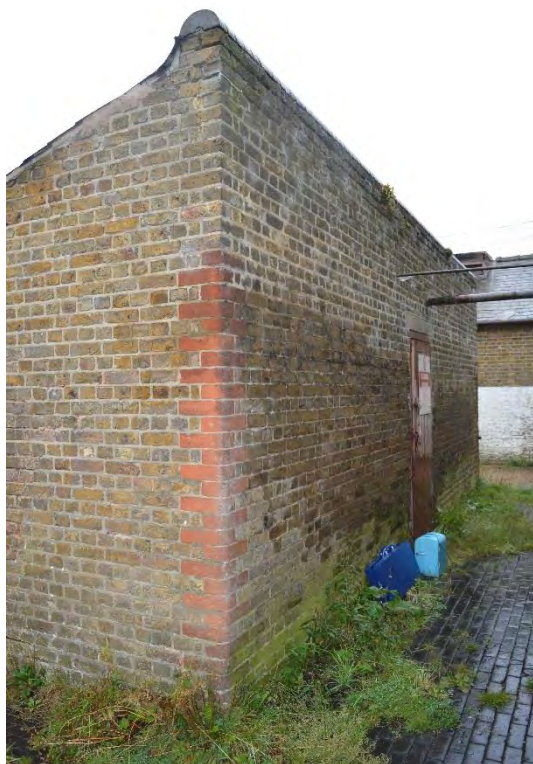
Plate 16: Building C, east elevation, facing north-west (73)
