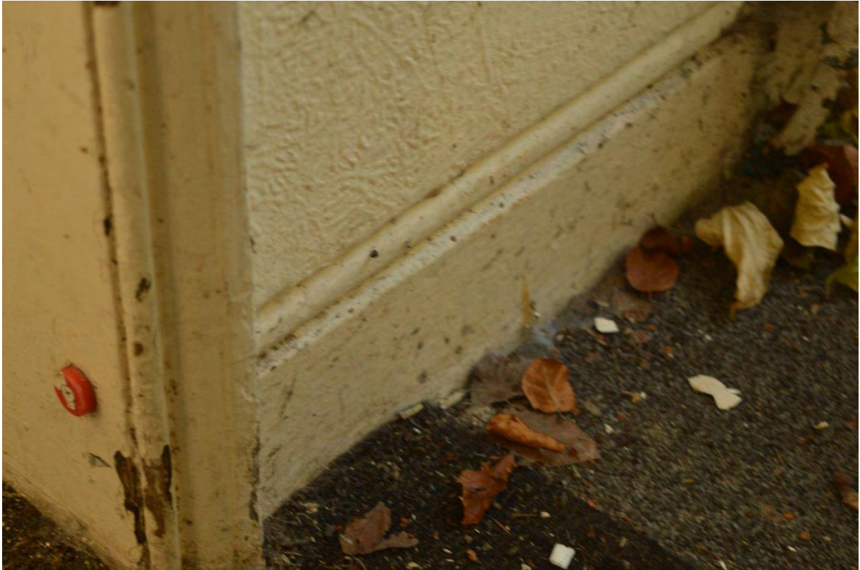
Plate 43: Farmhouse, ground floor, integral skirting within the corridor, facing north-east (241)
