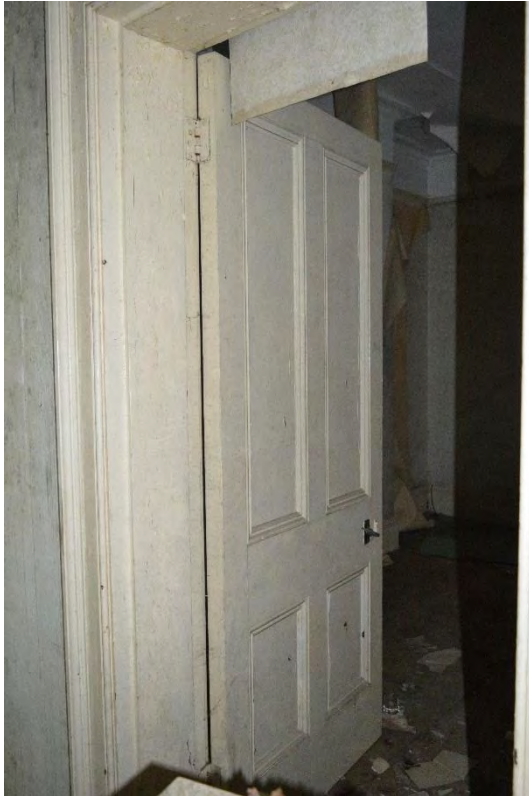
Plate 61: South Lodge, ground floor, Flat 1, Room 3 door detailing, facing south-east (370)
