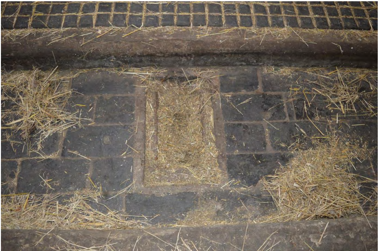
Plate 14: Building B, east unit, cast iron floor footings for former stalls/tethering pole, facing north (65)
