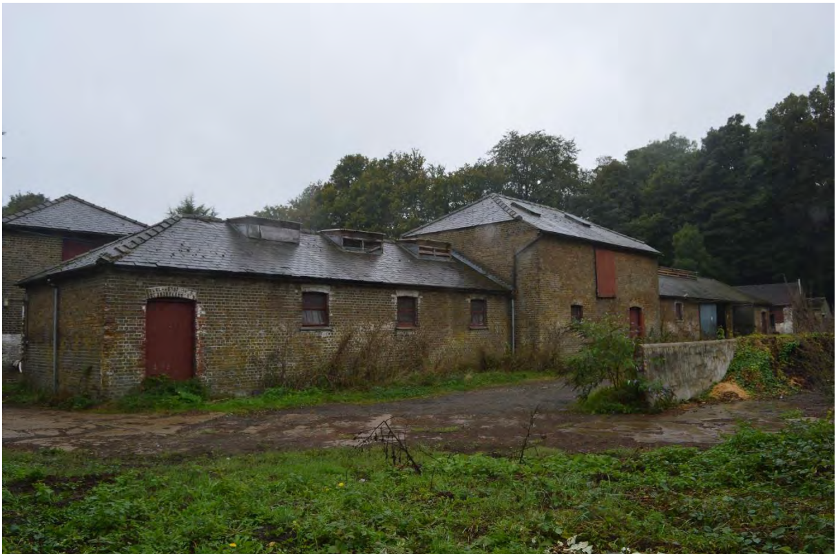
Plate 6: External north elevation of Building B, facing south-west (30)
