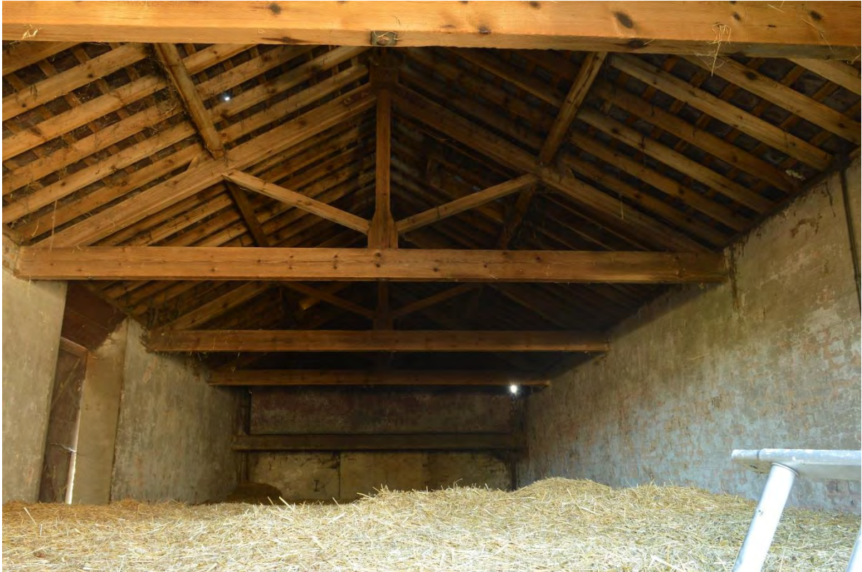
Plate 23: Building D, north unit, first floor hay loft, facing south (165)
