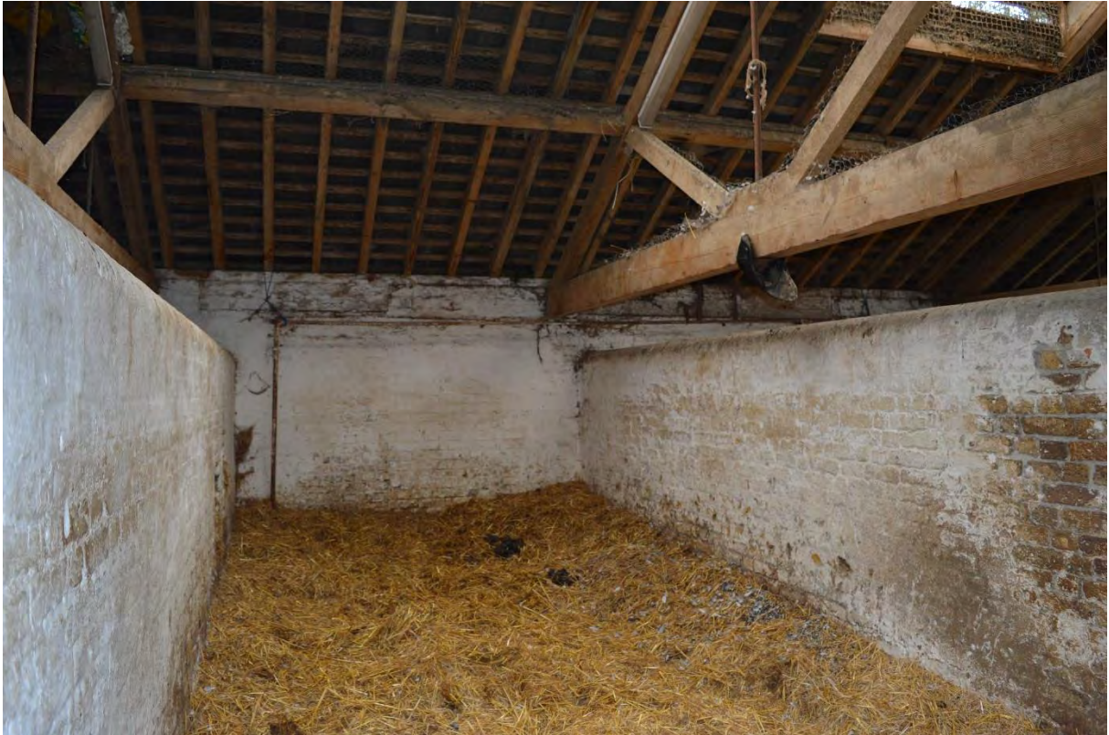
Plate 27: Building E, stable enclosure within Bay 2, facing east (160)
