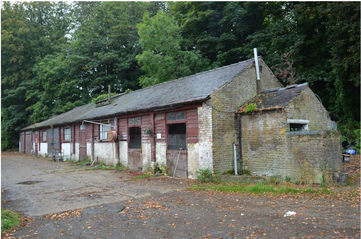
Plate 2: East elevation of Building A, facing south-west (7)
