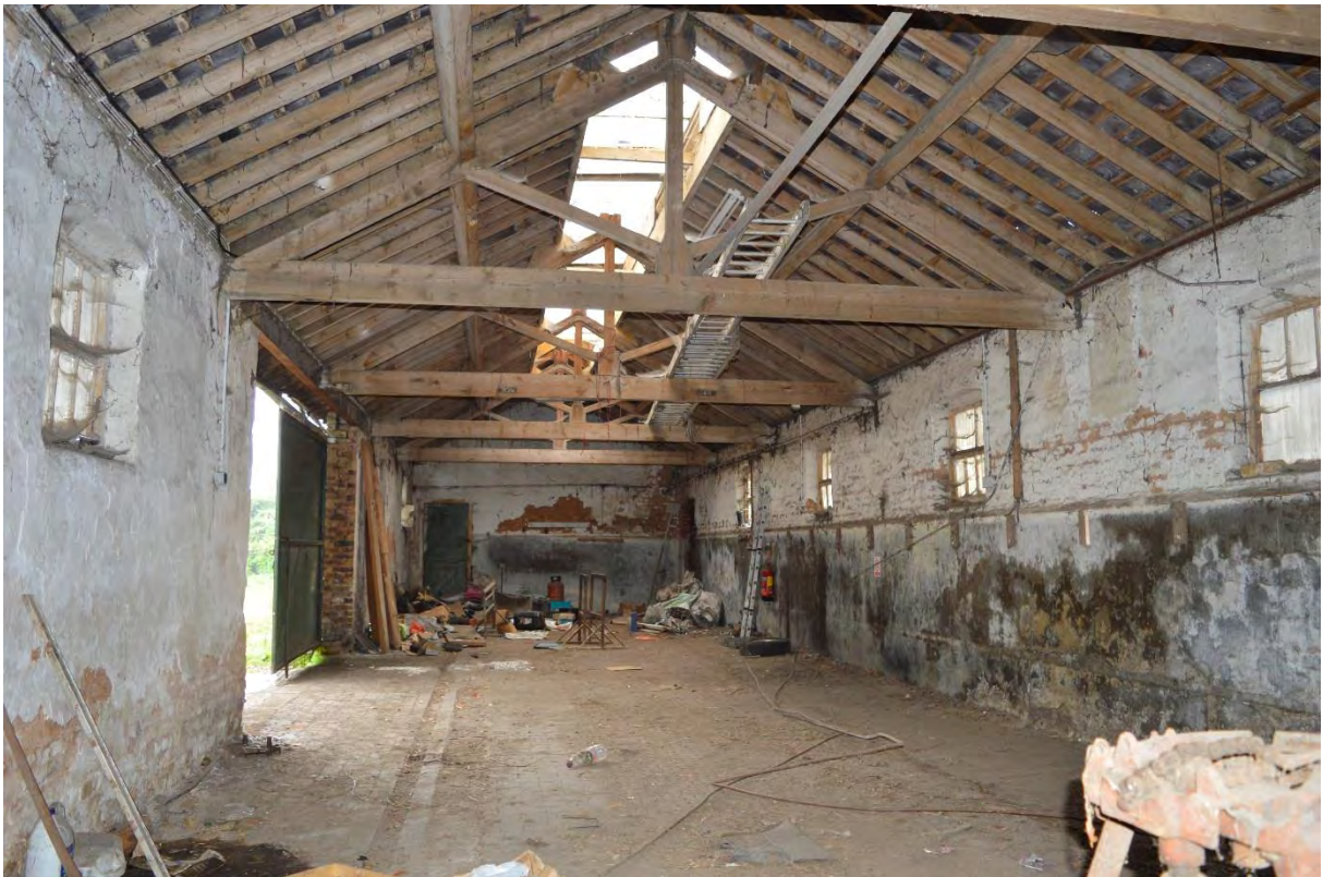
Plate 8: Building B, west unit, interior, facing east (37)
