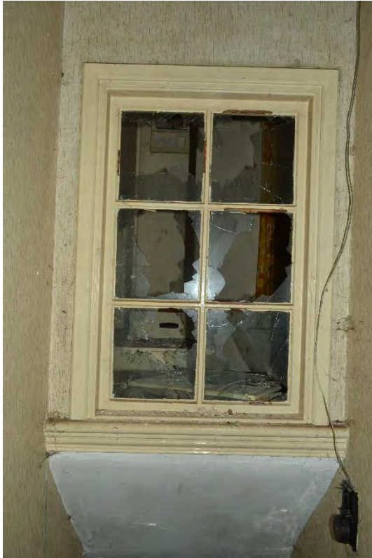
Plate 71: South Lodge, ground floor, Flat 3, internal stairwell window, facing west (432)
