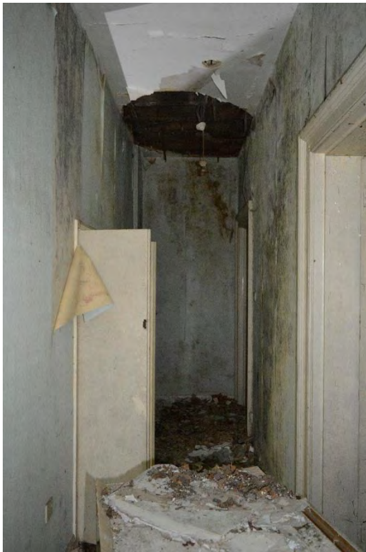
Plate 60: South Lodge, ground floor, Flat 1, eastern corridor, facing east (368)
