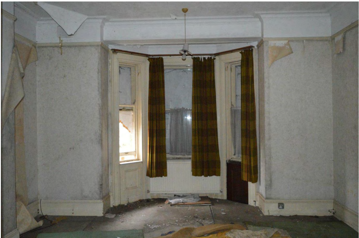
Plate 62: South Lodge, ground floor, Flat 1, Room 3, facing south (372)
