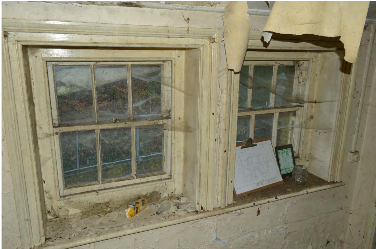
Plate 49: Farmhouse, first floor, stairwell windows, facing south-west (280)
