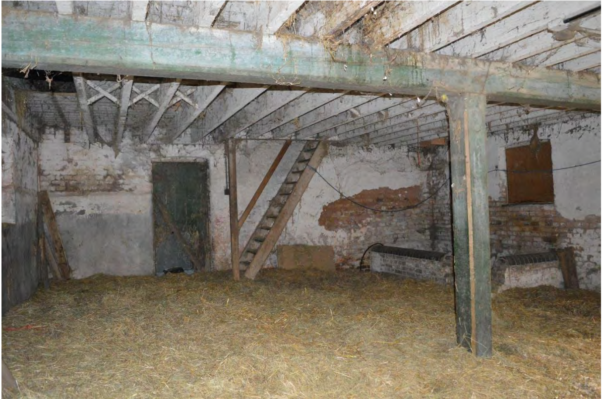
Plate 11: Building B, central unit, ground floor level, facing south-east (48)
