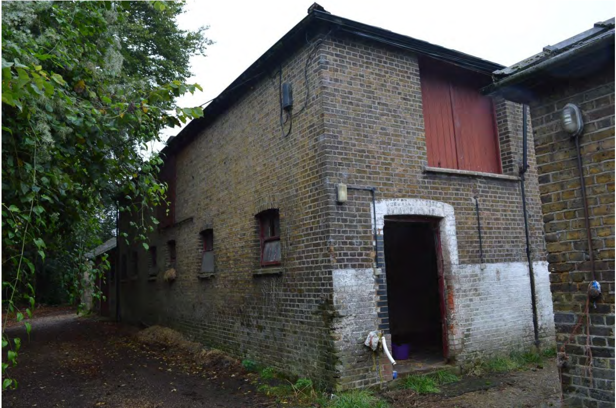
Plate 19: Building D, north unit, east and north elevations, facing south-west (104)
