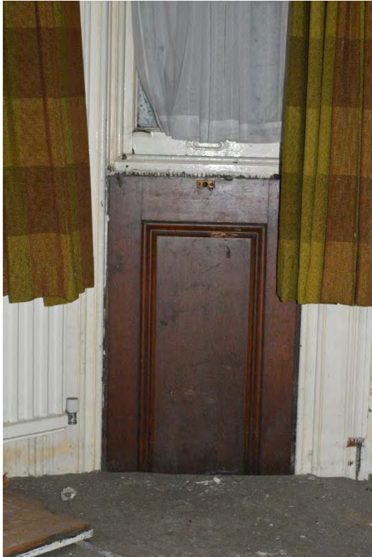
Plate 63: South Lodge, ground floor, Flat 1, Room 3 bay window detailing, facing south (418)
