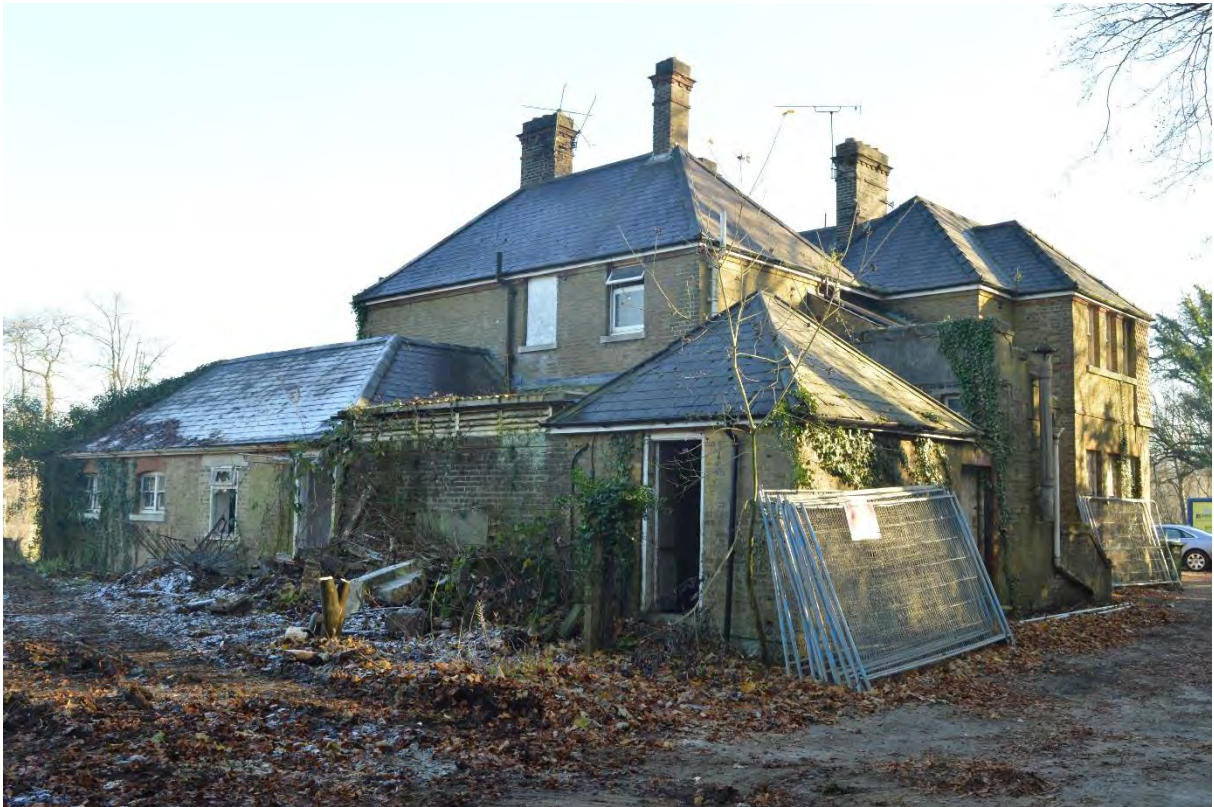
Plate 41: Farmhouse, north and west elevations, facing south-east (213)
