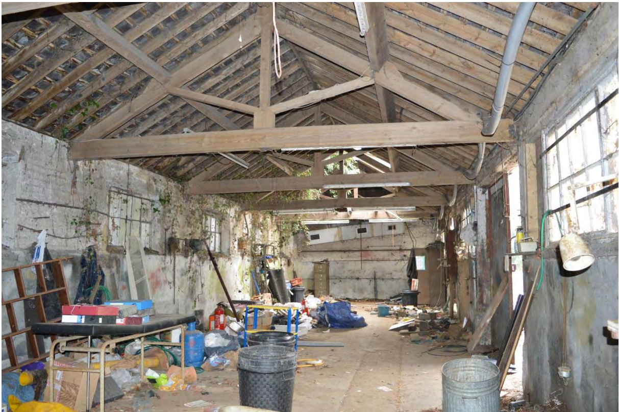
Plate 4: Building A, internal workshop area, facing north (14)
