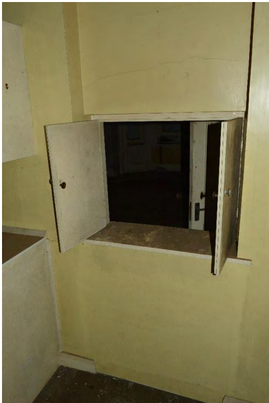
Plate 68: South Lodge, ground floor, Flat 2, Room 7 serving hatch, facing north (416)
