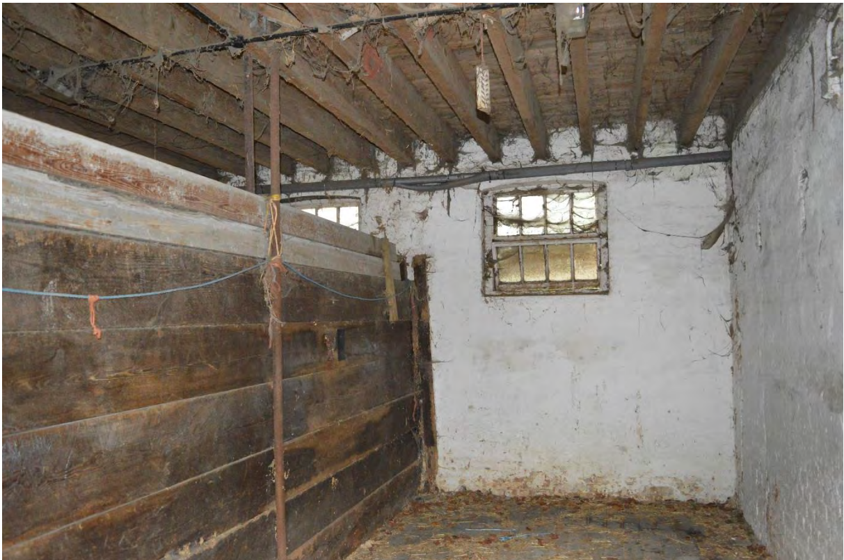
Plate 22: Building D, north unit, Bay 3 partition, facing north-east (112)
