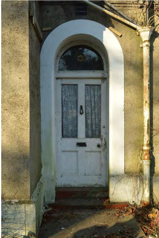
Plate 39: Farmhouse, main entrance, facing north-west (203)
