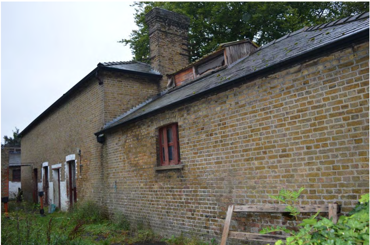
Plate 18: West elevation of Building D, facing north-east (99)
