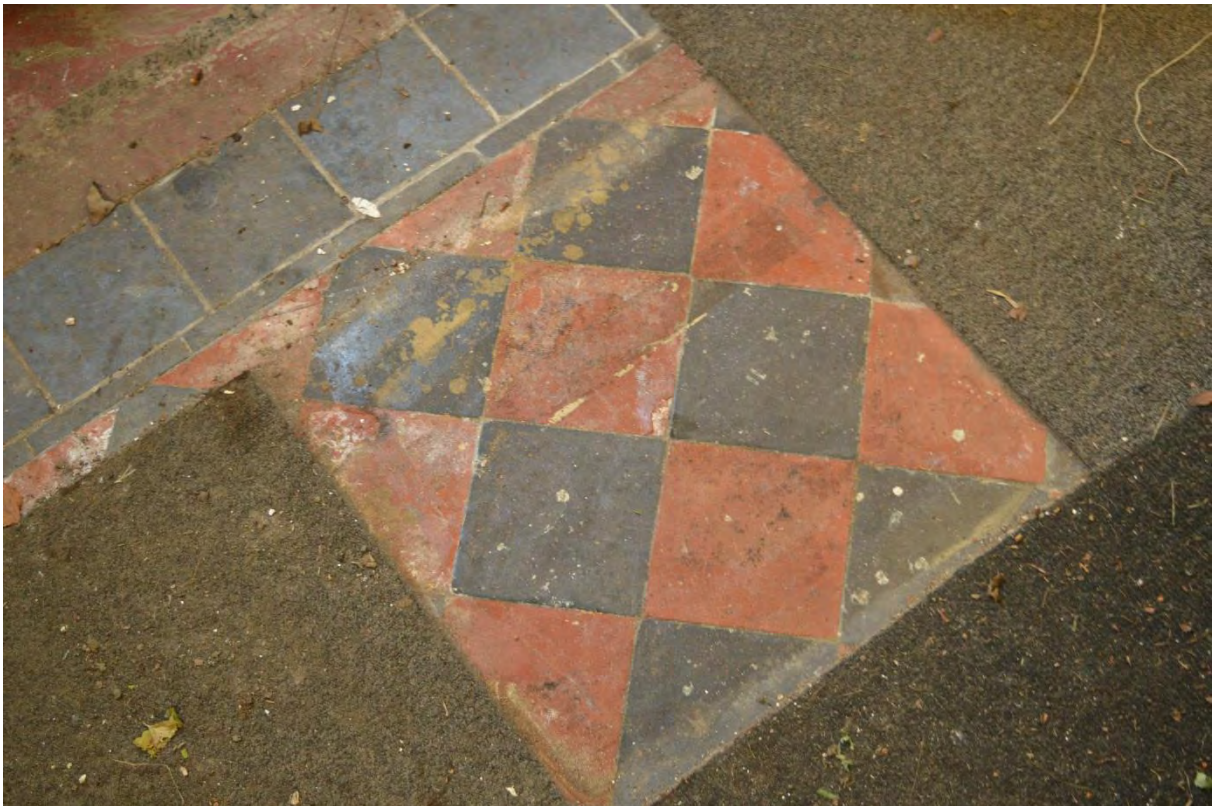
Plate 44: Farmhouse, ground floor, entrance floor tiles, facing north-east (237)
