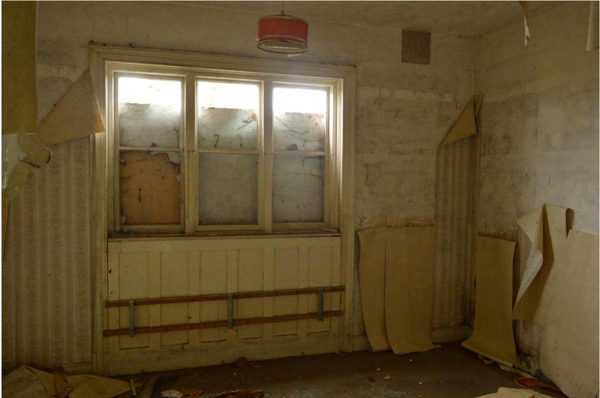
Plate 67: South Lodge, ground floor, Flat 2, Room 6, facing east (397)
