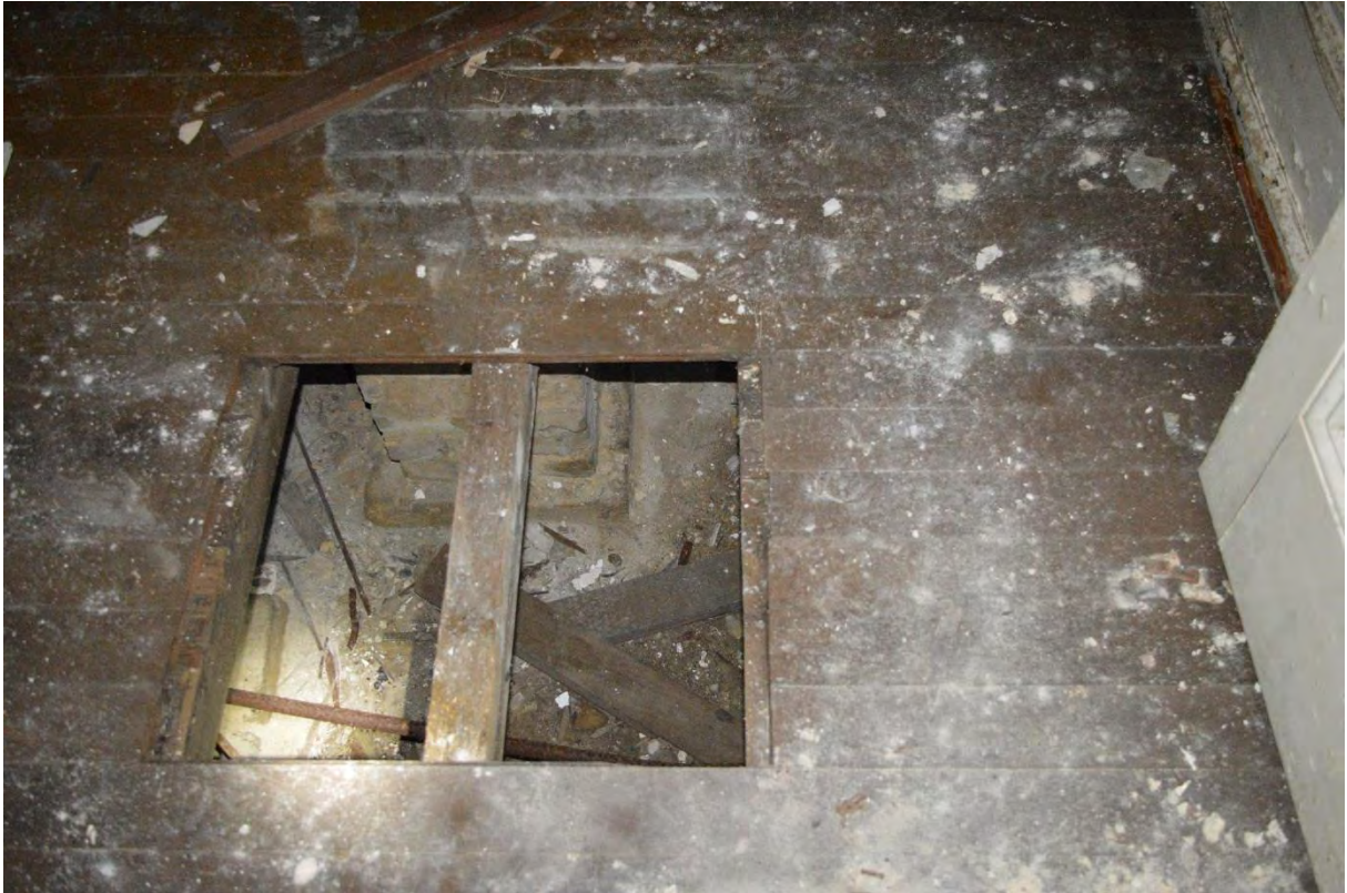
Plate 65: South Lodge, ground floor, Flat 1, Room 4 floor arrangement, facing south (388)
