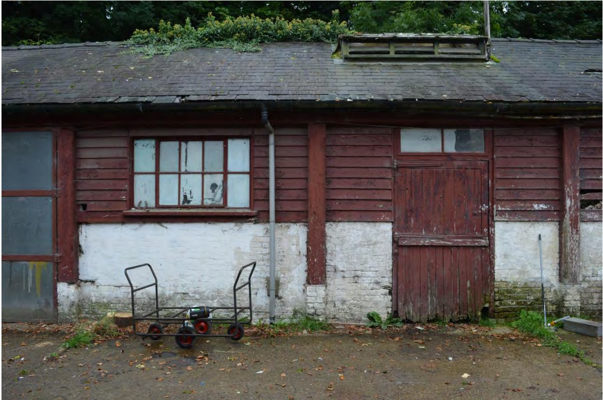
Plate 3: Detail of the former open front to Building A, facing west (5)
