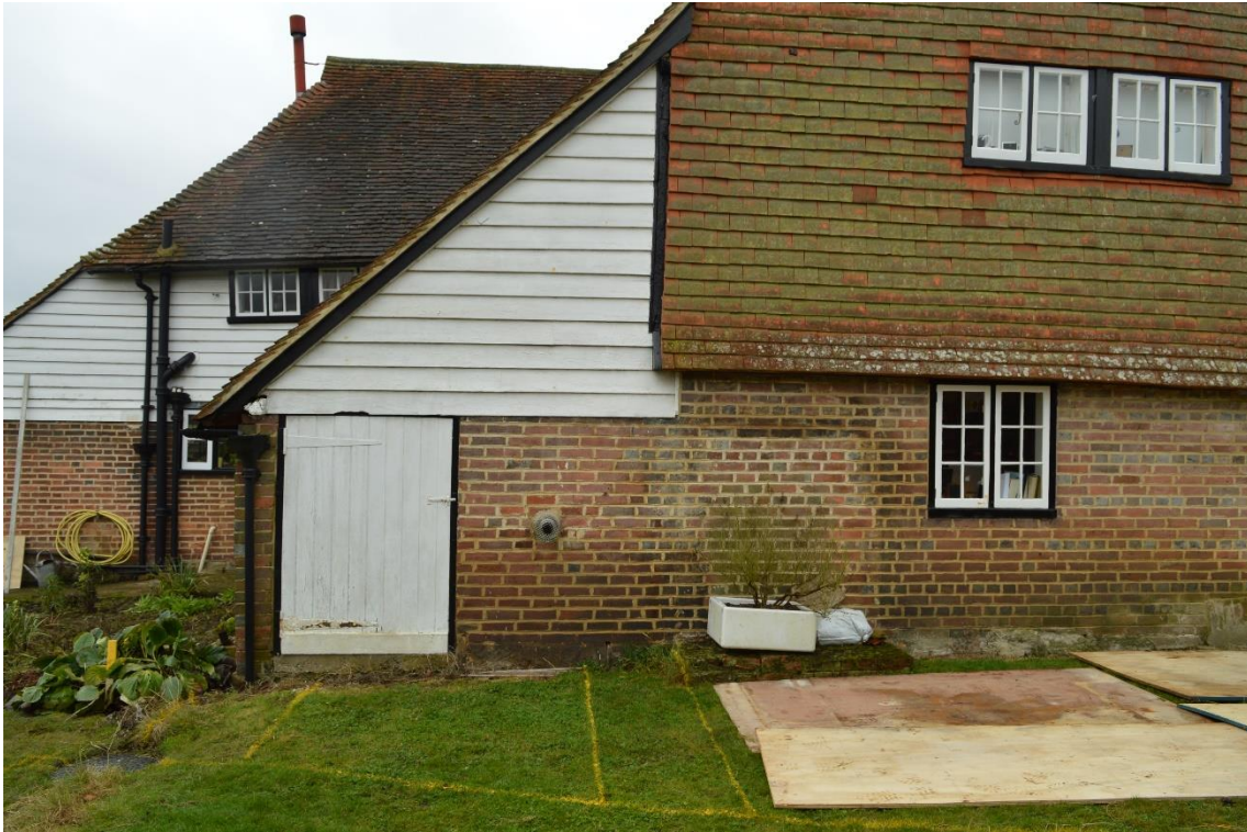
Plate 3: East elevation of farmhouse and lean-to (PEL17-0008)
