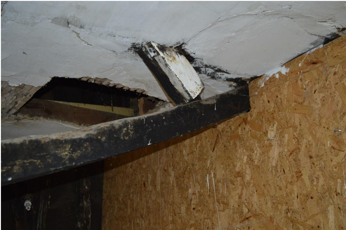
Plate 6: Lean-to tie beam and raking strut, facing west (PEL17-0019)
