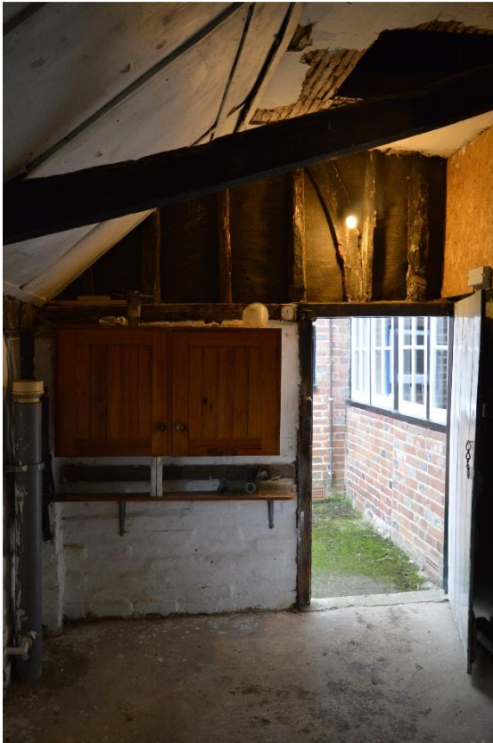
Plate 7: Interior of lean-to, facing west (PEL17-0012)
