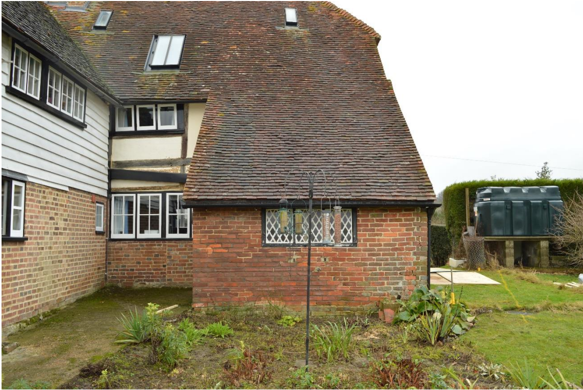
Plate 5: South elevation of lean-to (PEL17-0005)
