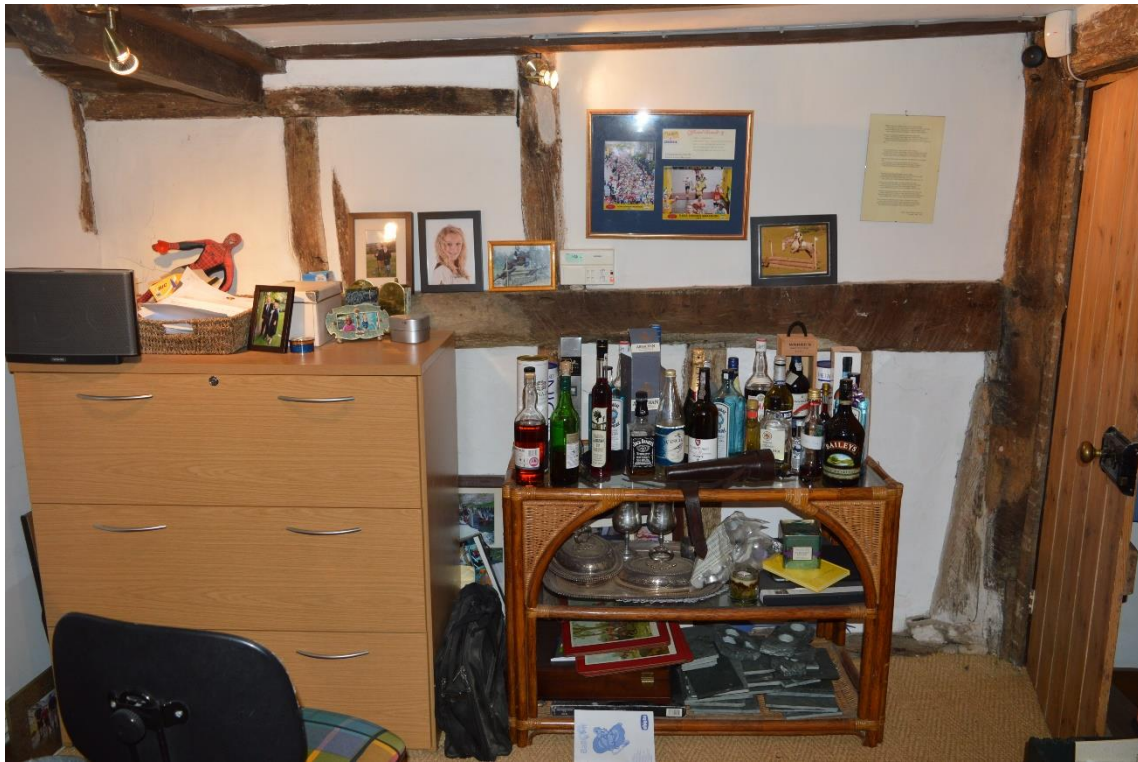
Plate 9: Wall shared between lean-to and main range, facing south (PEL17-0031)
