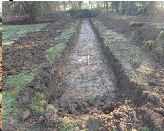
Figure 6: Trench 4, view southeast
