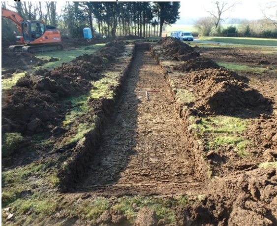
Figure 5: Trench 3, view southwest
