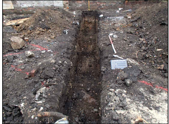
East trench with two services and natural between looking NE
