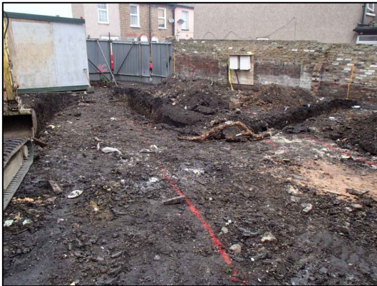
Overall shot, looking NW
