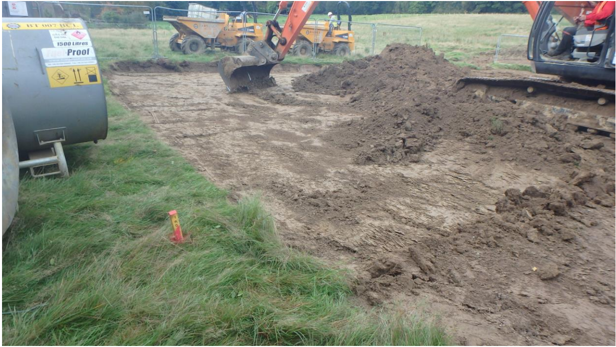
Plate 1: Stripping the compound area (looking south)
