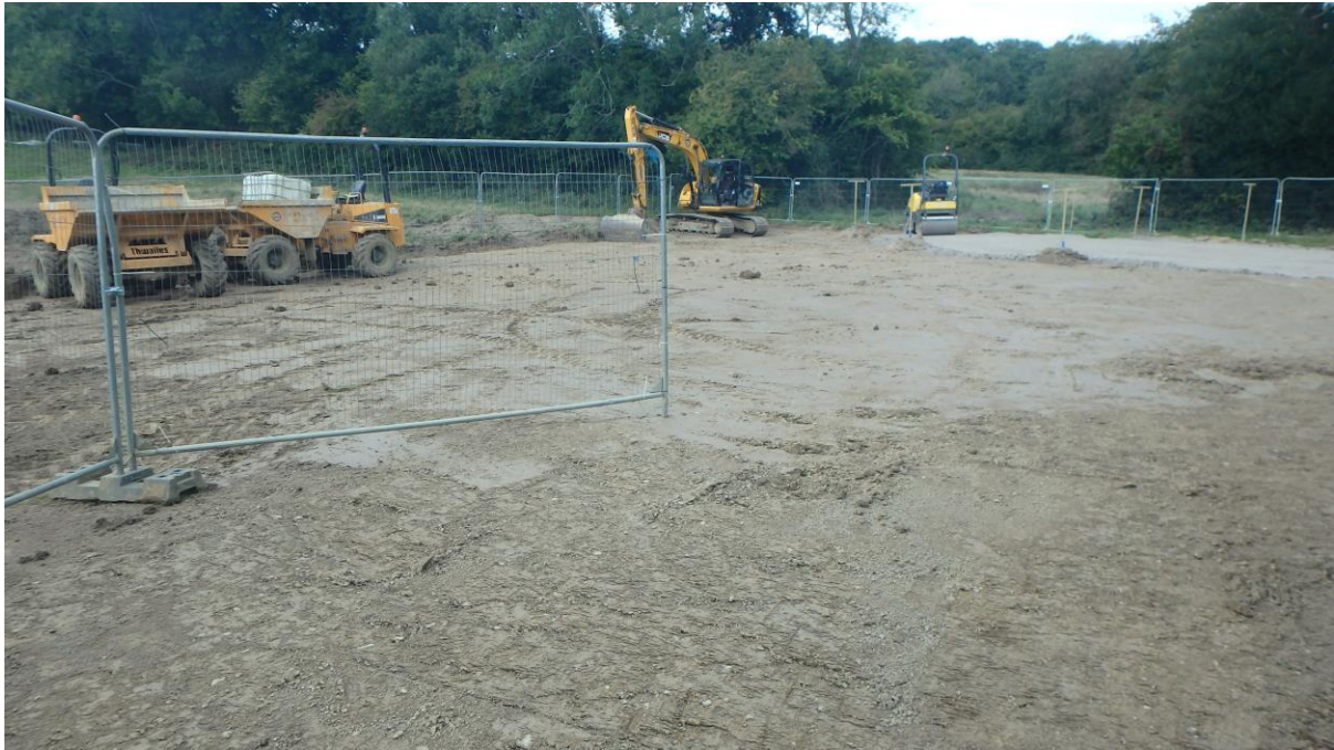
Plate 3: Stripped compound area showing breach though hedgerow in distance (looking north)
