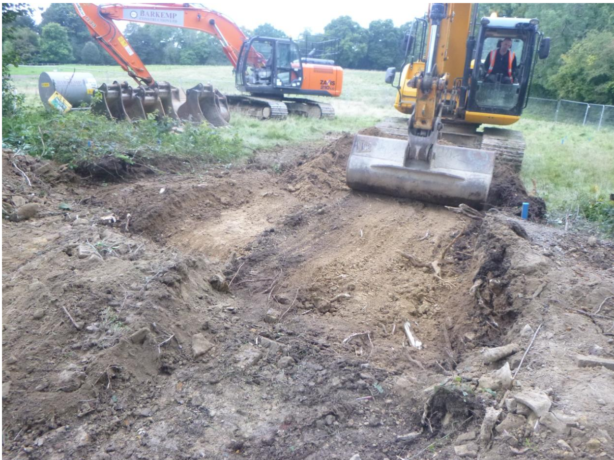
Plate 4: Breaching the hedgerow (looking south)
