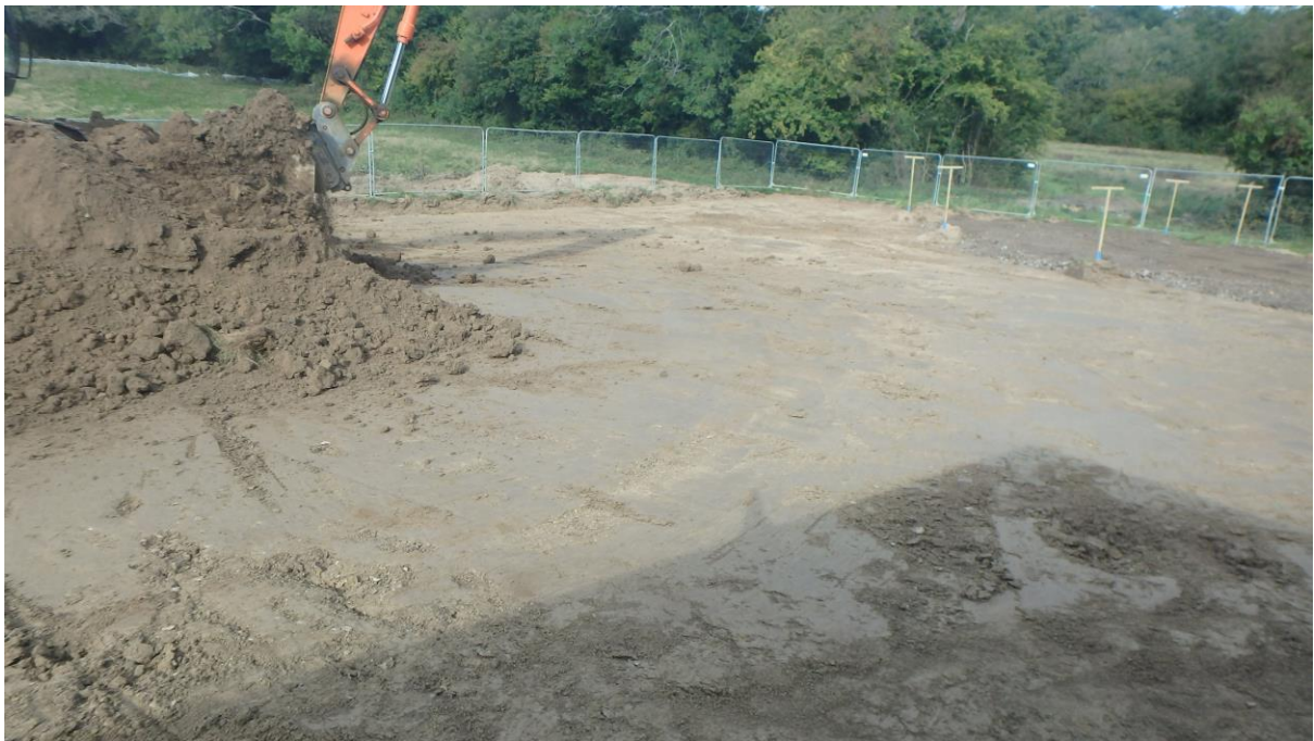
Plate 2: Stripping the compound area (looking north)
