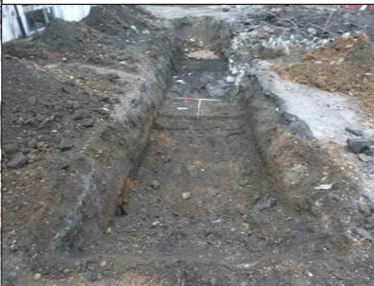
Trench 6 with asbestos sondage, looking east
