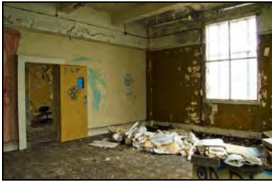
RER16-0068 G9 - Overview. Facing north-west
