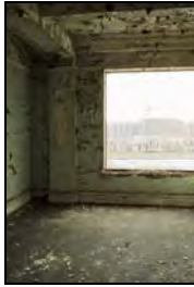
RER16-0196 S2 - Overview. Facing north
