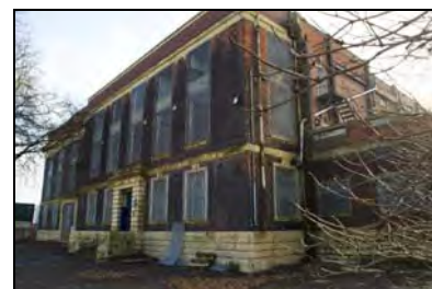
RER16-0012 North Elevation -. Facing south-east
