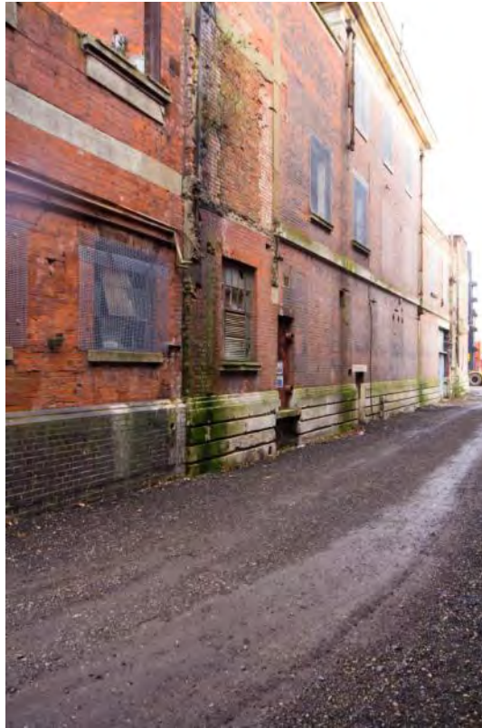
Plate 11: South elevation of the Control Room Building (#RER16-234)
