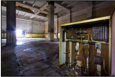
RER16-0241 Control Room F15 - Overview. Facing north-west
