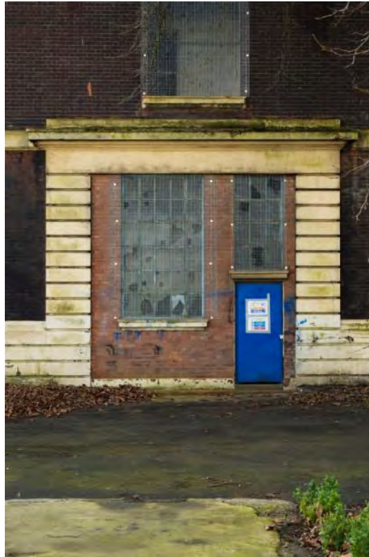
Plate 9: Bricked-up opening with window and door in the north elevation (#RER16-0009)
