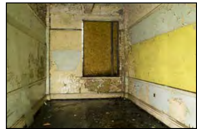
RER16-0159 F8 - Overview. Facing east
