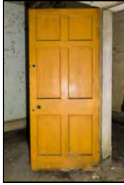
RER16-0163 F9 - Door. Facing south-west
