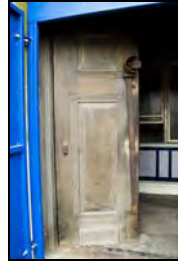
RER16-0044 North Elevation - Main door detail. Facing south
