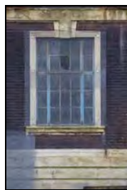
RER16-0224 North Elevation - Window. Facing south
