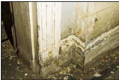
RER16-0169 F10 - Architrave detail. Facing east
