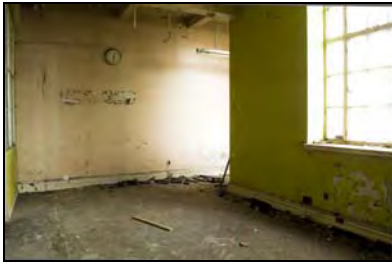
RER16-0059 G6 - Overview. Facing west
