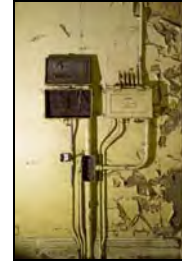
RER16-0165 F11 - Overview. Facing south
