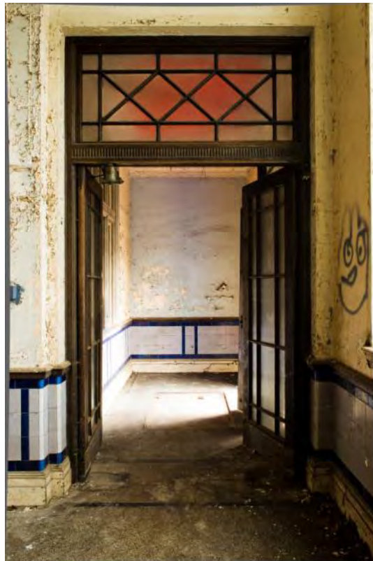
Plate 24: Lobby doors, seen from the hallway (G2) (#RER16-0052)
