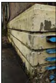
RER16-0037 South Elevation - Plinth Detail. Facing west
