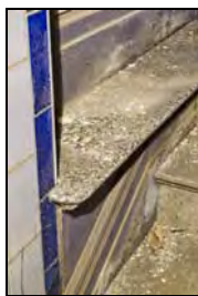
RER16-0209 Main Stair/Corridor - Granolithic floor detail. Facing east
