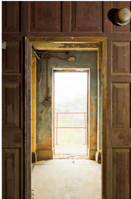
Plate 83: Panelled surround and second-floor egress (#RER16-0200)
