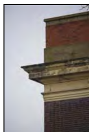
RER16-0227 North Elevation - Entablature/Parapet detail. Facing south-east
