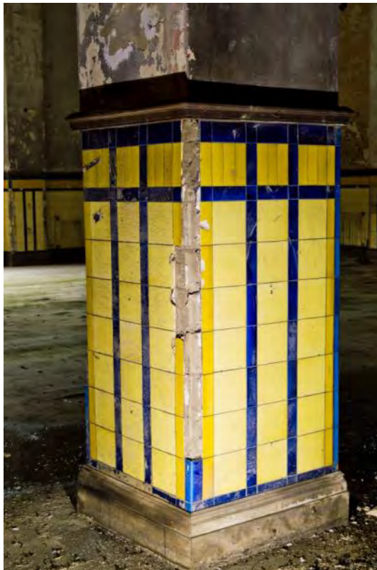
Plate 76: Detail of tiling on pier within the Control Room (#RER16-0123)
