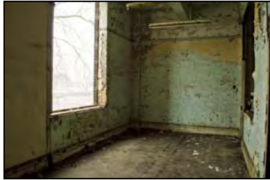
RER16-0151 F5 - Overview. Facing east
