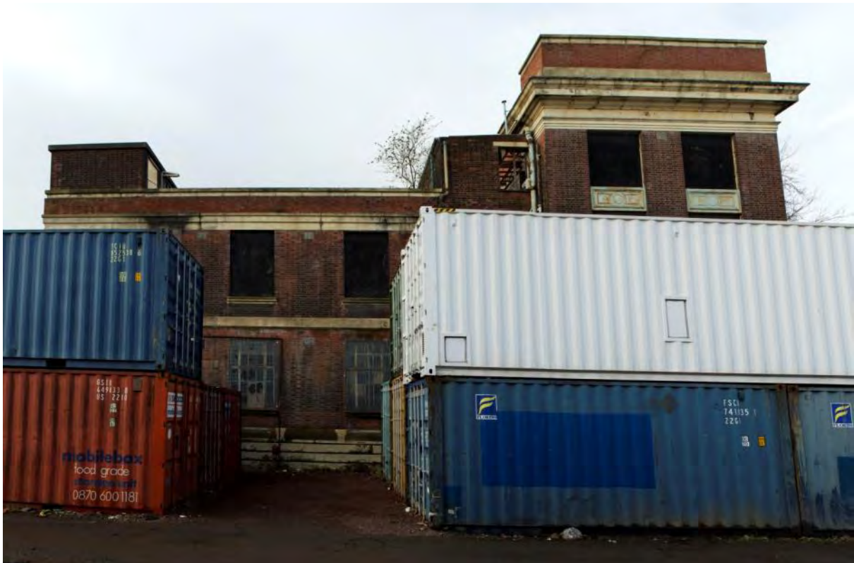
Plate 10: East elevation of the Control Room Building (#RER16-0033)
