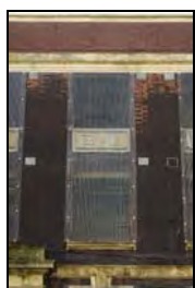
RER16-0007 North Elevation - Window. Facing south
