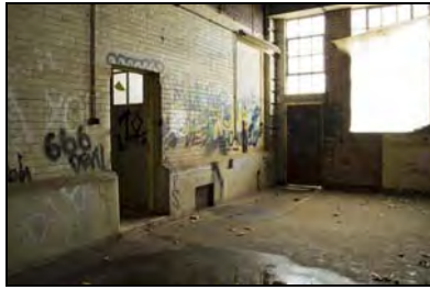
RER16-0063 G7 - Overview. Facing north-west
