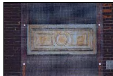
RER16-0228 North Elevation - Spandrel detail. Facing south
