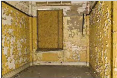
RER16-0166 F10 - Overview. Facing east
