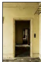
RER16-0096 G5 Telephone Exchange - Doorway east. Facing east
