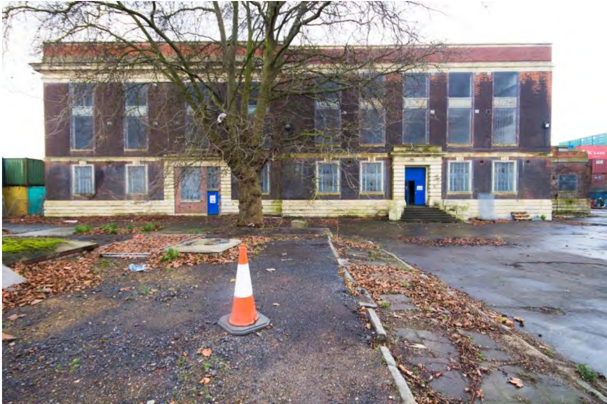
Plate 3: North elevation of the Control Room Building (#RER16-0229)
