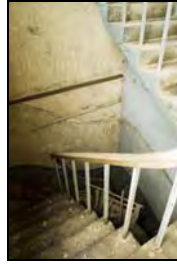
RER16-0179 Secondary Stair. Facing south-west
