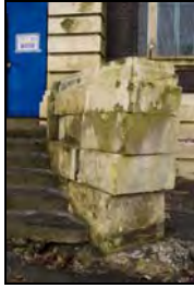
RER16-0043 North Elevation - Wall to principal doorway. Facing south
