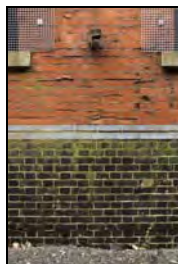
RER16-0039 South Elevation - Switch House plinth and brickwork. Facing north
