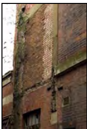
RER16-0038 South Elevation - Blocked opening to former bridge. Facing west
