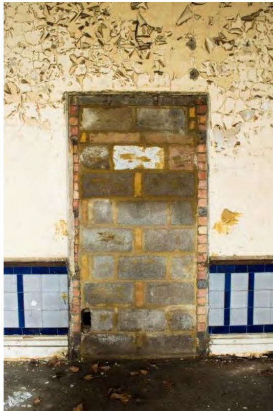
Plate 26: Blocked doorway from the hallway to Room G13 (#RER16-0053)
