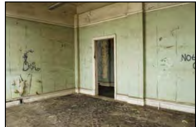
RER16-0114 F3 - Overview. Facing south-east
