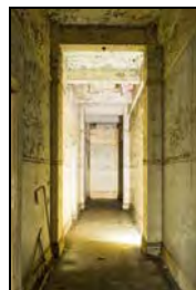
RER16-0161 Corridor. Facing south
