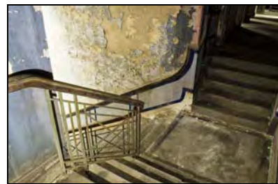
RER16-0204 Main Stair. Facing north-east
