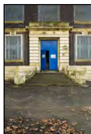
RER16-0005 North Elevation - Entrance. Facing south
