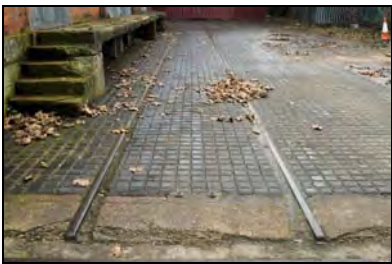
RER16-0041 West Elevation - Former railway siding. Facing south
