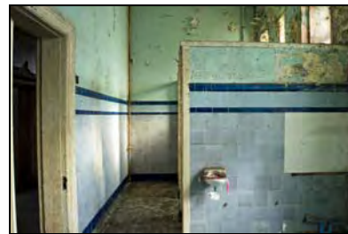
RER16-0081 WC G11 - Overview. Facing east
