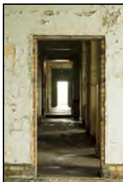
RER16-0157 F7 - Removed architrave and skirting. Facing west
