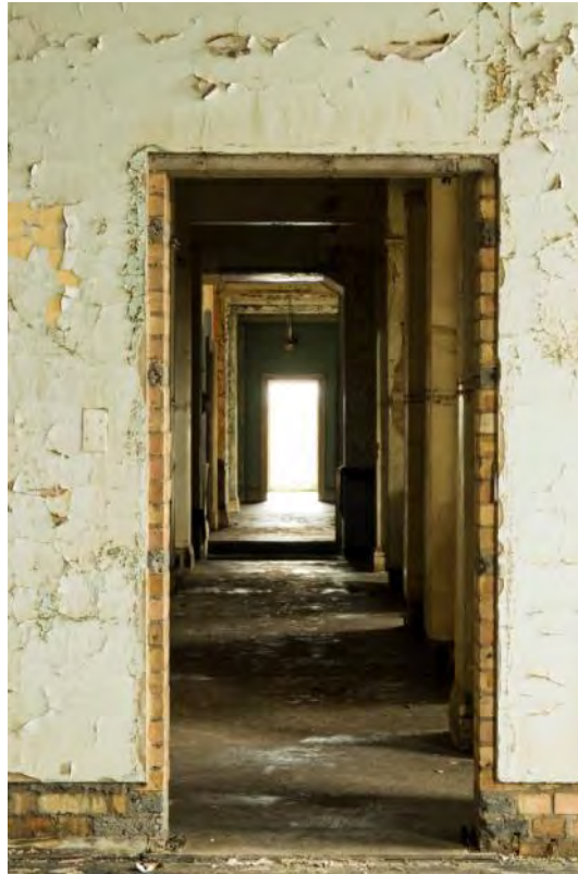
Plate 63: Stripped architrave and skirting from west wall of Room F7 (#RER16-0157)
