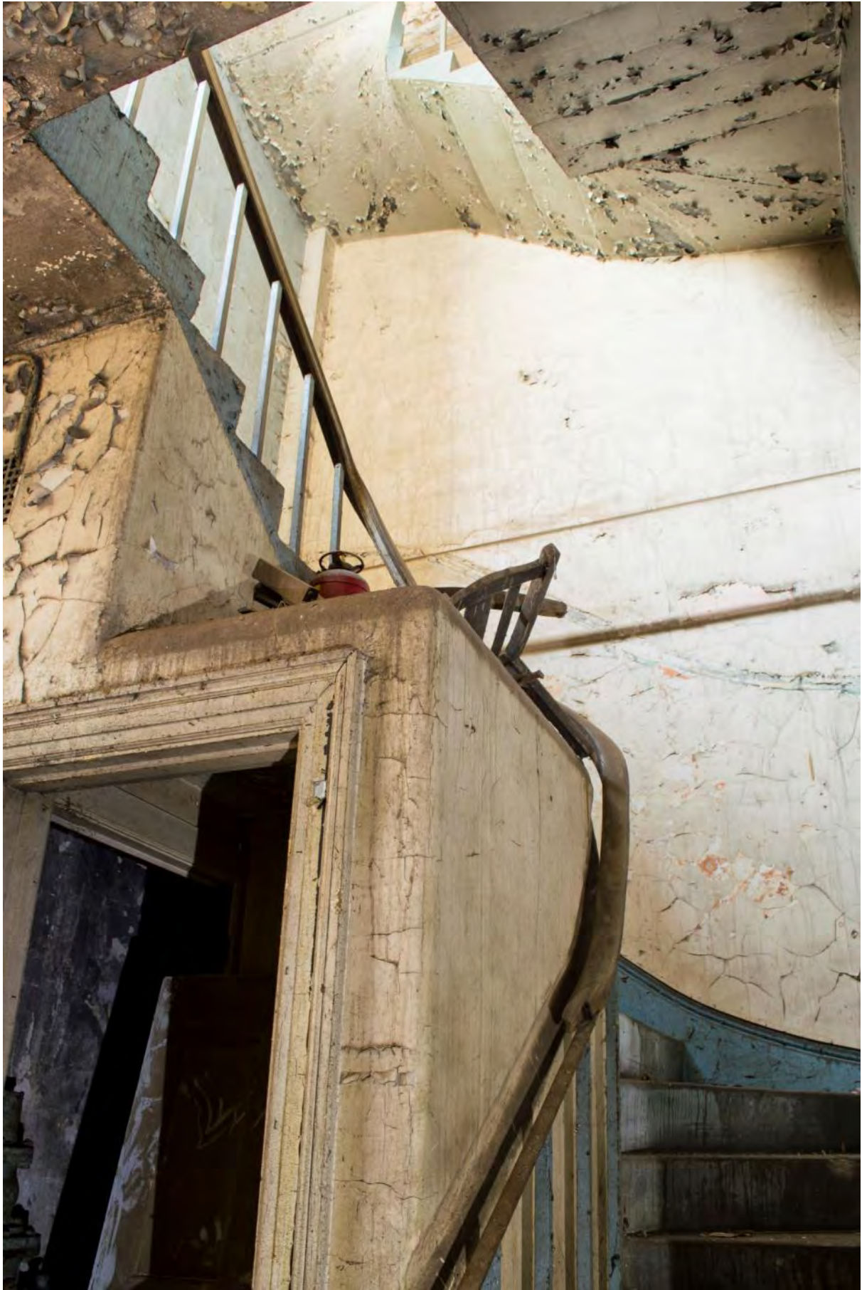
Plate 45: Secondary stair (#RER16-0079)
