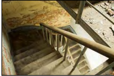
RER16-0182 Secondary Stair. Facing south-west
