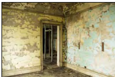
RER16-0215 S6 - Overview. Facing south-east
