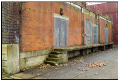
RER16-0042 West Elevation - Former railway siding and platform. Facing south-east
