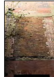
RER16-0021 South Elevation - Blocked opening to former bridge. Facing north
