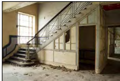
RER16-0056 G2 - Main Stair. Facing north-east
