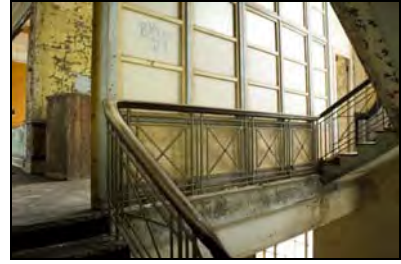
RER16-0105 F1 - Screen. Facing north-west
