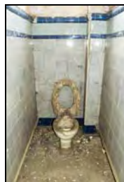
RER16-0176 WC F12 - Toilet. Facing south
