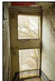
RER16-0206 Main Stair - Windows. Facing north
