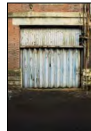
RER16-0027 South Elevation - Concertina door. Facing north
