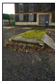
RER16-0008 Plinth - External. Facing south
