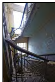
RER16-0248 Main Stair. Facing north
