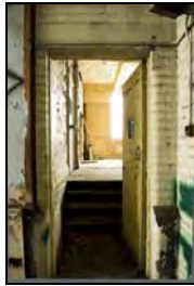
RER16-0065 G7 - Doorway to G8. Facing east
