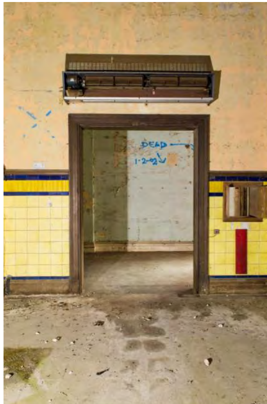
Plate 78: Doorway south from the Control Room (#RER16-0137)
