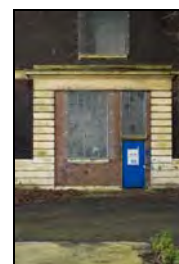
RER16-0009 North Elevation - Blocked opening for former siding. Facing south
