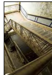
RER16-0207 Main Stair. Facing north-east
