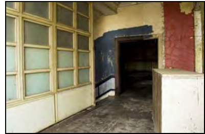
RER16-0108 F1 - Overview. Facing south-east
