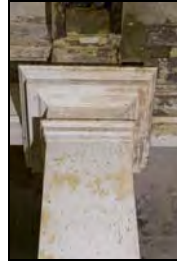
RER16-0134 Control Room F15 - Trim detail. Facing east
