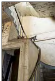
RER16-0079 Secondary Stair. Facing south-east
