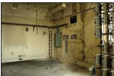
RER16-0095 G5 Telephone Exchange - Overview. Facing south-west
