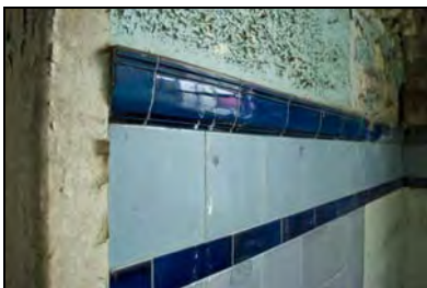
RER16-0083 WC G11 - Tiling detail. Facing south-east
