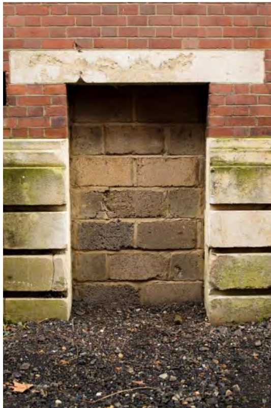
Plate 14: Low blocked opening in the south elevation (#RER16-0024)
