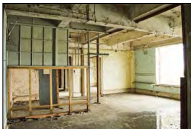
RER16-0218 S7 - Overview. Facing west
