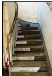
RER16-0080 Secondary Stair. Facing south
