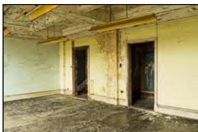
RER16-0191 S1 - Overview. Facing south-east
