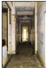
RER16-0170 Corridor. Facing north
