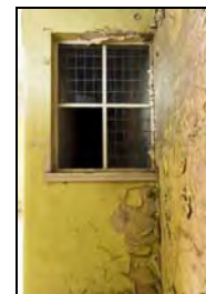
RER16-0144 Light to blocked stair. Facing west
