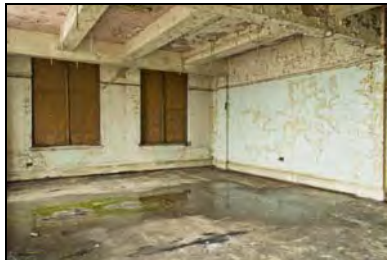
RER16-0155 F7 - Overview. Facing south-east
