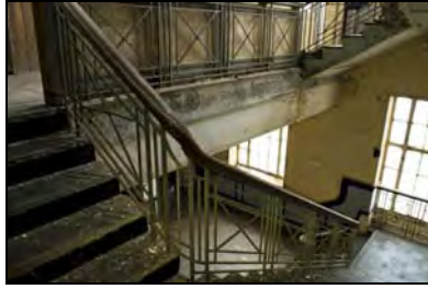
RER16-0104 Main Stair. Facing north-west
