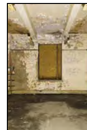
RER16-0162 F9 - Overview. Facing east
