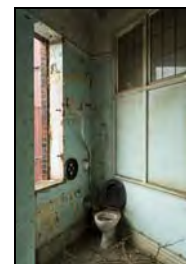
RER16-0147 F14 - Overview. Facing west
