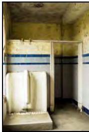
RER16-0199 WC S4 - Overview. Facing north
