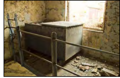
RER16-0180 Secondary Stair - Water tank and platform. Facing south-west
