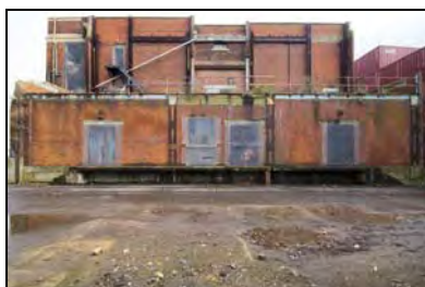
RER16-0230 West Elevation. Facing east
