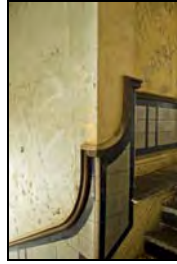
RER16-0149 Main Stair/Corridor - Dado detail. Facing north-east
