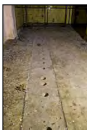
RER16-0131 Control Room F15 - Plant footing. Facing south
