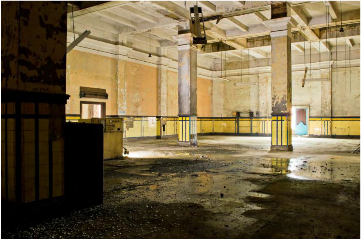
Plate 73: The Control Room F15 (#RER16-0128)
