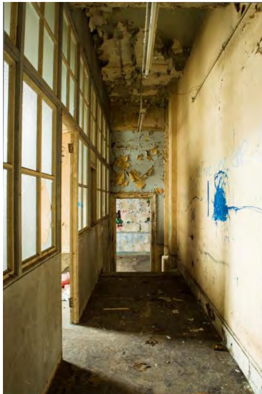
Plate 34: Corridor east of the hallway (#RER16-0058)
