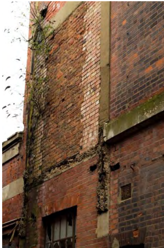
Plate 16: Blocked first-floor doorway and projecting steelwork of a former bridge (#RER16-0038)
