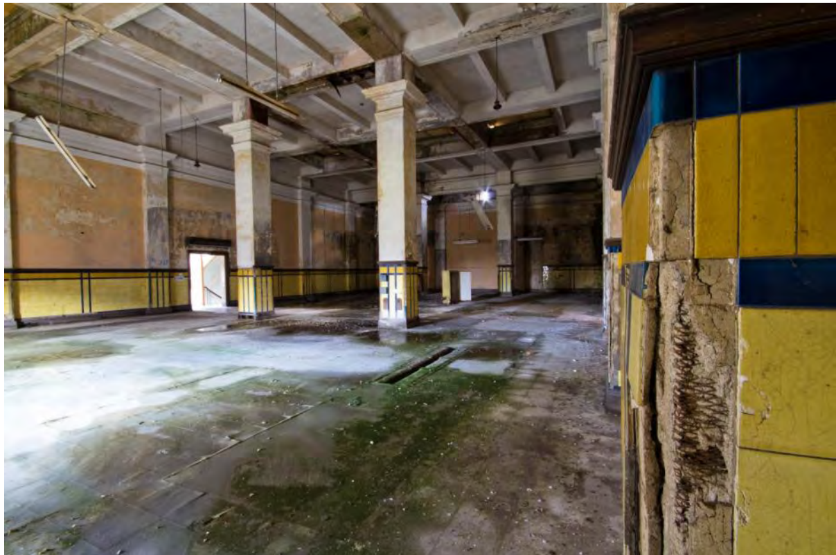
Plate 74: The Control Room F15 (#RER16-0240)
