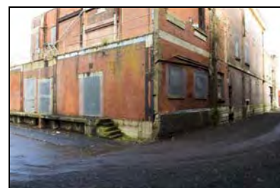
RER16-0015 West and South Elevations. Facing north-east
