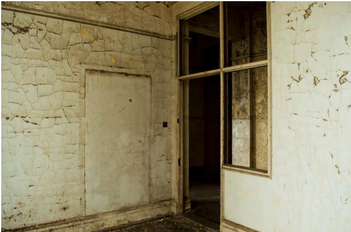
Plate 58: Room F6 – note the blocked doorway to Room F7 (#RER16-0154)
