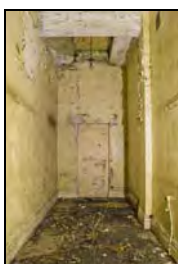
RER16-0130 F16 - Overview. Facing south
