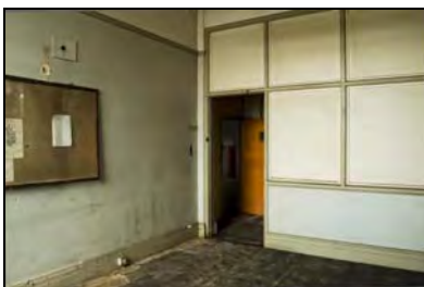
RER16-0089 G4 - Overview. Facing south-east
