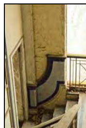
RER16-0188 Main Stair. Facing north
