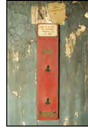
RER16-0195 Corridor - former fire extinguisher mount. Facing south
