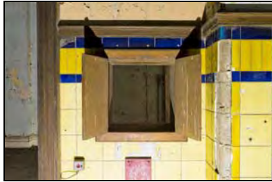
RER16-0136 Control Room F15 - Opening detail. Facing south
