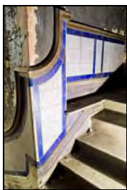
RER16-0208 Main Stair/Corridor - Dado detail. Facing north
