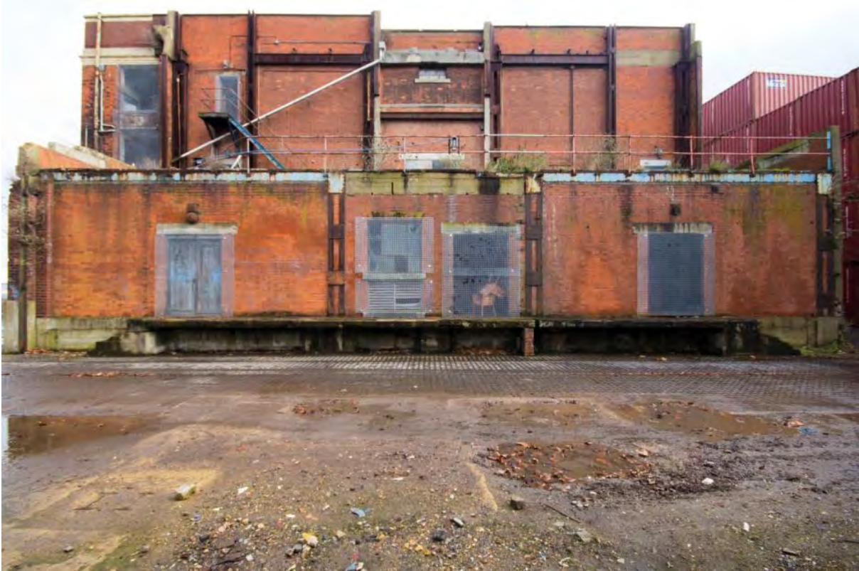
Plate 18: West elevation of the Control Room Building (#RER16-230)
