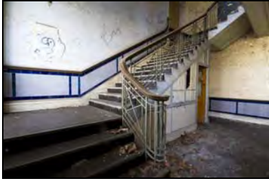
RER16-0238 G2 - Main Stair. Facing south-east
