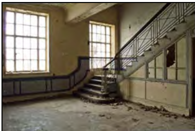
RER16-0055 G2 - Overview. Facing north-east
