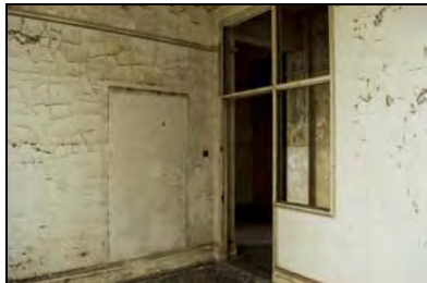
RER16-0154 F6 - Overview. Facing south-east
