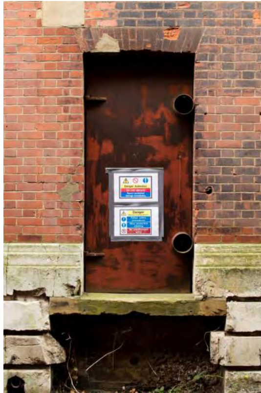
Plate 15: Opening to the west side of the south elevation (#RER16-0023)
