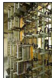
RER16-0093 G5 Telephone Exchange - Relay. Facing south-west
