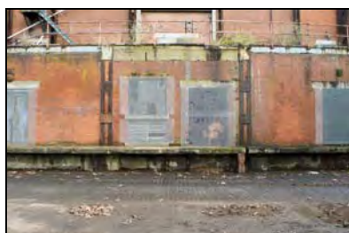
RER16-0013 West Elevation -. Facing east
