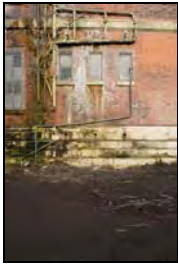
RER16-0029 South Elevation - WC windows. Facing north
