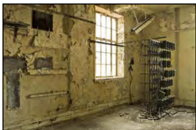
RER16-0091 G5 Telephone Exchange - Overview. Facing north-west
