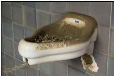
RER16-0172 WC F12 - Fitting. Facing north-west
