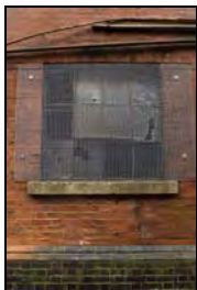
RER16-0040 South Elevation - Switch House window. Facing north
