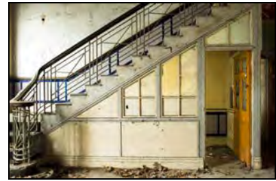
RER16-0054 G2 - Stair Cupboard. Facing east
