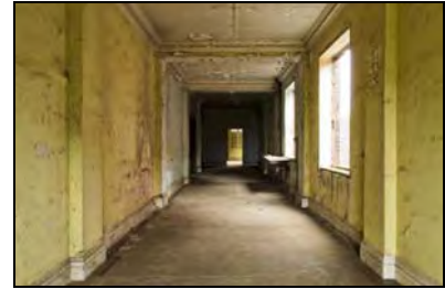
RER16-0138 F13 - Overview. Facing east
