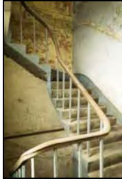
RER16-0178 Secondary Stair. Facing south-west
