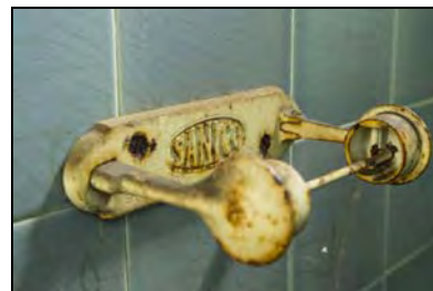
RER16-0084 WC G11 - Fitting. Facing south-east
