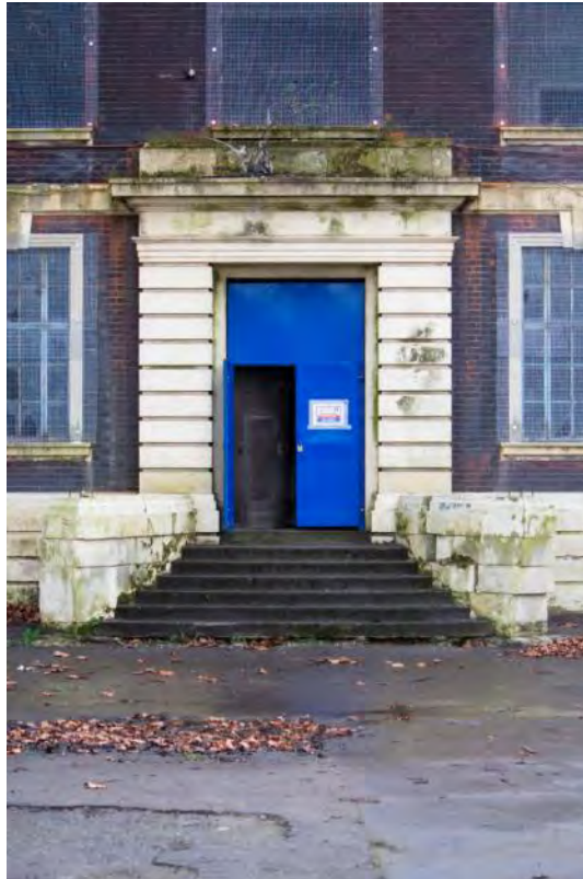
Plate 5: Main entrance to the building (#RER16-0225)
