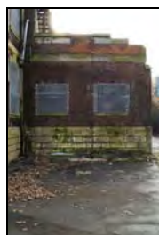
RER16-0011 North Elevation - truncated switch house. Facing south
