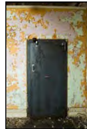
RER16-0072 G10 - Safe. Facing south
