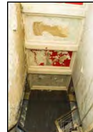
RER16-0186 Main Stair - Coffered ceiling. Facing south
