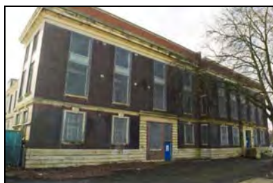
RER16-0010 North Elevation. Facing south-west
