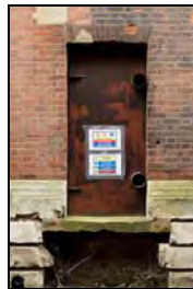
RER16-0023 South Elevation - Doorway. Facing north
