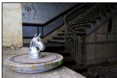
RER16-0004 G2. Facing south-east
