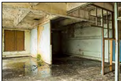
RER16-0217 S7 - Overview. Facing south-east
