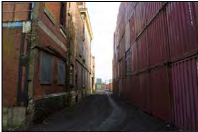
RER16-0019 Circulation south of the building. Facing east
