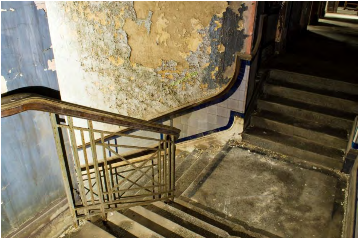
Plate 29: Top of the stairs, second floor (#RER16-204)
