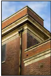
RER16-0028 South Elevation - Entablature detail. Facing north-west
