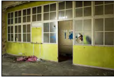
RER16-0060 G6 - Overview. Facing south-east
