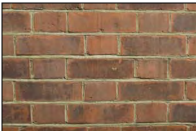
RER16-0025 South Elevation - Brick detail. Facing north
