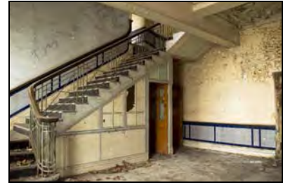
RER16-0048 G2 - Overview. Facing south-east
