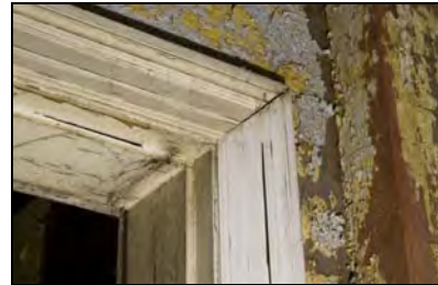
RER16-0168 F10 - Architrave detail. Facing east
