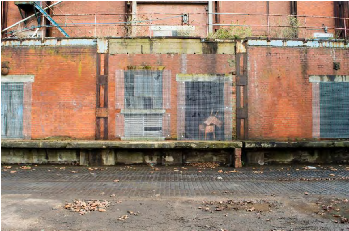
Plate 49: Sealed openings to Rooms G14- G 16 (#RER16-0013)
