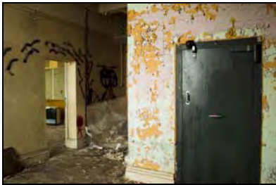
RER16-0071 G10 - Overview. Facing south-east
