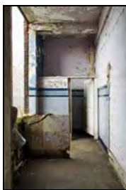
RER16-0118 WC F4 - Overview. Facing north
