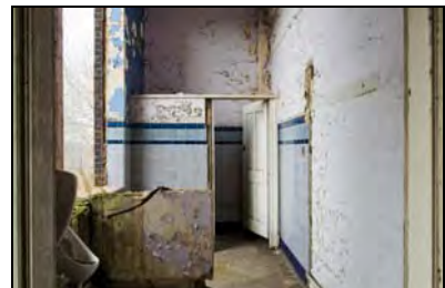
RER16-0117 WC F4 - Overview. Facing north
