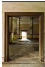
RER16-0140 F13/F15 - Dooway north to Control Room. Facing north
