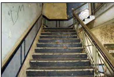
RER16-0101 G1 - Main Stair. Facing south
