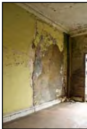
RER16-0139 F13 - Blocked opening to former bridge. Facing south-west
