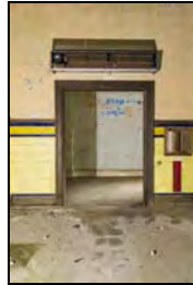
RER16-0137 Control Room F15 - Doorway south. Facing south
