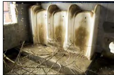
RER16-0171 WC F12 - Urinal. Facing south-west
