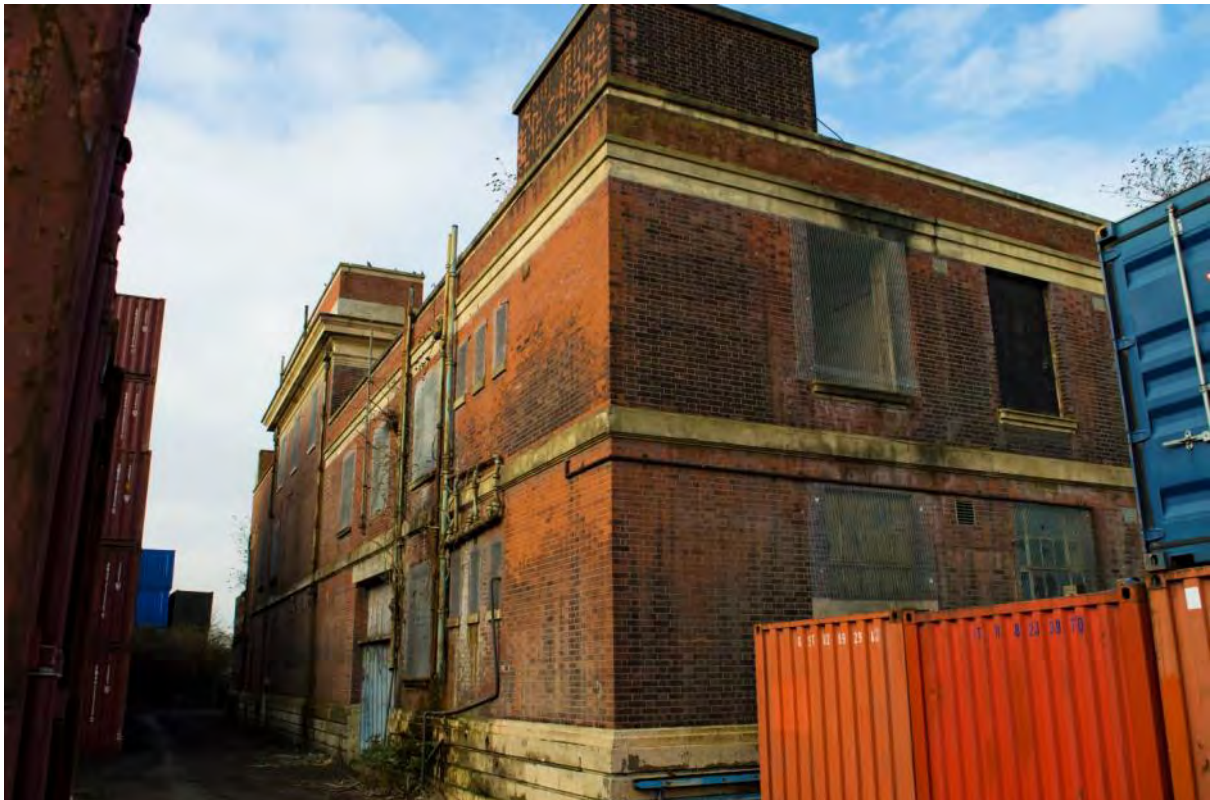
Plate 12: South elevation of the Control Room Building (#RER16-0031)
