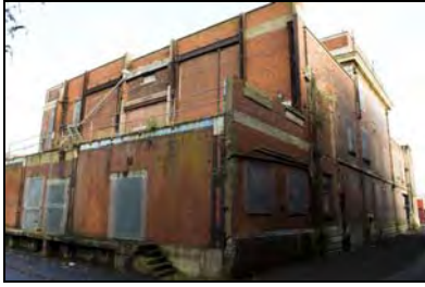
RER16-0016 West and South Elevations. Facing north-east
