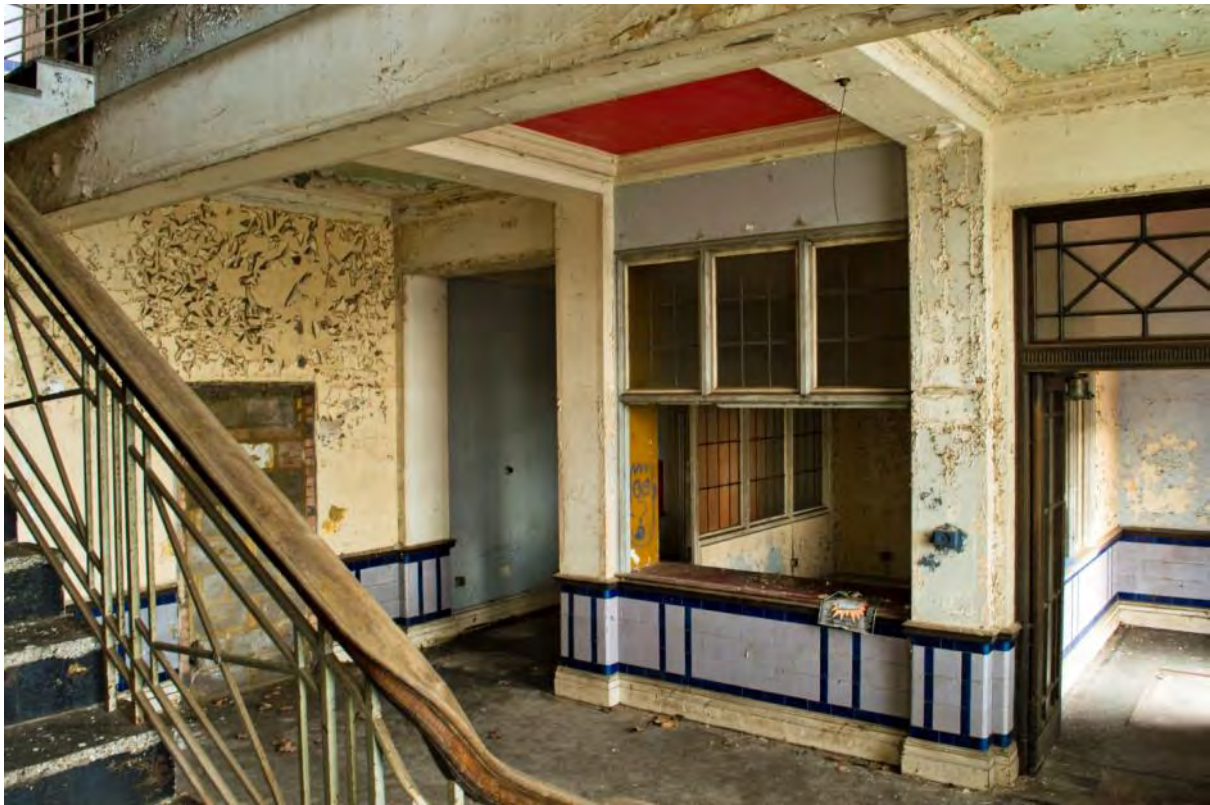
Plate 25: Overview of the hallway (G2) seen from the main stair (#RER16-0102)
