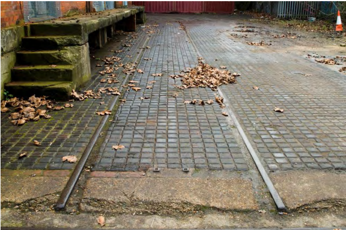
Plate 19: Remnant railway sidings adjacent to the west elevation (#RER16-0041)
