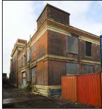
RER16-0017 East and South Elevations. Facing west
