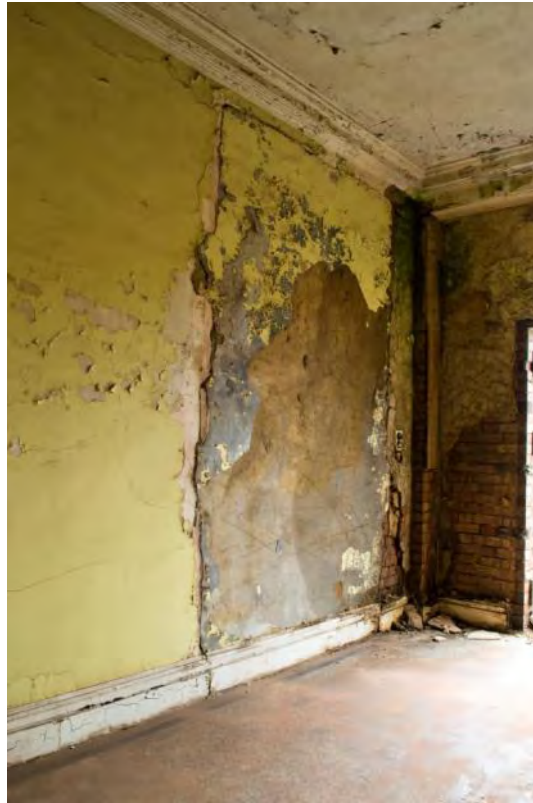
Plate 69: Blocked doorway to the presumed bridge south from Room F13 (#RER16-0139)
