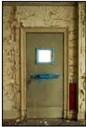
RER16-0067 G8 - Doorway to G10. Facing north
