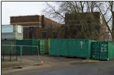
RER16-0034 Phase B Switch Houses. Facing east
