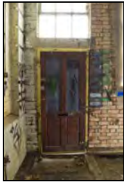
RER16-0061 G7 - Inserted door. Facing north
