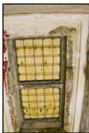
RER16-0223 Skylight. Facing west
