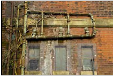
RER16-0030 South Elevation - WC windows. Facing north
