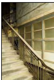
RER16-0187 Main Stair. Facing south-west
