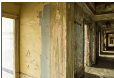
RER16-0203 Corridor. Facing north-east
