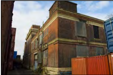
RER16-0031 East and South Elevations. Facing north- west
