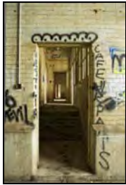
RER16-0064 G7 - Doorway to corridor. Facing west
