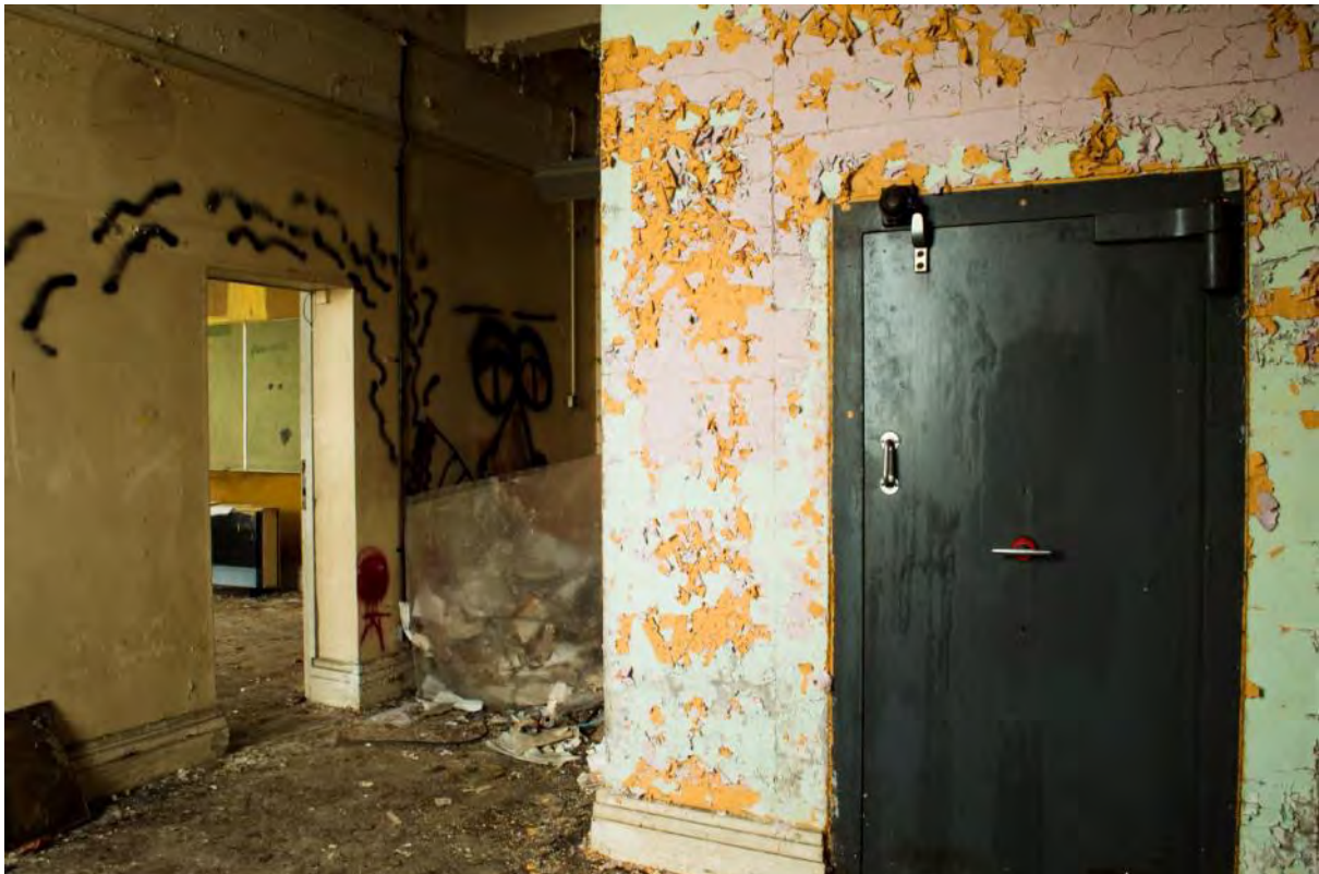
Plate 40: Room G10, with the safe to the right (#RER16-0071)
