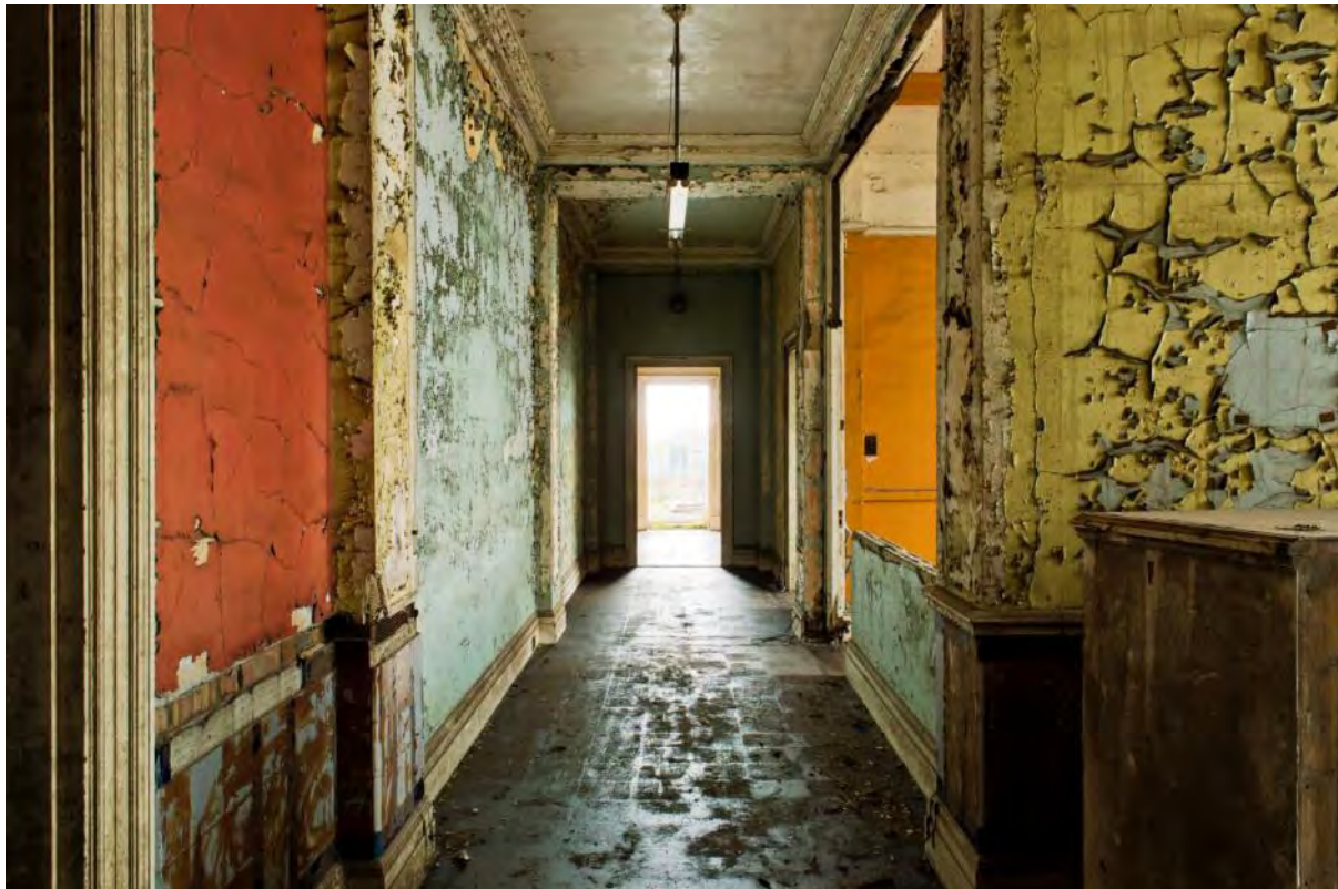
Plate 52: Corridor west of the landing (#RER16-0109)
