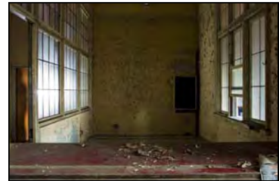
RER16-0051 G3 - Overview. Facing west
