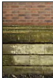
RER16-0026 South Elevation - Plinth and brick detail. Facing north
