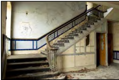
RER16-0049 G2 - Main Stair. Facing south-east
