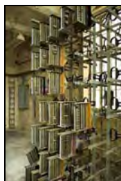
RER16-0092 G5 Telephone Exchange - Relay. Facing south-west
