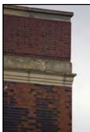
RER16-0226 North Elevation - Cornice/Parapet detail. Facing south-west
