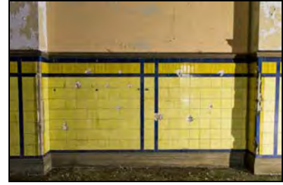
RER16-0135 Control Room F15 - Tiling detail. Facing south
