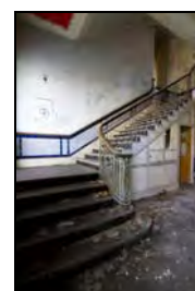
RER16-0237 G2 - Main Stair. Facing south-east
