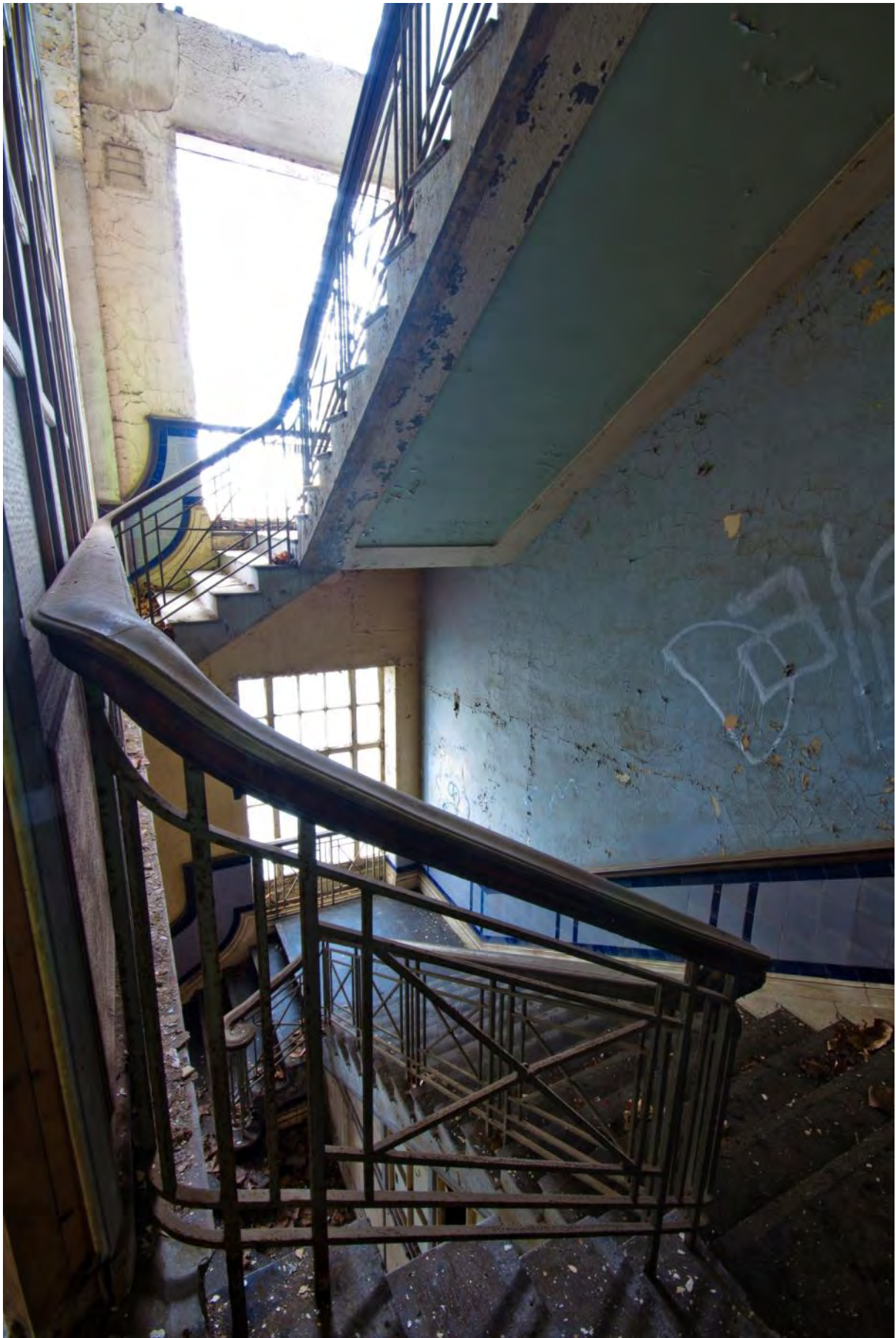
Plate 28: Main stair, from the first floor landing (#RER16-0248)
