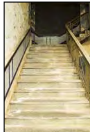
RER16-0185 Main Stair. Facing south
