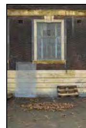
RER16-0006 North Elevation - Window. Facing south
