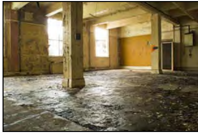
RER16-0066 G8 - Overview. Facing south-east
