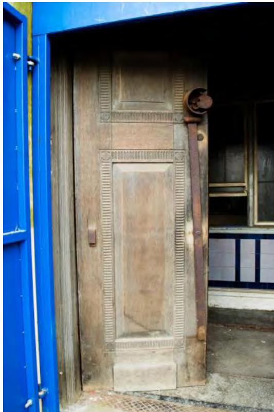
Plate 6: Door to the main entrance (#RER16-0044)
