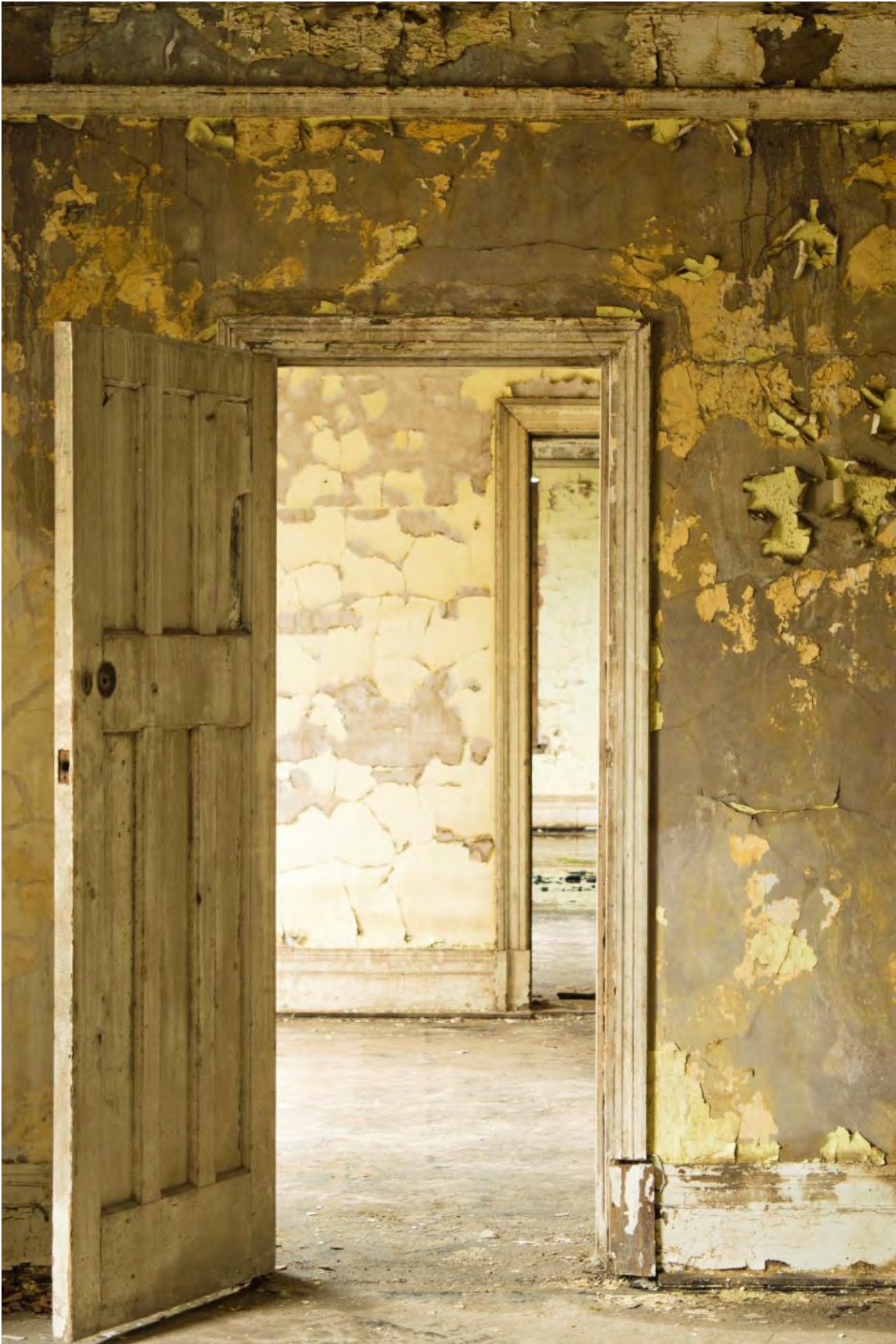
Plate 22: Typical architrave, door, skirting, and picture rail, east range, Room S5 (#RER16-214)
