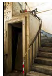
RER16-0078 Secondary Stair. Facing south-east
