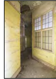
RER16-0243 Corridor - WC F14. Facing east
