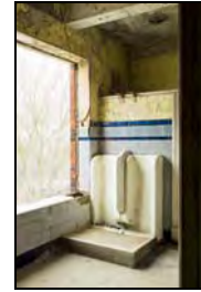
RER16-0198 WC S4 - Overview. Facing north-west
