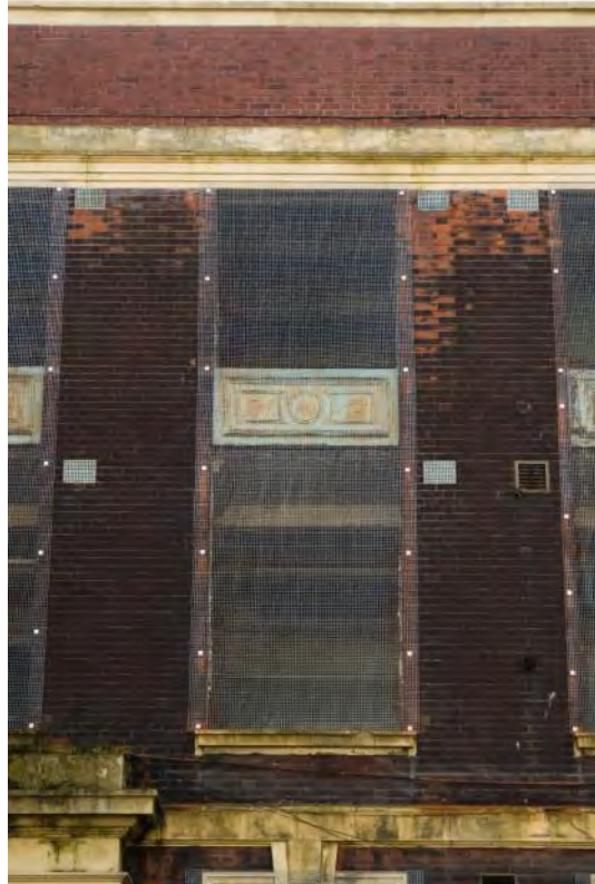
Plate 7: First and Second floor windows (#RER16-0007)
