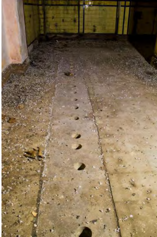
Plate 75: Concrete beds with channels for cabling in the Control Room (#RER16-0131)
