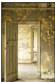
RER16-0214 S5 - Doorway to S6. Facing east
