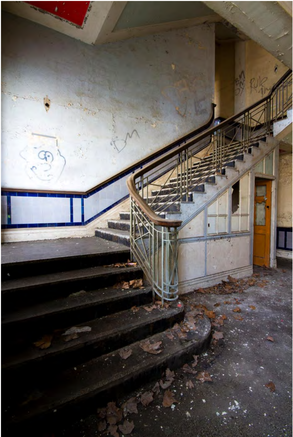
Plate 27: The main stair (#RER16-0237)
