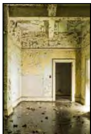
RER16-0160 F8 - Overview. Facing west
