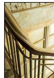
RER16-0189 Main Stair - Bannister Rail. Facing north-west
