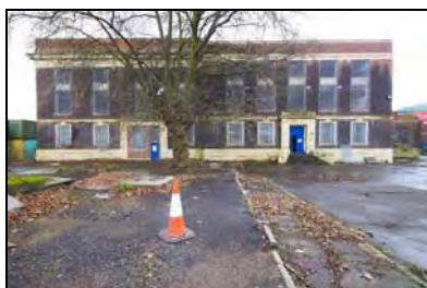
RER16-0229 North Elevation. Facing south
