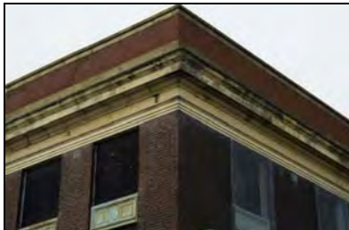
RER16-0036 North and East Elevations - Entablature detail. Facing south-west
