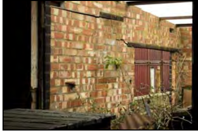
RER16-0181 Roof-space outbuilding. Facing south-west
