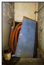
RER16-0086 Corridor - Blocked opening to G12. Facing west
