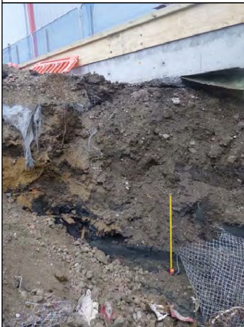
Photograph 3: View of section along south-eastern boundary showing silting fills 1000 and 1001 with 1m hand tape in yellow for scale
