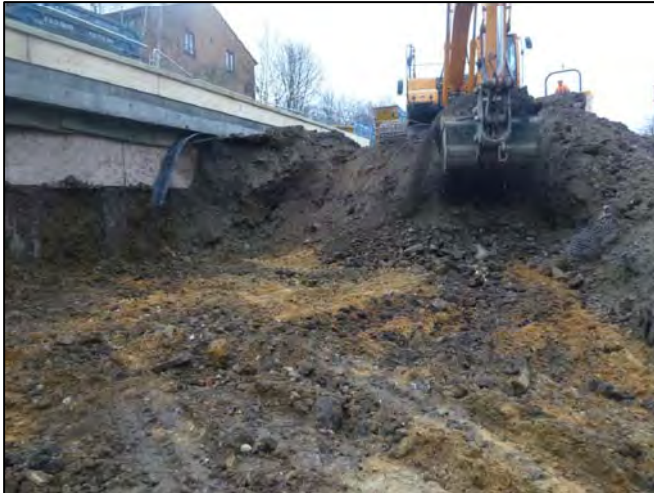
Photograph 1: View north into ground reduction
