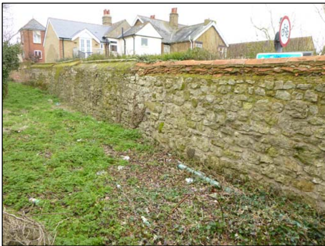
The extant precinct wall, interior looking north-east
