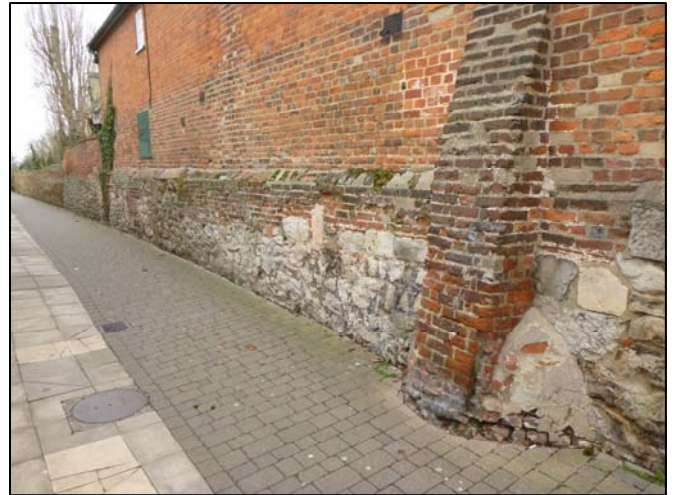
The extant precinct wall, exterior looking south-west
