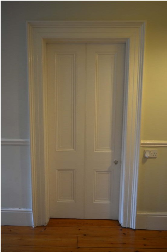
Plate 9: Door to ground floor south-west room, facing west (RLB17-0020)
