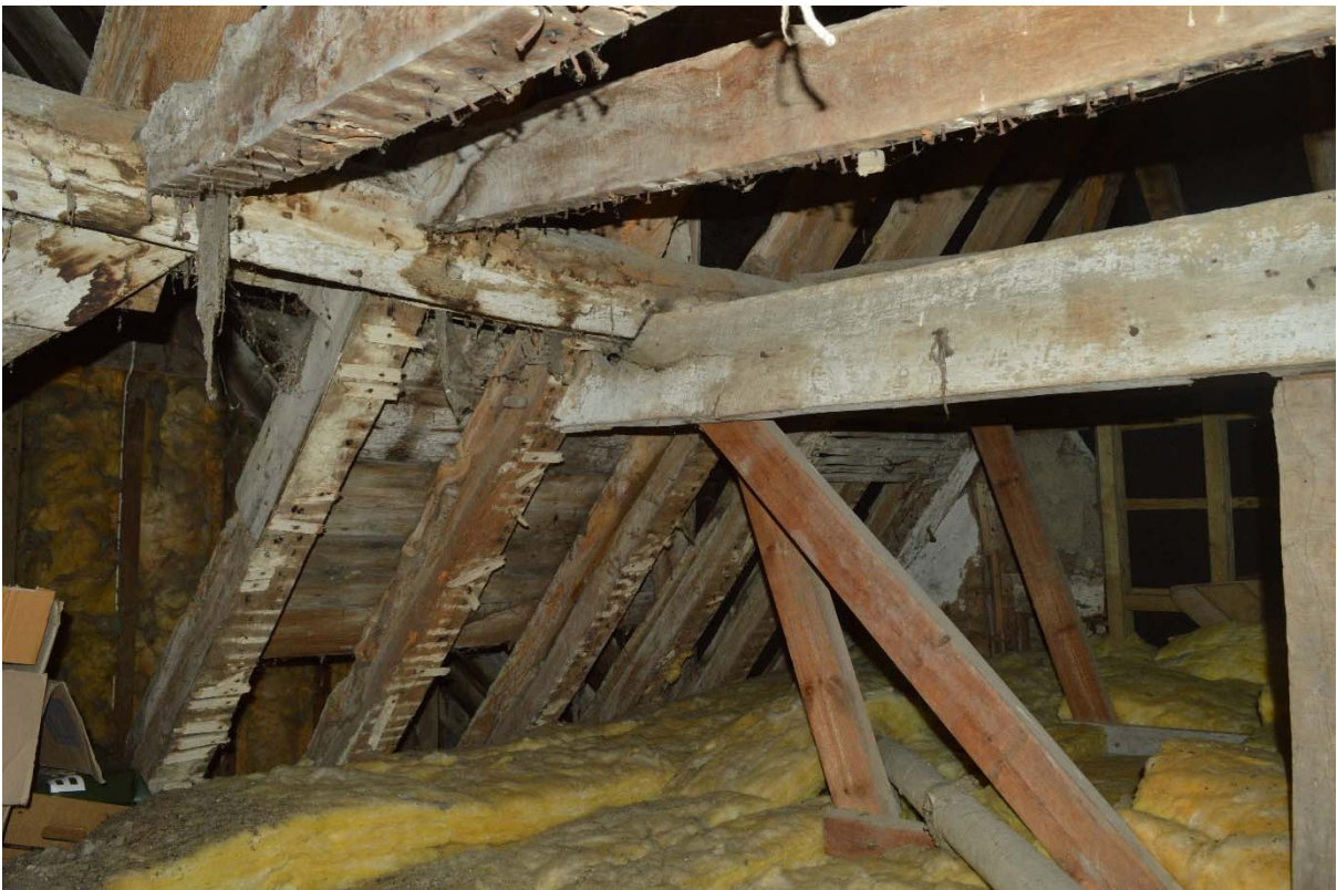
Plate 4: Remnants of lath and plaster in Bays 3 and 4 of roof (RLB17-0007)
