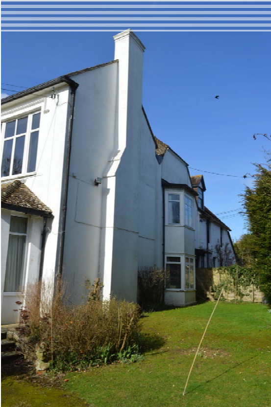
Plate 19: East elevation and bay window on rear range, facing north-east (RLB17-0070)
