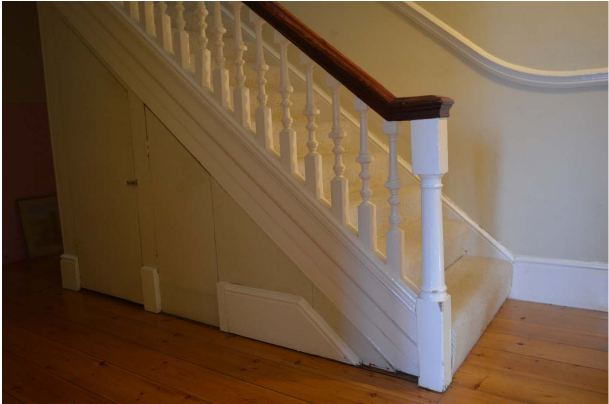
Plate15: Staircase, facing east (RLB17-0039)
