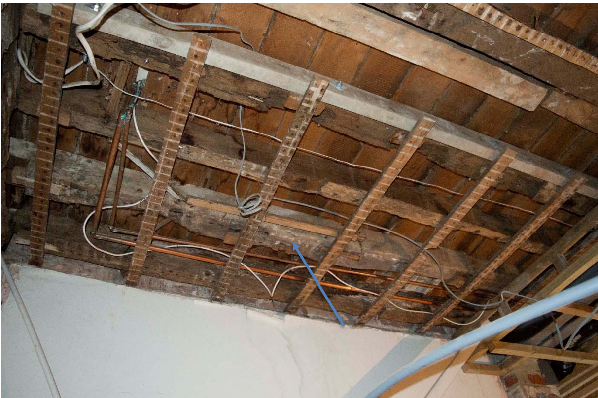
Plate A3.6: Joist with redundant stud mortices (RLB-0097)
