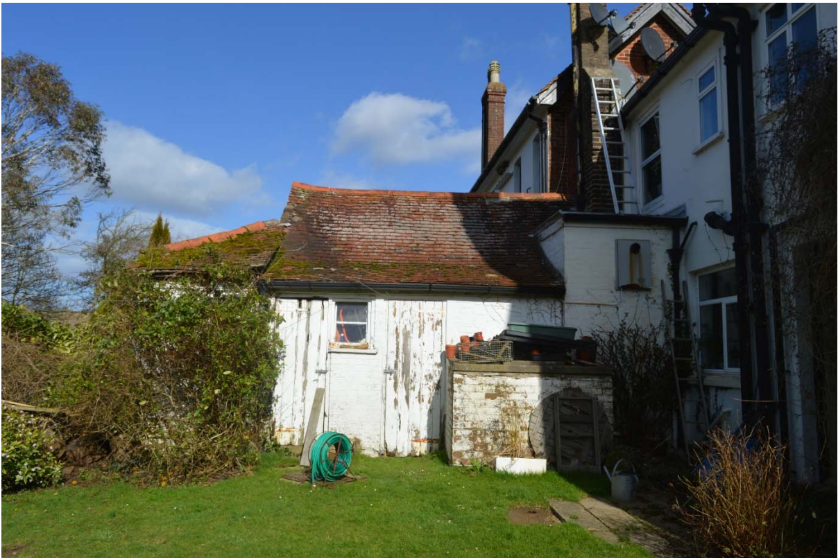
Plate 21: Outbuilding range, facing north (RLB17-0058)
