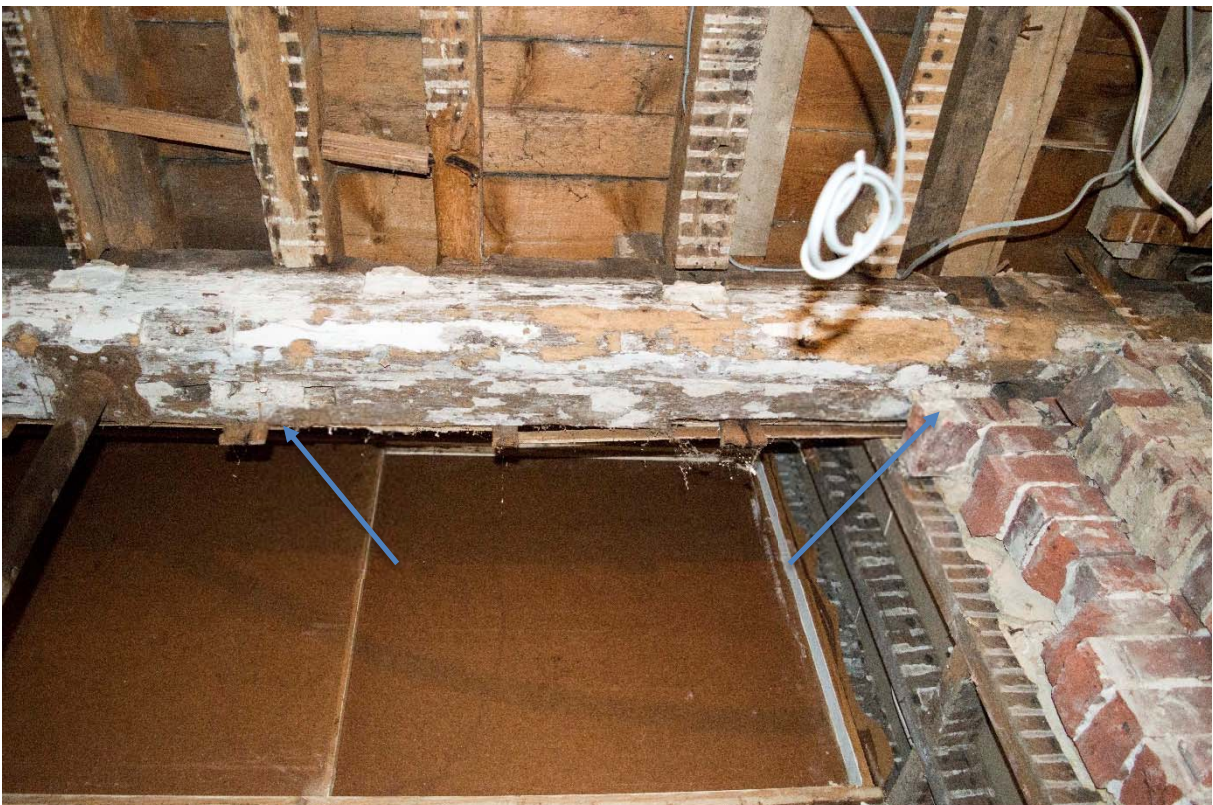
Plate A3.2: Redundant mortises for studs which formed the jambs of a doorway (RLB-0087)
