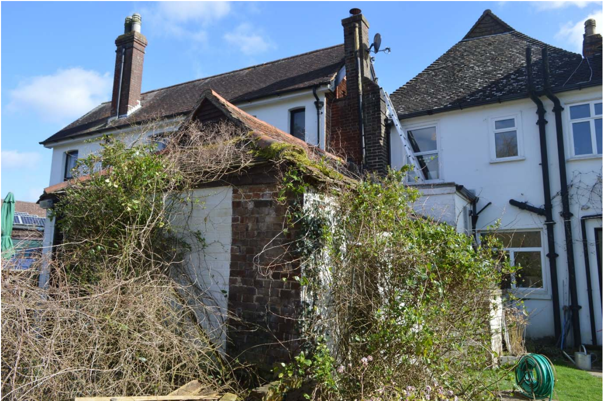
Plate 24: West end of outbuilding range, facing east (RLB17-0059)
