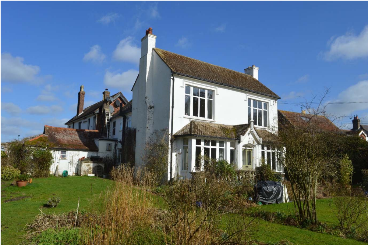
Plate 1: South and west elevations, facing north-east (RLB17-0055)
