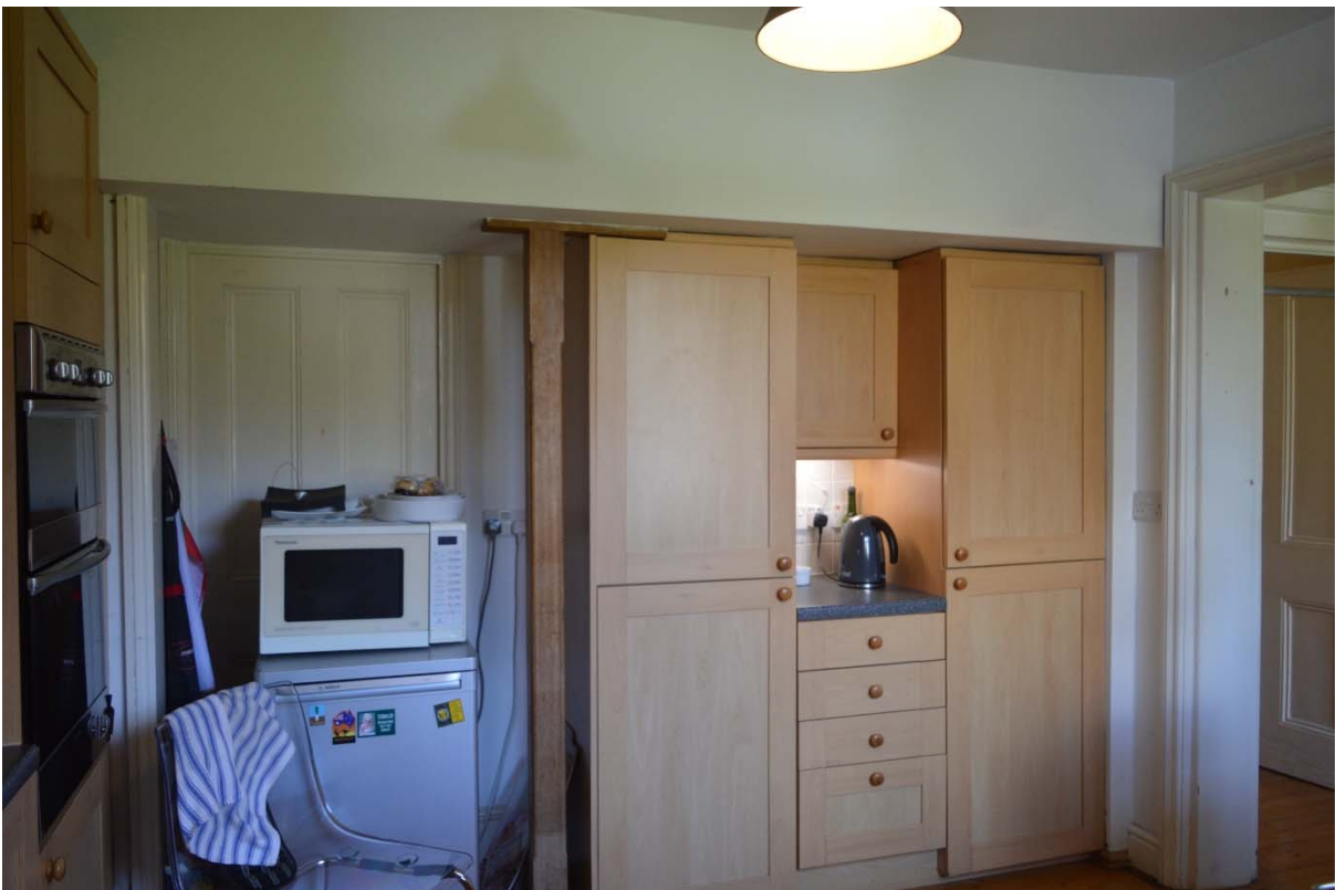
Plate 20: Reset wall in kitchen, facing east (RLB17-0030)
