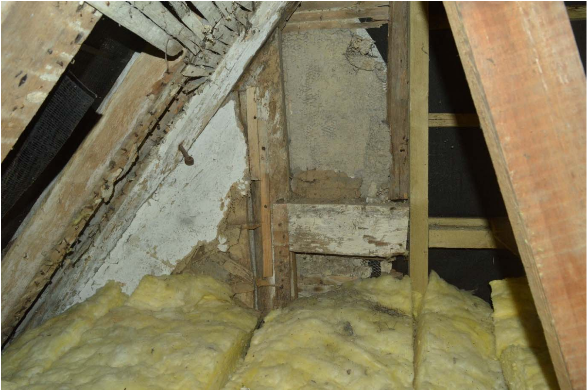
Plate 3: Small panel of daub in east wall of roof, facing east (RLB17-0078)
