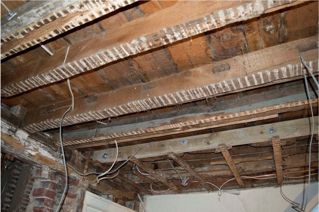
Plate A3.5: Joist with redundant stud mortices, turned through ninety degrees (RLB-0098)
