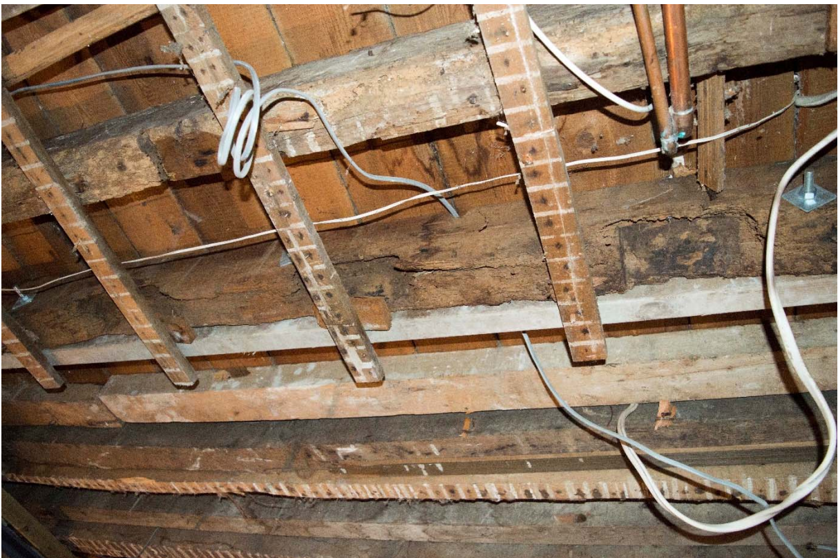
Plate A3.4: Joist formed by reused section of wallplate (RLB-0099)
