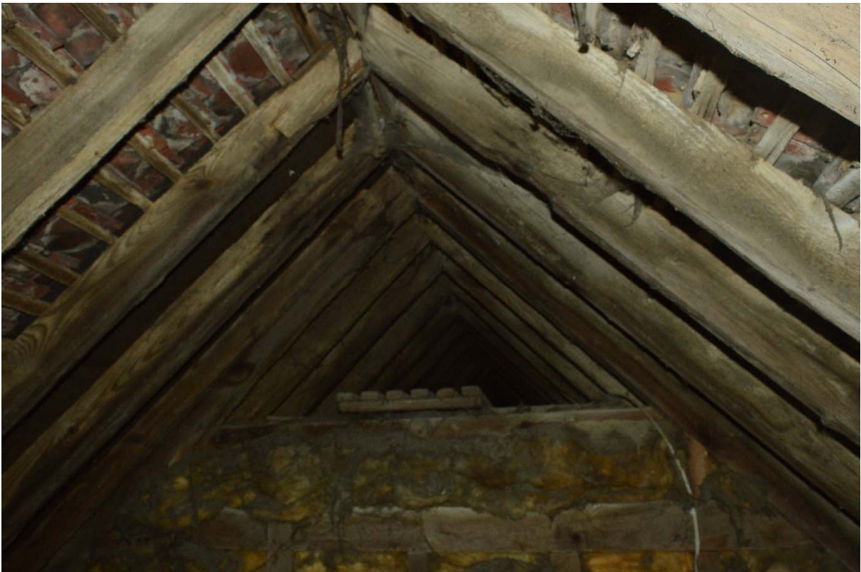
Plate 6: Roof of The Lawn Cottage, facing north (RLB17-0010)
