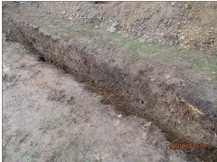
Photograph 5: trench looking south-east
