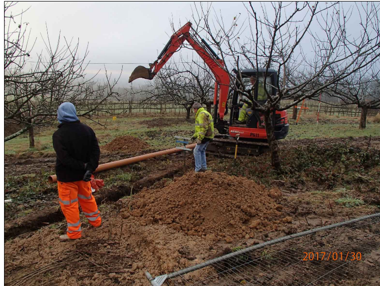
Photograph 3: trench looking south-east
