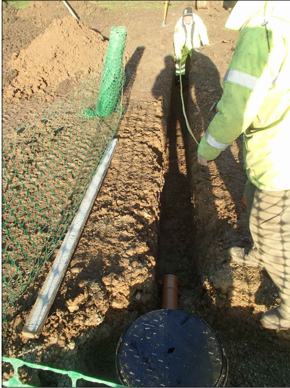
Photograph 1: trench looking north-east
