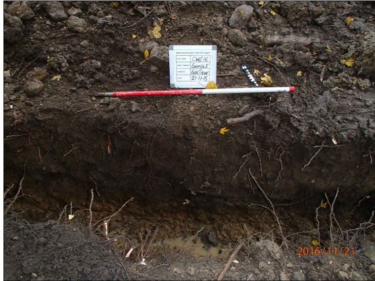
Photograph 4: trench looking north
