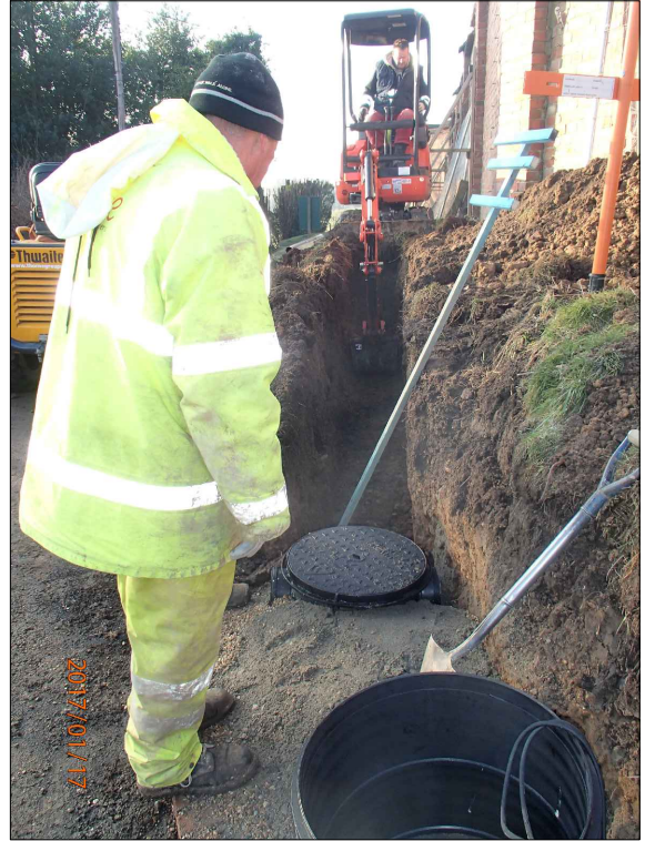
Photograph 2: trench looking north-east
