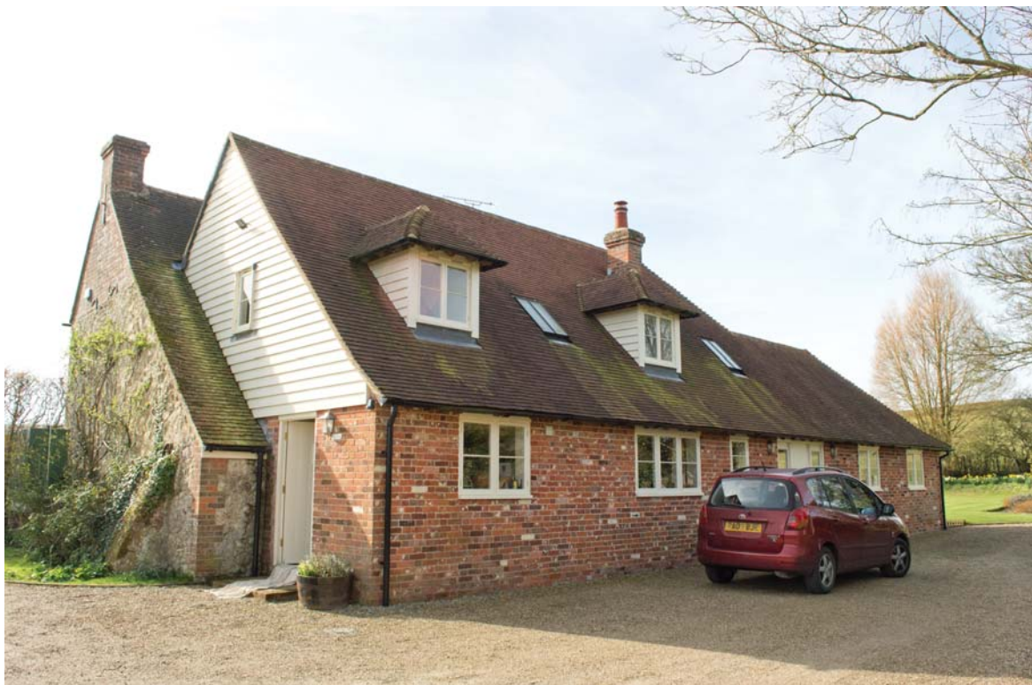
Rear elevation of the house, showing the later outshut and modern extension. View looking south-west
