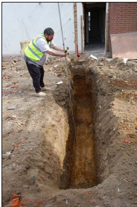
Building footings, south side looking east
