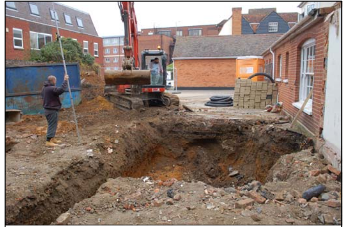
Building footings north-east corner, looking north
