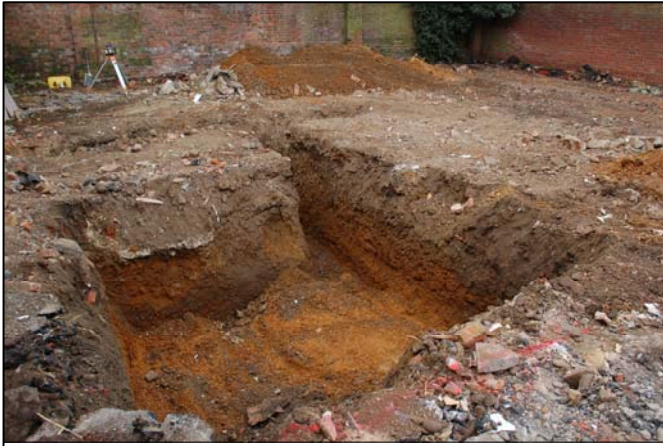
Building footings north-east corner, looking south-west
