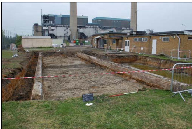
Area 3, looking south
