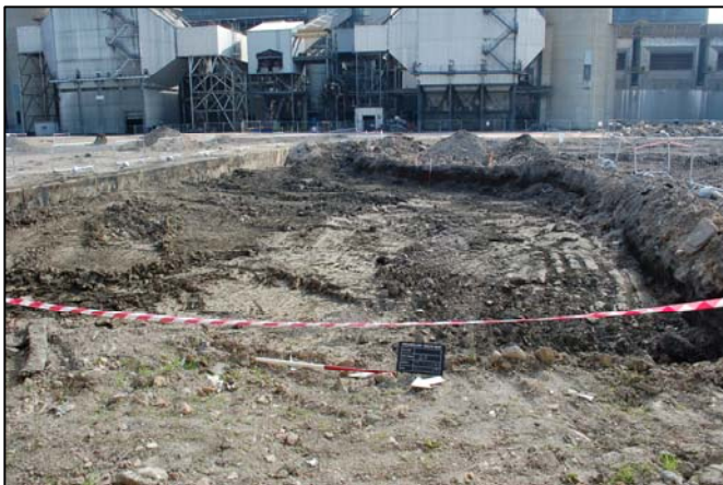
Area 2A, looking east
