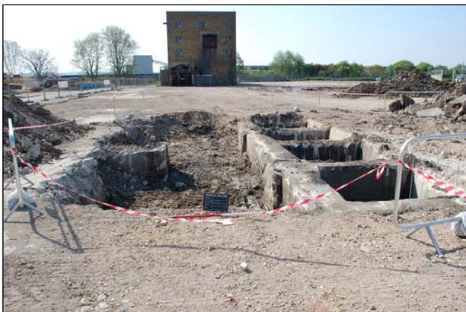
Area 2B, looking south
