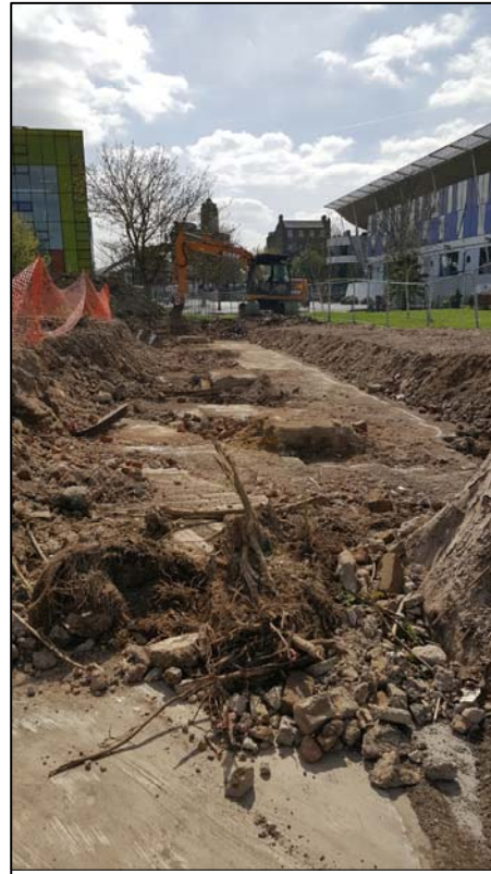
View north along the groundworks area
