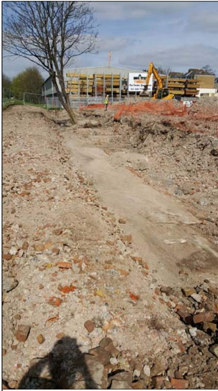
View north along the groundworks area
