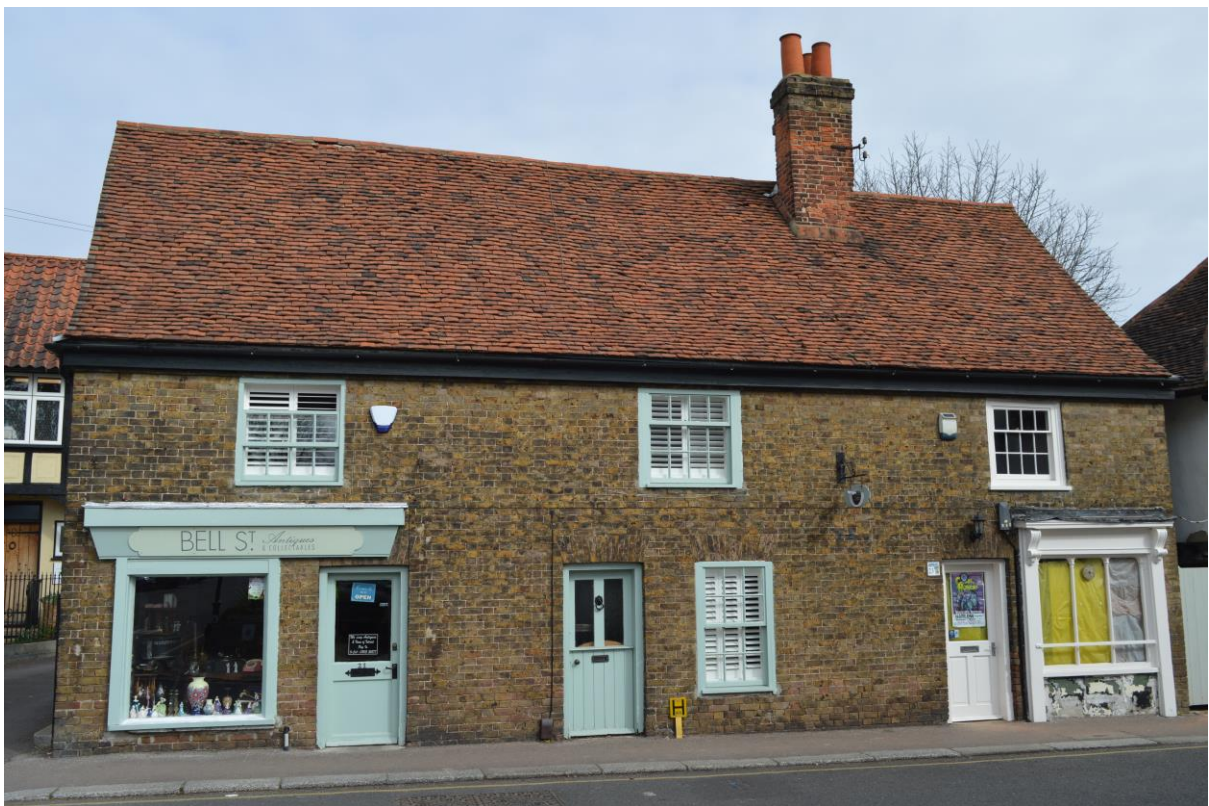
Plate 28: Brick façade on street frontage, facing north (BES-0021)
