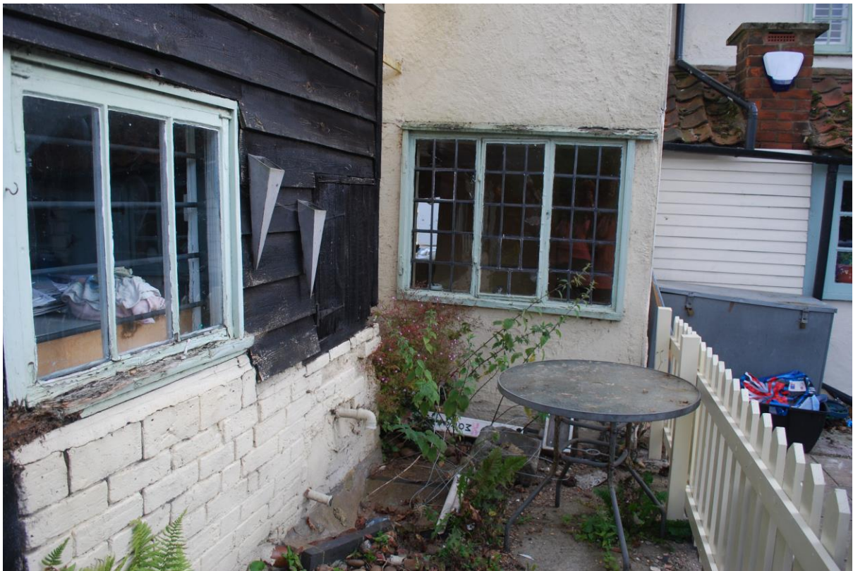
Plate 13: Three-light mullion window in north wall of rear wing, facing south (BES-120)
