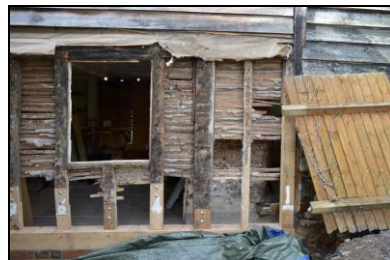
BES17-0036 Exposed wall framing of east elevation. Facing south-west
