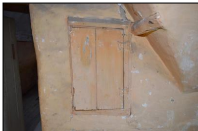
BES17-0110 Small hatch in attic. Facing north
