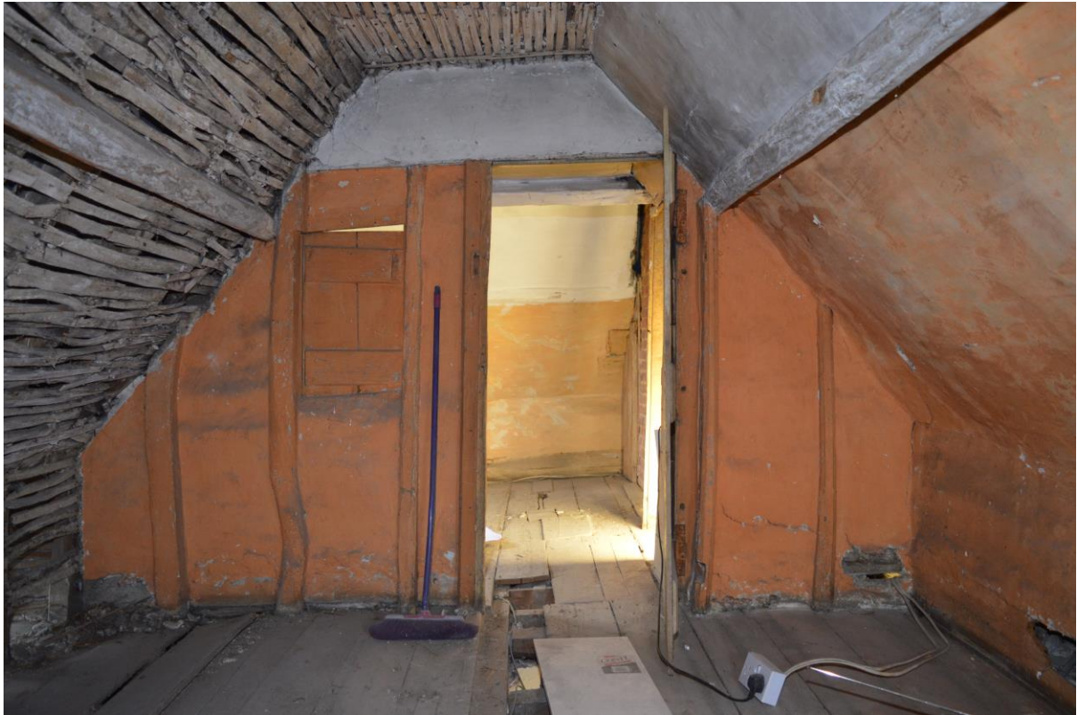
Plate 12: Lath and daub partition in attic, facing south (BES-0113)
