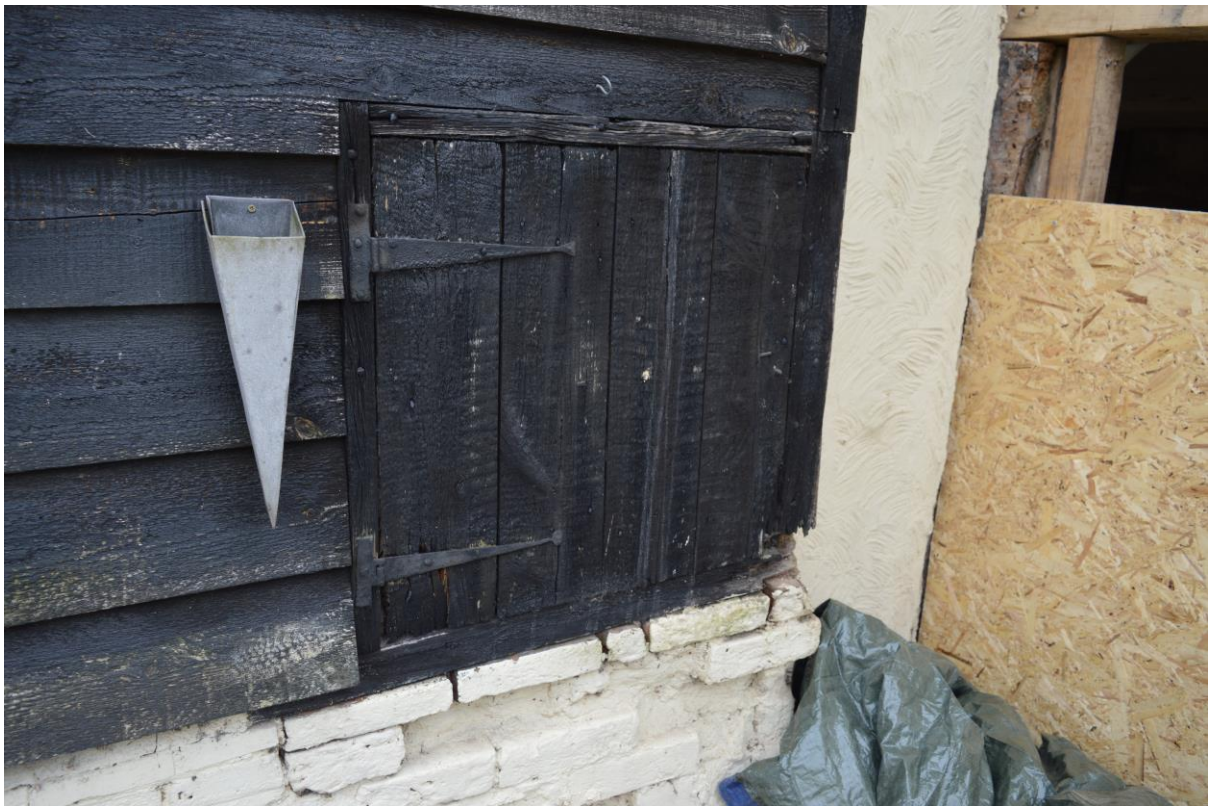
Plate 26: Plank and batten hatch in Phase 3 extension (BES-0031)
