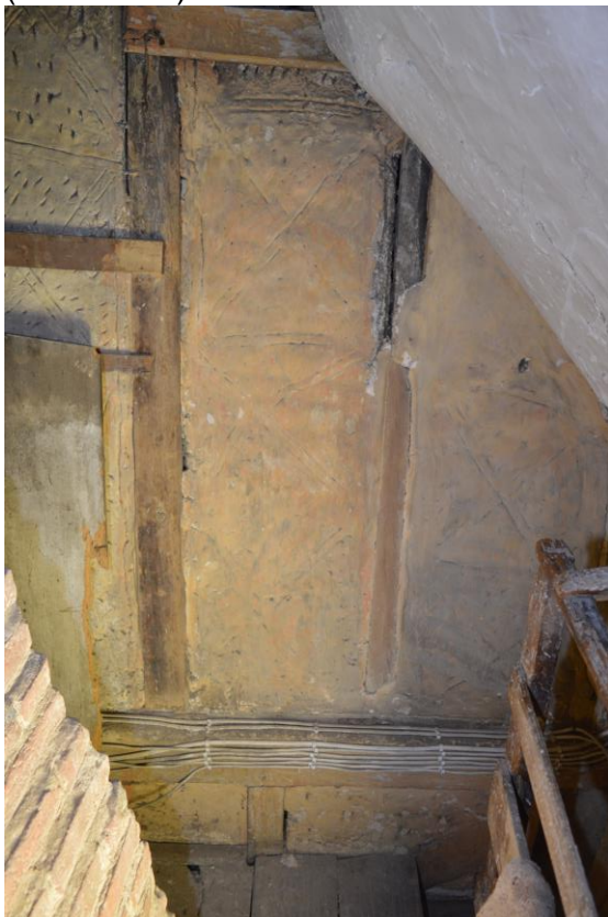
Plate 6: Daub panel with saltire patterns in high end partition, facing west (BES-0101)
