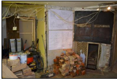
BES17-0046 Interior of ground floor south room. Facing west
