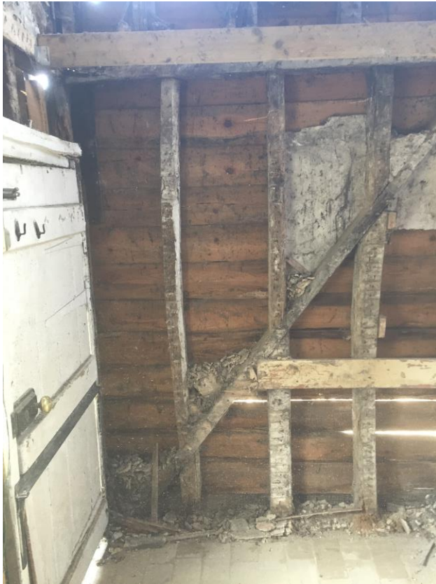
Plate 22: Wall framing of north wall of Phase 3 extension, facing north (BES-119)
