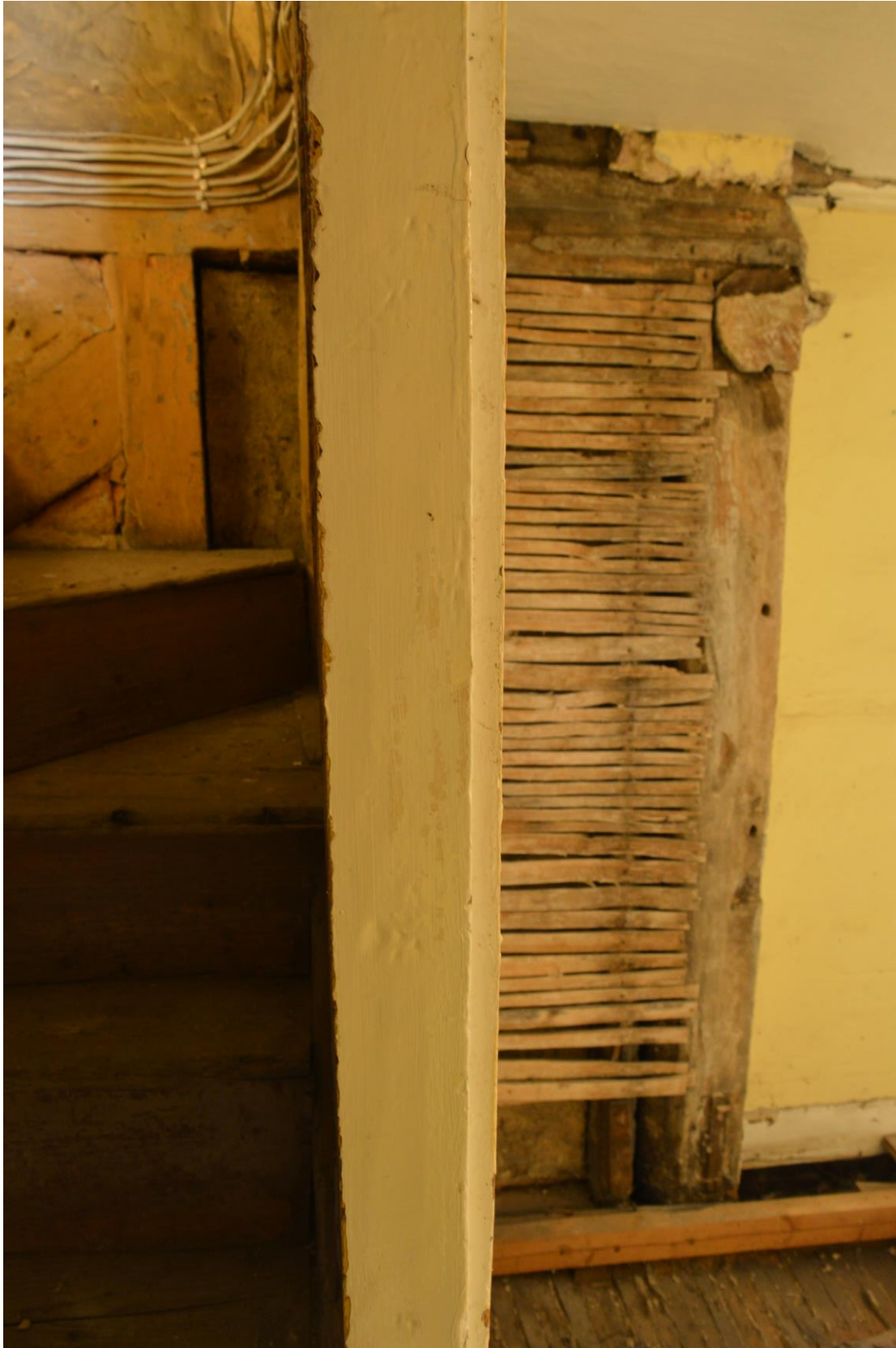
Plate 9: Blocked doorway between high end chamber and hall chamber, partially obscured by later partition, facing west (BES-0117)
