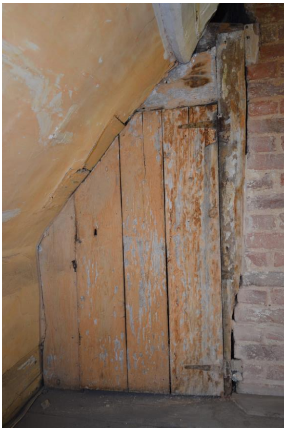
Plate 15: Plank and batten door in attic room, facing west (BES-0105)
