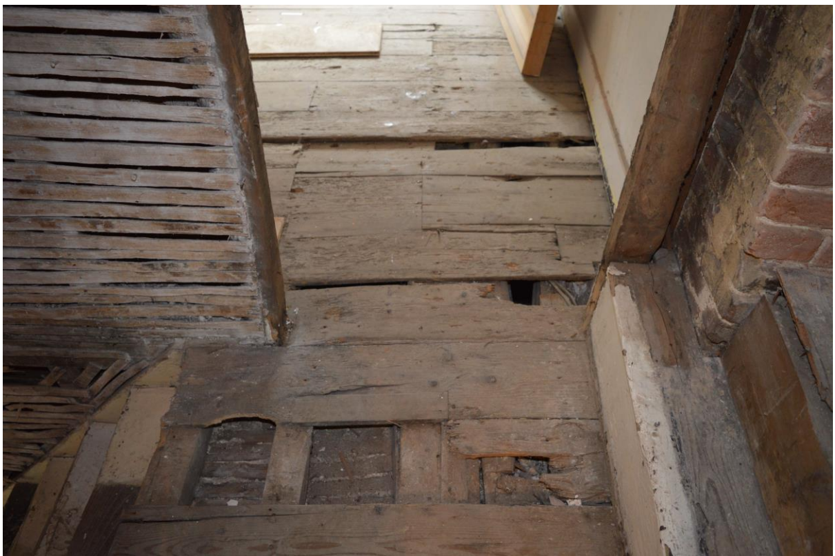
Plate 17: First floor joists and boards, facing south (BES-0086)
