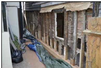
BES17-0035 Exposed wall framing of east elevation. Facing south-west
