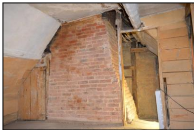
BES17-0107 Attic south room. Facing west
