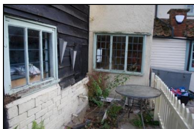
BES17-0120 External view of north wall and extension. Facing south
