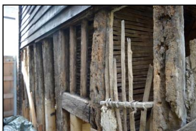
BES17-0043 Diamond mullion window in west wall. Facing south-west
