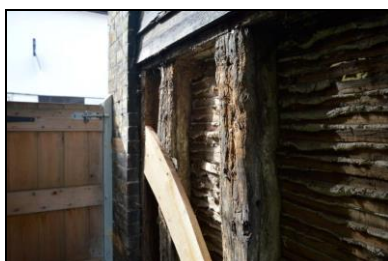
BES17-0044 Studs in west wall. Facing south-west
