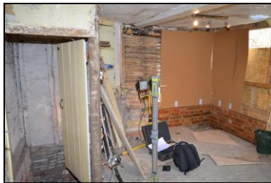
BES17-0056 Ground floor north room. Facing west
