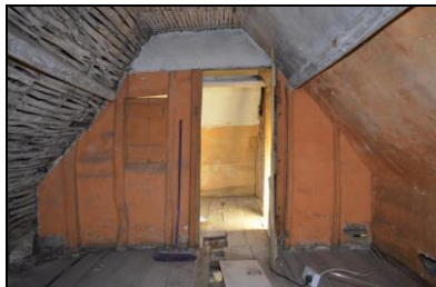
BES17-0113 Attic north room. Facing south
