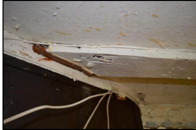
BES17-0049 Bridging joist with redundant mortice. Facing north
