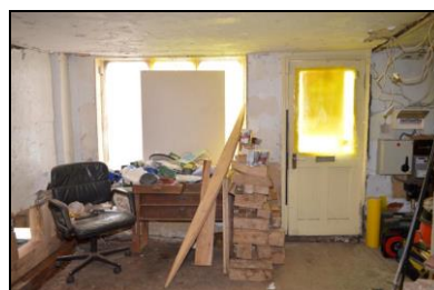
BES17-0045 Interior of ground floor south room. Facing south
