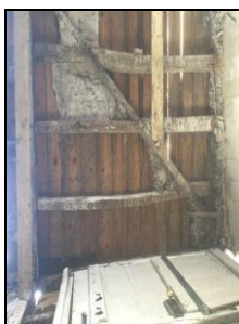
BES17-0119 Wall framing of north wall of Phase 3 extension. Facing north
