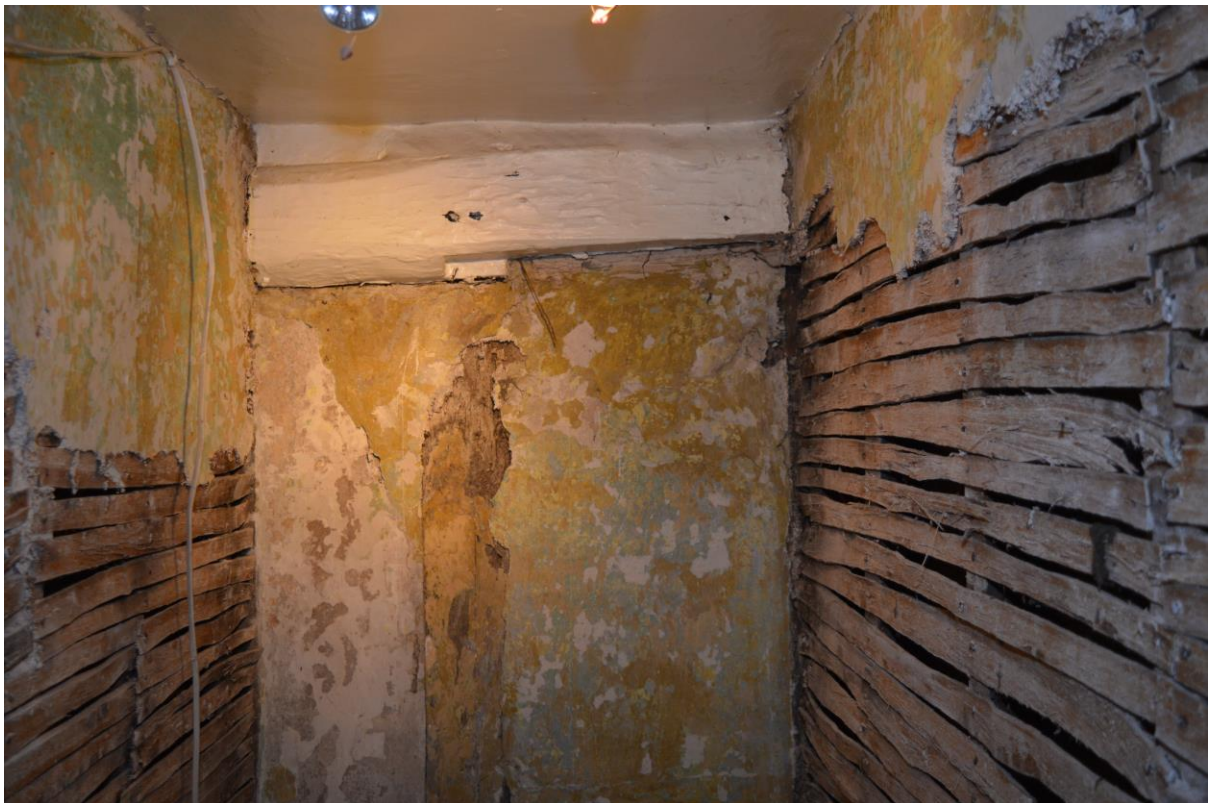
Plate 8: Shutter groove on wall plate of east wall, facing east (BES-0077)
