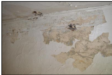
BES17-0052 Side girt in ground floor south room. Facing east
