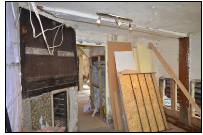
BES17-0048 Interior of ground floor south room. Facing north
