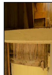
BES17-0117 Blocked door in high end wall frame. Facing west
