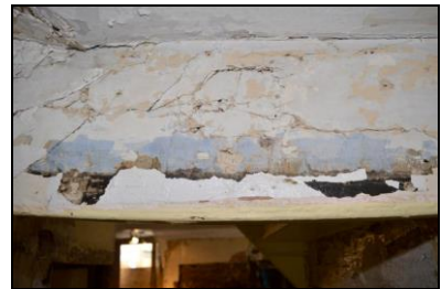
BES17-0054 Remains of wallpaper in ground floor south room. Facing north
