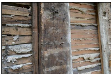
BES17-0037 Carpenter's mark on Phase 3 post. Facing west
