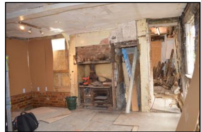
BES17-0057 Ground floor north room. Facing north
