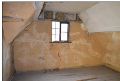
BES17-0108 Attic south room. Facing east
