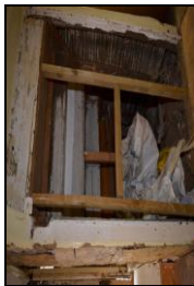
BES17-0055 Underside of stairs. Facing east
