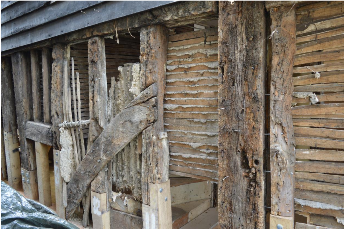
Plate 5: Phase 1 wall framing and remnants of stave and daub panels on east wall (BES-0040)
