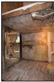
BES17-0076 Stairs. Facing east
