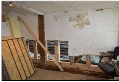
BES17-0047 Interior of ground floor south room. Facing east
