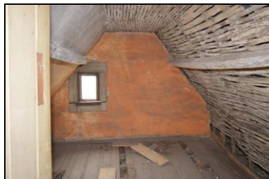
BES17-0111 Attic north room. Facing north
