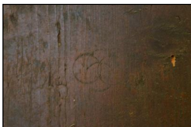
BES17-0118 Apotropaic mark above ground floor south fireplace. Facing north-west
