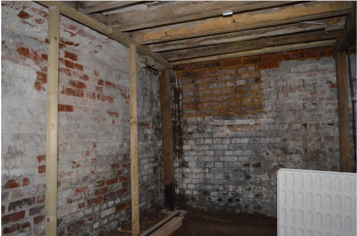
Plate 10: Basement, facing east (BES-0074)
