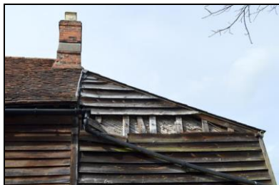
BES17-0034 Exposed studs of extension. Facing west
