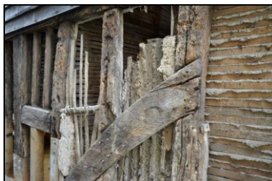
BES17-0041 Curved brace with staves and daub. Facing south-west
