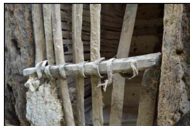
BES17-0042 Staves and daub in west wall. Facing west
