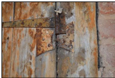
BES17-0106 Butterfly hinge on attic cupboard door. Facing west
