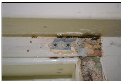
BES17-0085 Wallpaper in 1F south room. Facing south
