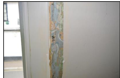
BES17-0084 Wallpaper in 1F south room. Facing south
