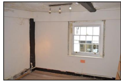
BES17-0078 First floor south room. Facing south
