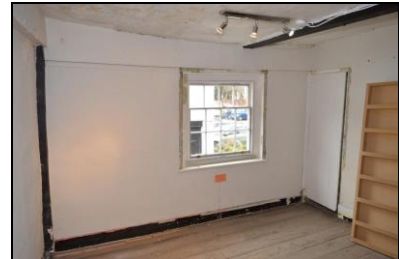
BES17-0081 First floor south room. Facing south
