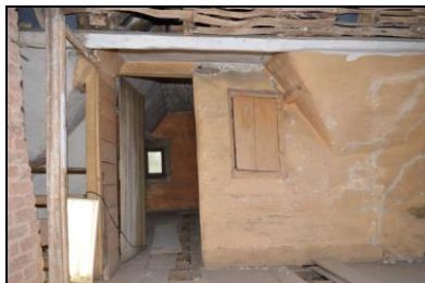
BES17-0109 Attic south room. Facing north
