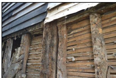
BES17-0038 Junction between main range and rear wing. Facing west
