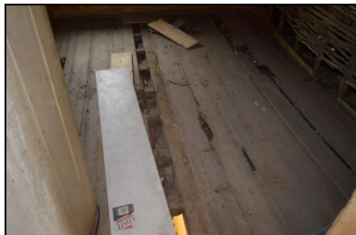
BES17-0112 Floorboards and joists in attic. Facing north
