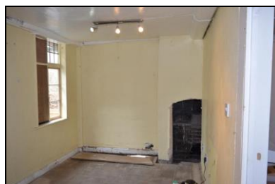
BES17-0089 First floor north-west room. Facing north
