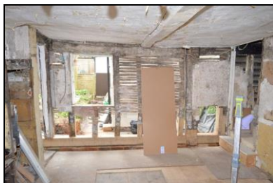
BES17-0058 Ground floor north room. Facing east
