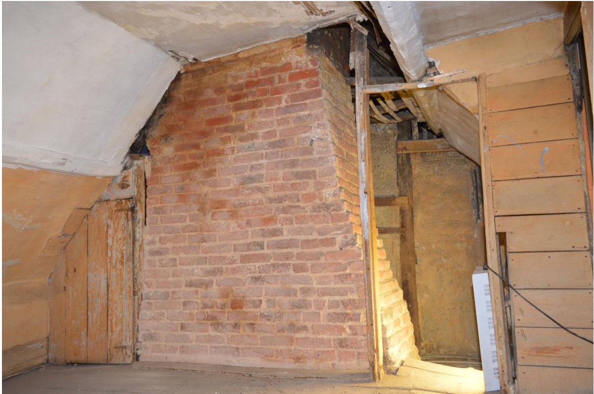
Plate 18: South chimneystack, facing west (BES-0107)
