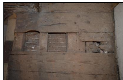
BES17-0087 First floor boards and joists. Facing south
