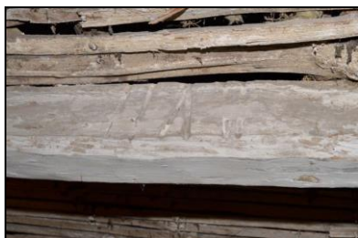
BES17-0116 Merchant's marks on purlin. Facing east
