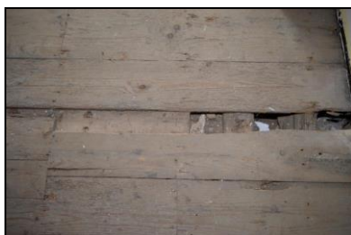
BES17-0088 First floor boards. Facing south
