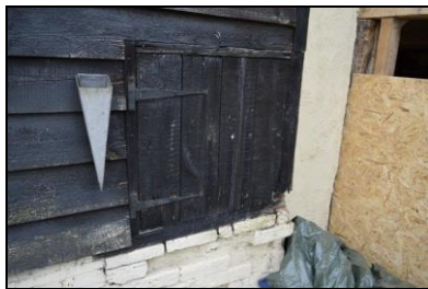
BES17-0031 Plank and batten shutter on extension. Facing east
