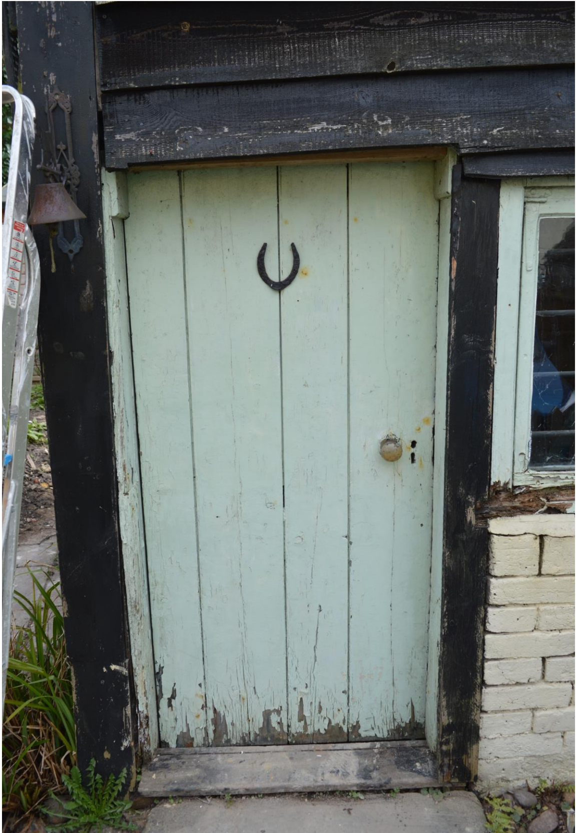
Plate 24: Plank and batten door leading to Phase 3 extension (BES-0029)
