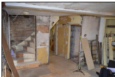
BES17-0059 Ground floor north room. Facing south
