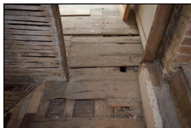
BES17-0086 First floor boards and joists. Facing south
