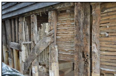
BES17-0040 Exposed wall framing of east elevation. Facing west
