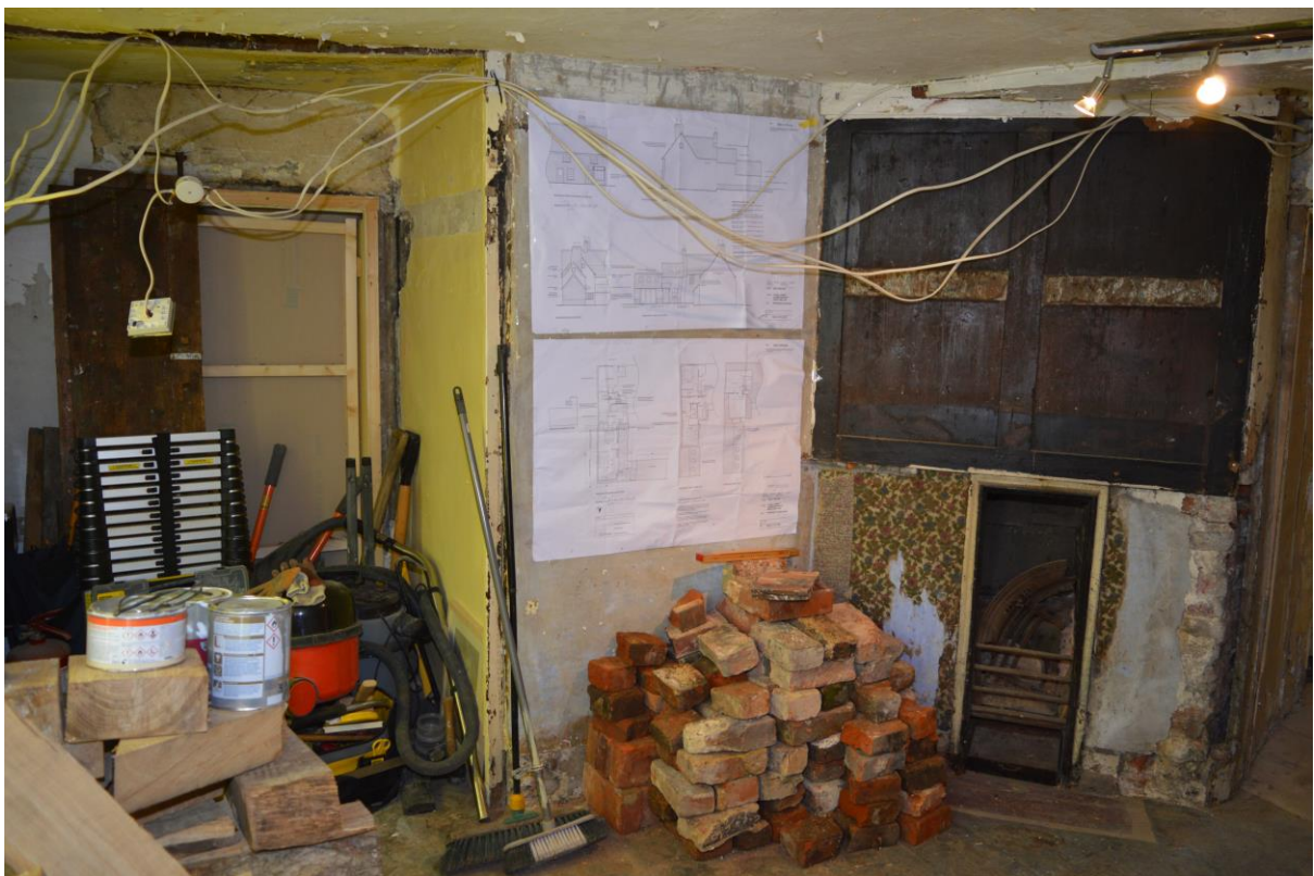
Plate 19: Panelling above ground floor south fireplace, facing west (BES-0046)
