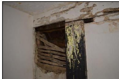
BES17-0083 Shutter groove in 1F south room. Facing east
