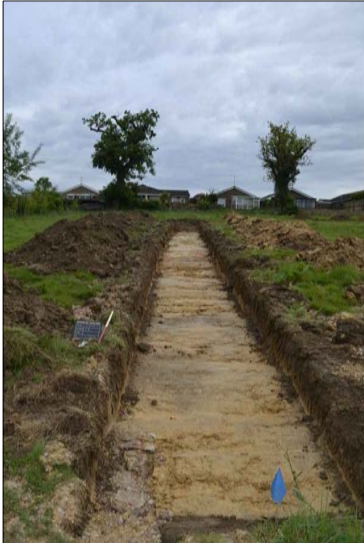
Trench 9 facing north
