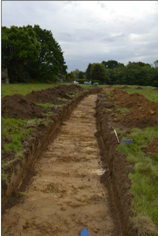
Trench 1 facing south west
