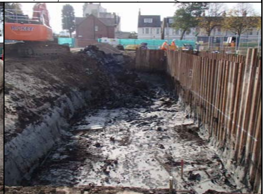
General view of trench, looking west
