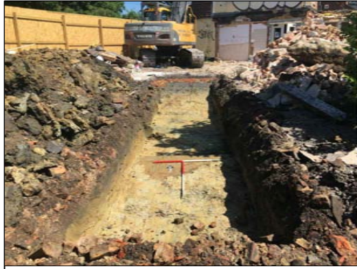
Trench 1 facing north
