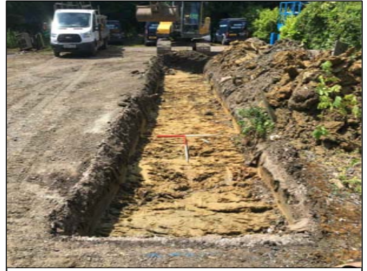
Trench 2 facing south west
