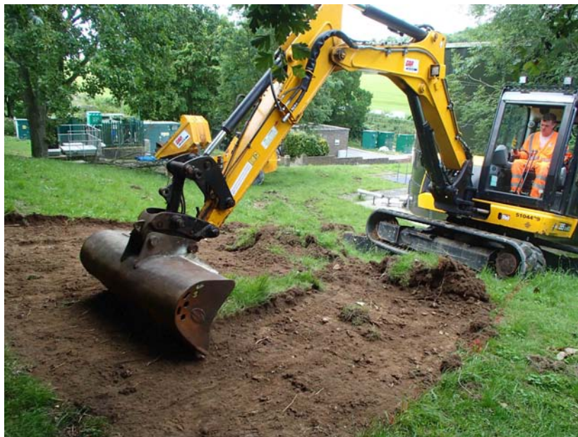
Topsoil stripping looking south-west
