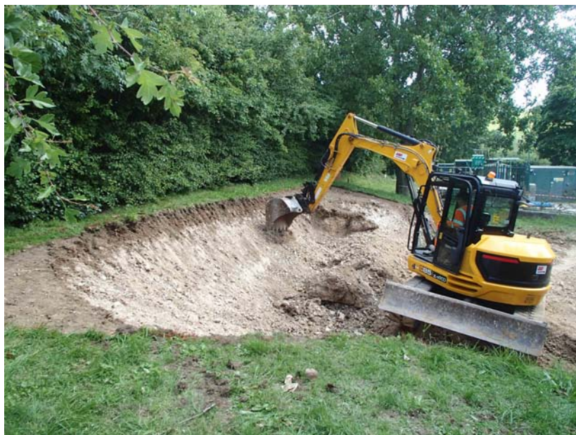
Working area looking south during excavation
