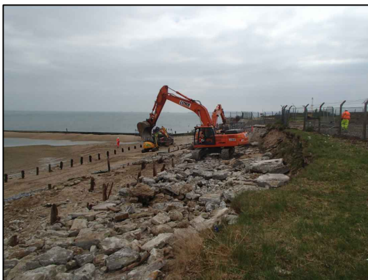
Removal of Concrete
