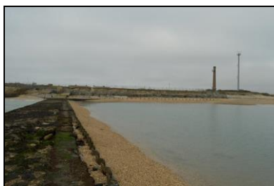
FCS17-0002 General view of site. Facing north-west
