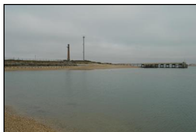
FCS17-0001 General view of site. Facing north
