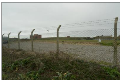
FCS17-0038 View of the fort. Facing south-west
