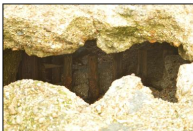
FCS17-0014 Wooden posts within the voids
