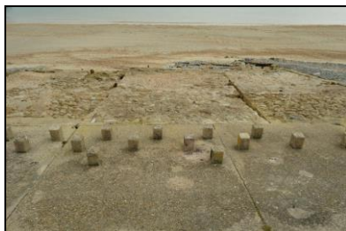
FCS17-0043 Concrete on the shore. Facing east
