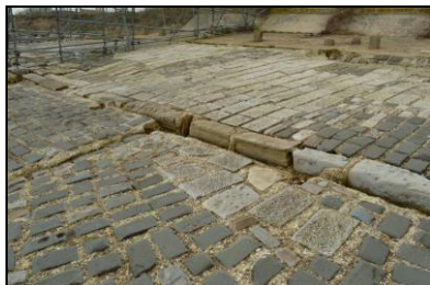
FCS17-0035 Detail of stone setts on the shore. Facing west
