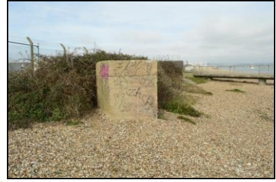
FCS17-0063 Ventilation Shaft detail. Facing north-west
