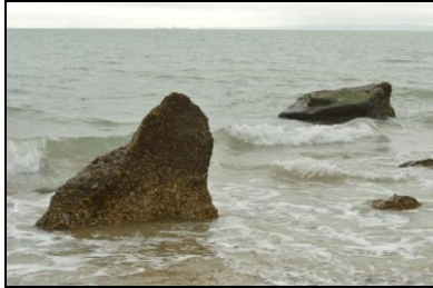
FCS17-0049 Broken concrete in the sea. Facing south
