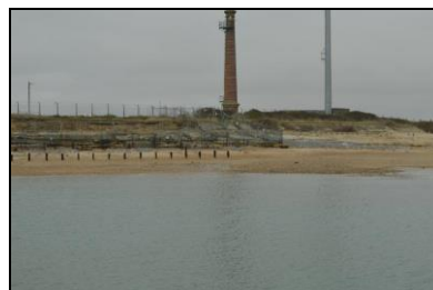
FCS17-0006 Detail of the coastal area nearest the chimney. Facing north-west
