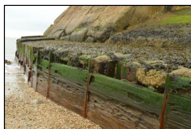
FCS17-0009 Detail of the wooden revetments. Facing south
