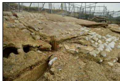
FCS17-0015 Condition of the shore before works. Facing north
