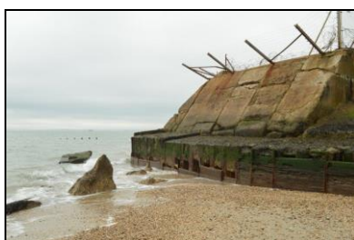
FCS17-0008 Detail of the fort promontory. Facing south
