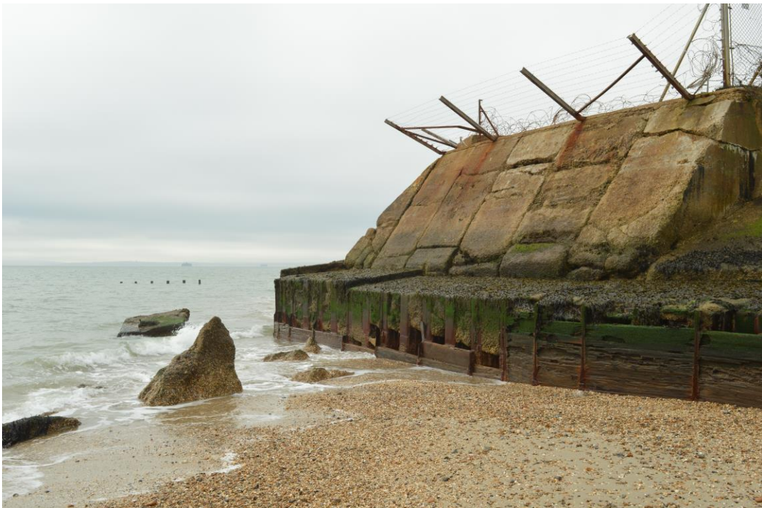
Plate 3: Concrete and timber defences of the fort
