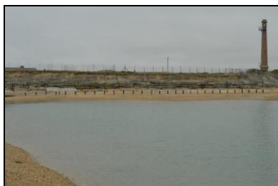
FCS17-0005 General view of the site. Facing north-west
