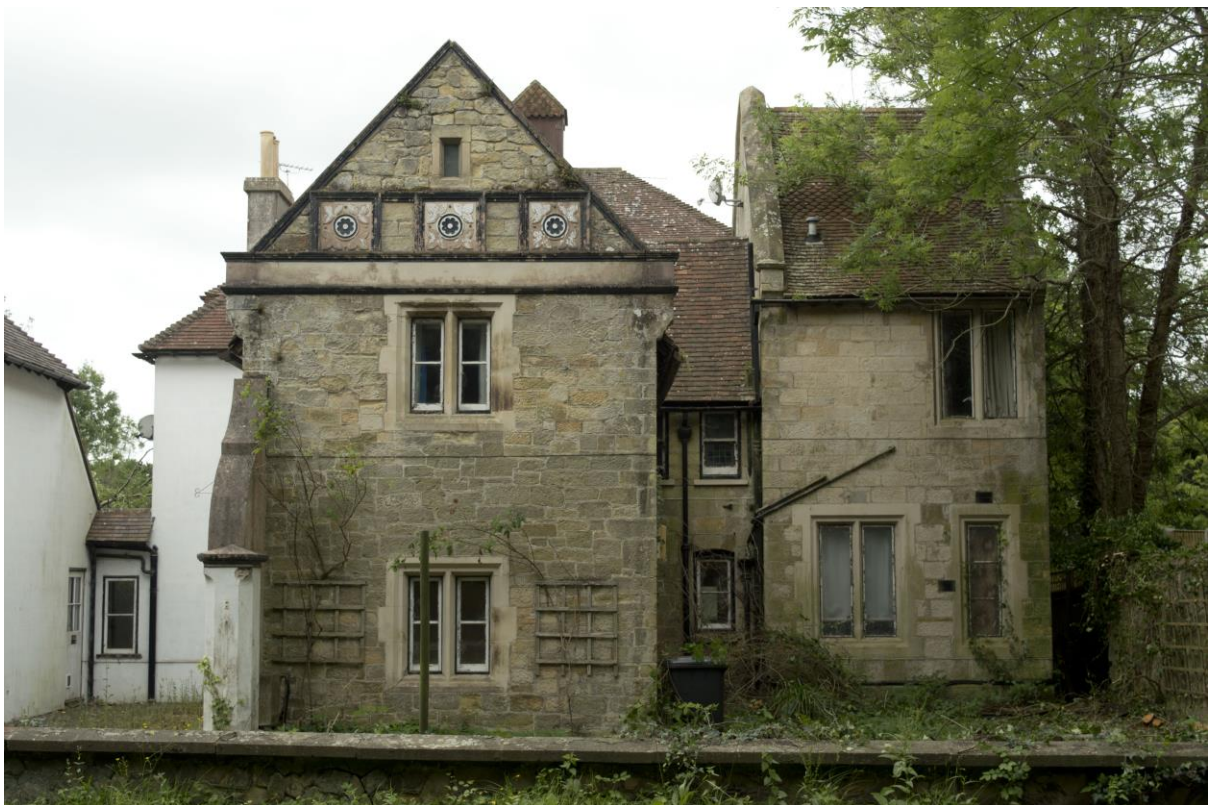
Plate 2: North elevation of main building (WOD17-0024)
