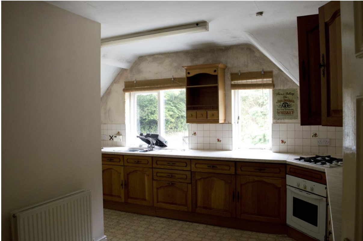
Plate 45: North-east room in Coach House first floor, facing east (WOD17-0121)
