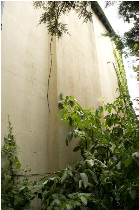
Plate 8: West elevation of main building (WOD17-0033)
