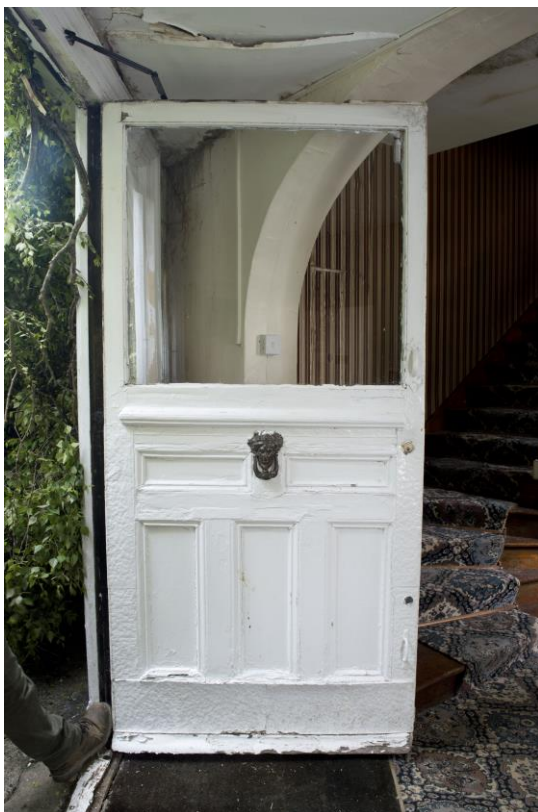
Plate 10: Main door in link, facing east (WOD17-0071)
