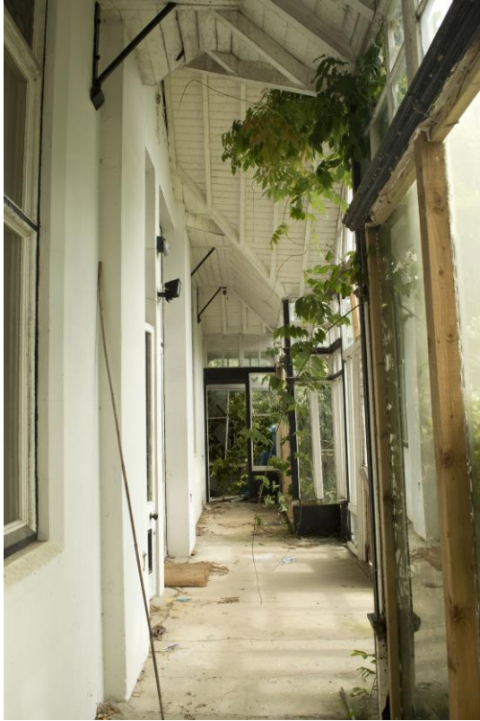
Plate 19: Interior of veranda, facing east (WOD17-0042)
