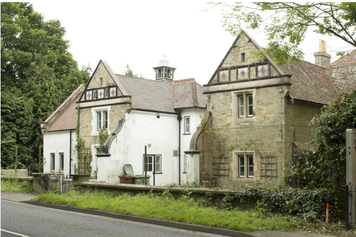
Plate 38: West elevation of the Coach House (WOD17-0025)
