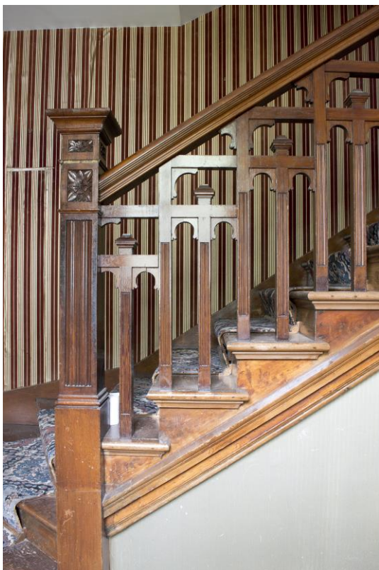
Plate 12: Detail of main staircase, facing south (WOD17-0072)
