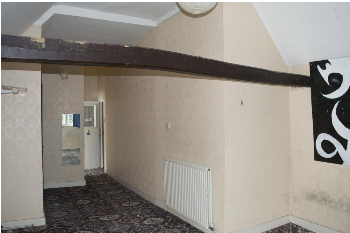
Plate 34: First floor bedroom in north range, facing south (WOD17-0112)
