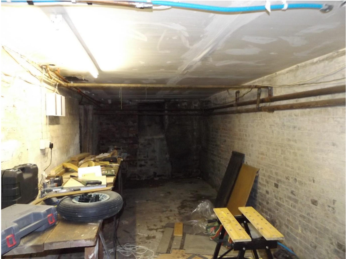
Plate 47: View of basement, facing east (photograph provided by Bellway Homes)
