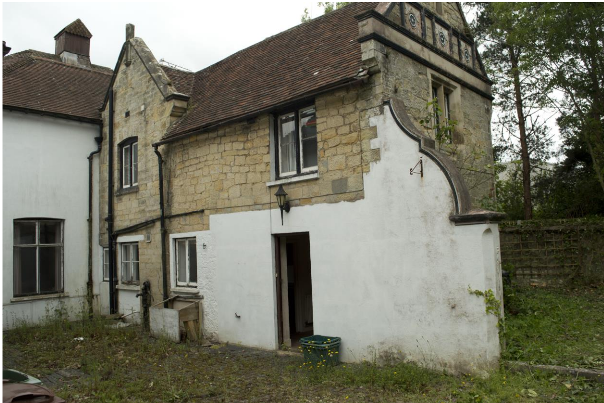
Plate 3: East elevation of the main building's north range (WOD17-0026)
