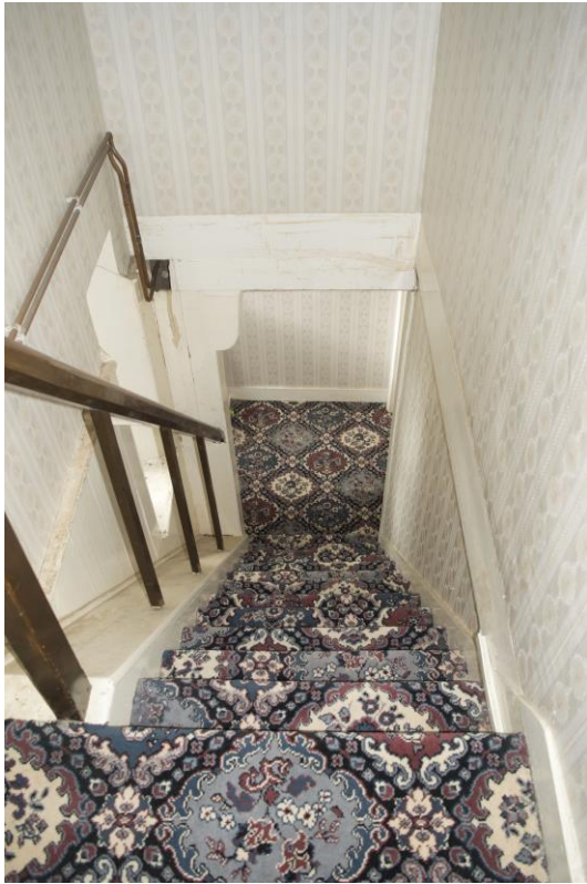
Plate 23: Stairs in the north range of the main building, facing north (WOD17-0113)
