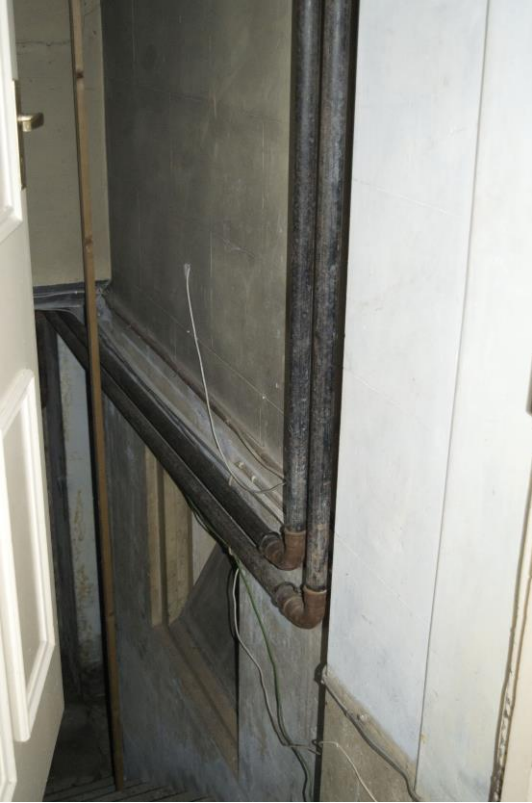
Plate 21: Previously external wall in stairs to basement, facing west (WOD17-0141)
