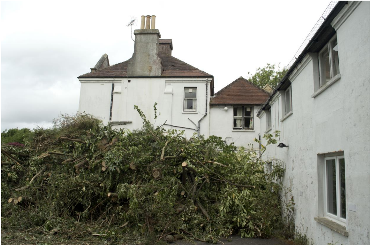
Plate 7: East elevation of main building (WOD17-0011)
