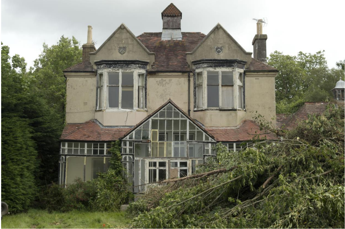
Plate 5: South elevation of main building (WOD17-0004)
