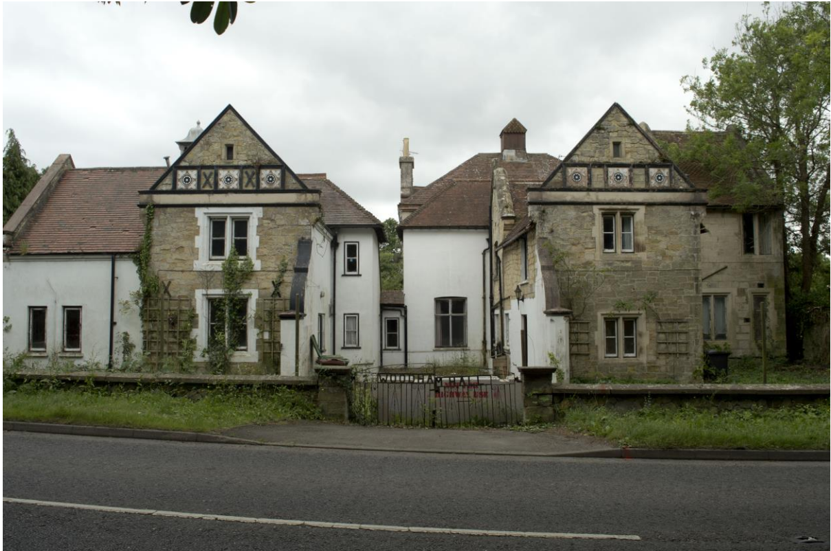
Plate 1: North elevation of main building and Coach House (WOD17-0023)
