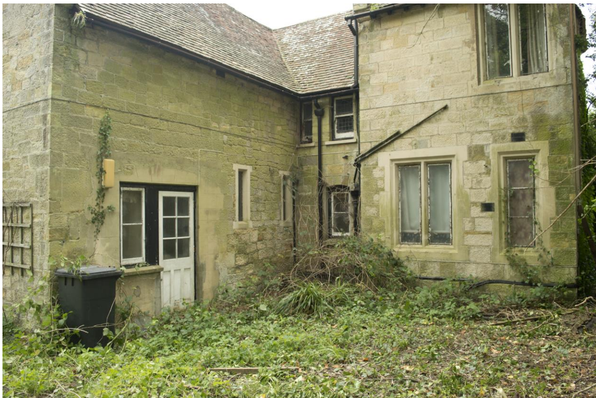
Plate 4: West elevation of main building's north range (WOD17-0029)
