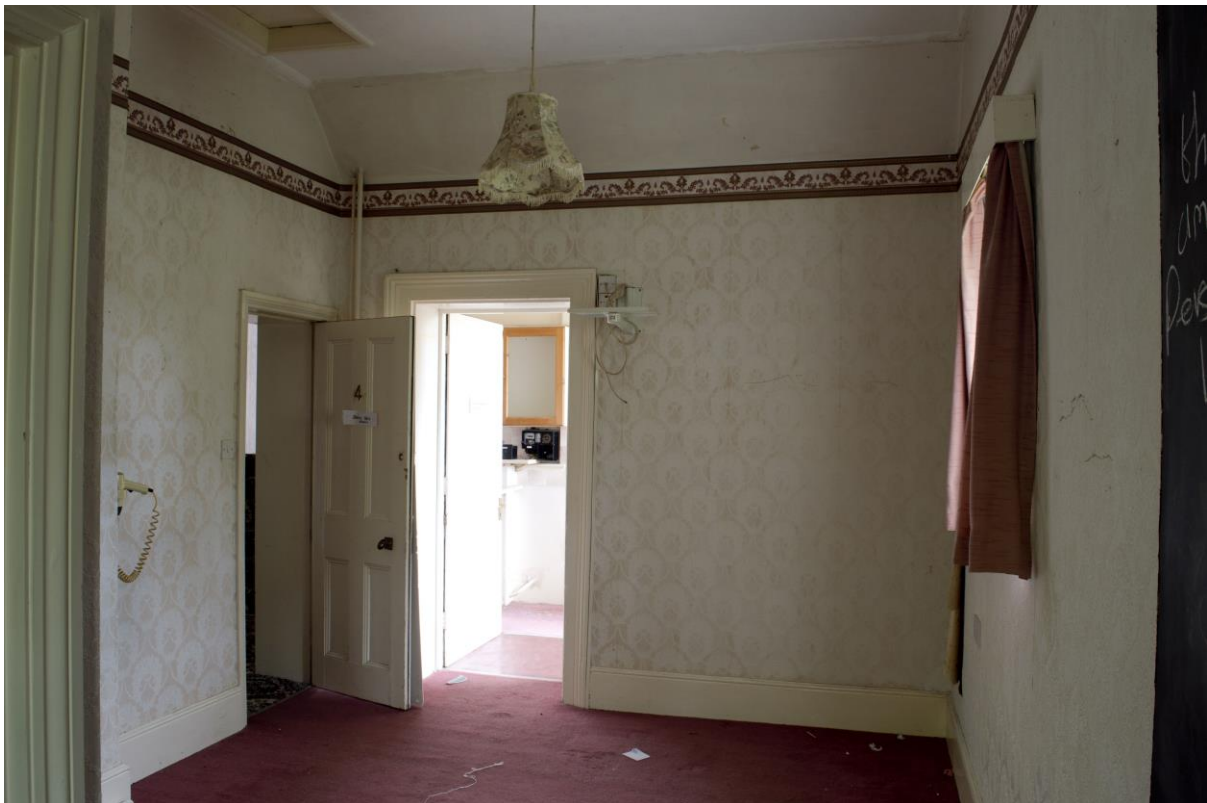
Plate 32: Bedroom in first floor of west range, facing south (WOD17-0091)
