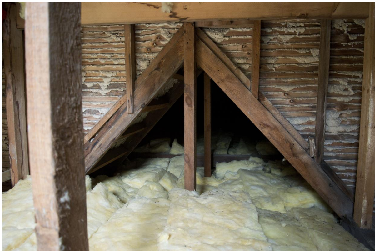
Plate 29: The two shafts where they converge in the south range roof, facing east (WOD17-0098)
