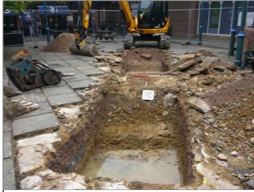
Trench 1 facing north west
