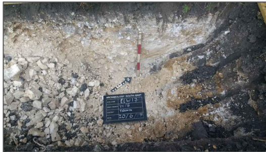
Representative section of site sequence at north west corner of foundations
