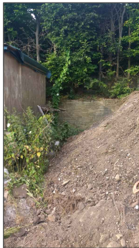
South west boundary, showing extant terrace retaining wall
