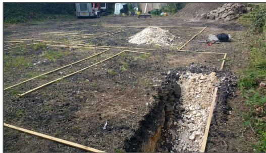
View of site foundation excavations looking north
