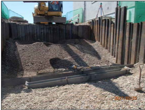
Monitored area looking south
