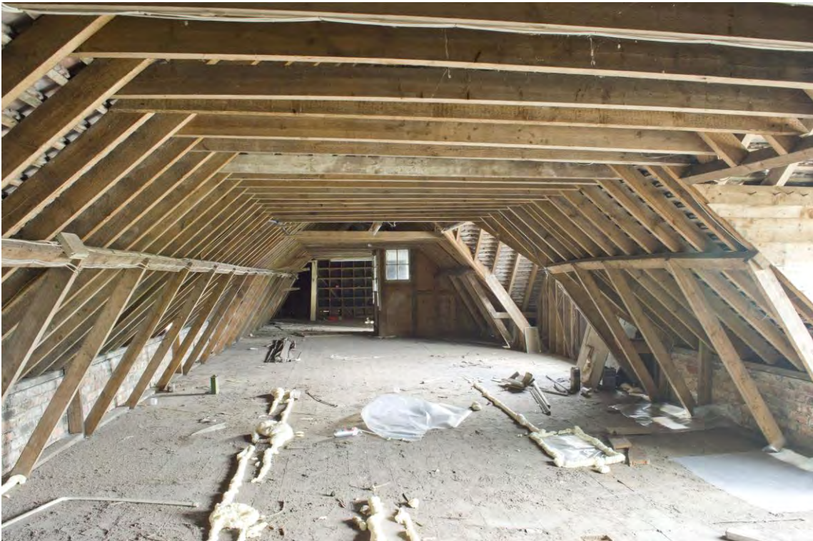
Plate 22 Attic of the northern half of Range 3, facing west (73)
