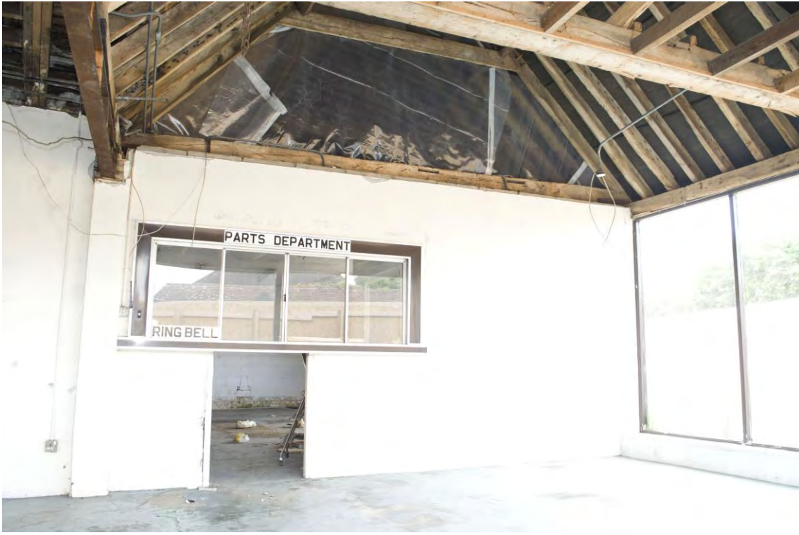
Plate 5 Northern end of Range 1, note the steel joist used to support the east elevation, facing south-west (38)
