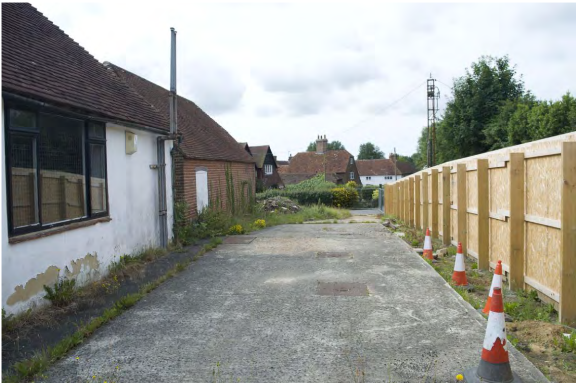
Plate 32 Area of the western underground petrol tank adjacent the west elevation of Range 1, facing south (6)
