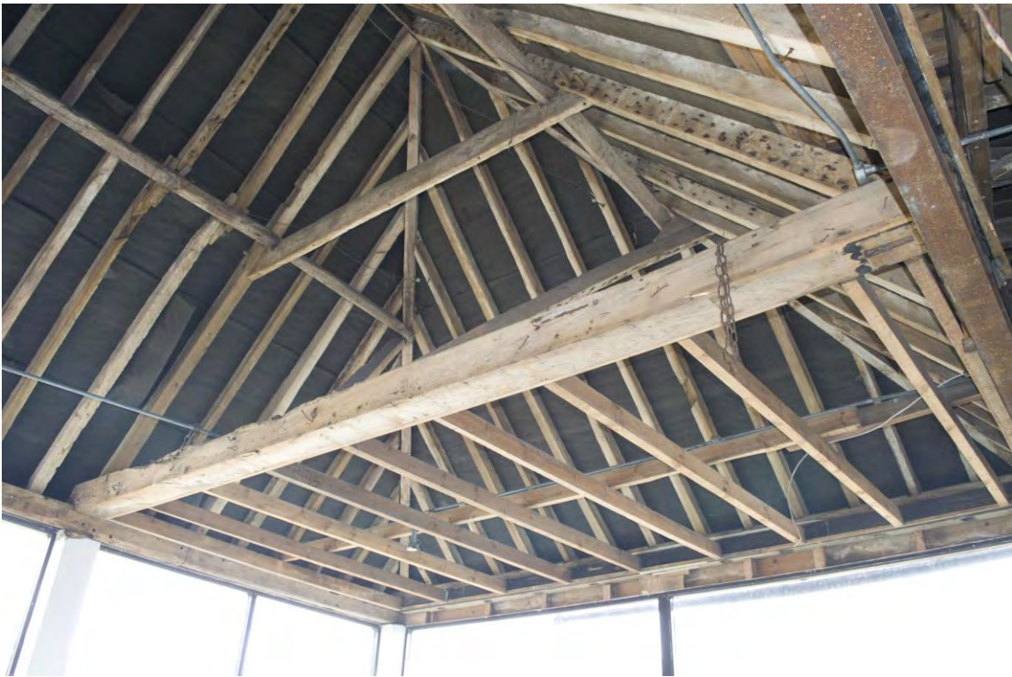
Plate 8 View of the Range 1 roof, facing north-west (36)
