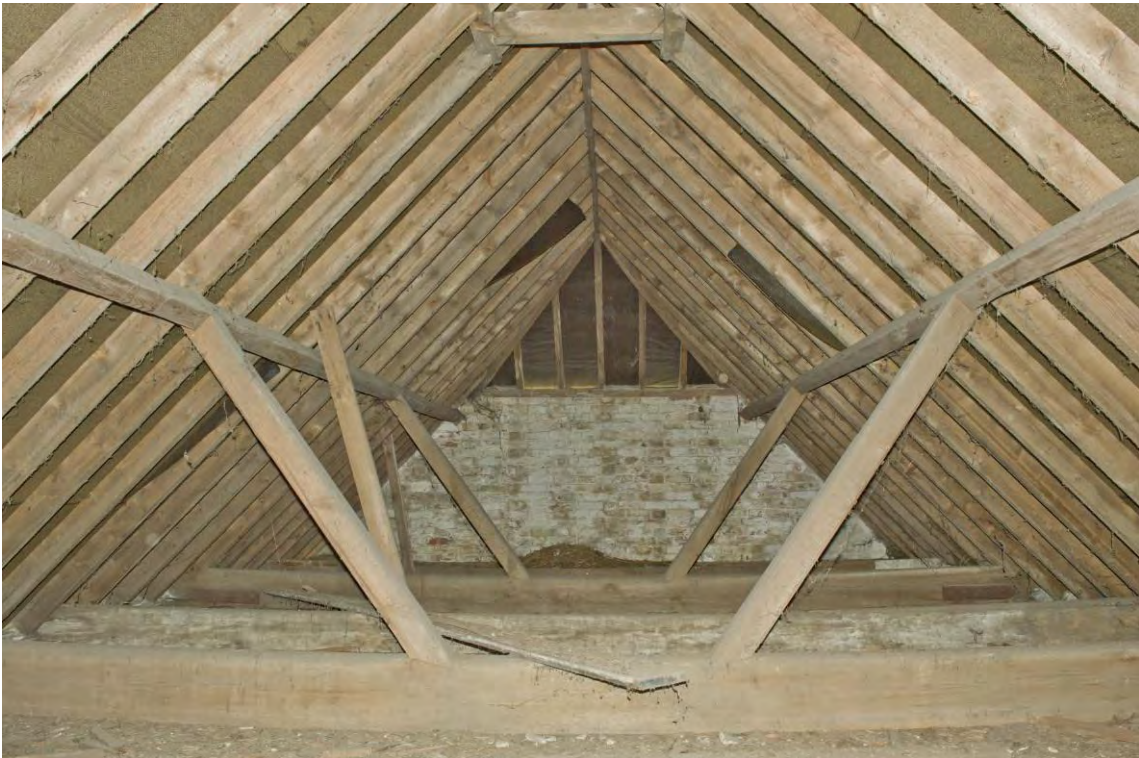
Plate 14 View of the roof construction above Range 2, facing south (95)
