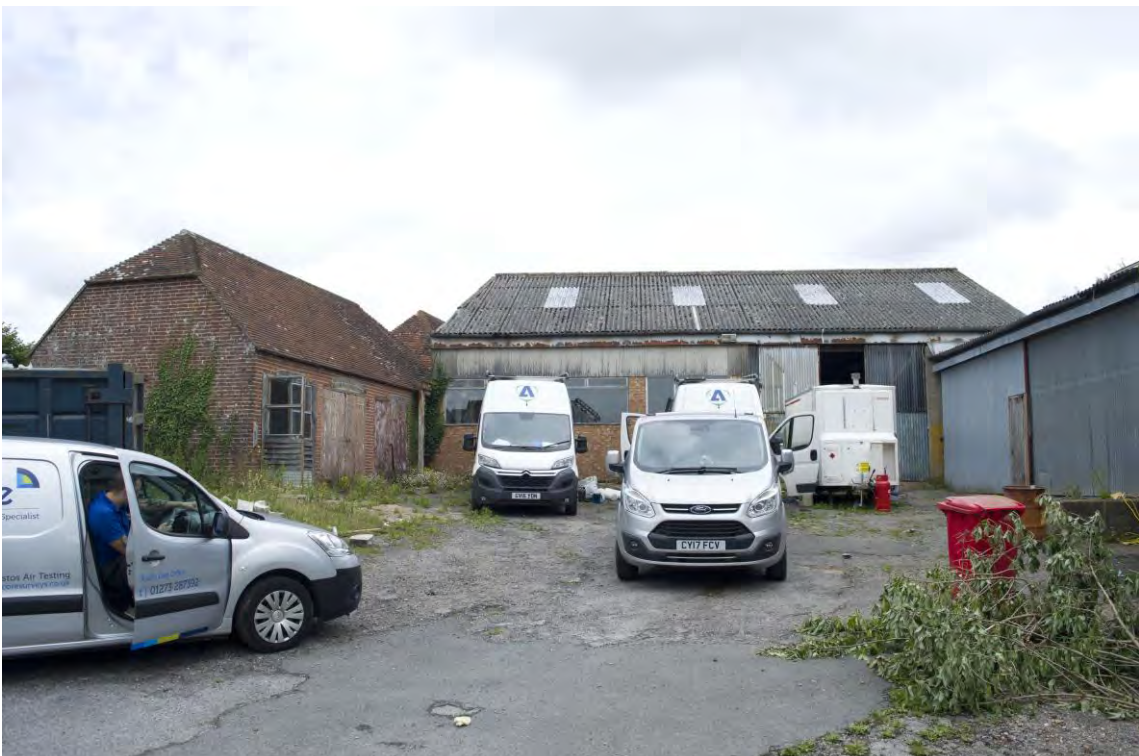
Plate 20 South elevation of Range 3 (southern extension), facing north (17)
