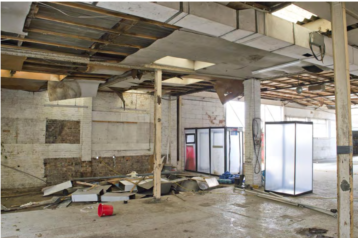
Plate 26 View of the eastern end of Range 3 (southern extension), facing south-west (56)
