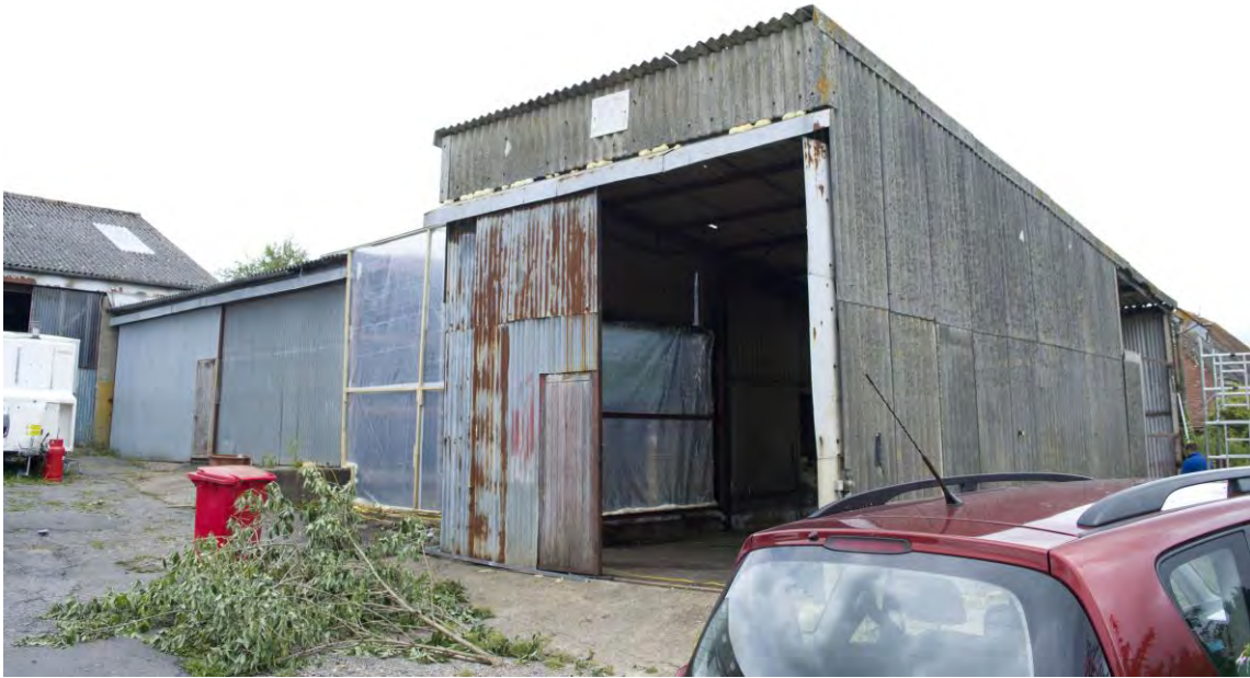
Plate 29 General view of Range 4, facing north-east (24)
