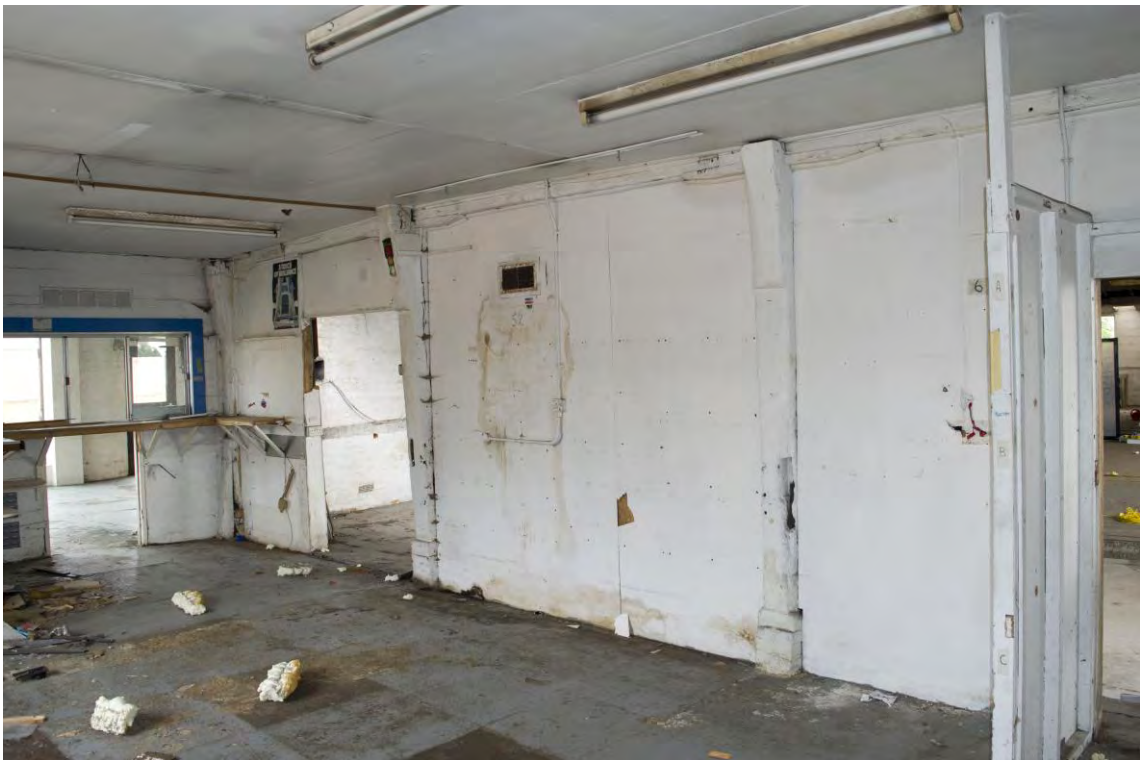
Plate 4 Interior of Range 1, note the bay divisions, facing north-east (29)
