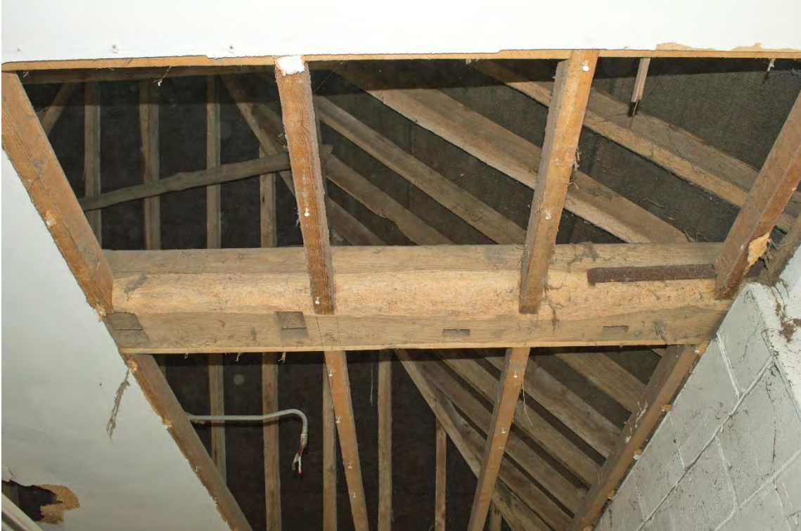
Plate 9 Detail of the chamfered edging to the southernmost tie beams within Range 1, facing south (79)
