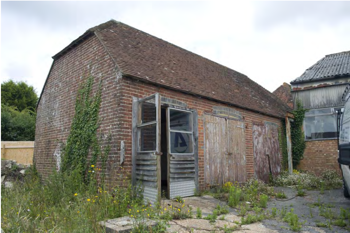
Plate 35 View of the disturbed ground of the rear yard, facing north (17)
