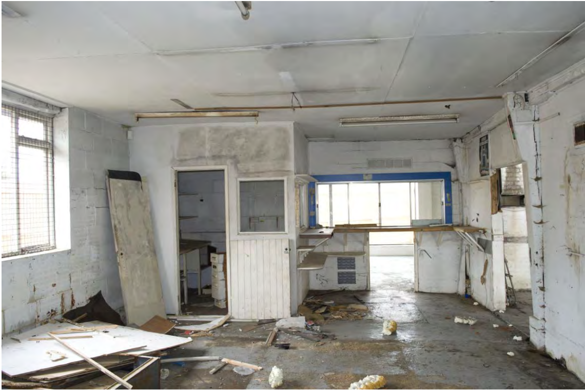
Plate 3 Internal view of the partitioning within Range 1, facing north (26)
