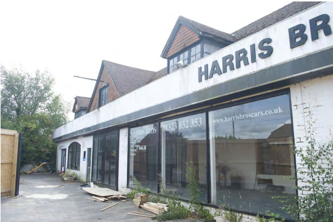
Plate 18 General view of the principal range of Range 3, facing south-east (8)
