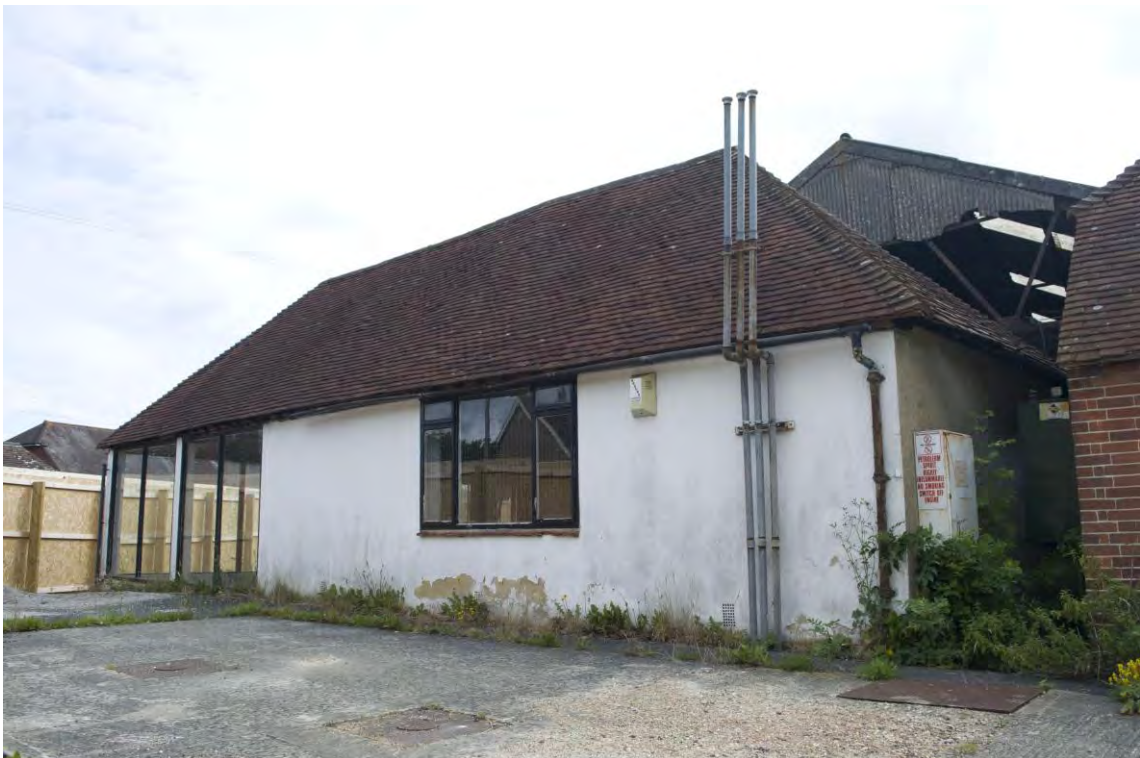
Plate 2 General view of Range 1, facing north-east (4)
