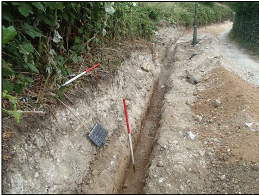
Monitored works, looking north east
