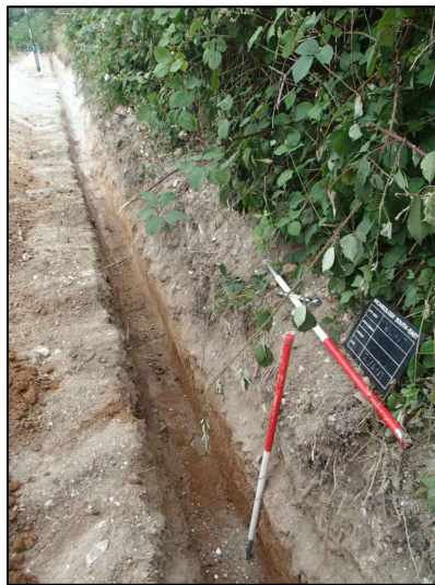
Monitored works, looking south west
