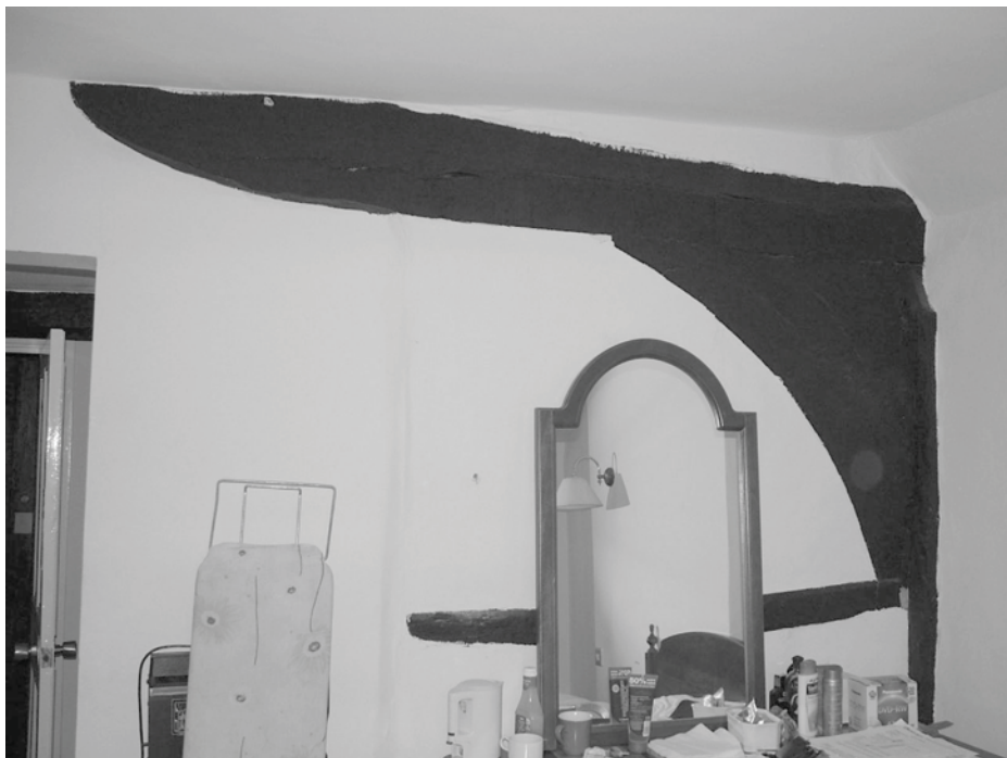
Plate 10 Service crossing. Remains of truss K-K' viewed from east
