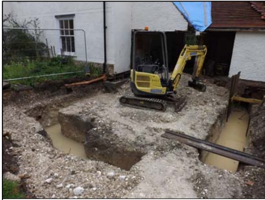
1. General view of groundworks
