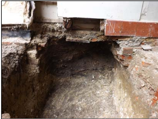
3. Wall foundation 19 and Trench 12 in UP1
