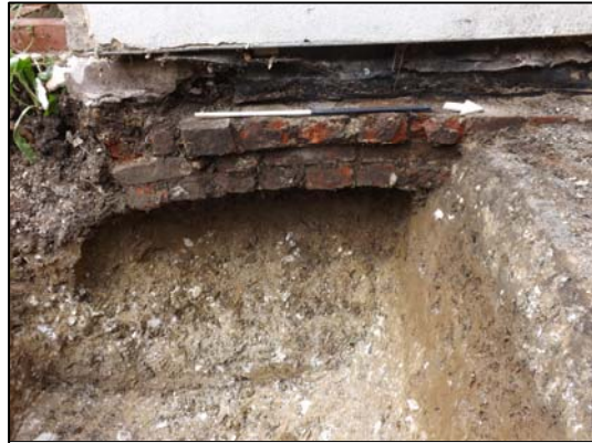
4. Wall foundation 19 in UP2
