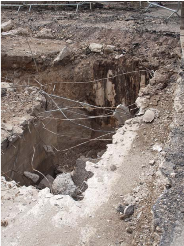
Plate 6: Blocked opening in south-west corner of the shelter, facing south (RSP17-0081)
