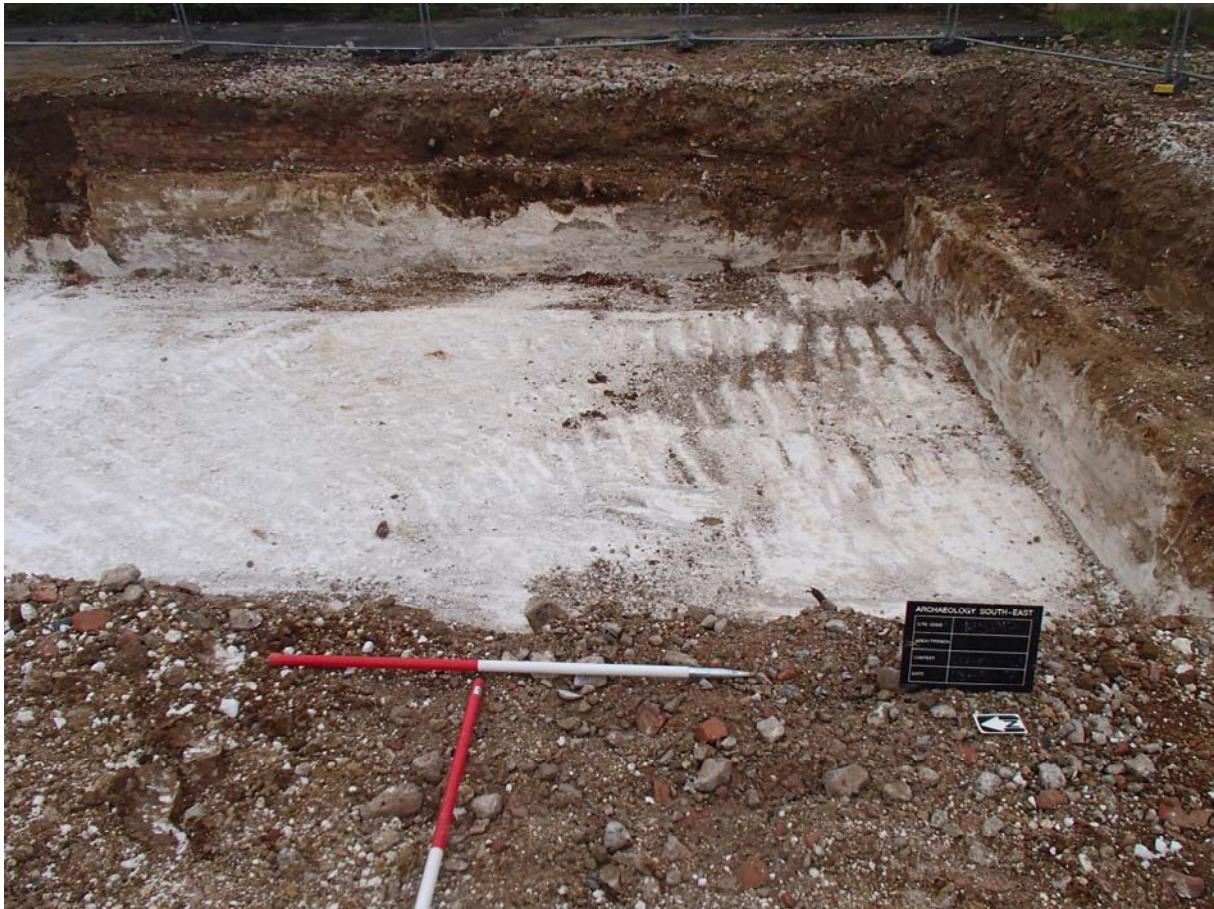
Plate 7: Soakaway 2, brick wall visible at far end, facing east (RSP17-0106)
