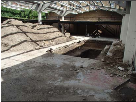
View across trench 6 looking north-west
