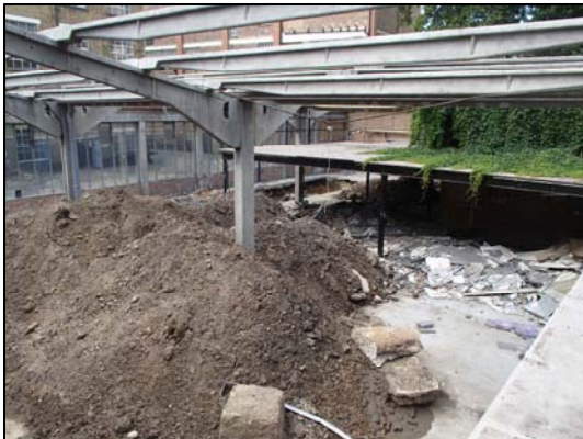
View across trench 7 looking south-west
