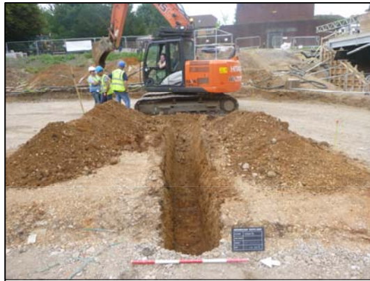
f. Drainage Trench 2
