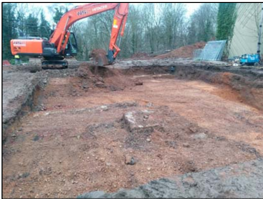
a. Area 1 general view
