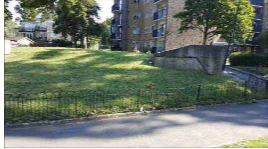
View north across Site C showing above ground blocked up stairwell
