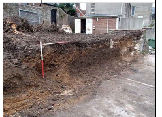
Wall 1089 looking north-west
