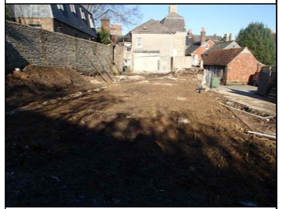
Overall view of site looking north
