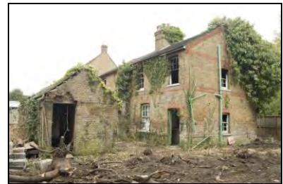
HRI17-0012 Rear of n. 15. Facing east
