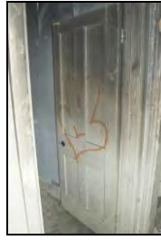
HR117-0077 Detail of internal door, room 18. Facing north
