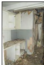
HR117-0089 Interior of room 3. Facing east
