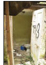
HR117-0039 Interior of room 14. Facing north-west
