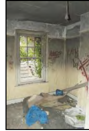
HR117-0081 Interior of room 8. Facing north-west
