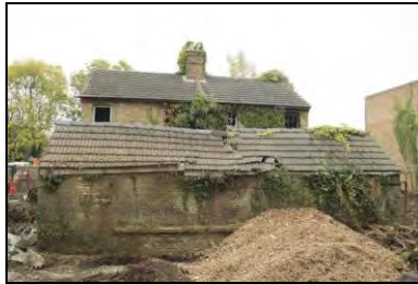
HRI17-0008 NW elevation of outbuilding. Facing south-east
