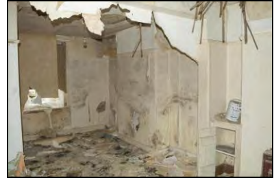
HR117-0096 Interior of room 2. Facing north
