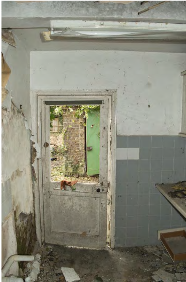
Plate 9 – The back door of no.15 (HRI17-0092)
