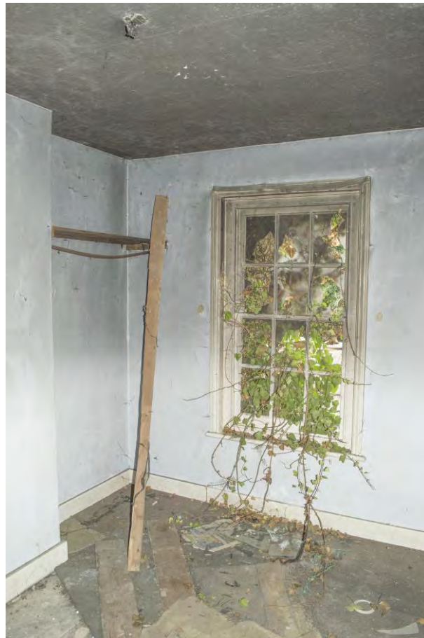
Plate 48 – Room 18, no. 17 (HRI17- 0076)
