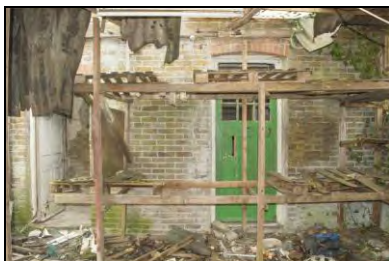
HR117-0040 Rear elevation of n. 17. Facing south-west
