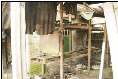
HR117-0037 Interior of the lean too structure (room 13). Facing south
