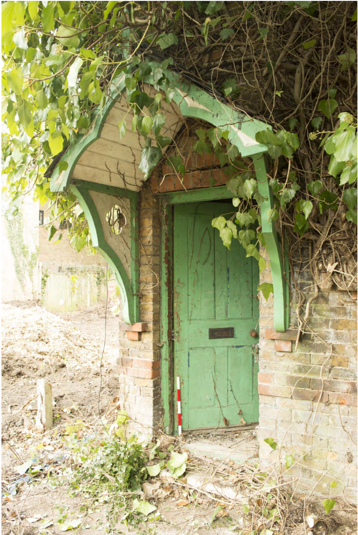
Plate 4 – The front door of no.15 with Arts and Crafts porch canopy (HRI17- 0027)
