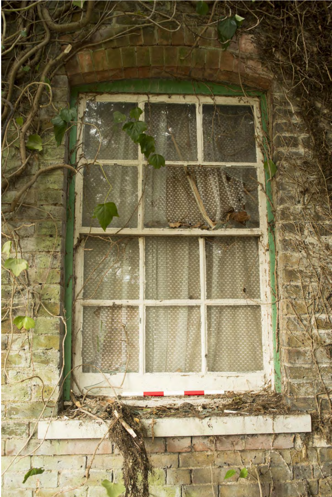
Plate 3 – Twelve paned sash window (HRI17- 0026)
