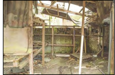
HR117-0036 Interior of the lean too structure (room 13). Facing south-west
