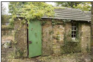
HRI17-0013 SW elevation of the outbuilding, n. 15. Facing north
