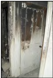
HR117-0082 Detail of internal door to room 8. Facing west
