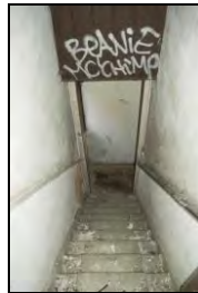
HR117-0068 Stairs in n. 17 (room 1). Facing south-east
