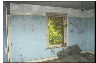
HR117-0072 Interior of room 17. Facing south
