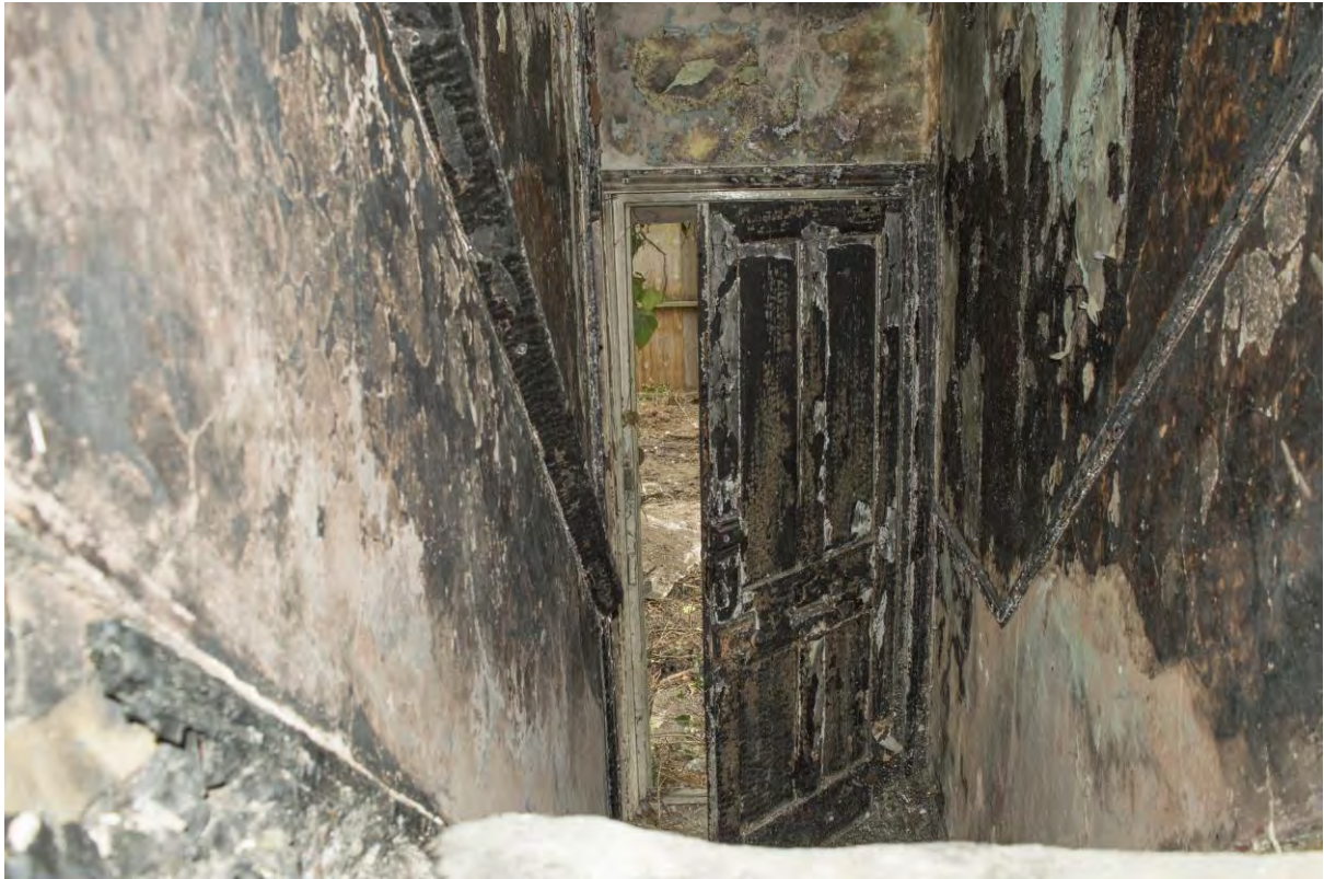
Plate 15 – Stairway and front door, no. 15 (HRI17-0093)
