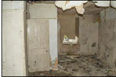
HR117-0095 Interior of room 2. Facing north
