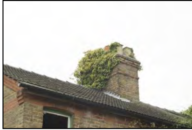
HRI17-0005 Detail of the Chimney Stack. Facing south
