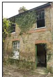
HRI17-0014 NW elevation of n. 15. Facing east
