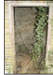
HR117-0066 Interior of room 15. Facing south
