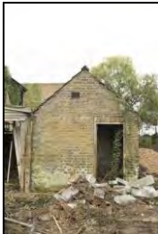
HRI17-0007 NE elevation of the outbuilding of n.17. Facing south-west
