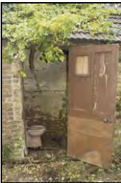
HR117-0067 Interior of room 4. Facing north-west
