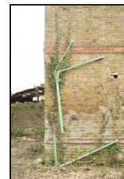
HRI17-0015 Detail of external piping, n. 15. Facing north-east
