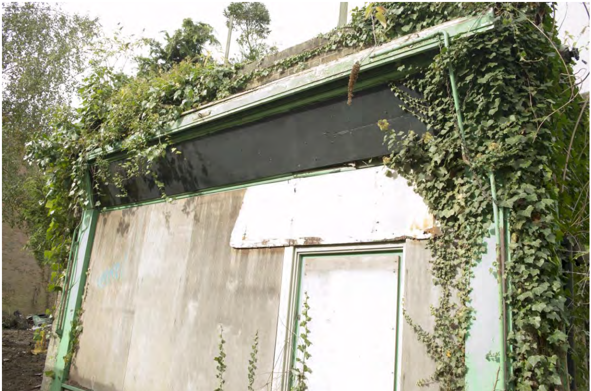
Plate 29 – The shop front, (south east elevation) no. 17 (HRI17-0021)
