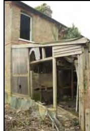
HR117-0035 Lean too structure at the rear of n. 17. Facing south
