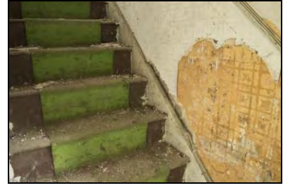
HR117-0063 Detail of stairs in n. 17 (room 10). Facing north
