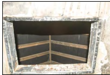
HR117-0086 Roof structure from access hatch
