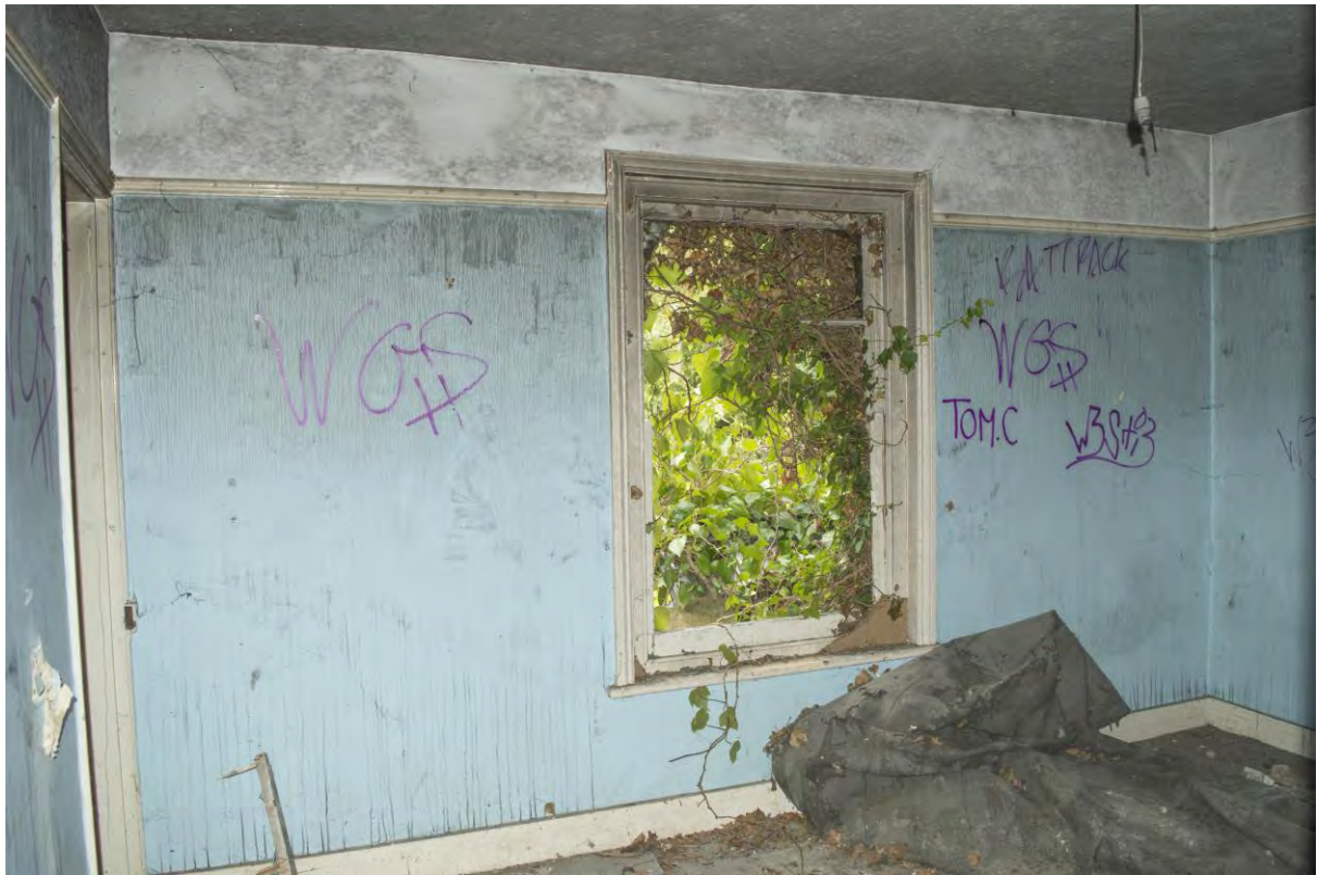
Plate 47 – Room 17, no. 17 (HRI17- 0072)
