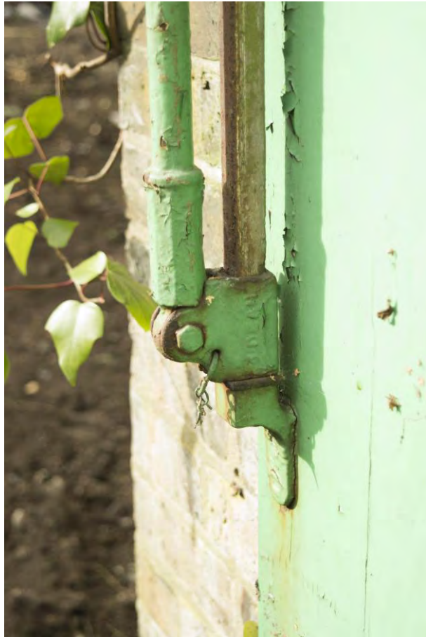
Plate 32 – Detail of the blind bracket, no. 17 (HR117- 0022)
