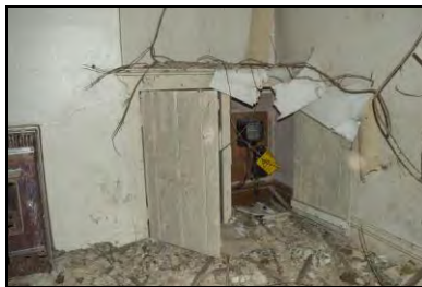
HR117-0101 Detail of fitted cabinet, room 2. Facing north-east
