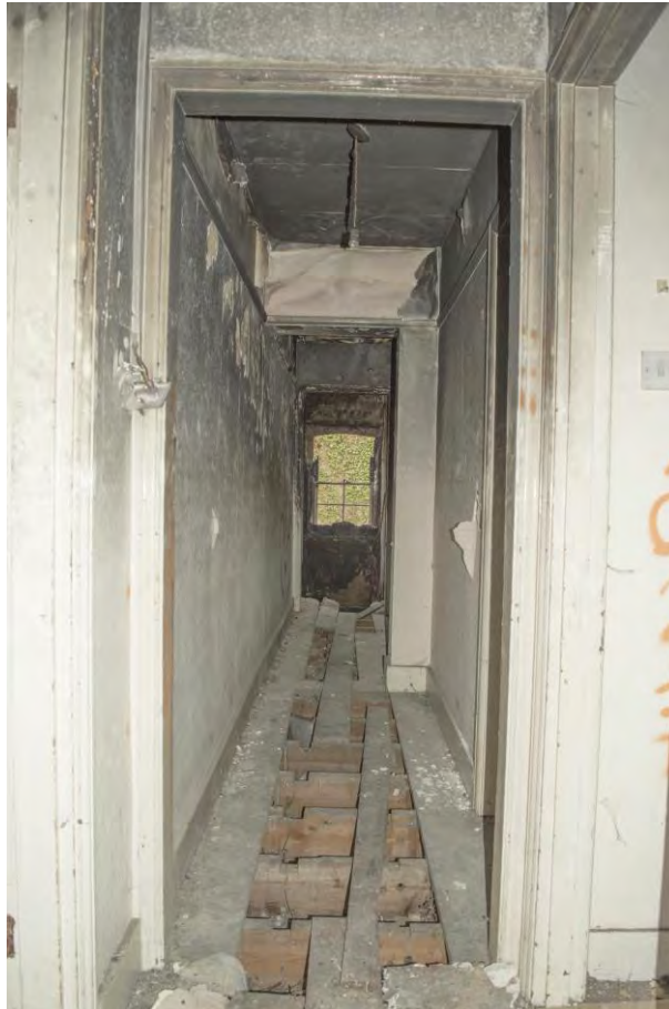
Plate 22 – The corridor addition on the first floor (HR117-0069)
