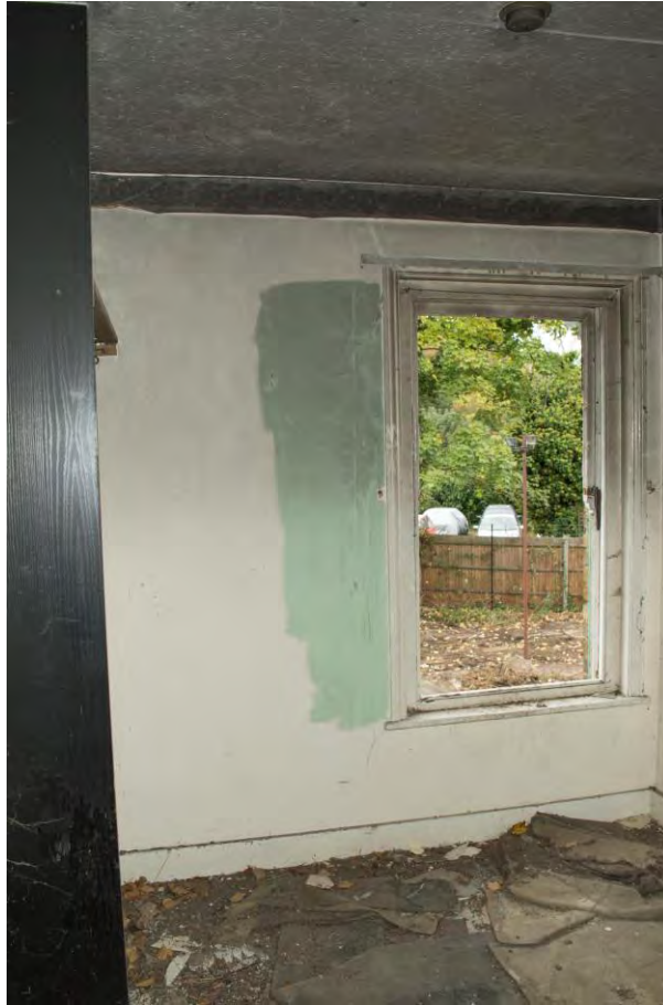
Plate 49 – Room 19, no. 17 (HRI17- 0074)
