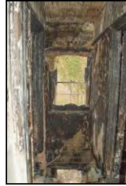
HR117-0080 Interior of room 1. Facing south-east
