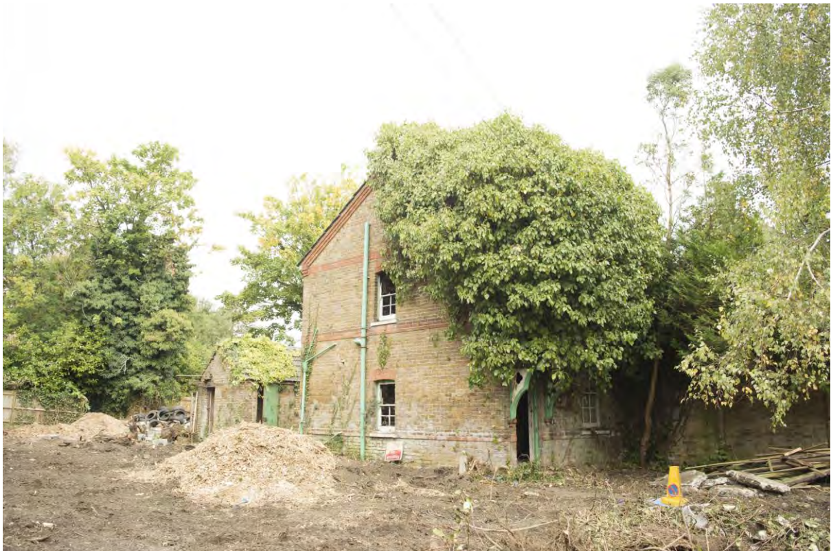
Plate 2 – No. 15, general view looking north (HR117-0018)
