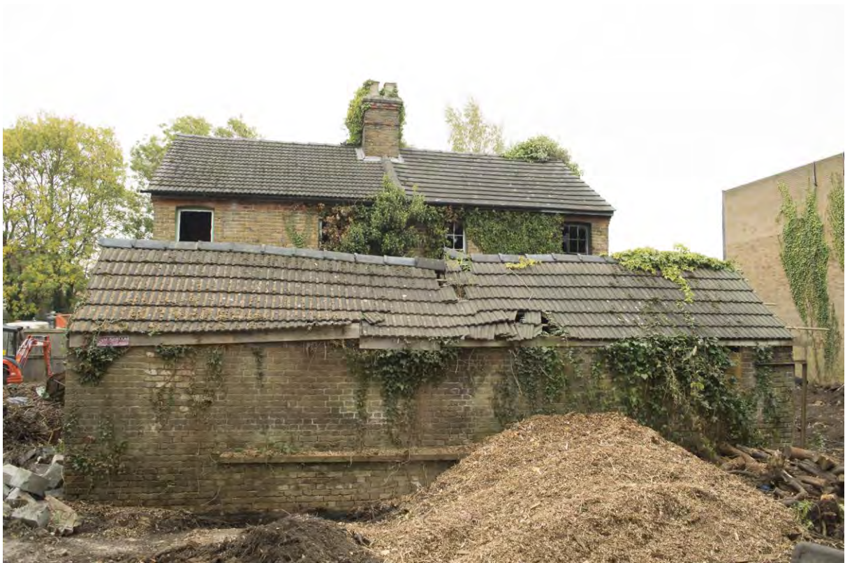
Plate 13 – North west (or rear) elevation of the outbuildings (HR117- 0008)
