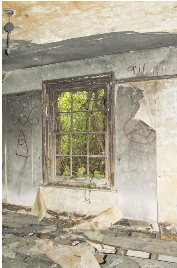
Plate 25 – The window, room 6, no. 15 (HRI17-0085)
