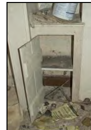
HR117-0099 Detail of fitted cabinet, room 2. Facing north-east
