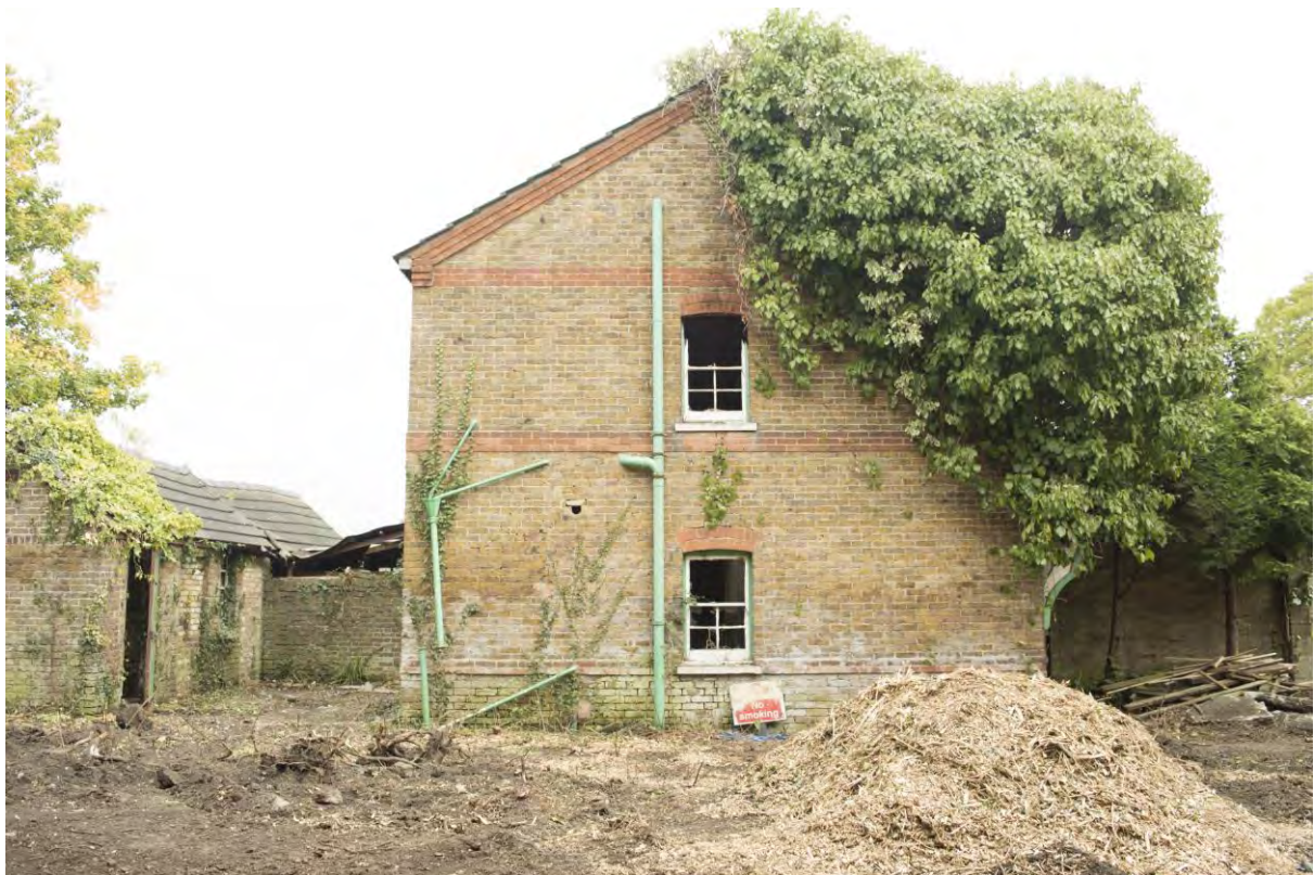
Plate 6 – South west elevation of no. 15 (HRI17- 0016)
