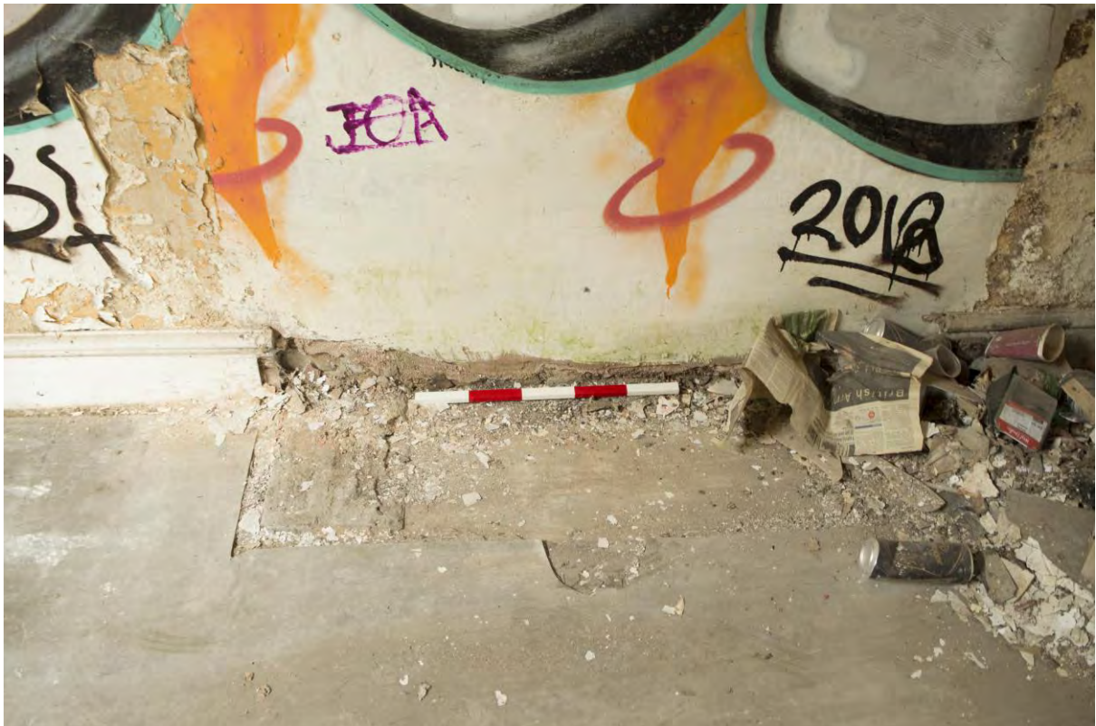
Plate 40 – One of the former chimney breast locations, room 9, no. 17 (HRI17- 0051)
