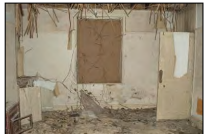
HR117-0102 Interior of room 2. Facing south-east
