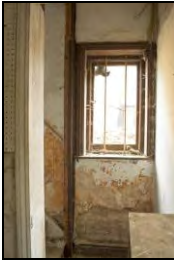
HR117-0061 Interior of room 10. Facing north-east
