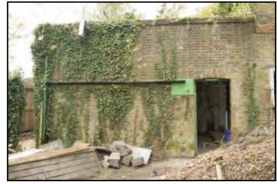
HR117-0033 NE elevation of the shop extension to n. 17. Facing south-west
