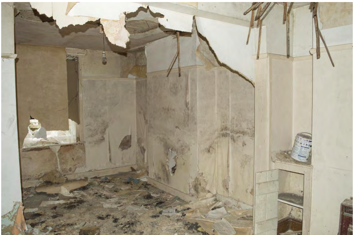
Plate 16 – The interior of room 2, no. 15 (HRI17-0096)
