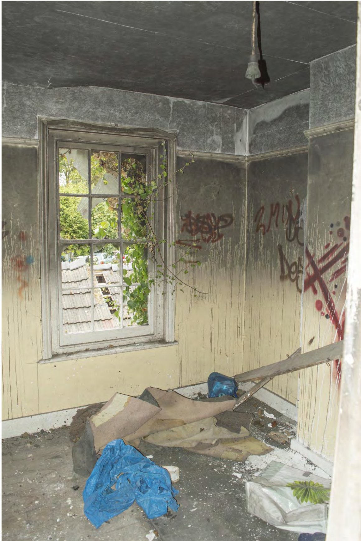
Plate 27 – Room 8, no. 15 (HRI17-0081)
