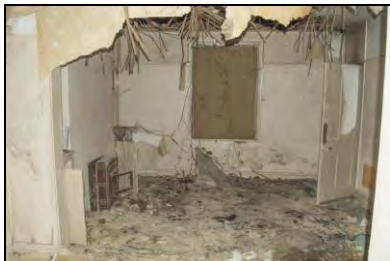
HR117-0097 Interior of room 2. Facing south-east
