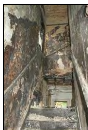
HR117-0104 Interior of stairwell (room 1) n. 15. Facing north-west
