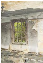
HR117-0085 Interior of room 6. Facing east
