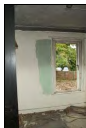
HR117-0074 Interior of room 19. Facing north
