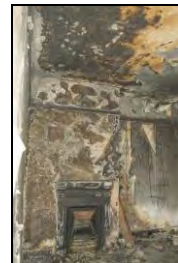
HR117-0087 Interior of room 6. Facing north-east
