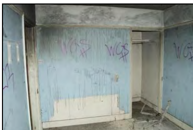
HR117-0073 Interior of room 17. Facing north-east
