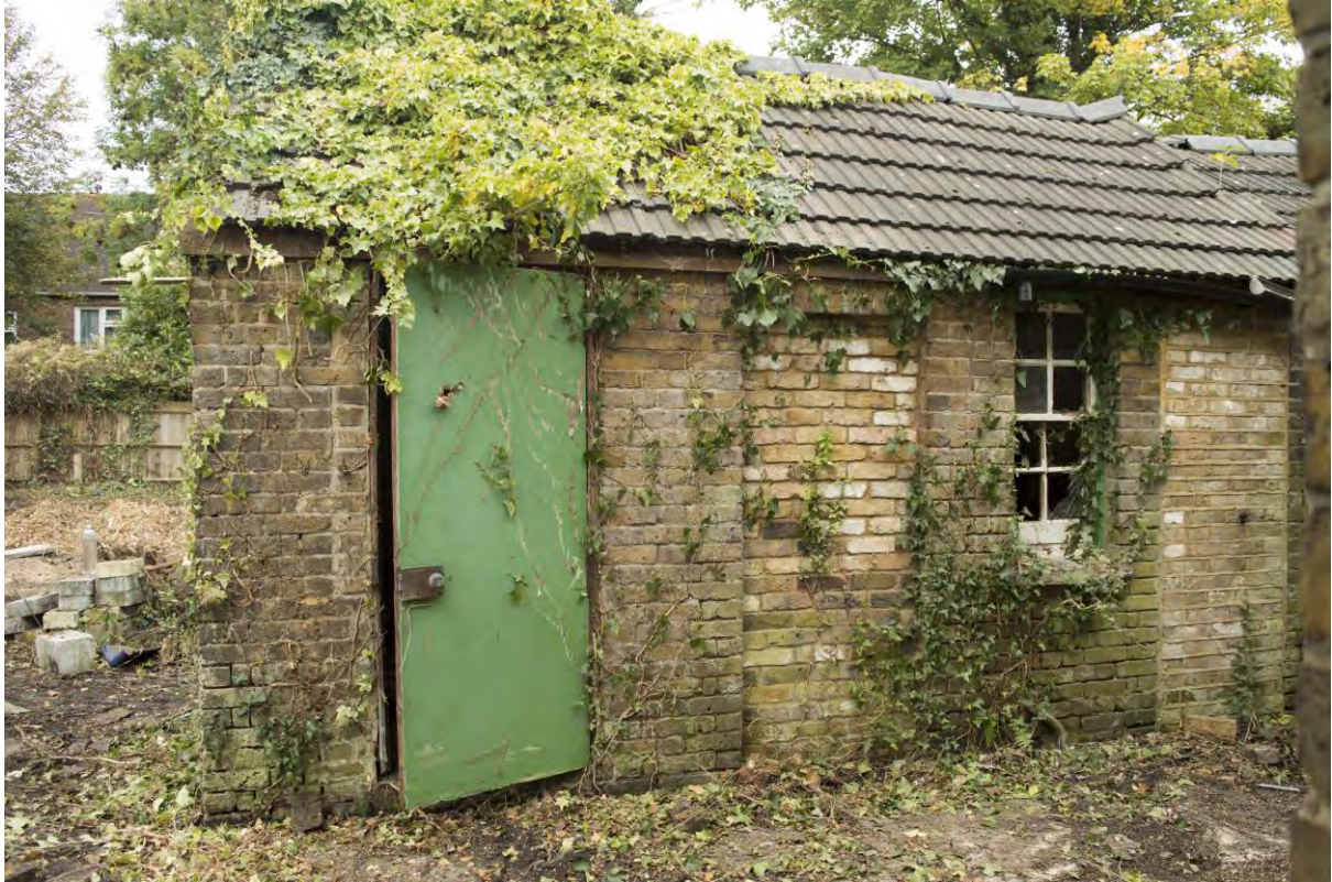
Plate 11 – South east elevation of the outbuilding, no. 15 (HRI17-0013)
