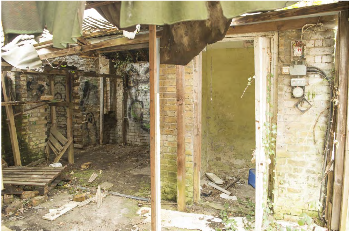
Plate 43 – Rooms 14 and 16, no. 17 (HR117- 0038)
