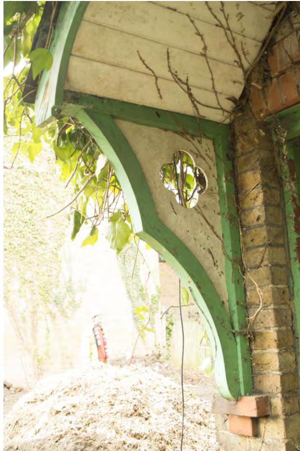
Plate 5 – Detail of the porch canopy construction (HRI17 0028)
