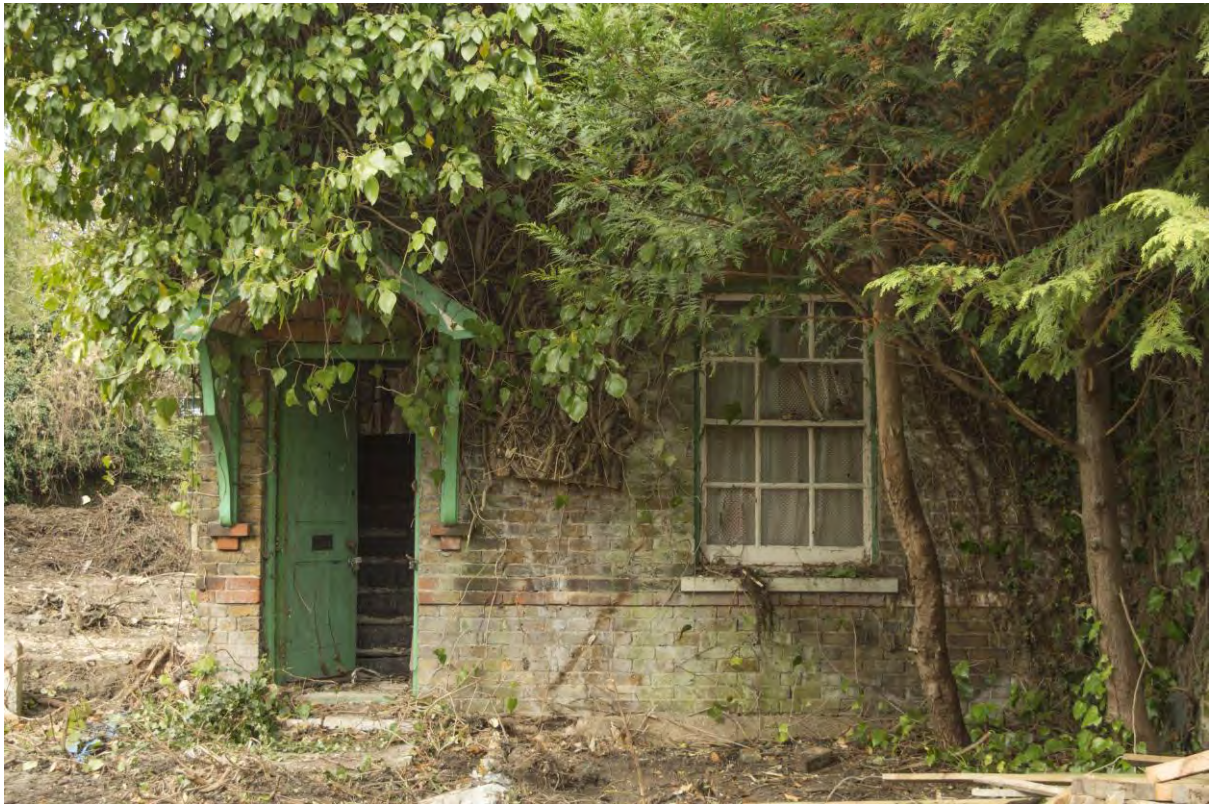
Plate 1 – The principal elevation of no.15 (HR117-0020)
