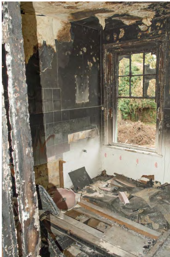
Plate 26 – Room 7, no. 15 (HRI17-0083)
