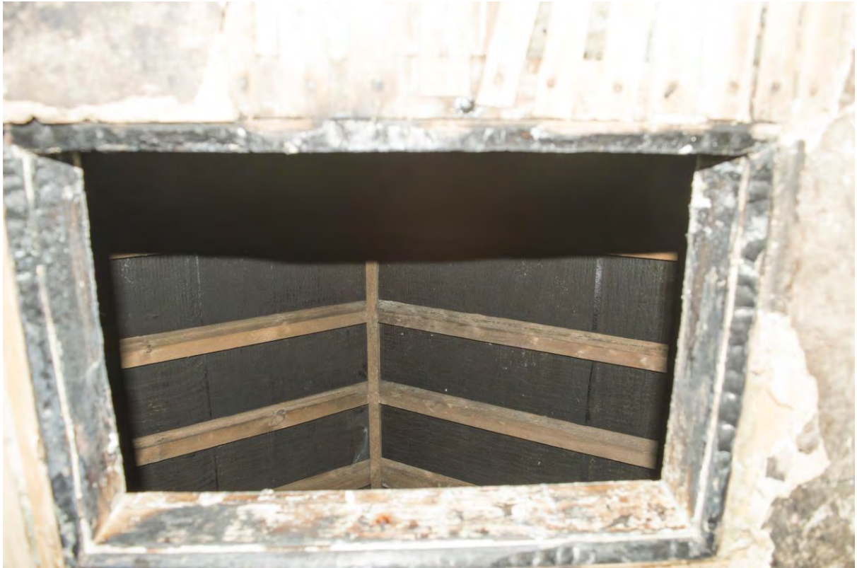
Plate 28 – The roof construction, no. 15 (HRI17-0086)
