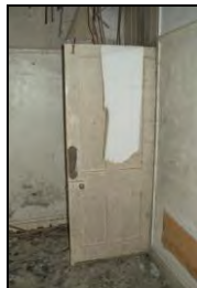
HR117-0098 Internal door, room 2. Facing south-west
