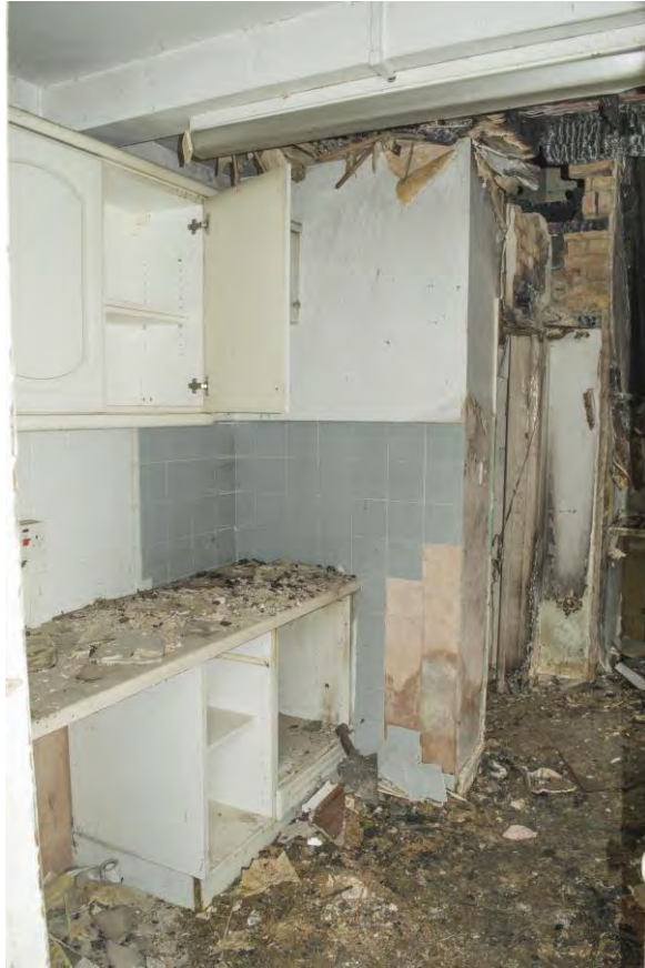
Plate 19 – The interior of room 3, no. 15 (HRI17-0089)
