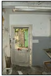
HR117-0092 Interior of room 3. Facing north-west
