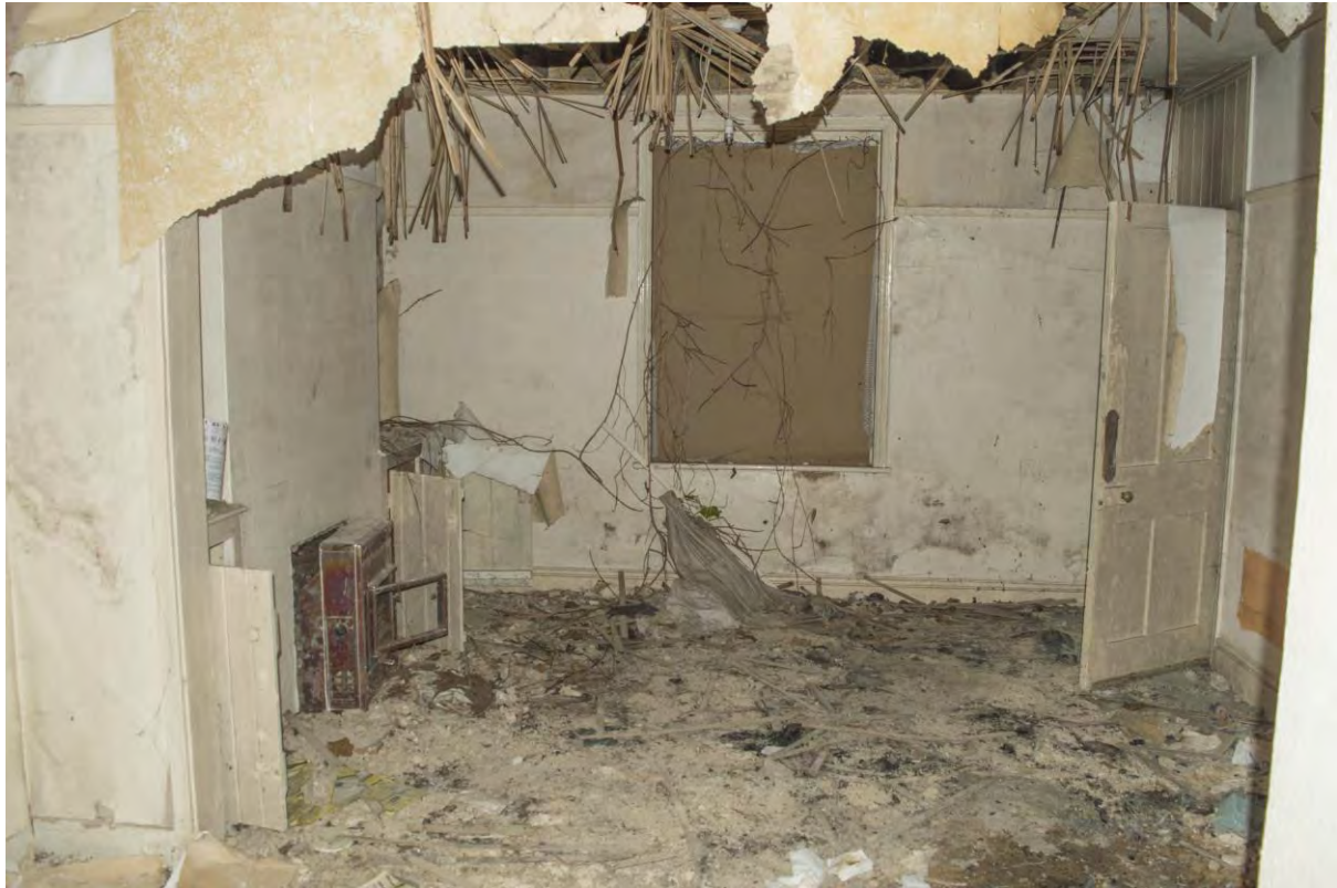
Plate 17 – The interior of room 2, no. 15 (HRI17-0097)
