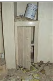
HR117-0100 Detail of fitted cabinet, room 2. Facing north-east
