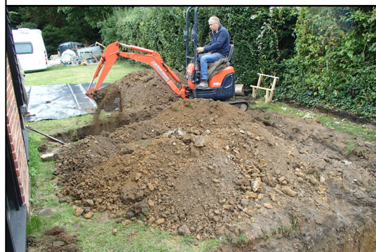
The foundation trench during excavation
