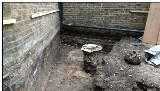
Ground reduction in southwest corner, detailing modern drain and wall [1009]
