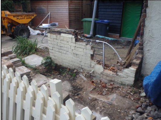
Site view prior to groundworks, looking north-east
