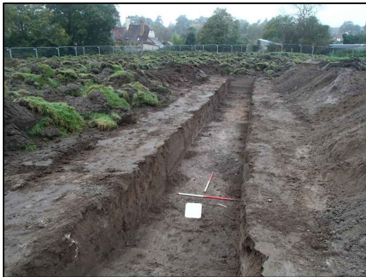
Trench 3, looking west
