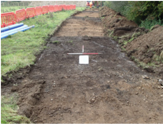
Excavations for new reservoir, looking north
