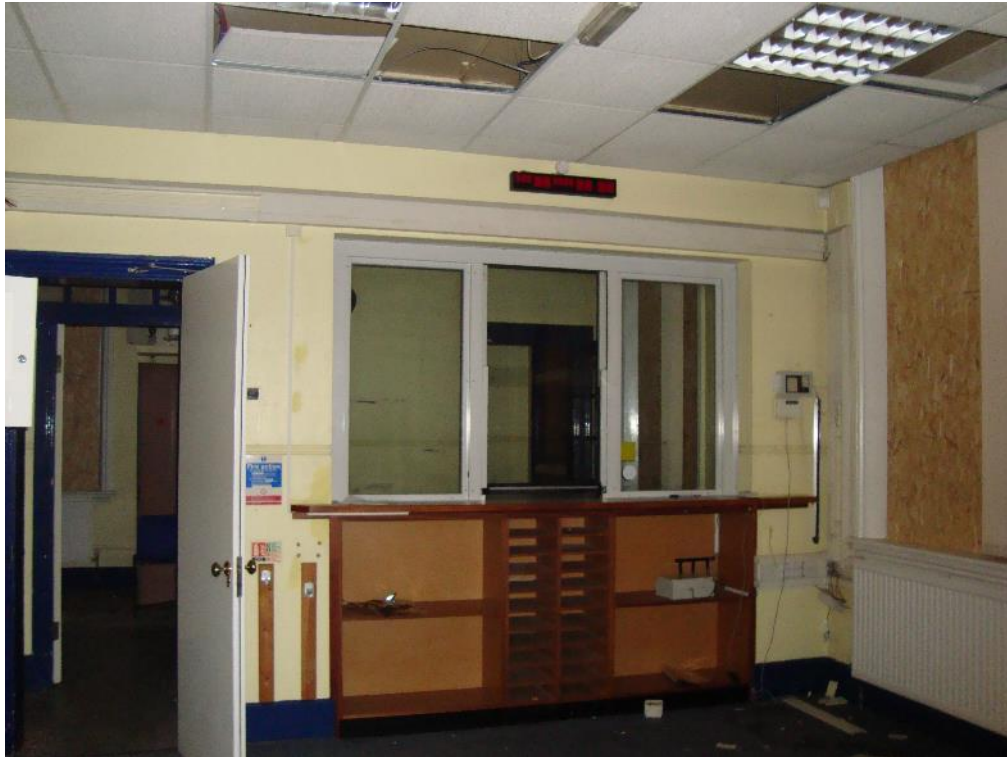
Plate 25: Station, Range 1, Room 6, note inserted enquiry counter, facing north-west (CgMs_0125)
