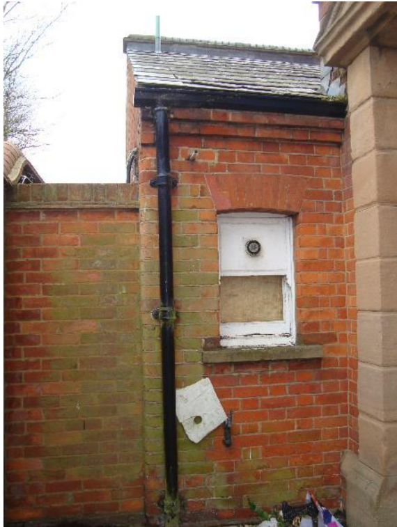
Plate 55: Station, Range 3, north-east elevation, facing south-west (CgMs_0211)
