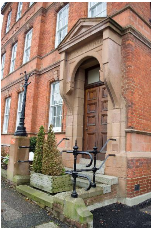
Plate 2: Station, Range 1, principal doorway within the north-east elevation, facing south-east (170859_0040)
