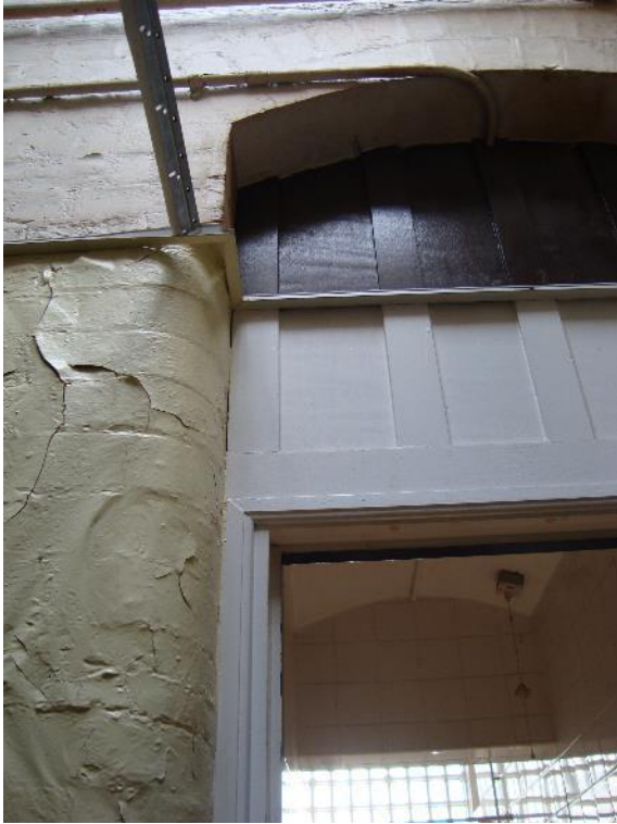
Plate 51: Station, Range 2, Room 21, door jamb detail, facing south-east (CgMs_0251)
