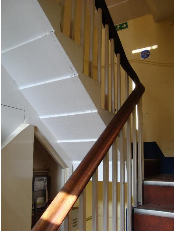
Plate 27: Station, Range 1, Room 8, south-east side entrance, facing south-west (CgMs_0134)
