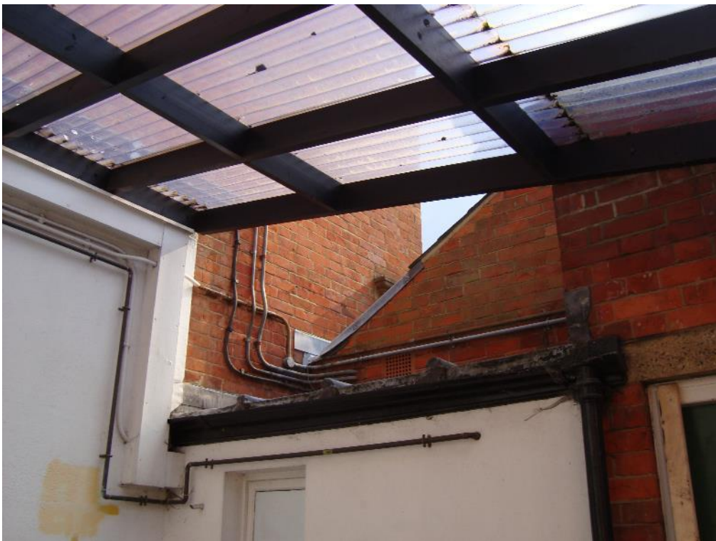
Plate 54: Station, Range 3, roof detailing, facing east (CgMs_0184)
