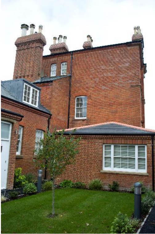
Plate 9: Station, rear south-west elevation, facing north (170859_0069)
