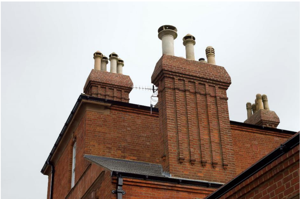
Plate 10: Station, Ranges 1 and 2, chimneystack detail, facing north-east (170859_0077)
