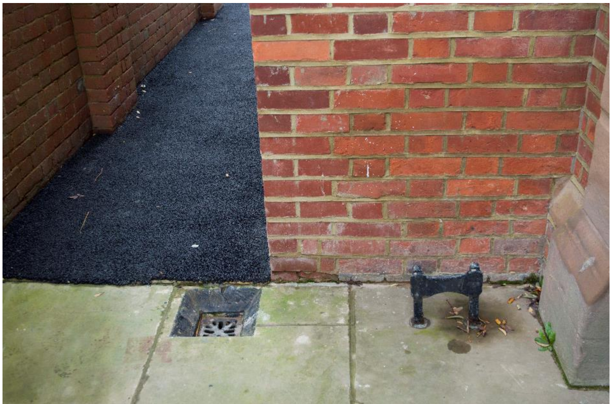
Plate 8: Station, Ranges 1 and 2, boot-scraper detail adjacent the south-east doorway, facing south-west (170859_0059)
