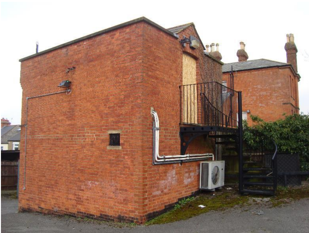
Plate 64: Hay Loft (stable), south-east elevation, facing north-west (CgMs_0189)
