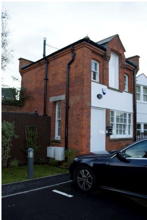
Plate 62: Hay Loft (stable), north-east elevation, facing south (170859_0088)
