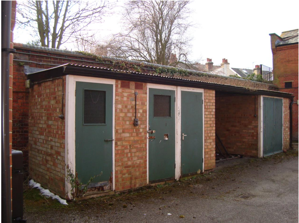
Plate 65: Photograph of the demolished structure formerly located within the rear yard along the site's south-eastern boundary, facing south-east (CgMs_0182)
