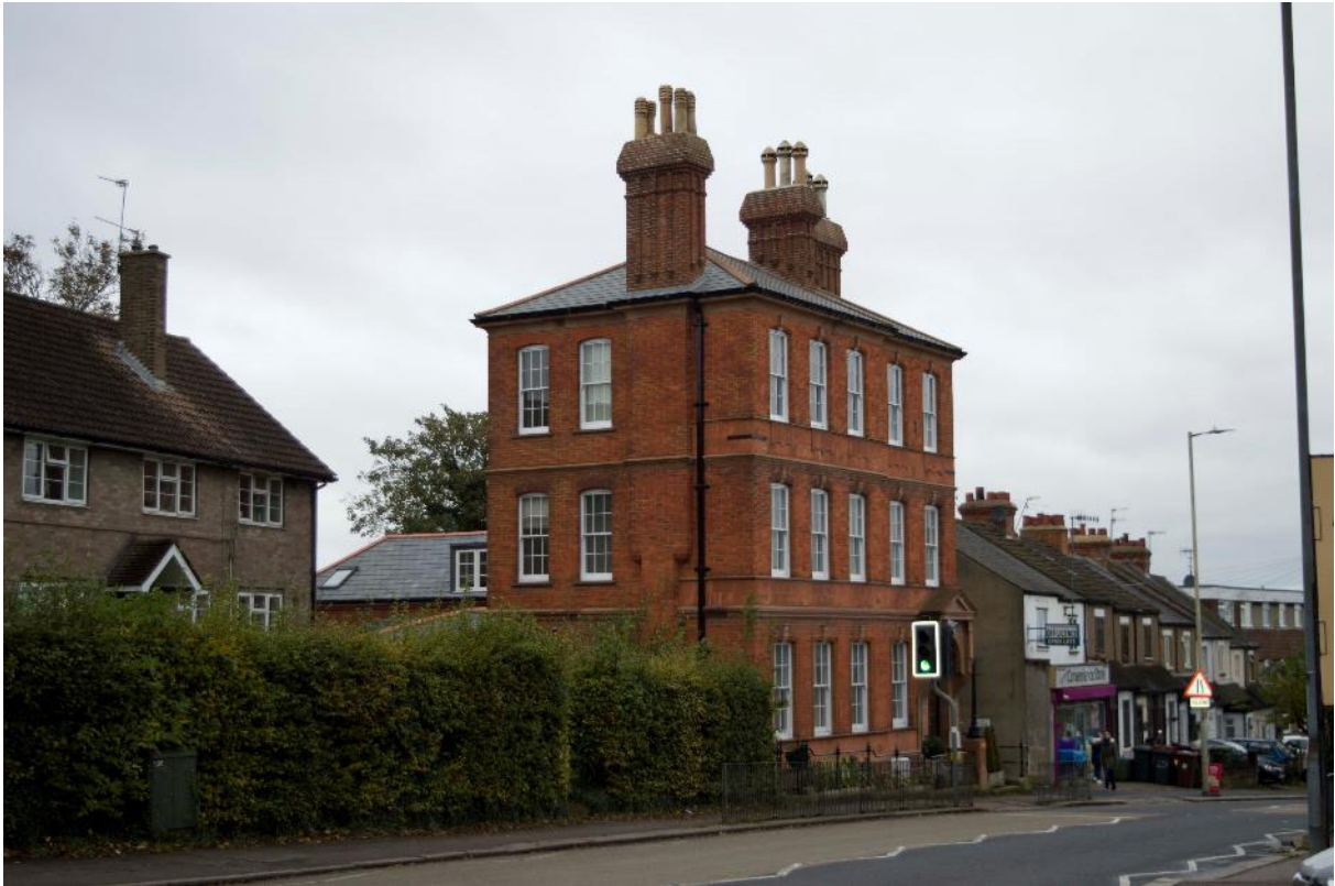
Plate 5: Station, Range 1, south-east elevation, facing west (170859_0027)
