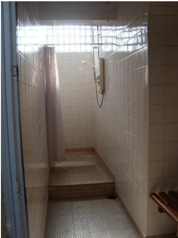
Plate 50: Station, Range 2, Room 21, facing south-east (CgMs_0252)
