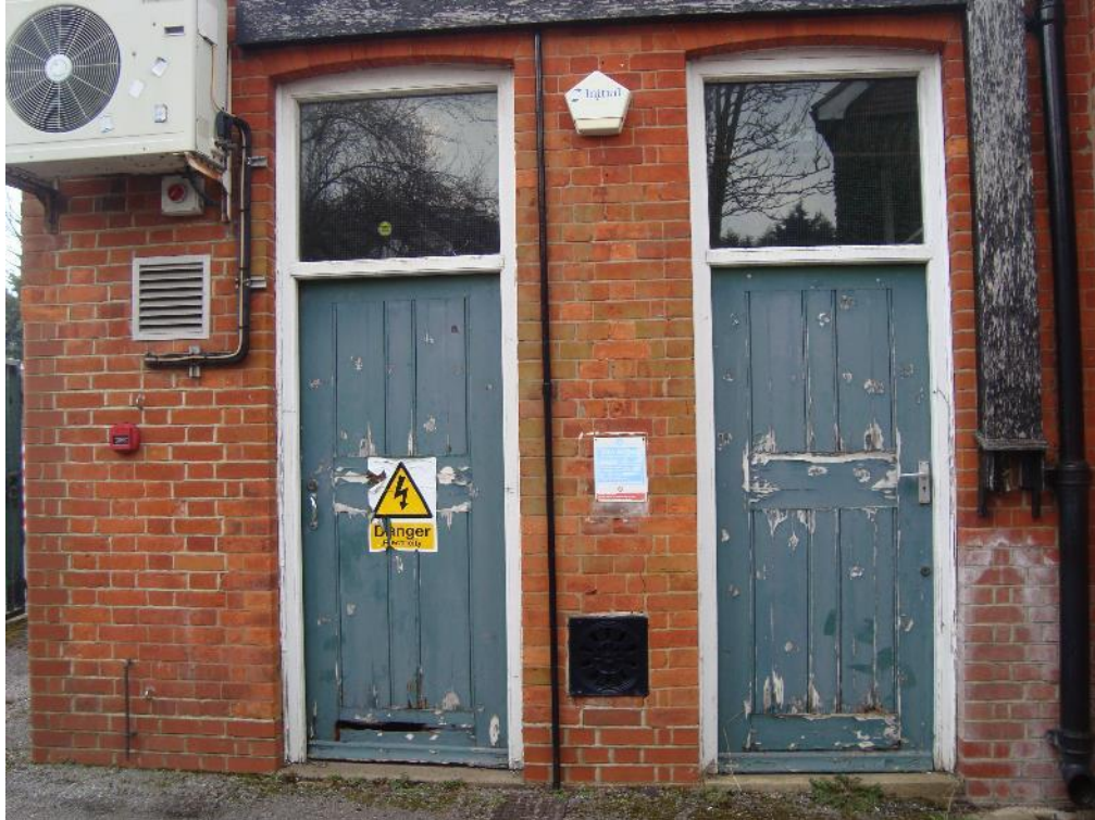
Plate 43: Station, Range 2, doorway openings within the south-east elevation, facing north-west (CgMs_0202)
