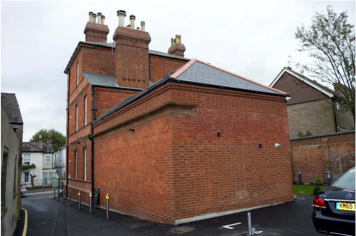
Plate 13: Station, Range 2, south-west elevation, facing north-east (170859_0075)
