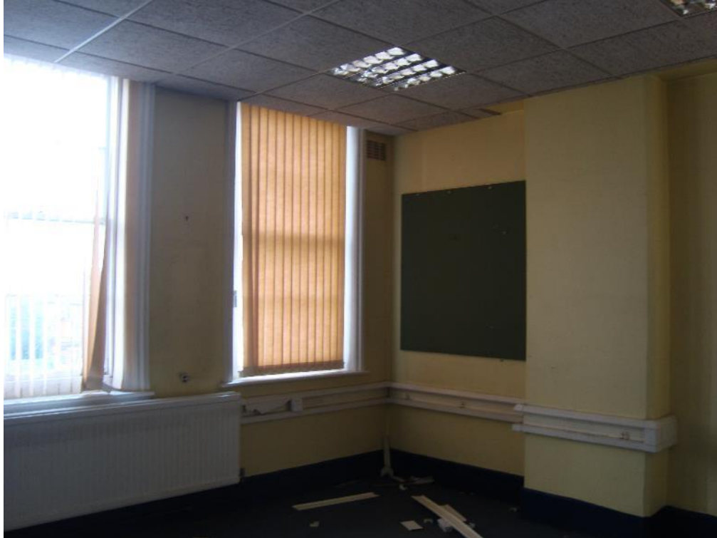
Plate 37: Station, Range 1, Room 14, note south-east chimneystack truncation, facing south-east (CgMs_0154)
