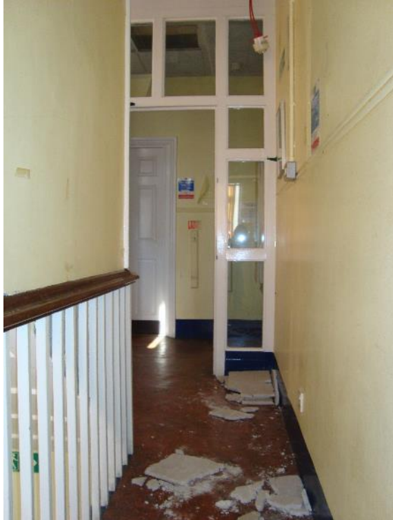
Plate 29: Station, Range 1, Room 9, first floor level stairwell partition, facing north-west (CgMs_0138)
