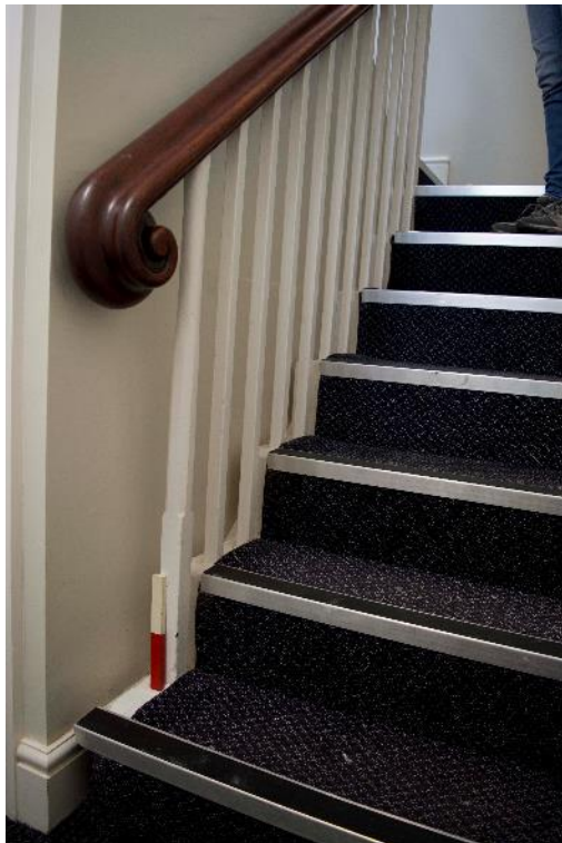
Plate 18: Station, Range 1, detail of stairwell and handrail, facing west (170859_0068)
