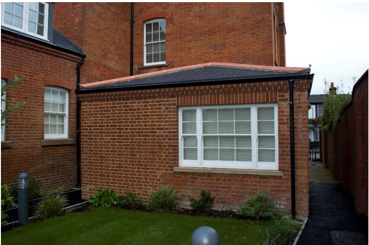
Plate 14: Station, Range 3, south-west elevation, facing north-east (170859_0062)
