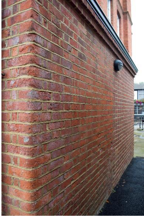
Plate 15: Station, Range 3, south-east elevation phasing, facing north (170859_0061)
