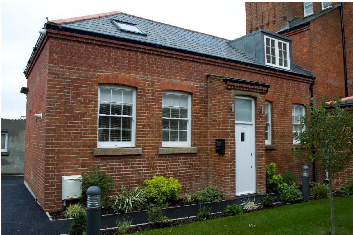
Plate 12: Station, Range 2, south-east elevation, facing north-west (170859_0071)
