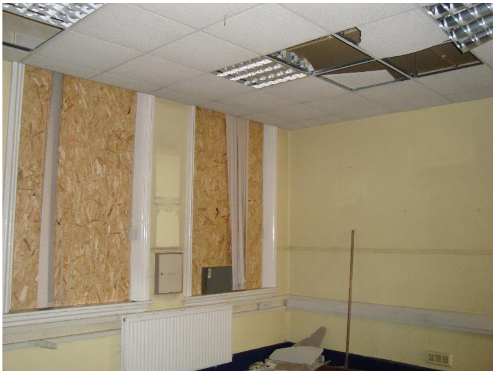
Plate 26: Station, Range 1, Room 6, window architrave detailing, facing south (CgMs_0124)
