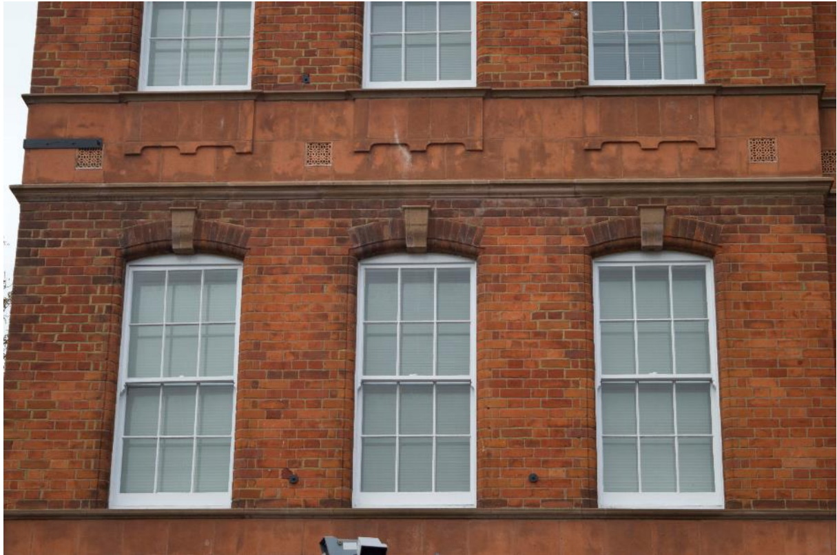
Plate 3: Station, Range 1, first floor window detail, facing south-west (170859_0037)
