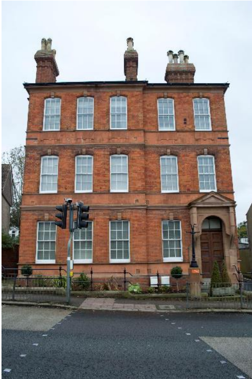
Plate 1: Station, Range 1, north-east elevation, facing south-west (170859_0020)
