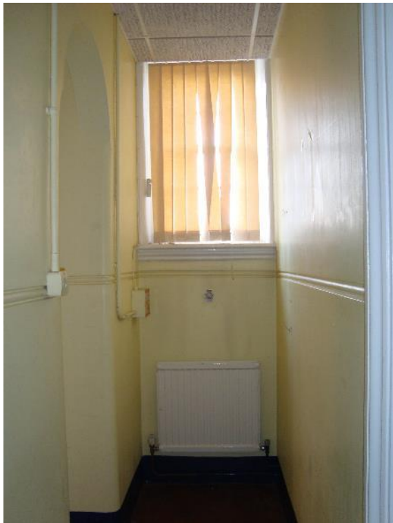
Plate 38: Station, Range 1, Room 15, facing south-west (CgMs_0156)
