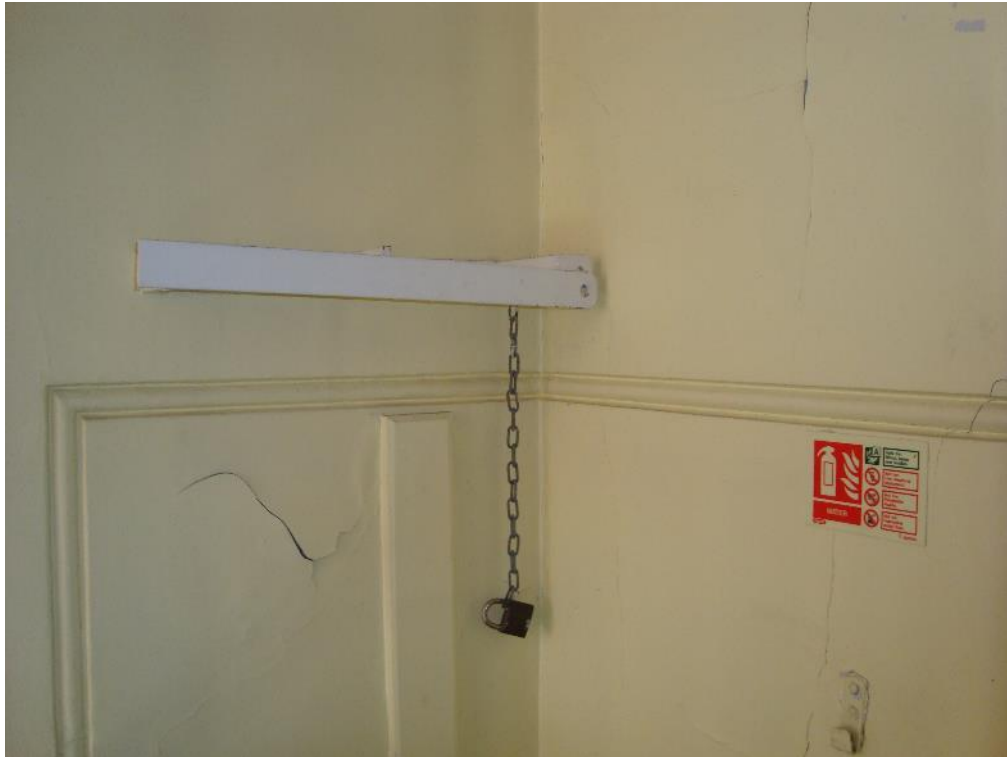
Plate 35: Station, Range 1, second floor level stairwell, integral dado rail detailing, facing south-west (CgMs_0152)
