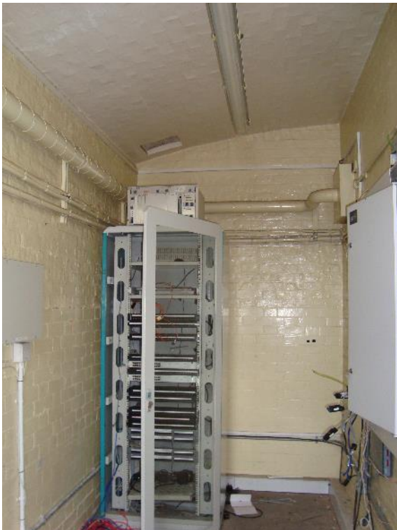
Plate 52: Station, Range 2, Room 23, facing north-west (CgMs_0201)
