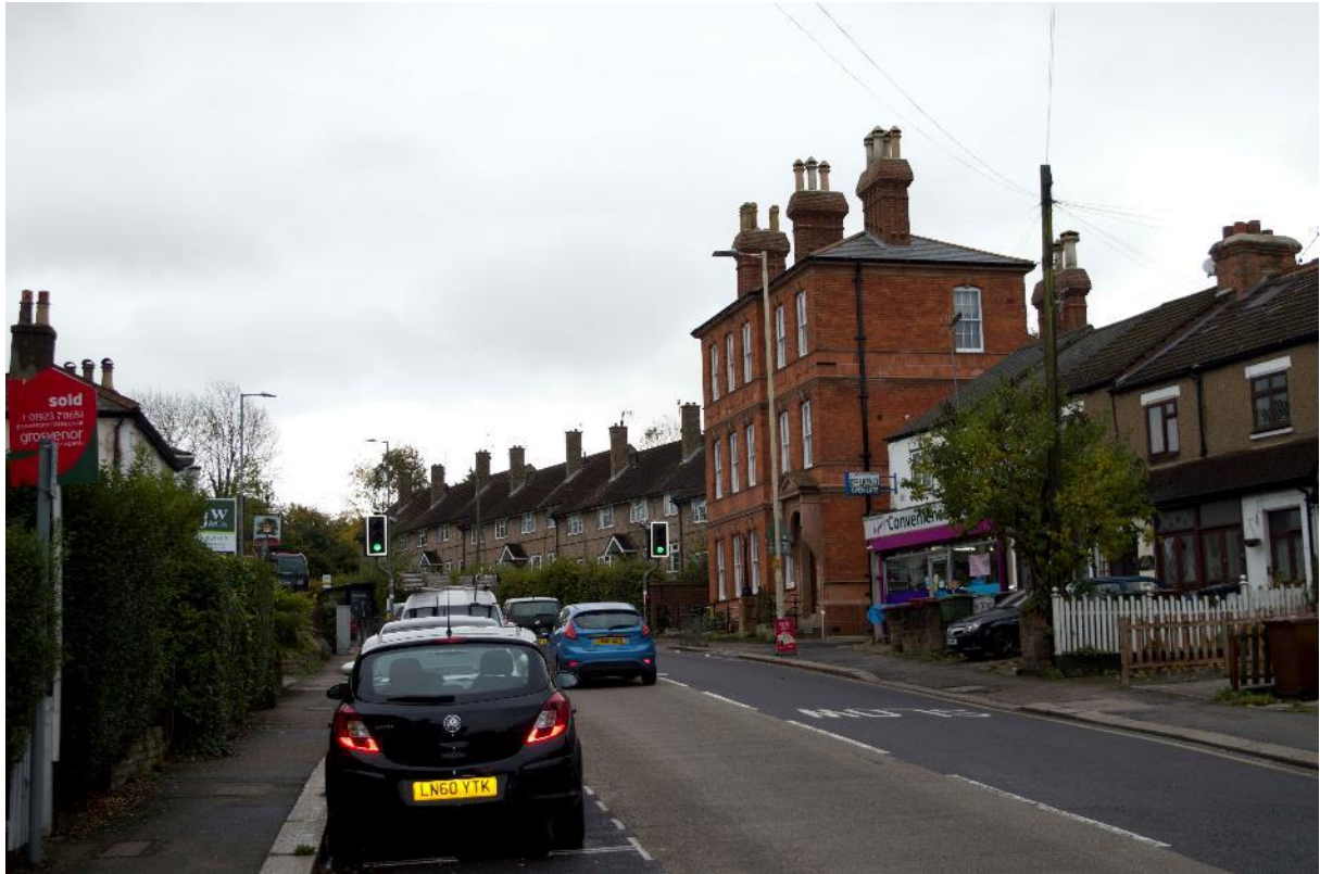
Plate 11: Station, Range 1, north-west elevation, facing south (170859_0031)
