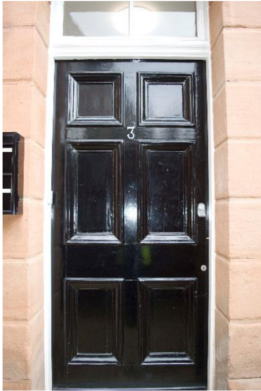
Plate 7: Station, Range 1, side entrance doorway, facing north-west (170859_0056)
