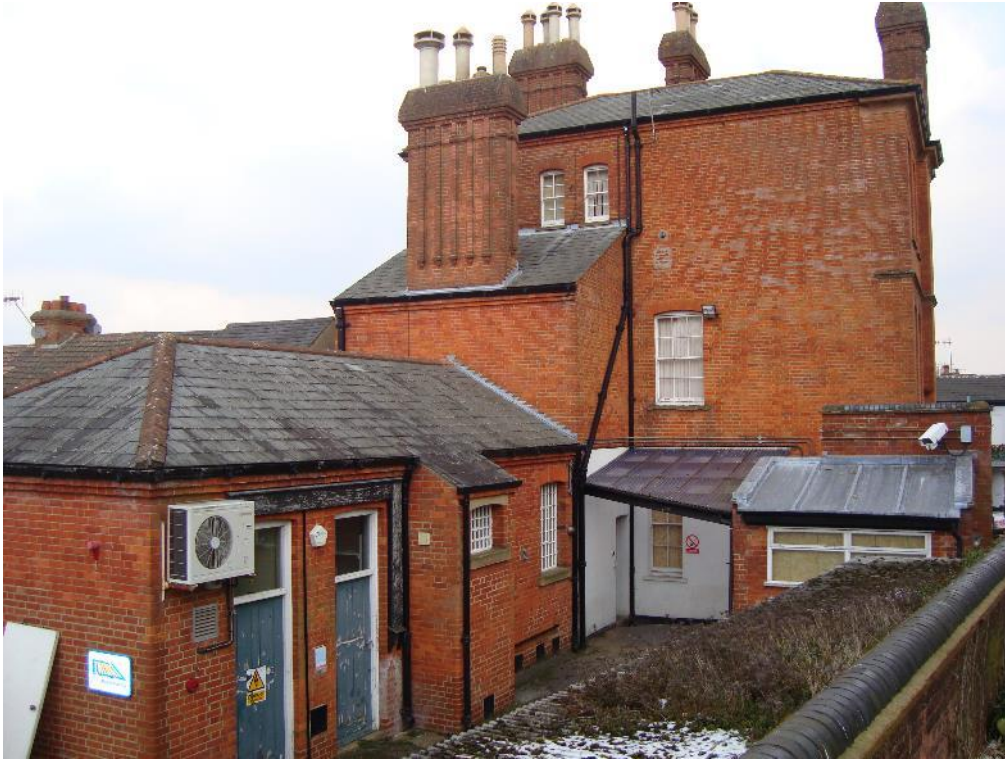
Plate 53: Station, Range 3, south-west elevation, facing north-east (CgMs_0190)
