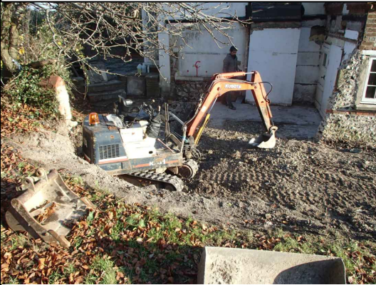
The site looking N
