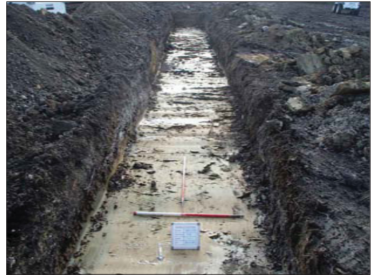
Trench 2, looking south
