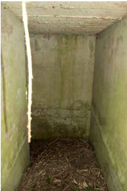
Plate 4: Structure 1, southern entrance, internal blast wall (0004)
