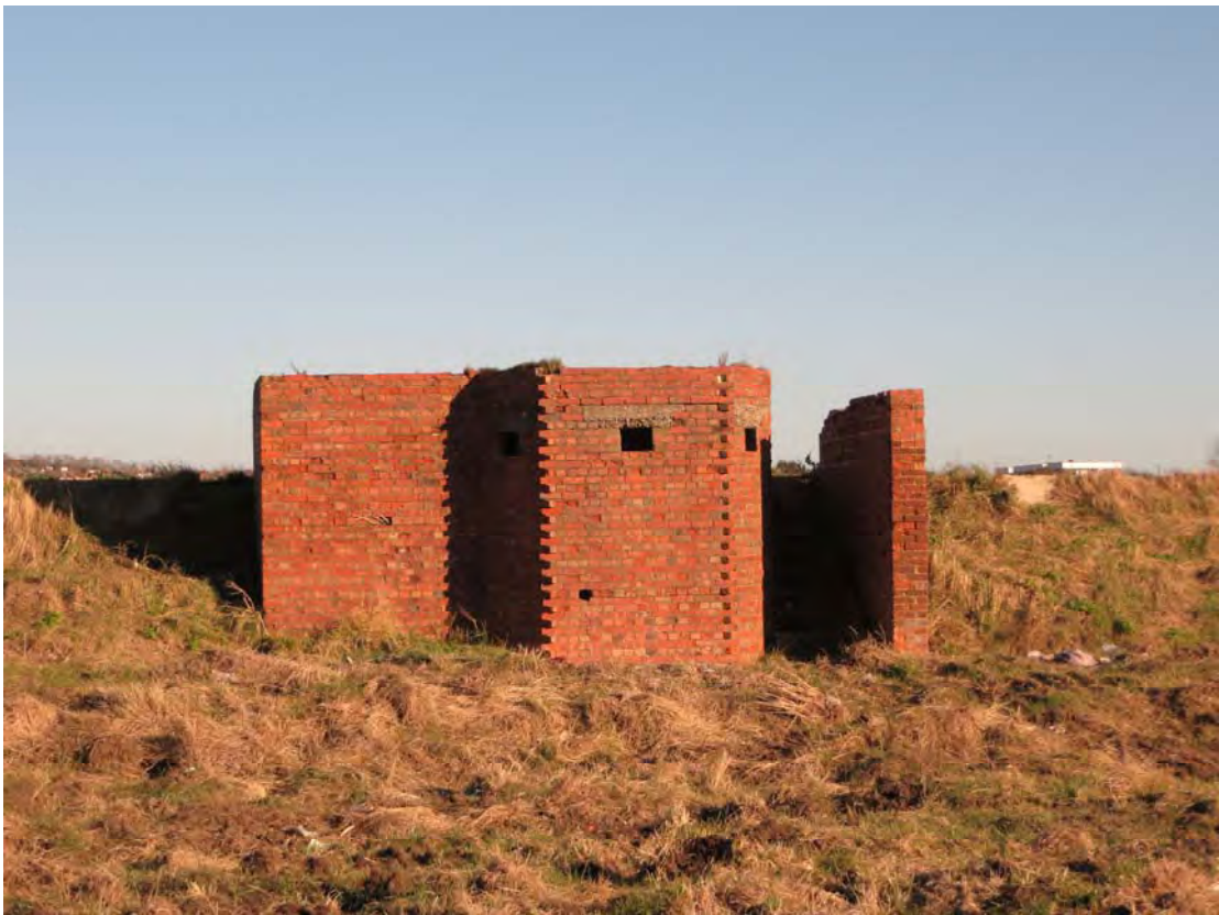
Plate 56: Structure 12, looking north-east (0330)
