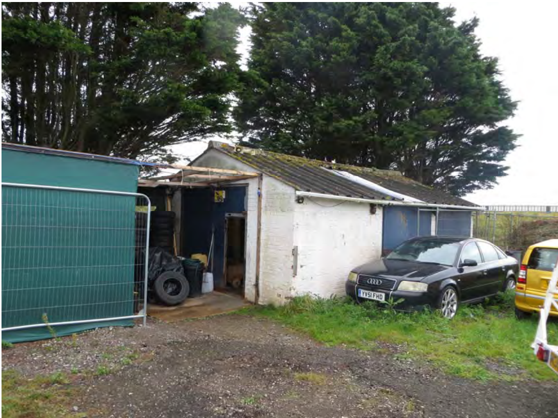
Plate 6: Structure 2, showing main entrance and boarded windows, looking south-east (0033)
