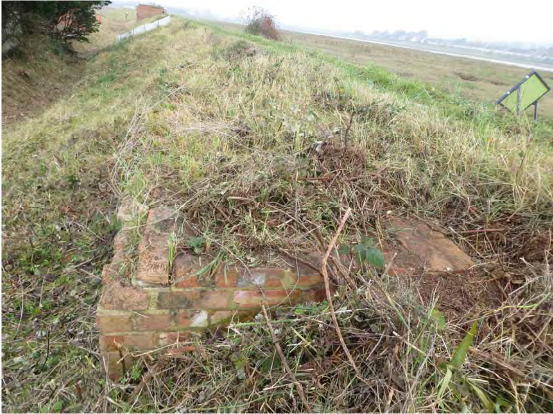
Plate 65: Structure 14 looking north-west (0356)
