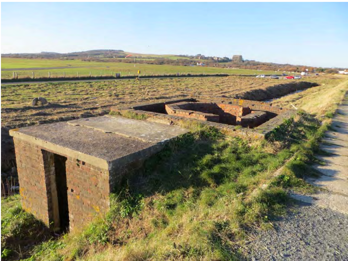
Plate 50: Structure 11 looking north-west (0279)
