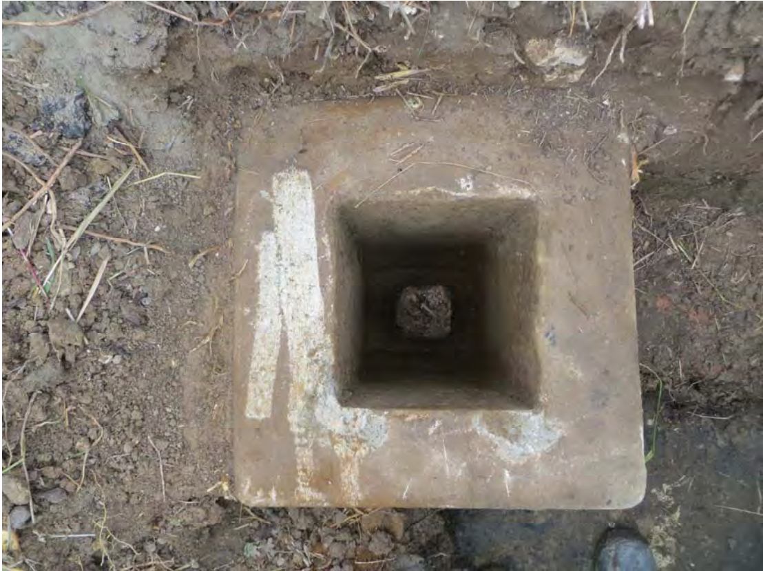
Plate 19: Structure 4, plan view of plinth window in-situ wooden post (0090)
