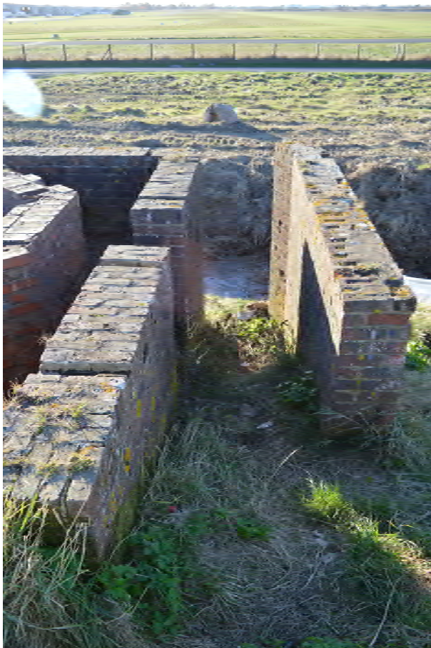
Plate 52: Structure 11, entrance, access steps and blast wall, looking west (0255)
