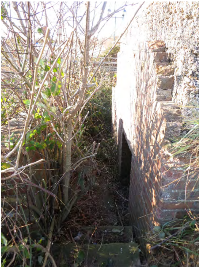
Plate 36: Structure 8, entrance, access steps and blast wall, looking west (0172)
