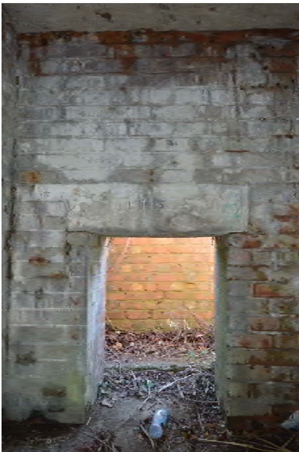
Plate 38: Structure 8, interior view of entrance, looking south (0164)
