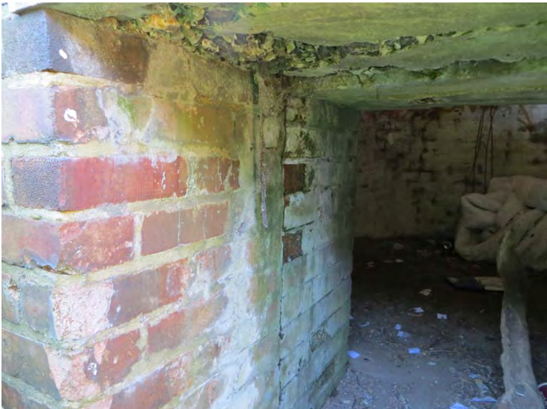
Plate 44: Structure 9 entrance passage, showing thickened wall on left and original wall on right (0229)
