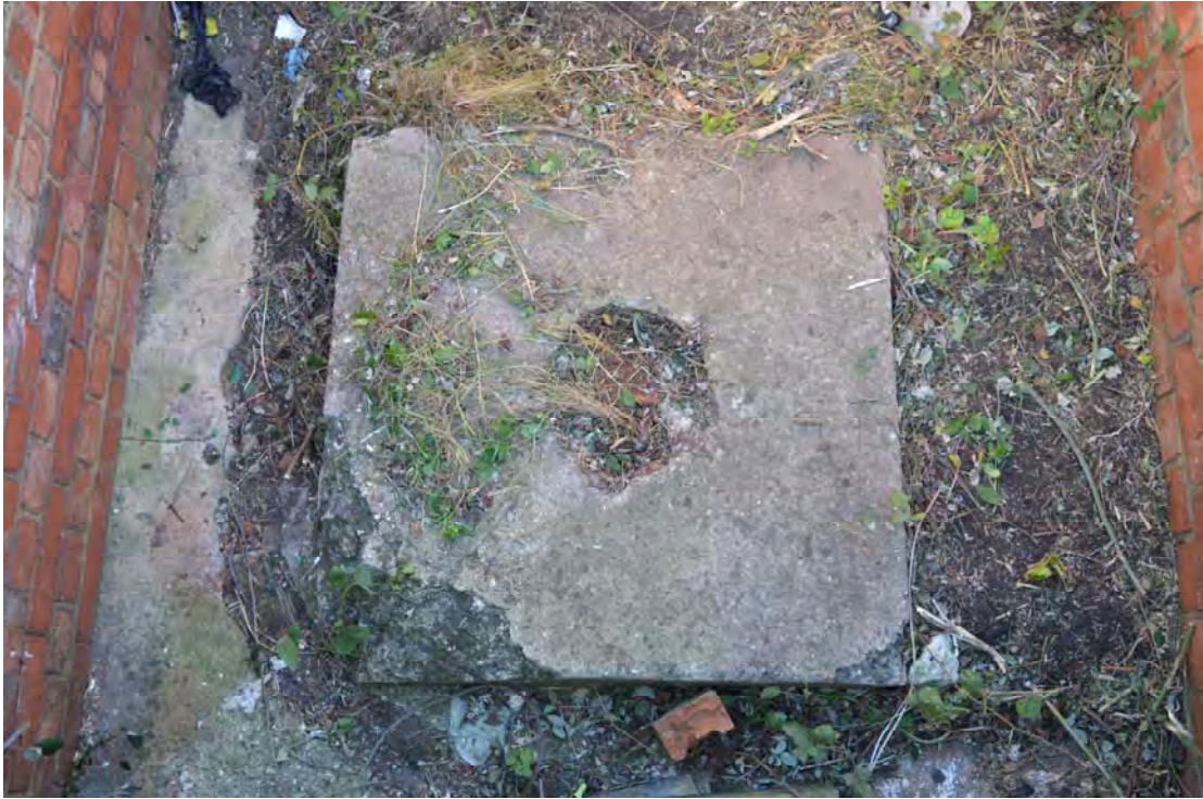
Plate 61: Structure 12, concrete base of light machine gun mount (0296)
