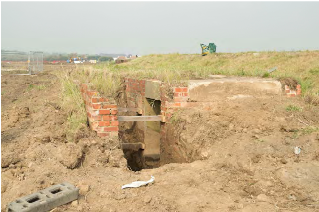
Plate 12: Structure 3, southern entrance and blast wall, looking north (0041)
