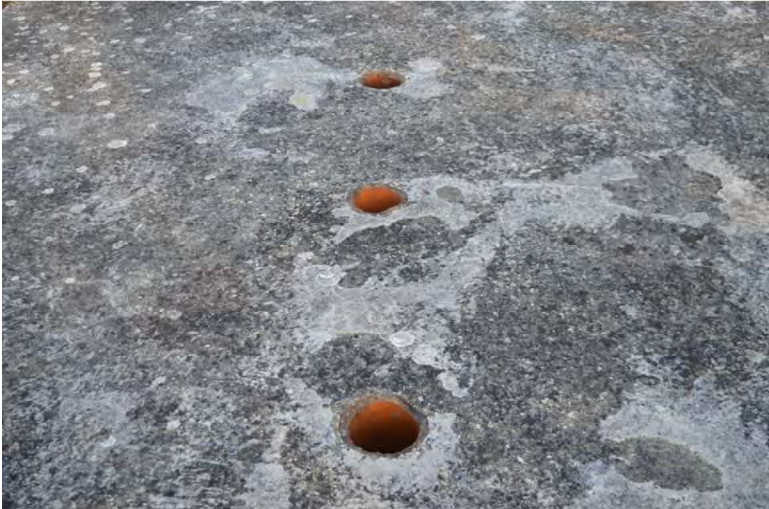
Plate 27: Structure 6, ventilation pipes in roof, looking north (0128)
