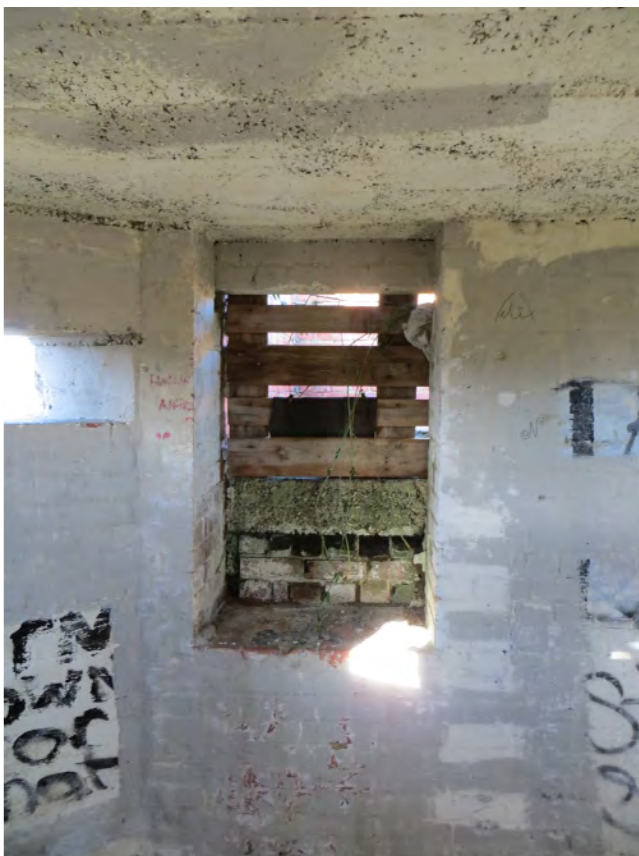
Plate 60: Structure 12, interior view of access to light anti-aircraft post, looking north-west (0320)
