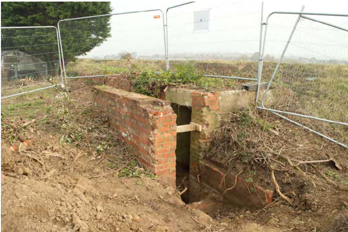
Plate 2: Structure 1, southern entrance and blast wall, looking north-east (0003)
