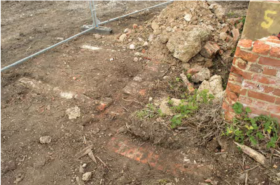
Plate 23: Structure 5, footings for southern blast wall and buttresses, looking west (0101)
