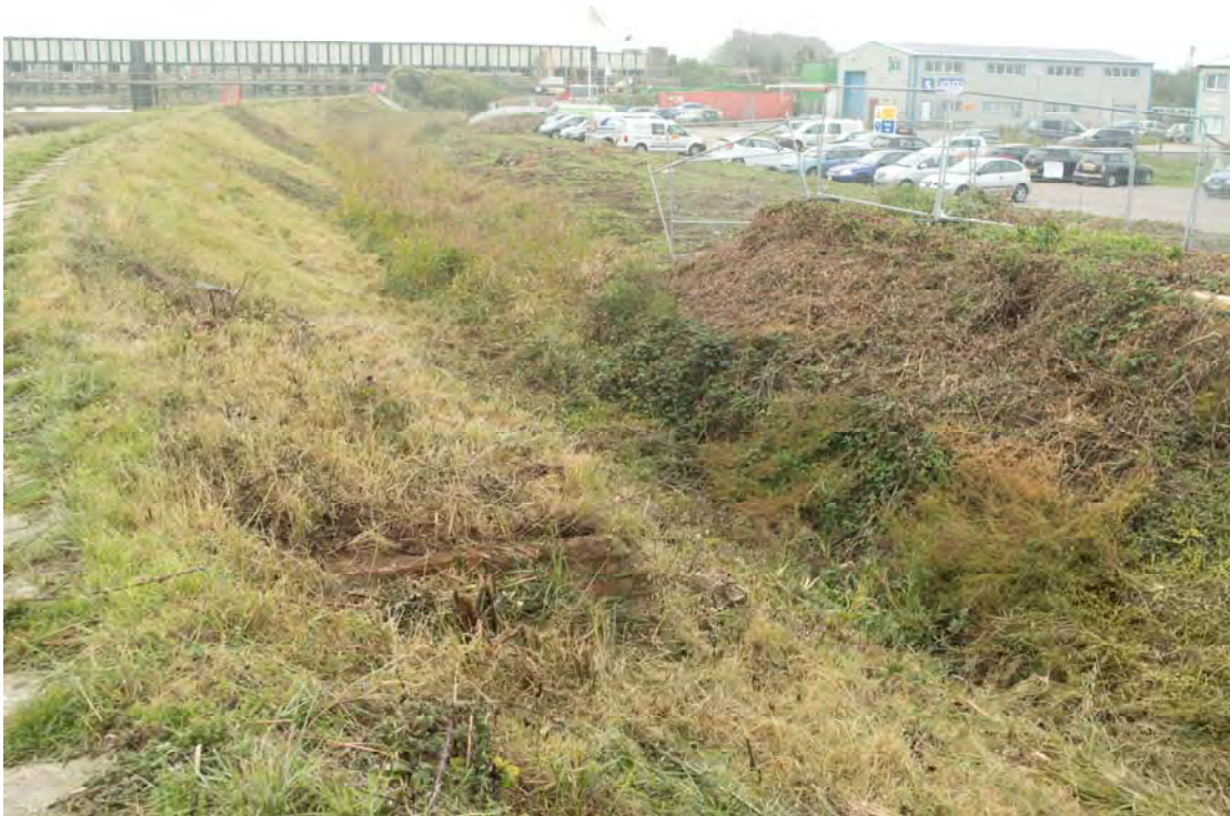
Plate 64: Structure 14 looking south-east (0351)
