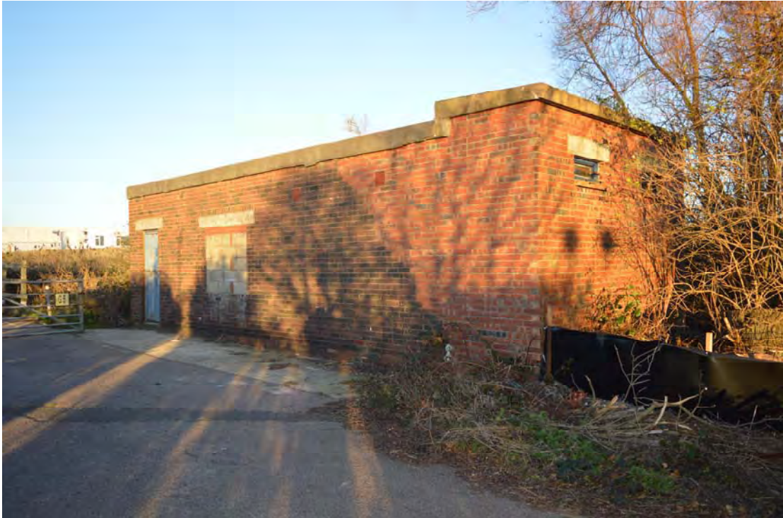
Plate 31: Structure 7, looking north-east, showing cell windows on right (0154)
