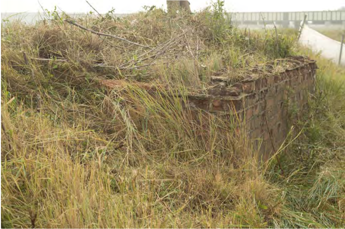
Plate 63: Structure 13 looking south-east (0343)
