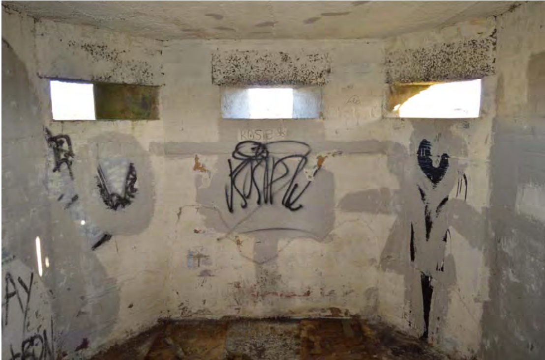
Plate 59: Structure 12, interior view of loopholes, looking north-east (0293)
