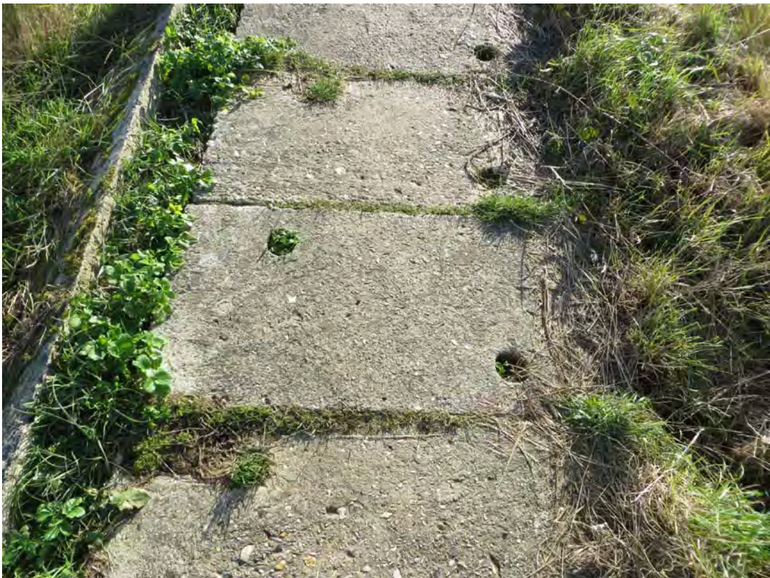
Plate 68: Structure 15 concrete, slabs showing repeating holes (0363)
