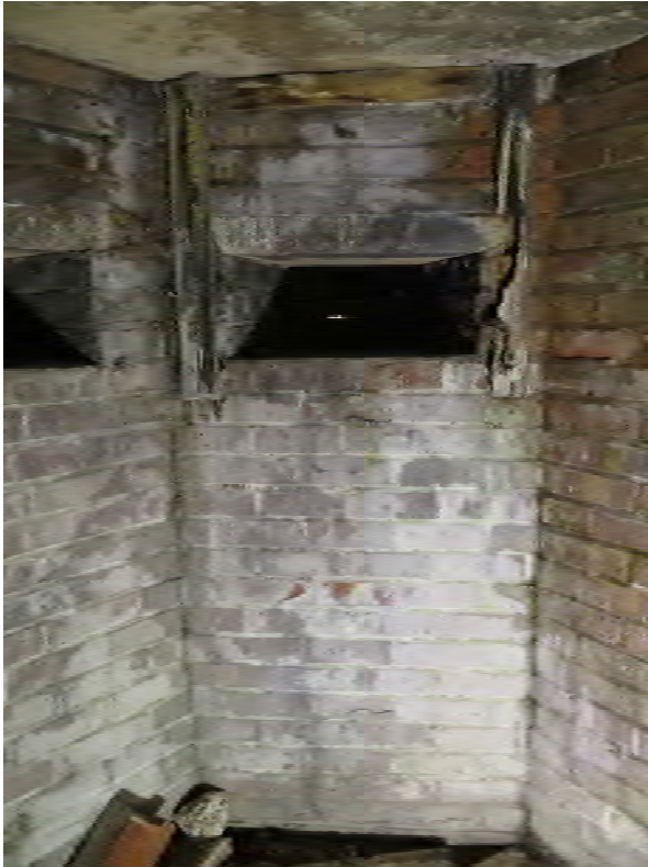
Plate 37: Structure 8, north facing loophole and remnant wooden shuttering (0176)
