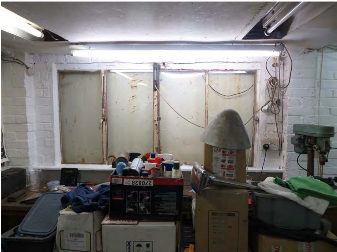
Plate 10: Structure 2, windows in centre of west wall, looking west (0026)
