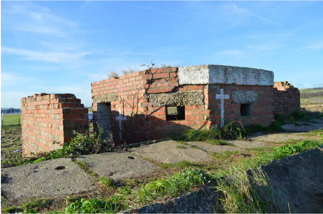
Plate 57: Structure 12 looking north-west, showing blast wall, entrance and concrete roof without brick shuttering (0290)
