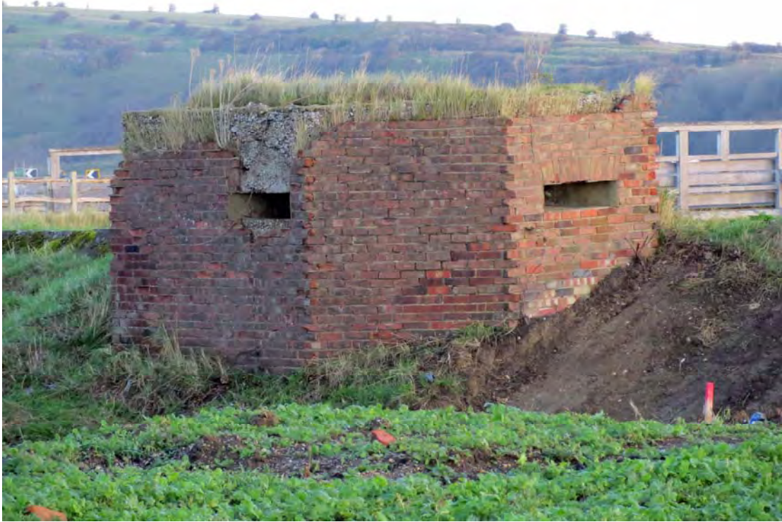
Plate 39: Structure 9, looking north-east (0235)
