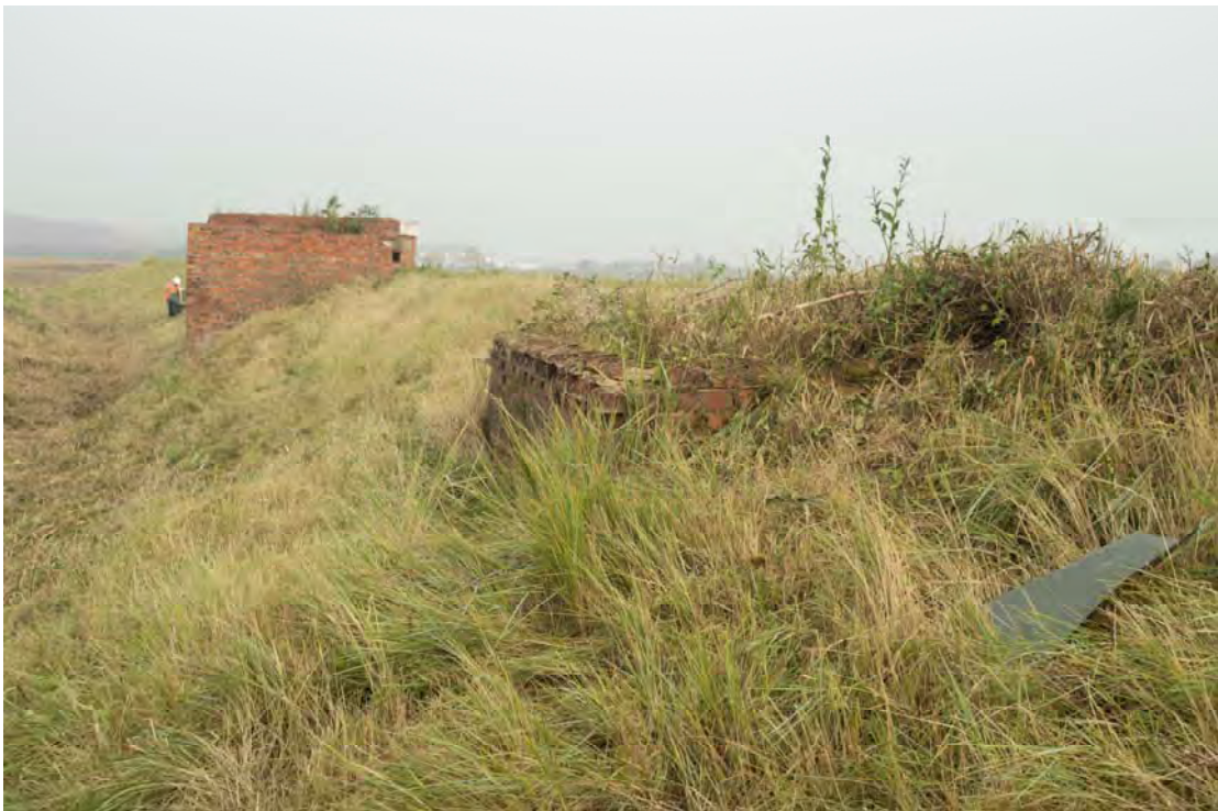
Plate 62: Structure 13 looking north-west (0341)
