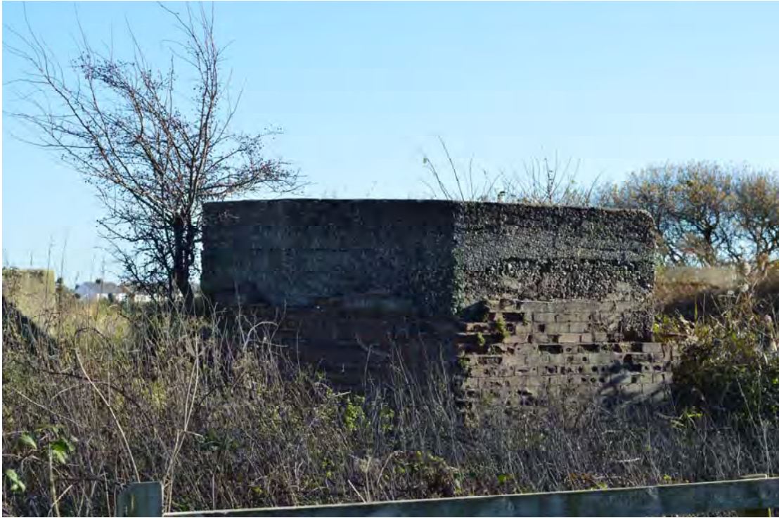
Plate 35: Structure 8, looking south-east (0169)
