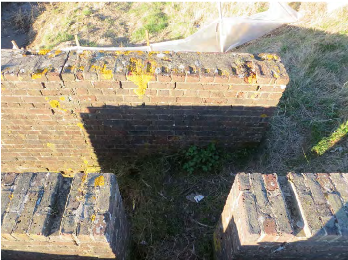
Plate 54: Structure 11, blast wall, showing original segment, covering only the entrance (0281)
