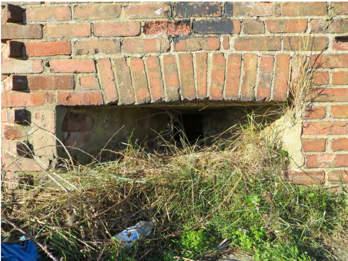
Plate 42: Structure 9, widened loophole, looking north-west (0216)
