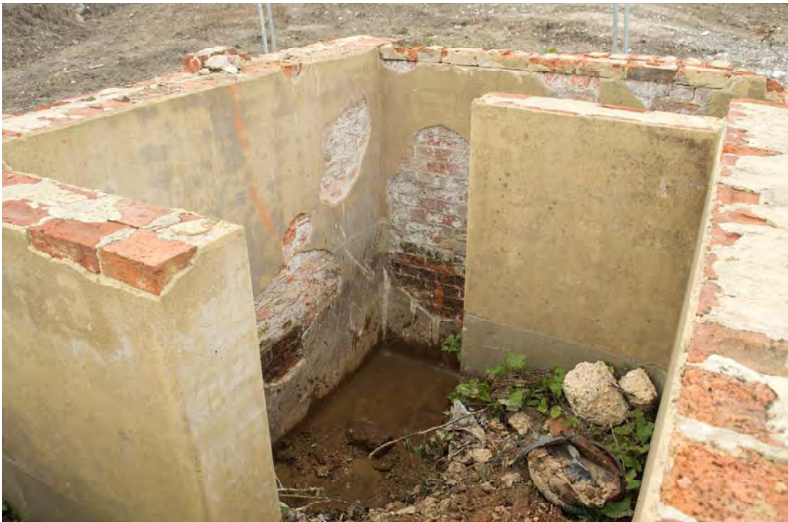
Plate 22: Structure 5, interior, showing fully excavated floor, looking north-east (0103)
