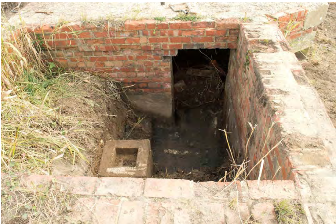
Plate 18: Structure 4, concrete plinth for light machine gun mount, looking south-east (0059)
