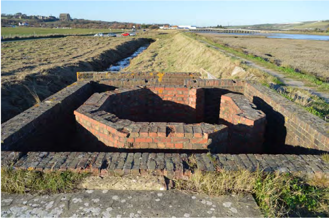
Plate 51: Structure 11, light anti-aircraft post, looking north (0256)
