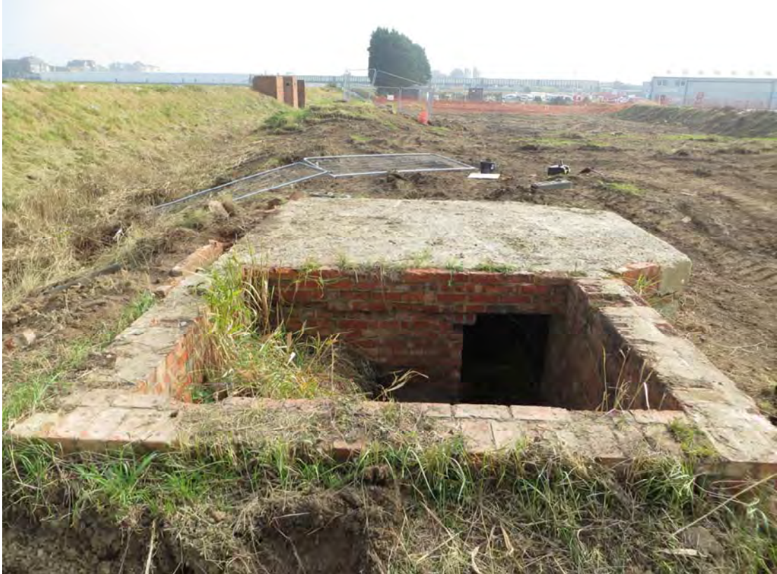
Plate 16: Structure 4, light-anti aircraft post and access door to pillbox, looking south-east (0075)
