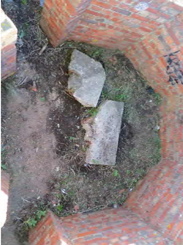
Plate 53: Structure 11, concrete fragments of light machine gun mount, with trace of earlier circular mount visible below (0278)
