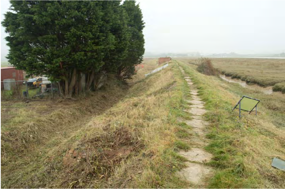
Plate 67: Structure 15 (footpath) looking north-west (0361)
