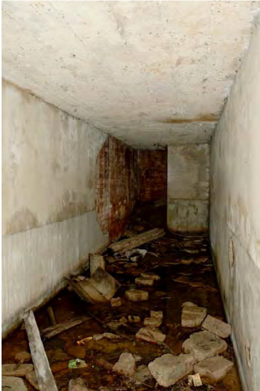
Plate 5: Structure 1, main chamber, looking north (0005)
