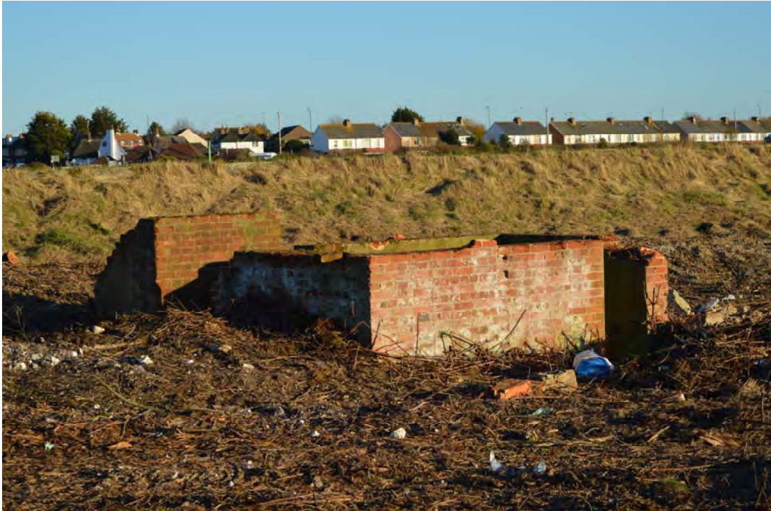
Plate 21: Structure 5, looking south-east (0107)
