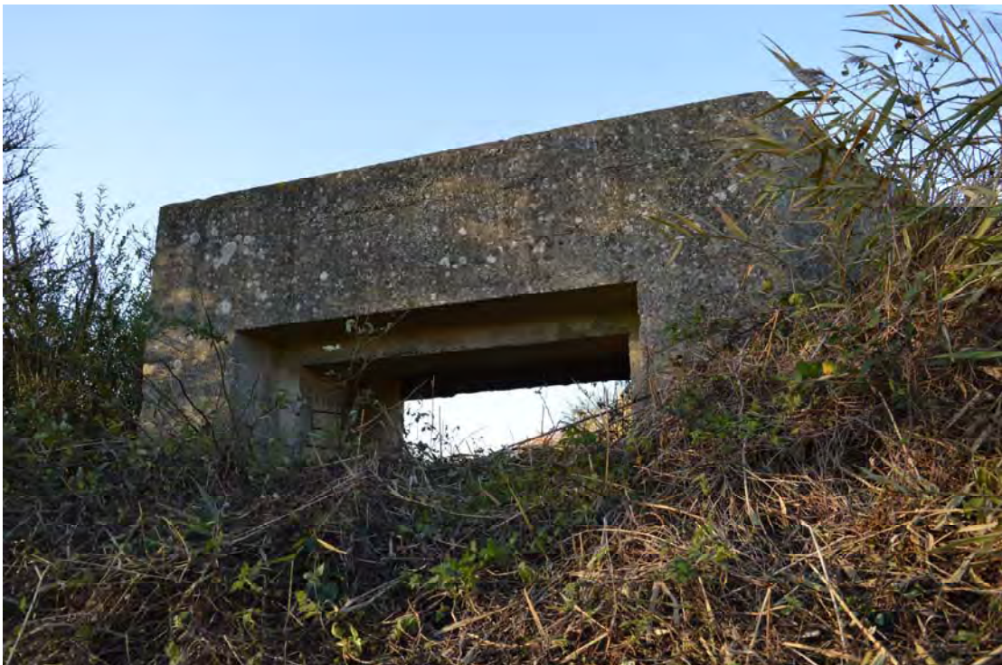
Plate 24: Structure 6, looking south-west (0133)
