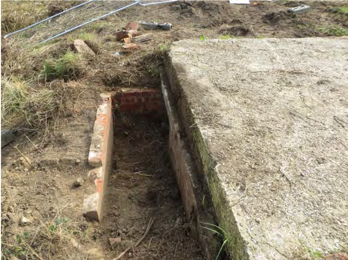
Plate 15: Structure 4, entrance and blast wall, looking south-east (0073)
