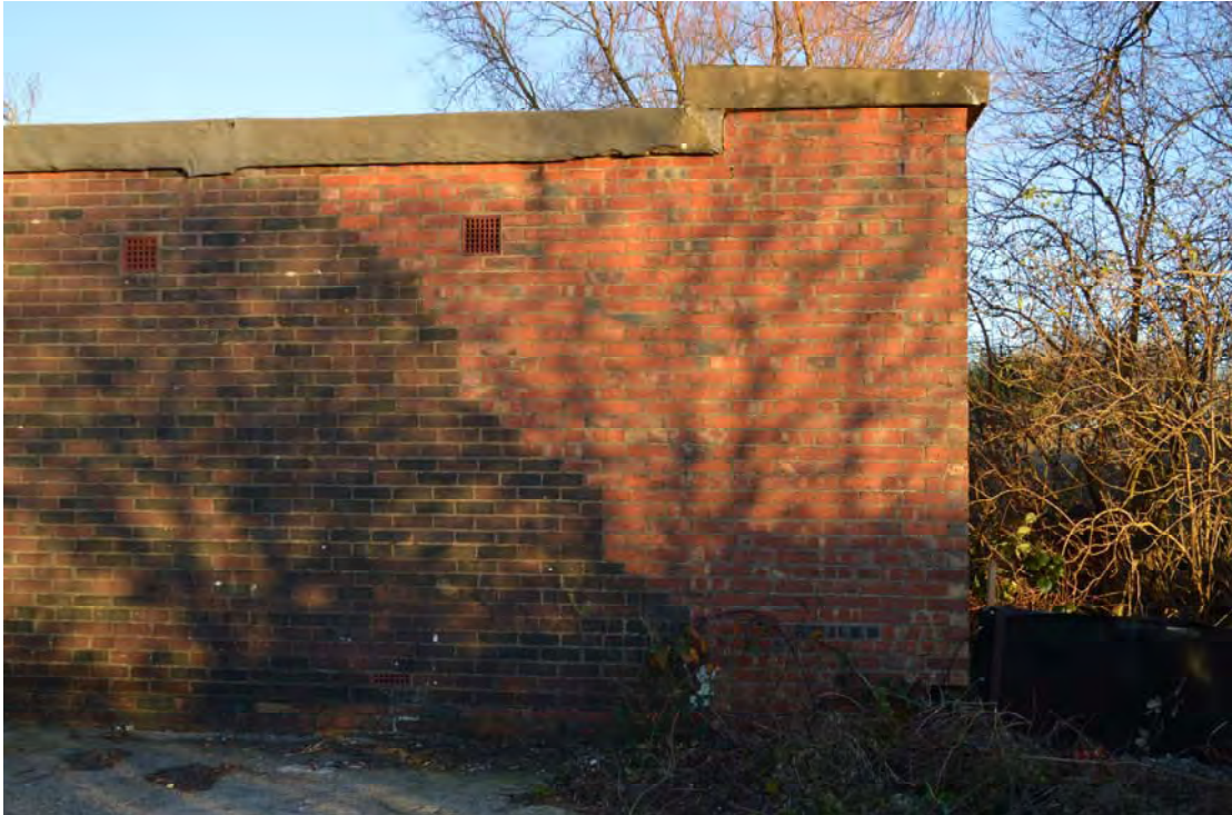
Plate 33: Structure 7, detail of repaired southern end, looking west (0157)
