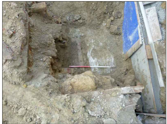
Walls 023 and 027 facing east
