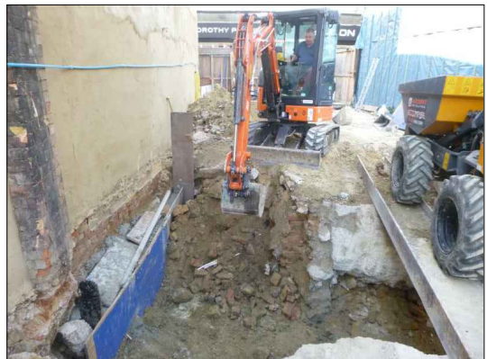
Working shot area 2
