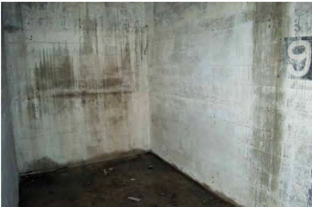
Plate 126: Store 9 – View of the bay arrangement (Bin 9), facing west (394)
