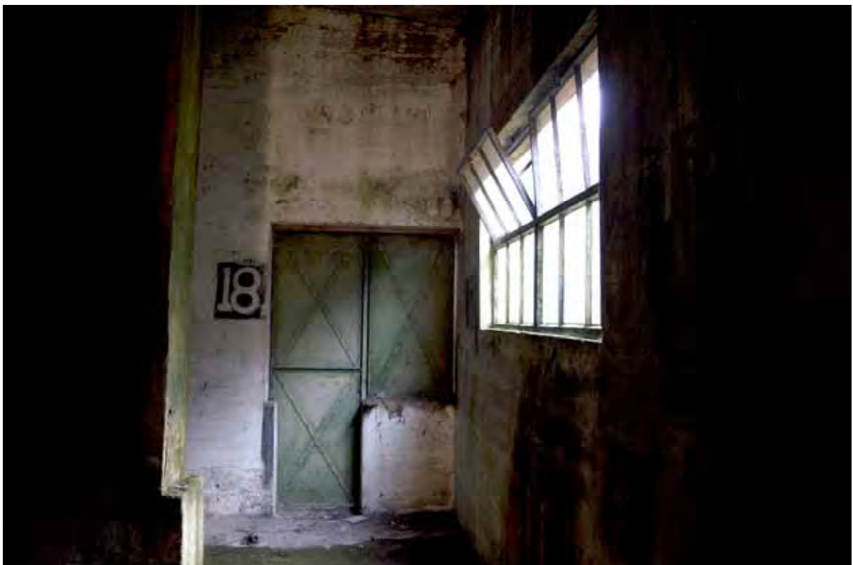
Plate 22: Store 4 – Detail of the internal door and window arrangement within each store (western door to southern loading bay), facing south-east (258)
