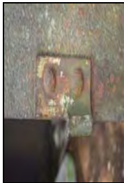
CFB17-0592 South-eastern sentry post
