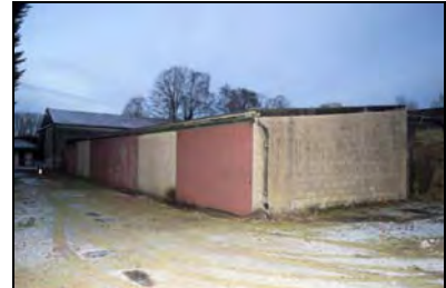
CFB17-0531 Buildings 10b and 10c (2017)
