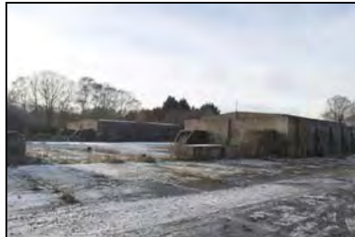
CFB17-0326 Stores 8 and 12 (2017)
