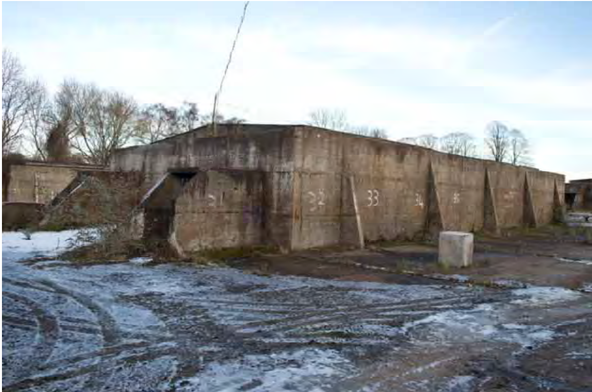
Plate 91: Store 8 – View of the north-west and south-west elevations, facing east (419)
