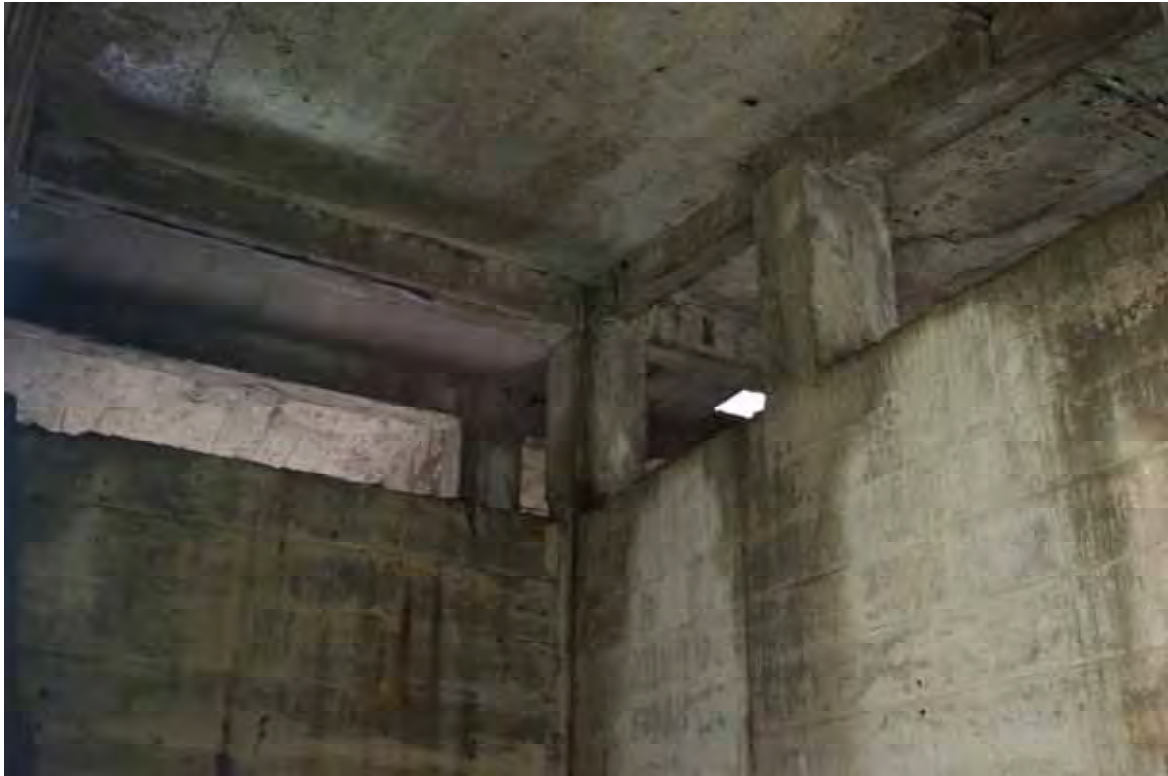
Plate 31: Store 4 – View of a typical bay arrangement (western half), facing north-east (264)
