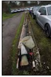
CFB17-0122 Feature along southern end of site (2015)
