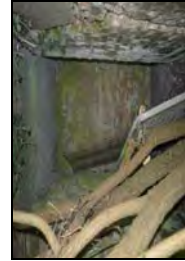
CFB17-0606 Air-raid shelter
