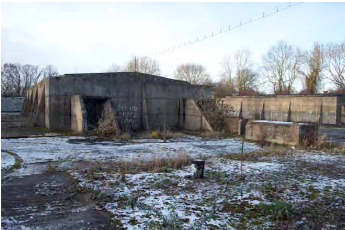
Plate 92: Store 8 – View of the southern loading bay, facing north (411)
