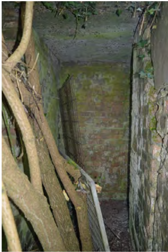
Plate 192: View of the air-raid shelter entrance interior, facing south-east (606)
