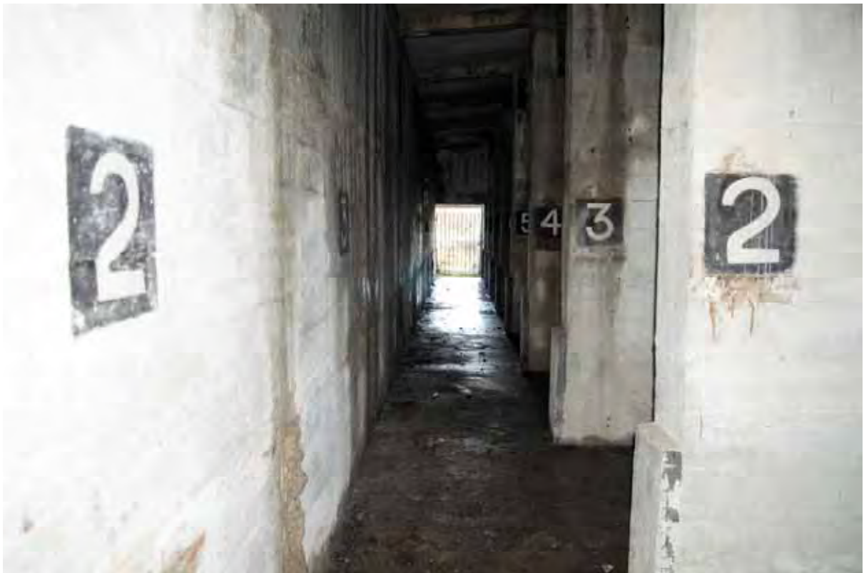
Plate 124: Store 9 – View of the eastern passage, facing south-east (397)
