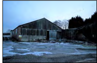
CFB17-0561 Store 10 / Building 10e (left) (2017)
