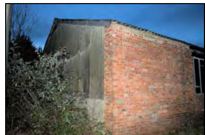
CFB17-0570 Building 10e (2017)
