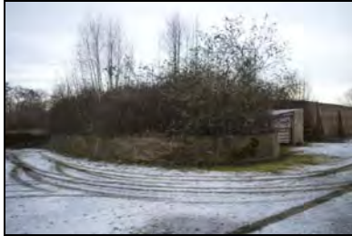
CFB17-0485 Bund separating Store 12 and 14 (2017)
