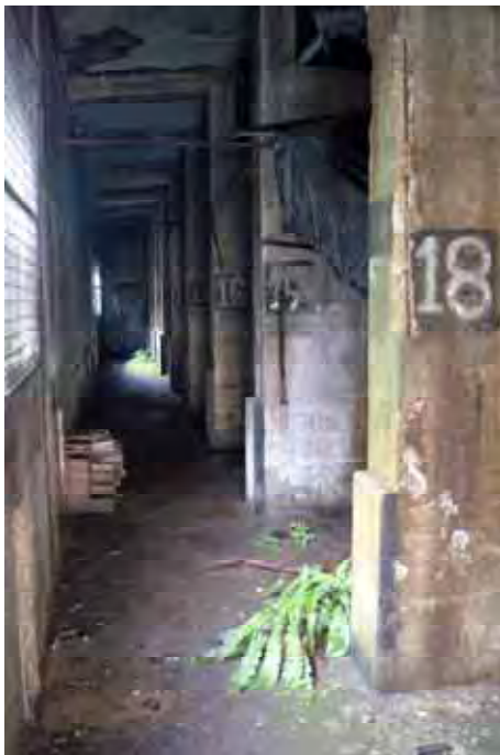
Plate 64: Store 5 – View of the western passage, facing north-west (301)
