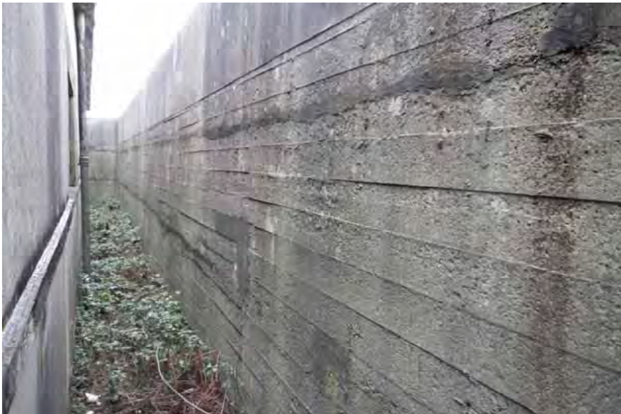
Plate 6: Store 4 – View of the open walkway separating the internal store structure from the outer blast walls, facing south-east (50)
