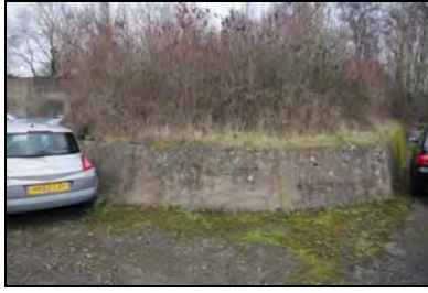
CFB17-0107 Bund separating Store 5 and 6 (2015)
