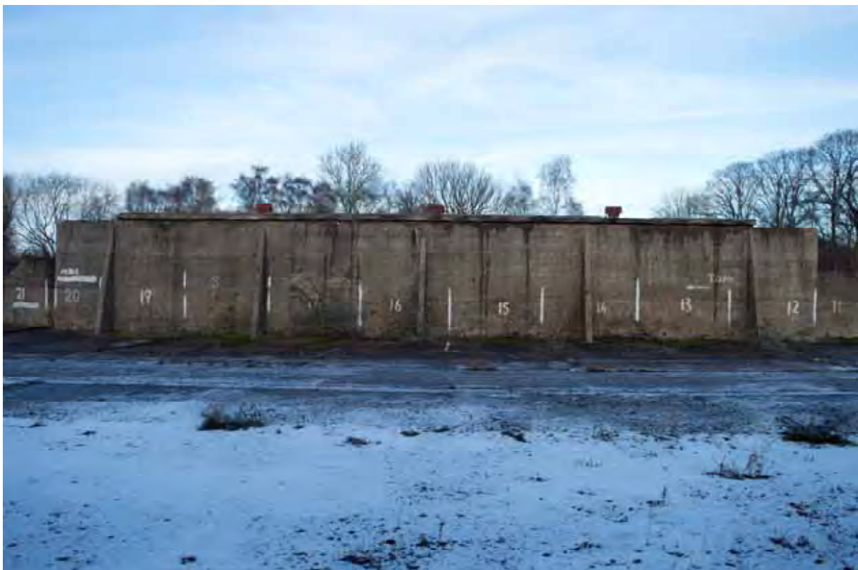
Plate 110: Store 9 – View of the south-west elevation, facing north-east (399)
