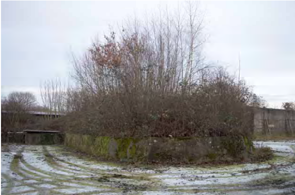
Plate 135: View of the bund separating Stores 10 and 12, facing east (514)
