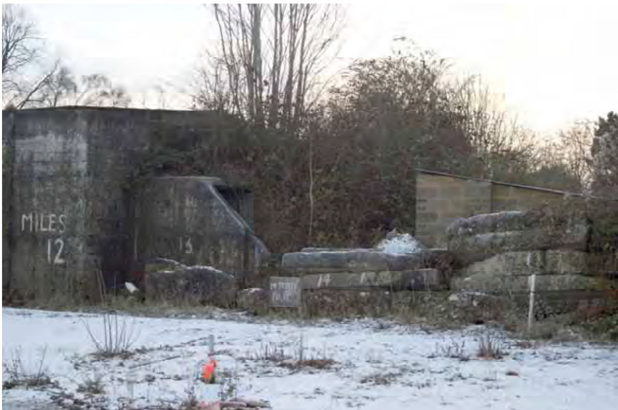
Plate 158: Store 14 – View of the eastern entrance serving the northern loading bay, note the retained bund walls from the removed bund separating Store 8 and 9, facing south-west (448)
