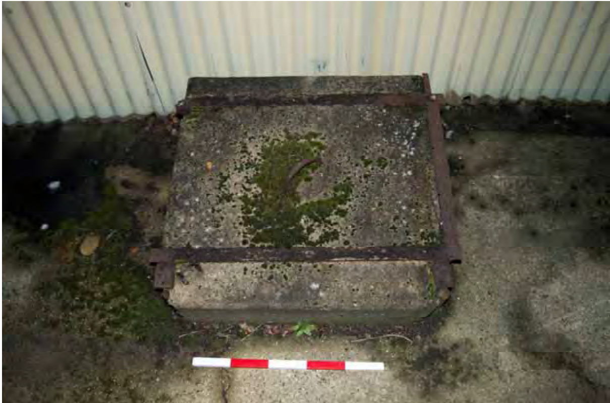
Plate 203: Detail of the displaced feature situated between Building 2 and 3, facing north-east (550)
