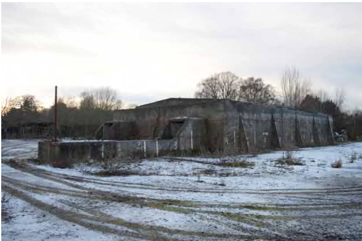
Plate 154: Store 14 – View of the north-east and south-east elevations, facing west (453)
