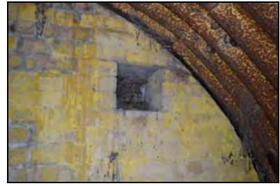
CFB17-0603 Air-raid shelter
