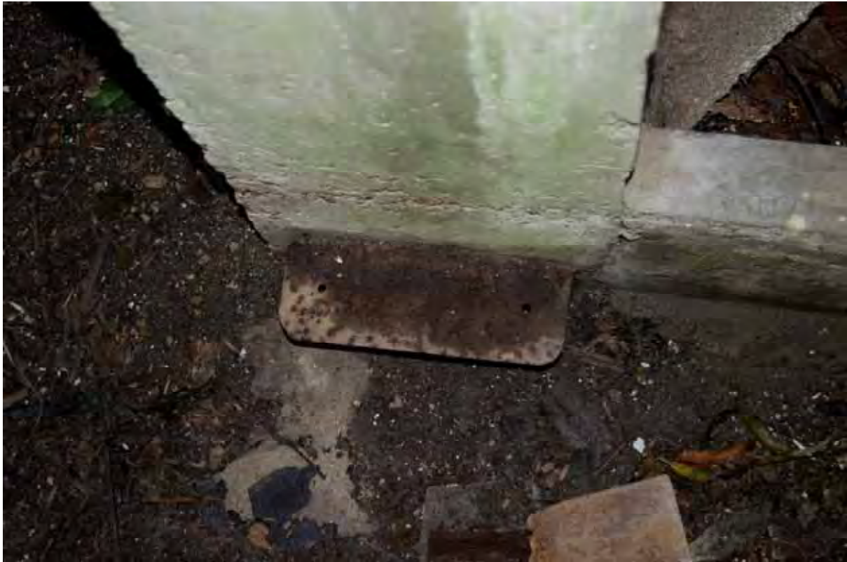
Plate 165: Store 14 – Detail of the brackets fitted to the end of each of the eastern bay containment end walls, facing south-west (467)
