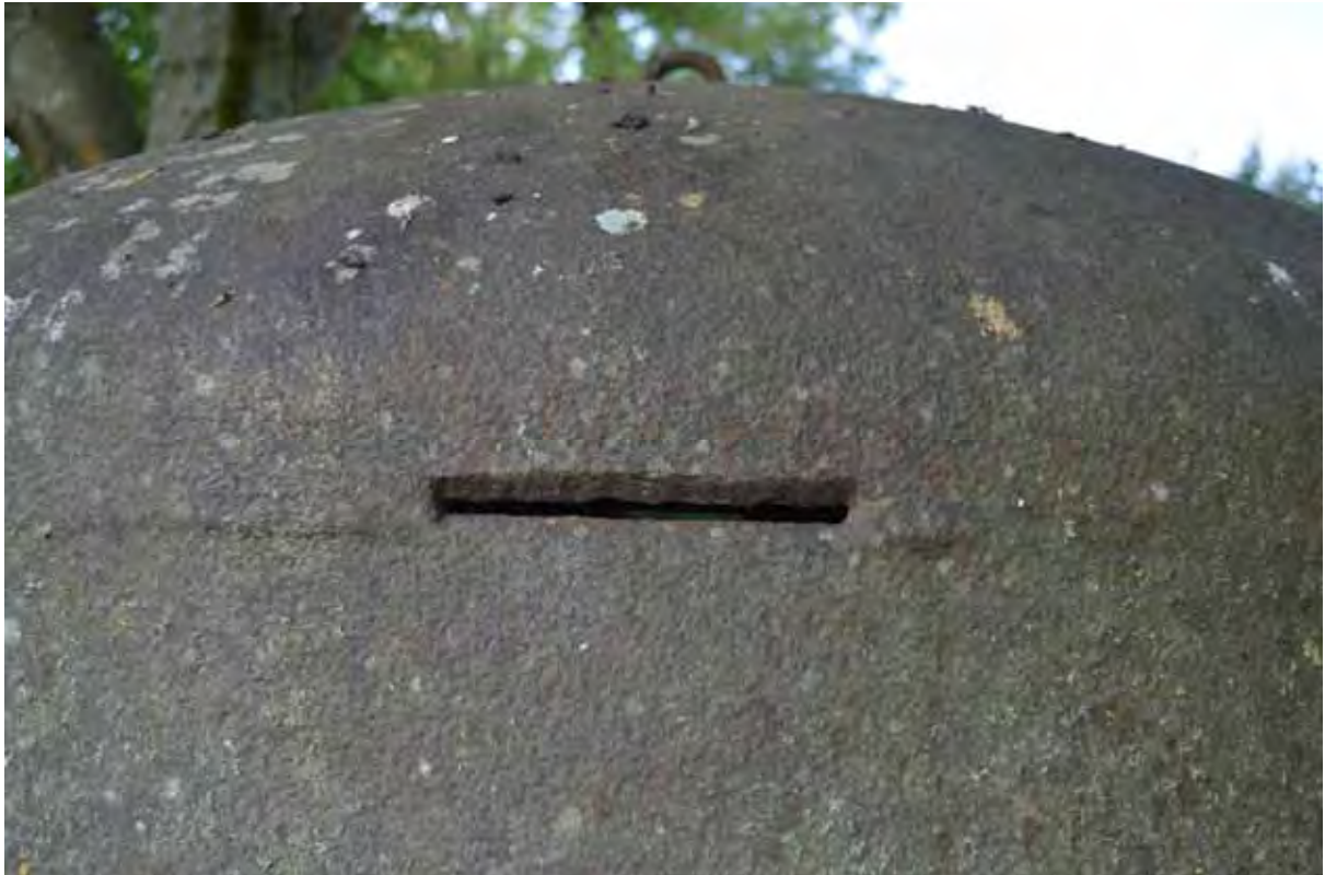
Plate 171: Detail of the air vent around the top of the south-eastern sentry post, facing north-east (593)
