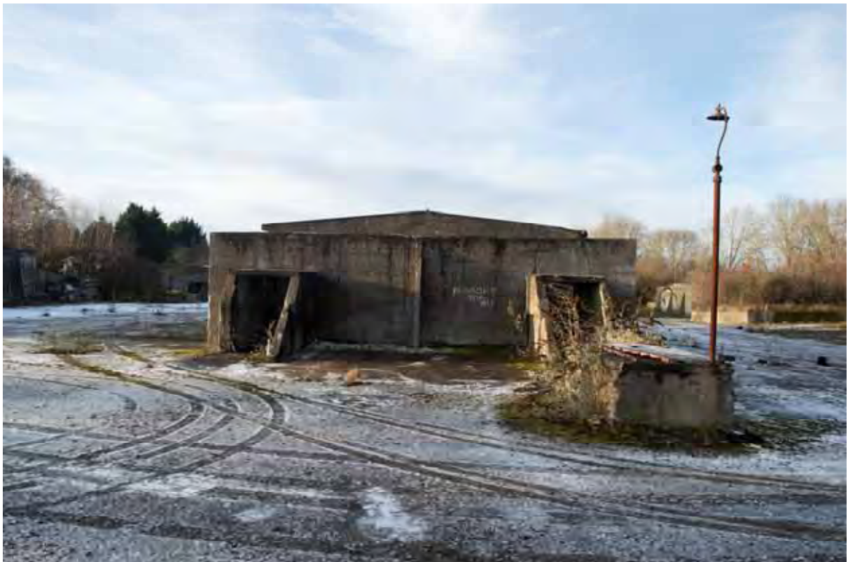
Plate 112: Store 9 – View of the southern loading bay, facing north-west (370)
