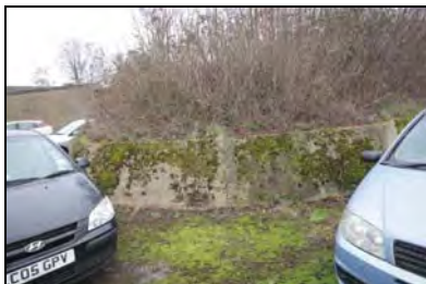
CFB17-0145 Bund separating Stores 12 and 10 (2015)
