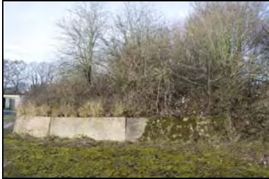
CFB17-0289 Bund separating Stores 4 and 5 (2017)
