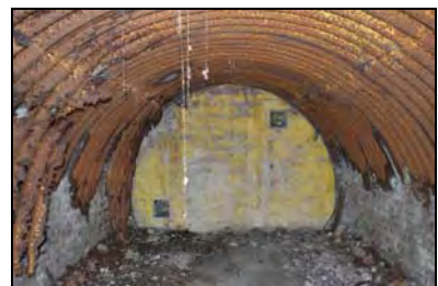
CFB17-0600 Air-raid shelter
