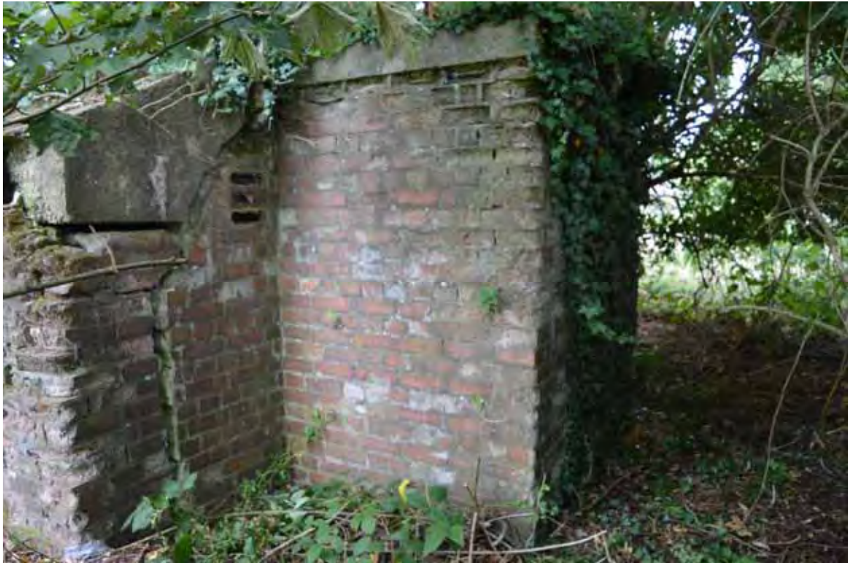
Plate 191: View of the north-east elevation of the air-raid shelter, facing west (610)
