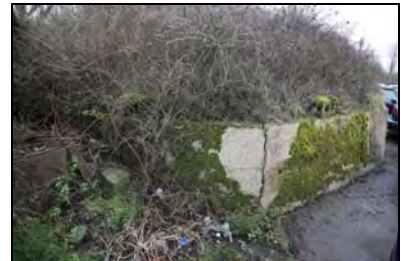
CFB17-0090 Bund separating Store 4 and 5 (2015)
