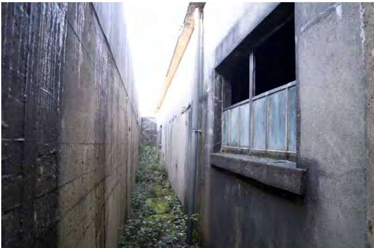
Plate 120: Store 9 – View of the western walkway, facing north-west (379)
