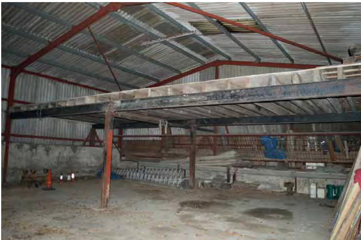
Plate 200: View of the interior of Building 2, facing north (546)
