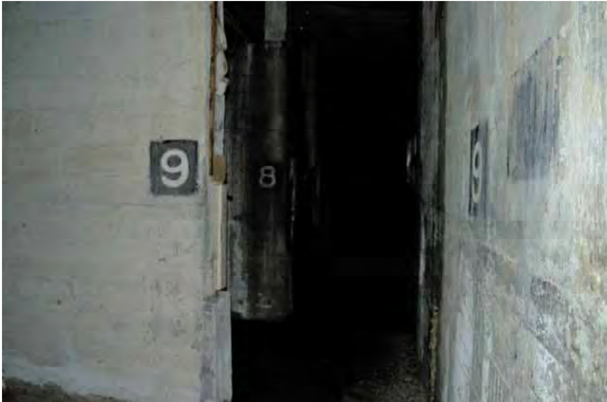
Plate 139: Store 10 – Detail of the clear bay signage and white-washed walls within the eastern passage, facing north-west (526)
