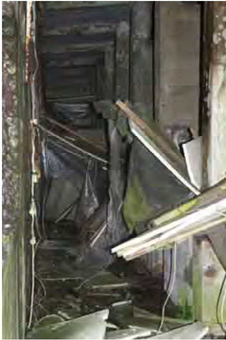
Plate 153: Store 12 – View of the western passage, facing north-west (498)
