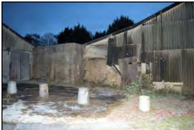
CFB17-0562 Store 10 (centre) / Buildings 10d (right) and 10e (left) (2017)
