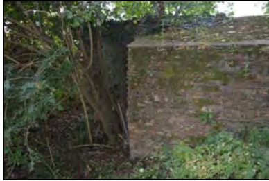
CFB17-0605 Air-raid shelter
