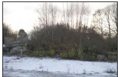
CFB17-0450 Bund separating Stores 14 and 12 (2017)
