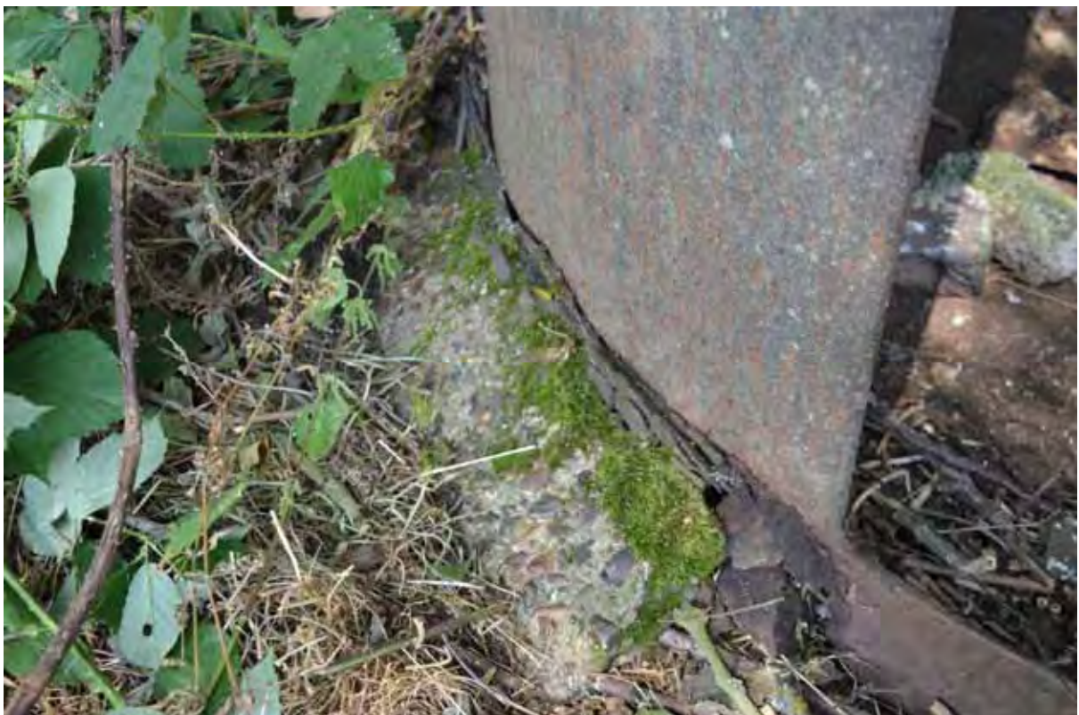
Plate 174: Detail of the ramped mortar base edge beneath the south-eastern sentry post, facing north-west (597)
