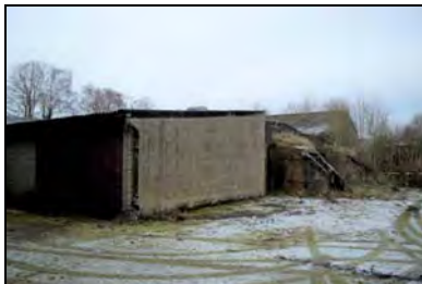
CFB17-0533 Store 10 / Buildings 10b (2017)
