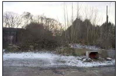
CFB17-0444 Bund separating Store 12 and 10 (2017)
