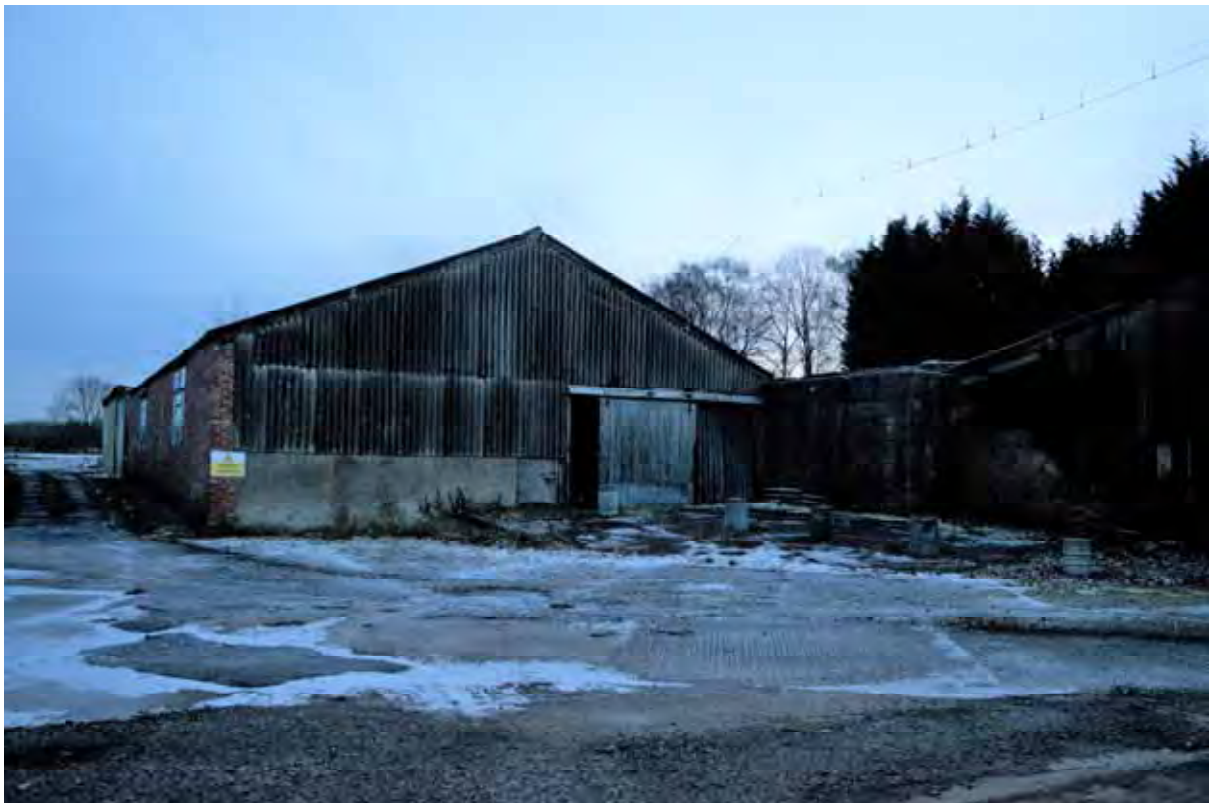
Plate 214: View of the north-west elevation of Building 10e, facing south (561)
