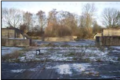
CFB17-0412 Area of former bund separating Stores 8 and 9 (removed) (2017)
