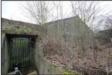
CFB17-0154 Store 10 / Building 10e (2015)
