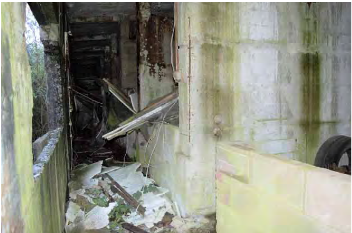
Plate 152: Store 12 – View of the western passage, facing north-west (497)
