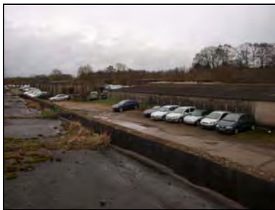
CFB17-0185 Store 4 - looking south-west across the site (2015)
