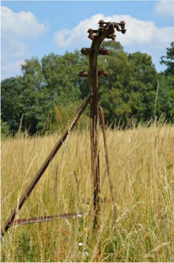
Plate 3: Detail of an original perimeter fence bracket along the site's north-eastern boundary, facing north-east (622)
