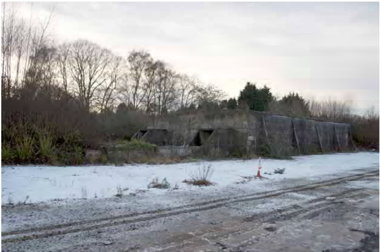
Plate 142: Store 12 – View of the north-east and south-east elevations, facing west (445)
