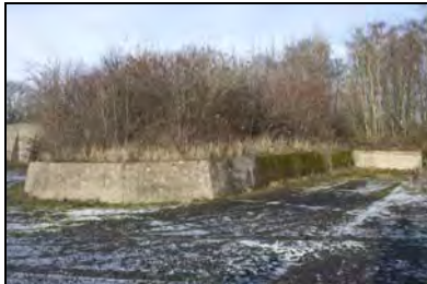
CFB17-0325 Bund separating Store 5 andf 6 (2017)
