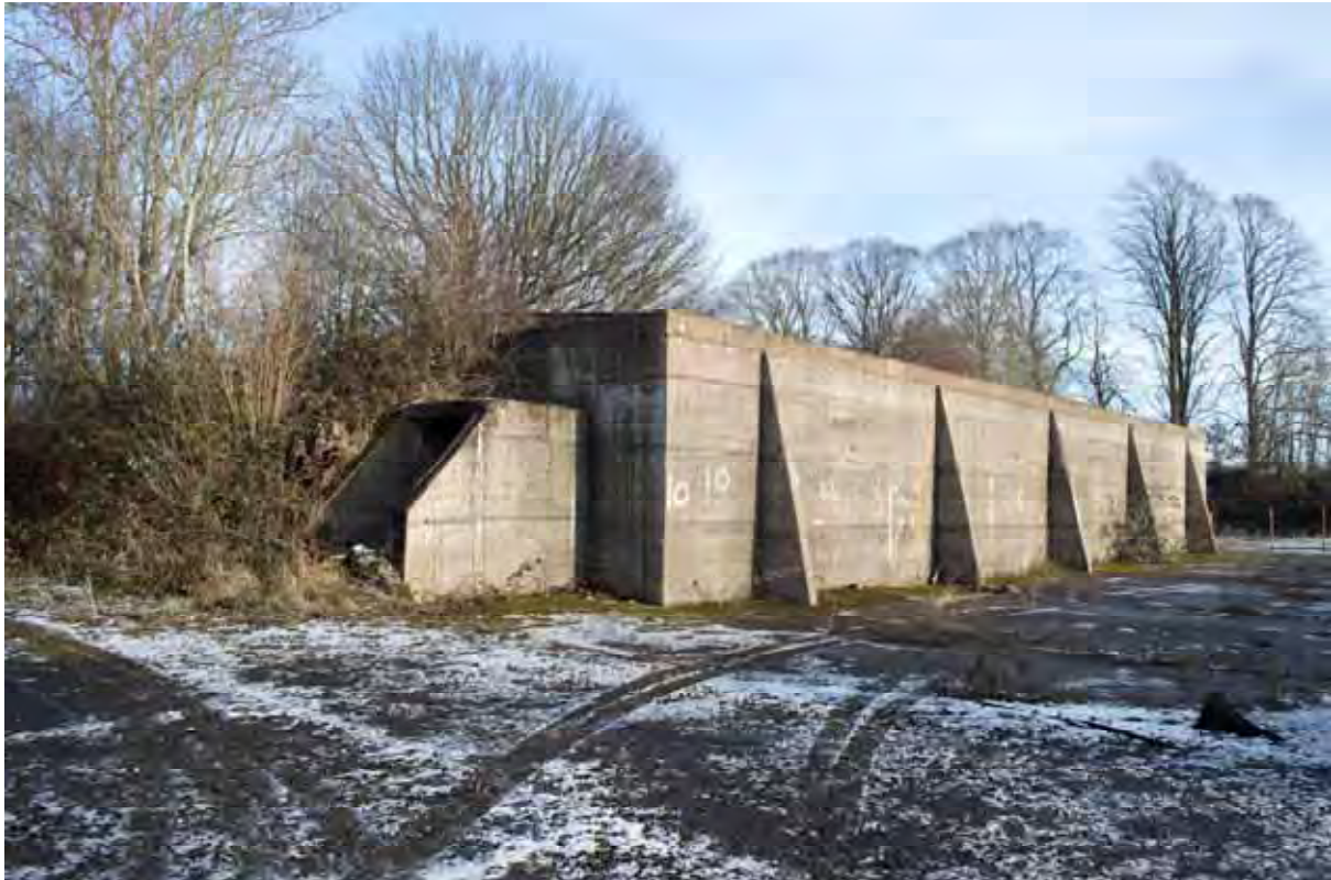
Plate 73: Store 6 – General view of the north-west and south-west elevations, facing east (328)
