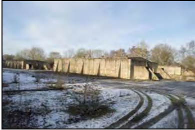
CFB17-0364 Stores 9 (foreground) and 8 (2017)
