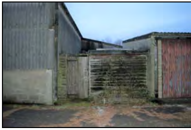
CFB17-0541 Building 10b (2017)
