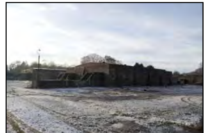
CFB17-0360 Stores 9 and 14 (2017)
