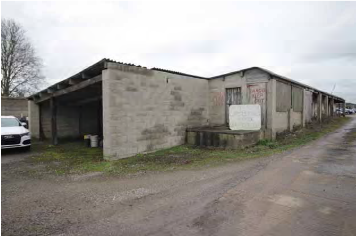
Plate 207: View of the north-west and south-west elevations of Building 7, facing east (158)
