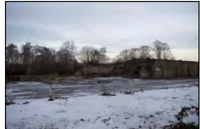
CFB17-0489 Stores 9 (foreground) and 6 (2017)
