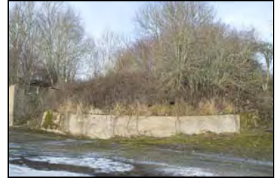
CFB17-0288 Bund separating Stores 4 and 5 (2017)
