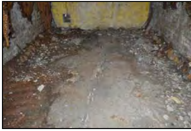
CFB17-0602 Air-raid shelter
