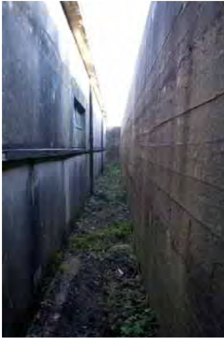
Plate 49: Store 4 – Detail of the continuous cill running the length of the store's south-west elevation, facing south-east (241)
