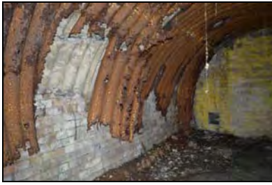
CFB17-0601 Air-raid shelter
