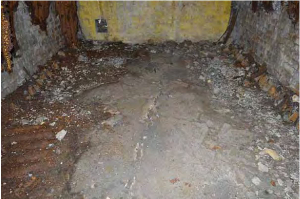
Plate 197: Detail of the air-raid shelter floor, facing south-west (602)
