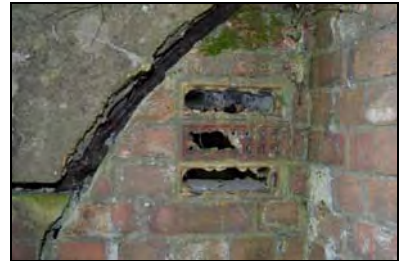
CFB17-0609 Air-raid shelter
