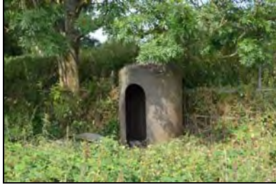
CFB17-0590 South-eastern sentry post
