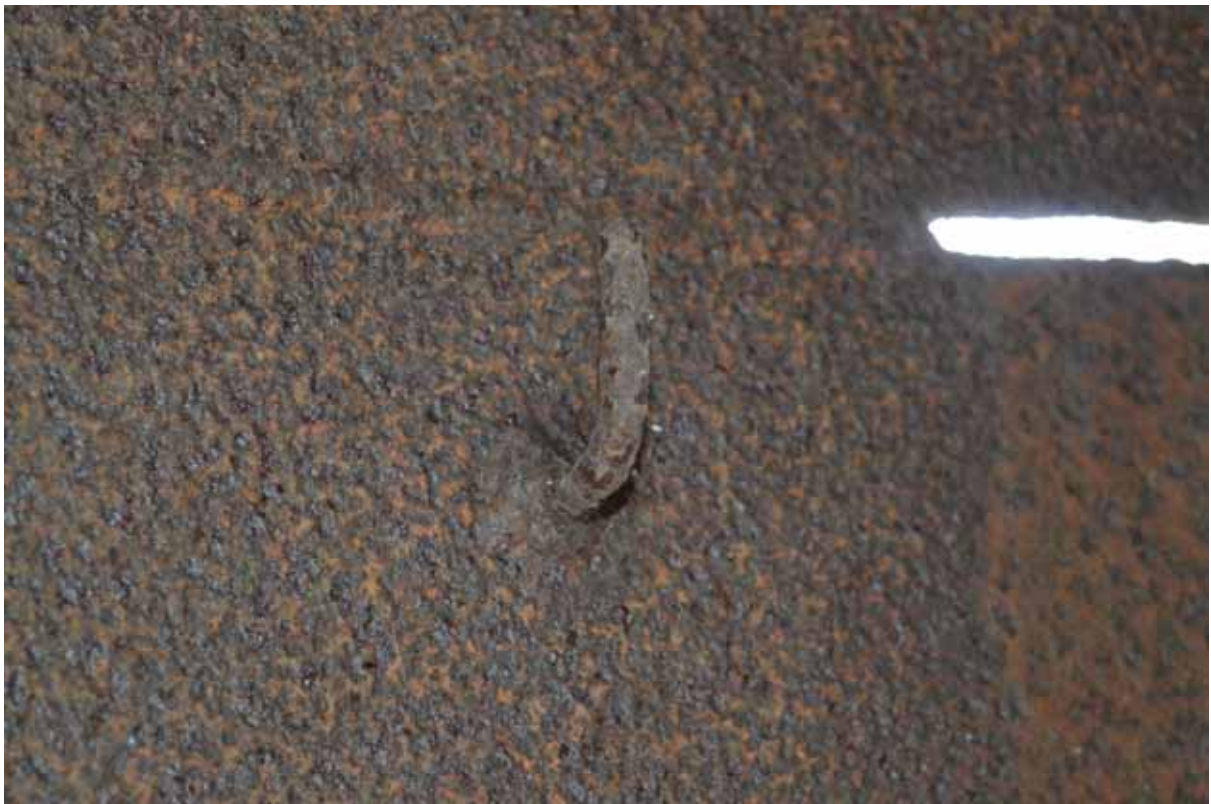
Plate 180: Detail of a hook within the south-eastern sentry post, facing south-west (598)
