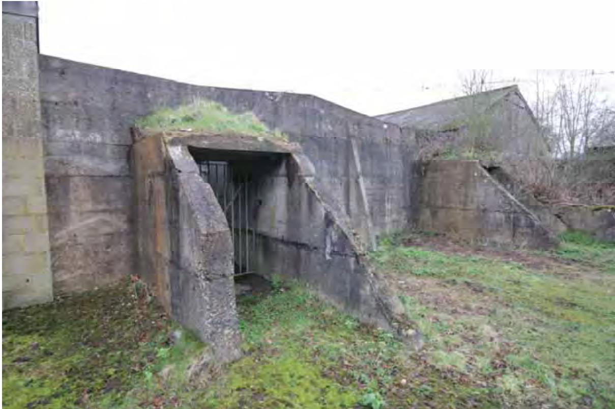
Plate 133: Store 10 – View of the south-east elevation, facing north (8)
