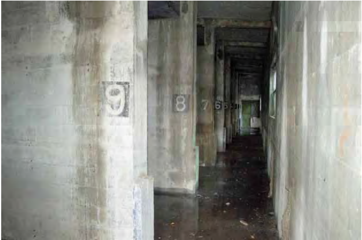
Plate 123: Store 9 – View of the eastern passage, facing north-west (393)
