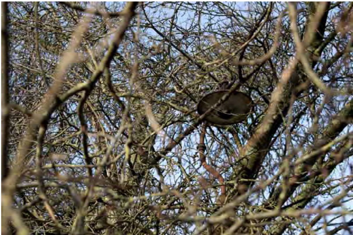
Plate 58: Store 5 – Light fixture retained on the eastern loading platform serving the northern bay, facing north-east (291)
