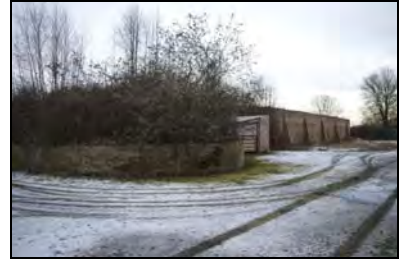
CFB17-0486 Bund separating Store 12 and 14 (2017)
