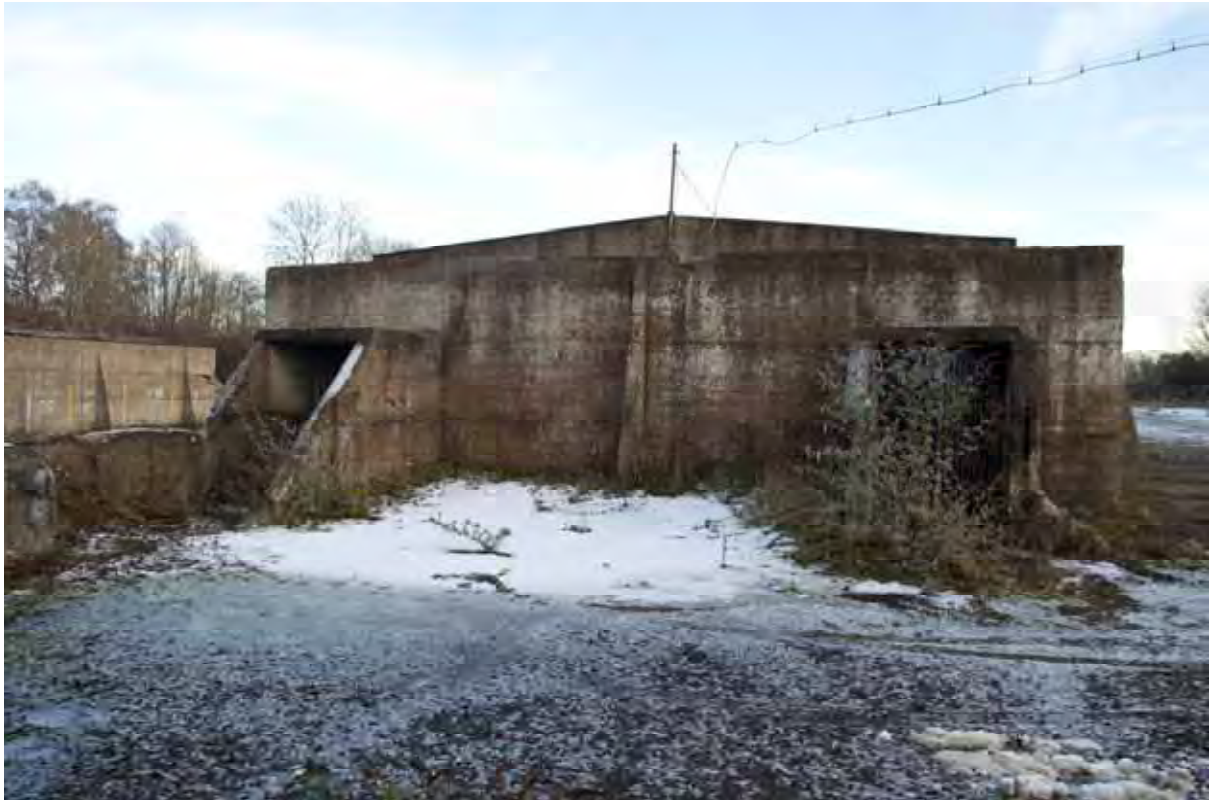
Plate 93: Store 8 – View of the northern loading bay, facing south-east (420)
