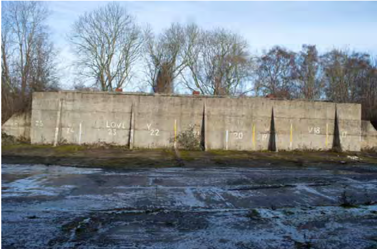
Plate 57: Store 5 – View of the south-west elevation, facing north-east (293)
