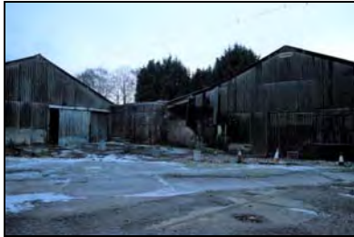
CFB17-0560 Store 10 (centre) / Buildings 10d (right) and 10e (left) (2017)
