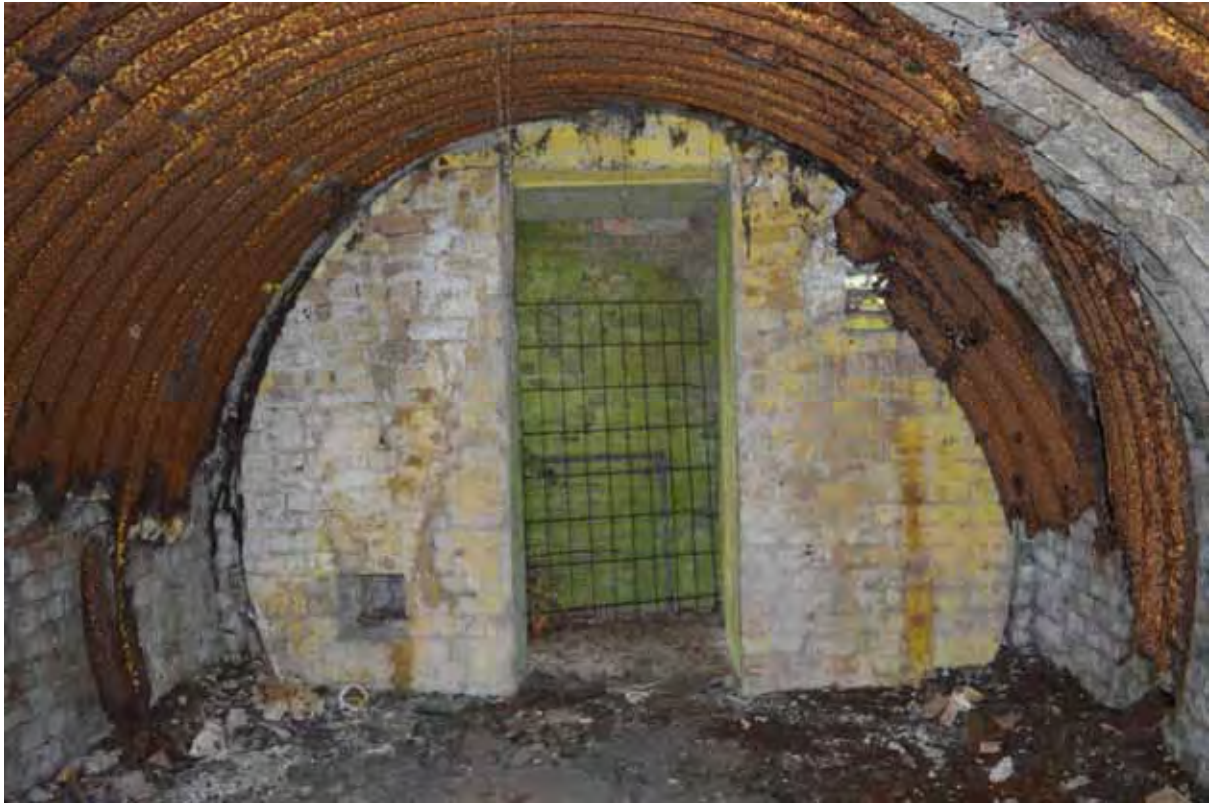
Plate 193: Interior of the air-raid shelter, facing north-east towards the entrance (604)
