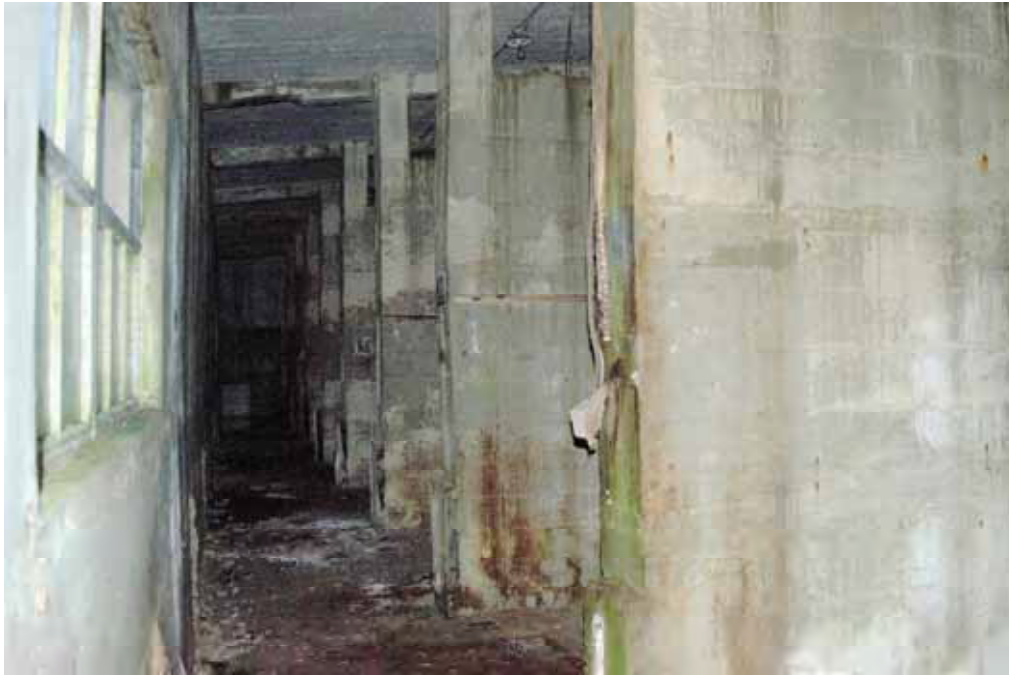
Plate 137: Store 10 – View of the western passage, facing north-west (522)
