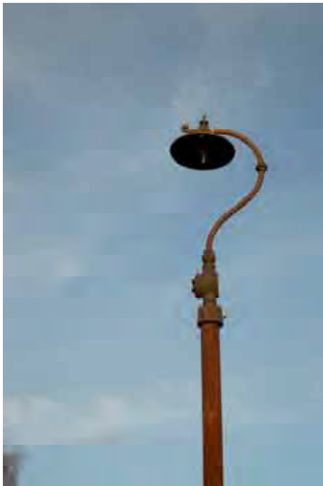
Plate 114: Store 9 – Detail of the retained lamp post on the eastern platform of the southern loading bay, facing east (373)
