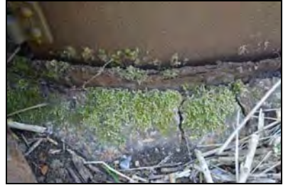
CFB17-0621 North-eastern sentry post
