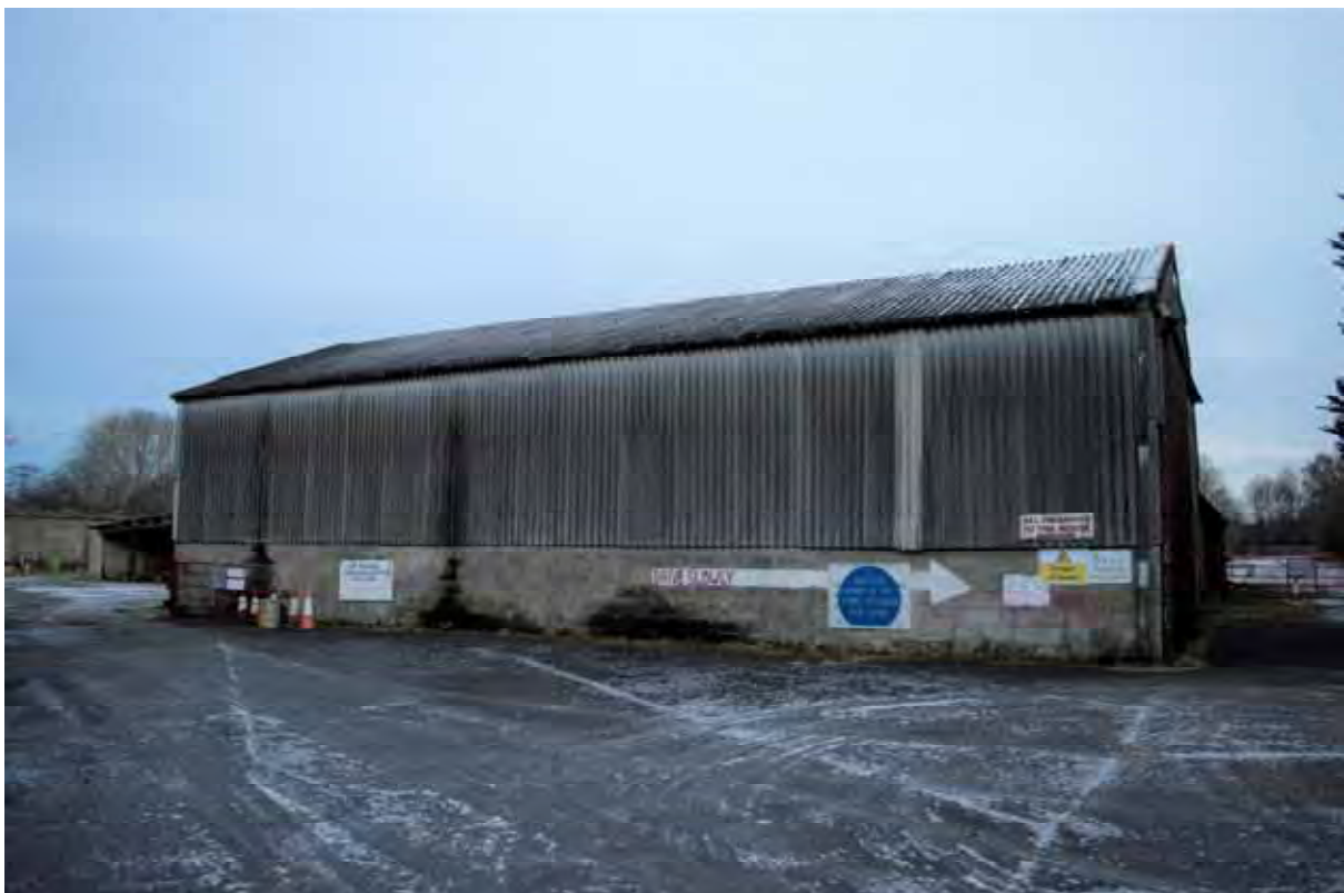
Plate 212: View of the north-west elevation of Building 10c / 10d, facing south-east (544)
