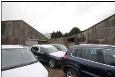
CFB17-0157 Store 10 / Building 10d and 10e (2015)
