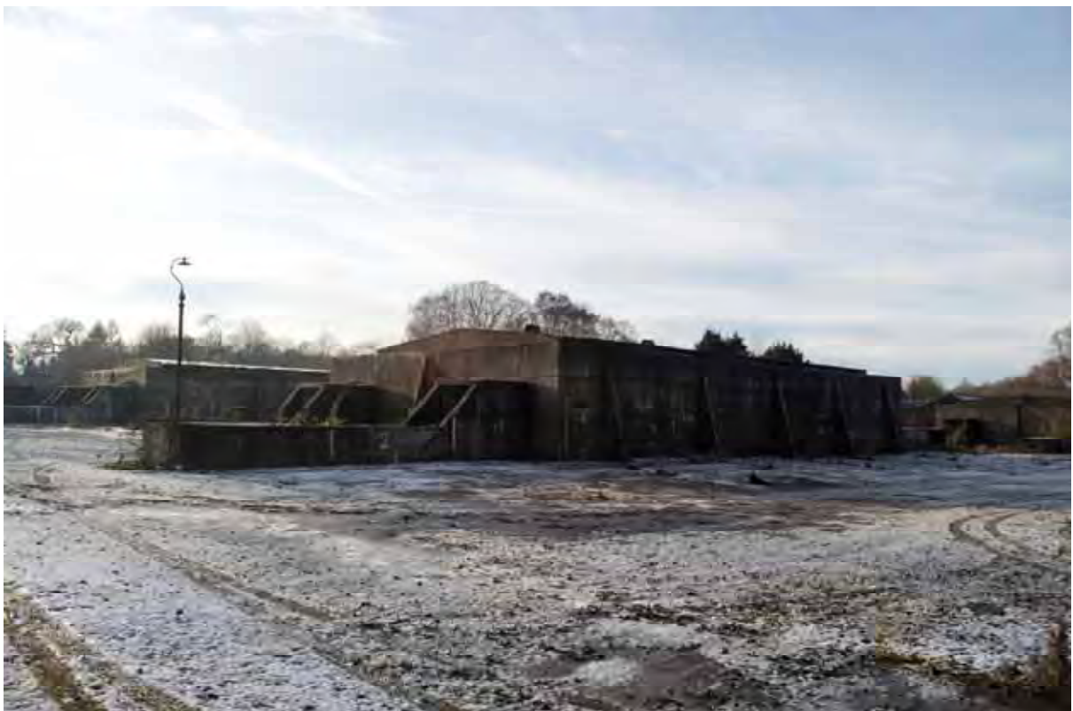
Plate 108: Store 9 – View of the south-east and north-east elevations, facing west (360)
