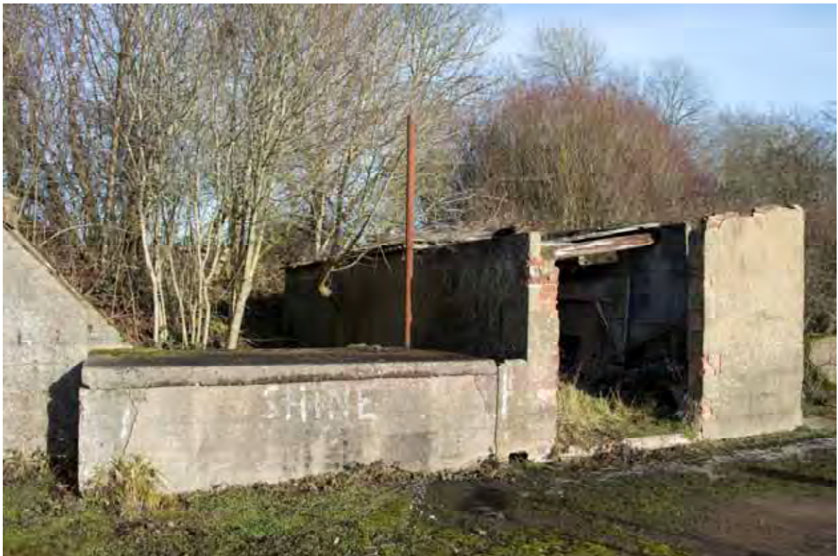
Plate 220: View of the north-west and south-west elevations of Building 15, facing east (282)
