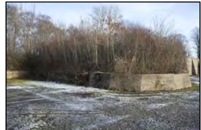
CFB17-0324 Bund separating Store 5 andf 6 (2017)
