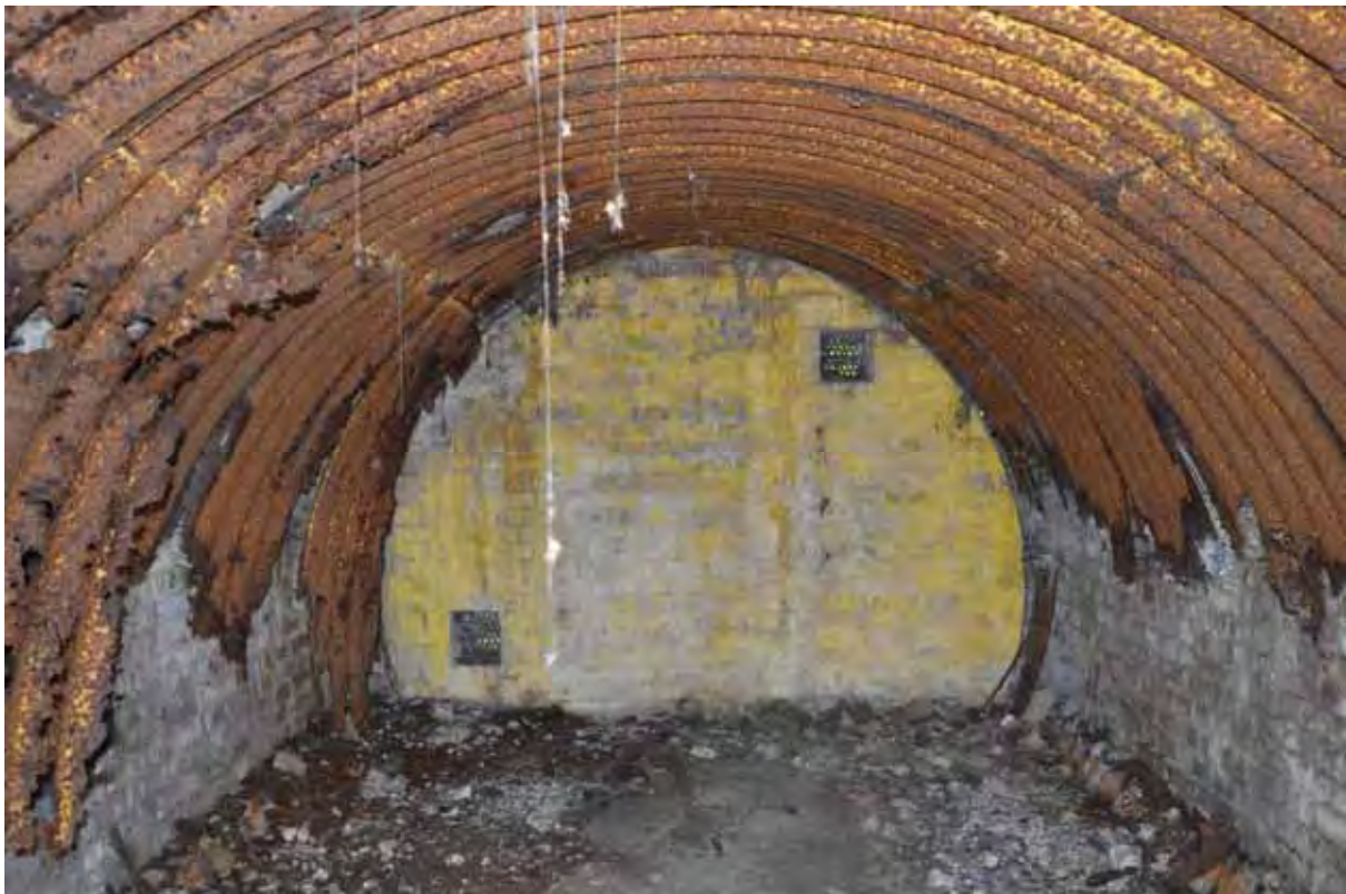
Plate 194: Interior of the air-raid shelter, facing south-west (600)
