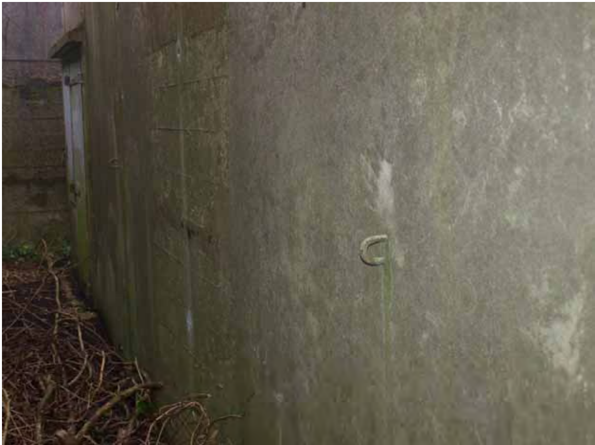
Plate 28: Store 4 – Padlock hook located adjacent to each doorway (south-east elevation), facing west (220)
