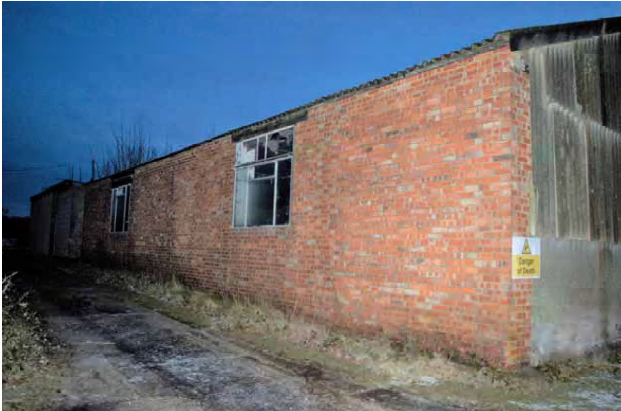
Plate 215: View of the north-east brick-built elevation of Building 10e, facing south (569)
