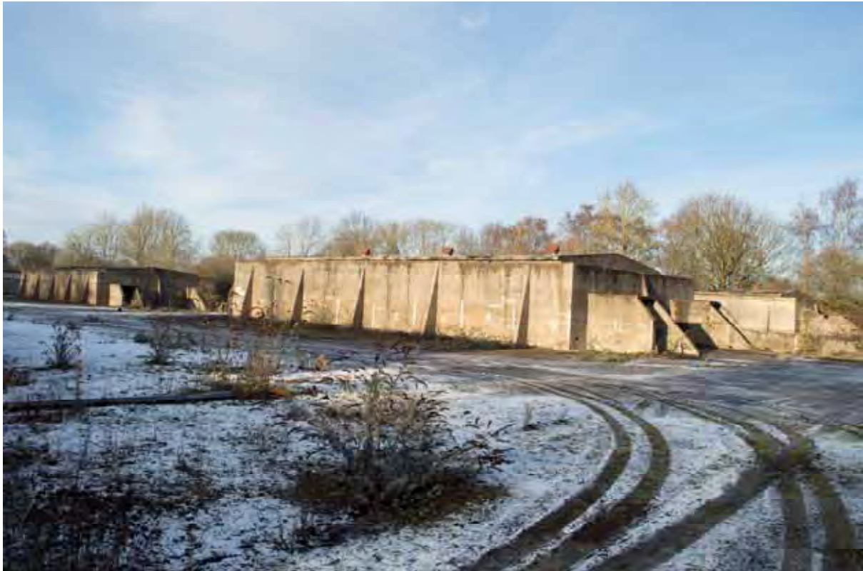
Plate 109: Store 9 – View of the south-east and south-west elevations, facing north (364)
