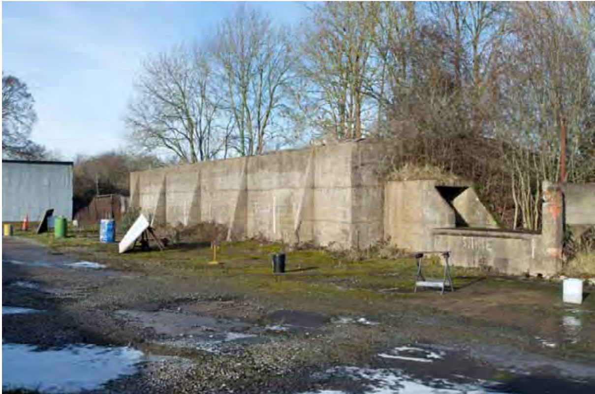
Plate 5: Store 4 – View of the south-west and south-east elevations, facing north-east (229)
