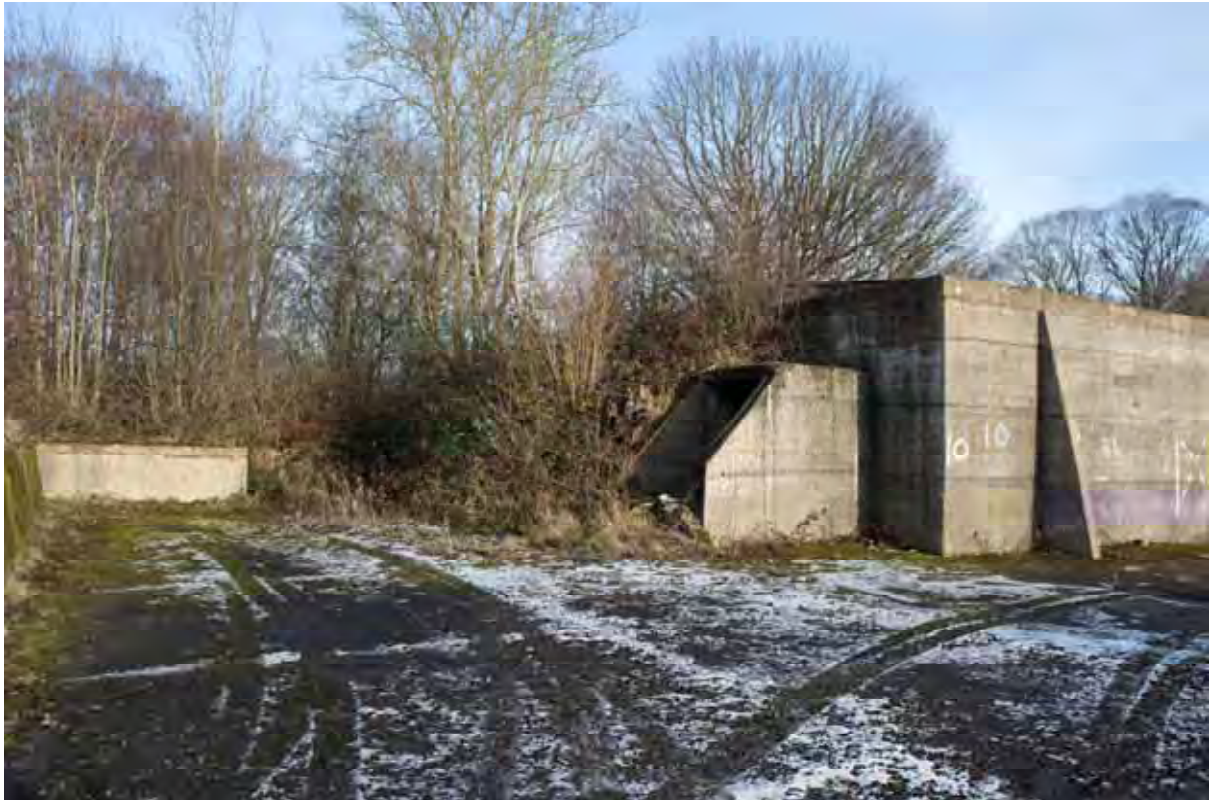
Plate 75: Store 6 – View of the northern loading bay, facing north-east (327)
