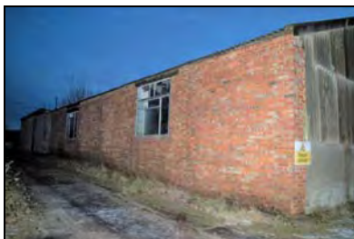
CFB17-0569 Building 10e (2017)
