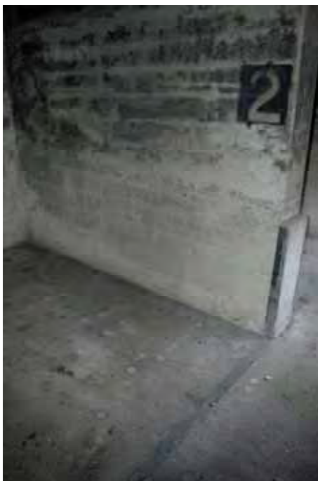
Plate 104: Store 8 – Detail of the bay divisions, note the absence of floor sockets, facing west (442)
