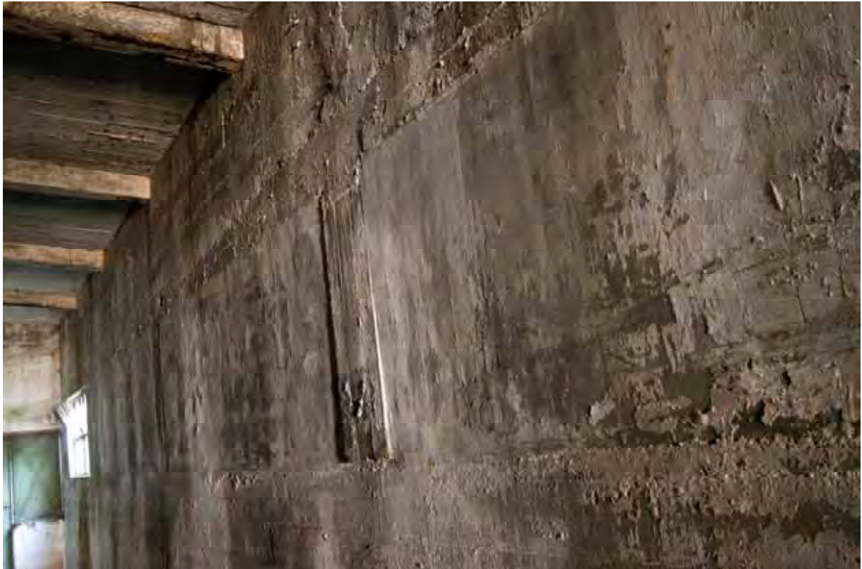
Plate 21: Store 4 – Detail of the blocked opening within the store's south-west elevations, facing south-east (254)
