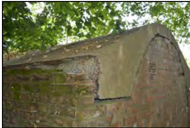
CFB17-0611 Air-raid shelter
