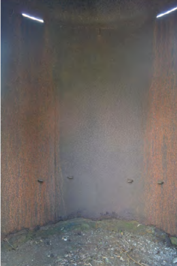
Plate 178: Internal view of the north-eastern sentry post, facing south-west (619)
