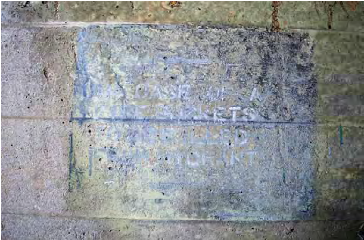
Plate 119: Store 9 – Detail of the fire hydrant signage found on the south-west wall of the western entrance serving the southern loading bay, facing south-west (376)
