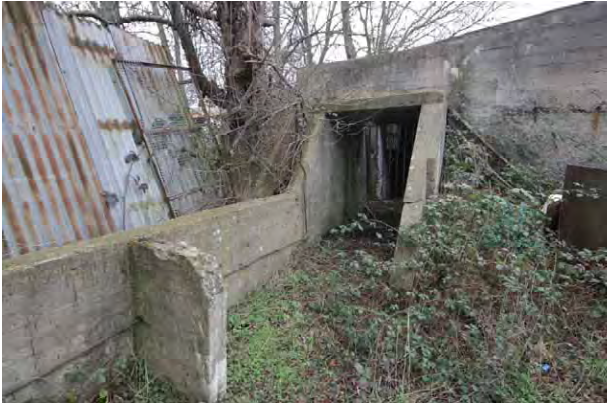
Plate 15: Store 4 – View of the northern loading bay entrance and conveyor base, serving the eastern half of the store, facing south-east (55)
