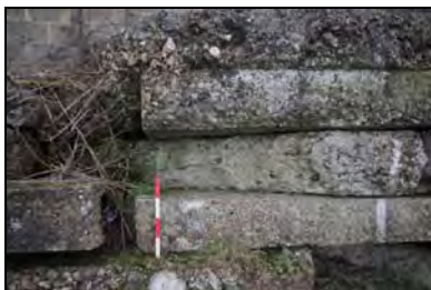
CFB17-0179 Store 14 - bund containment walls (2015)
