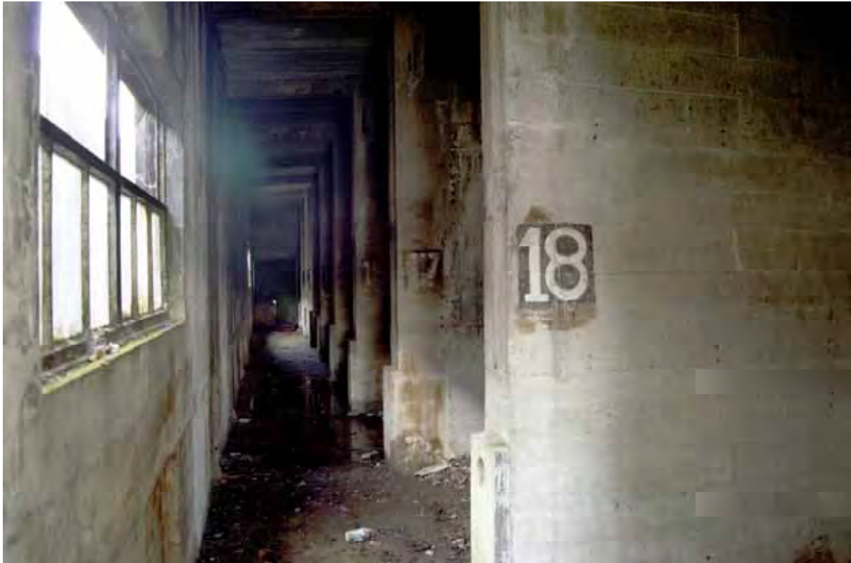
Plate 121: Store 9 – View of the western passage, facing north-west (381)
