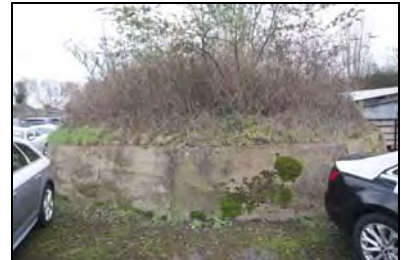
CFB17-0132 Bunt separating Stores 14 and 12 (2015)
