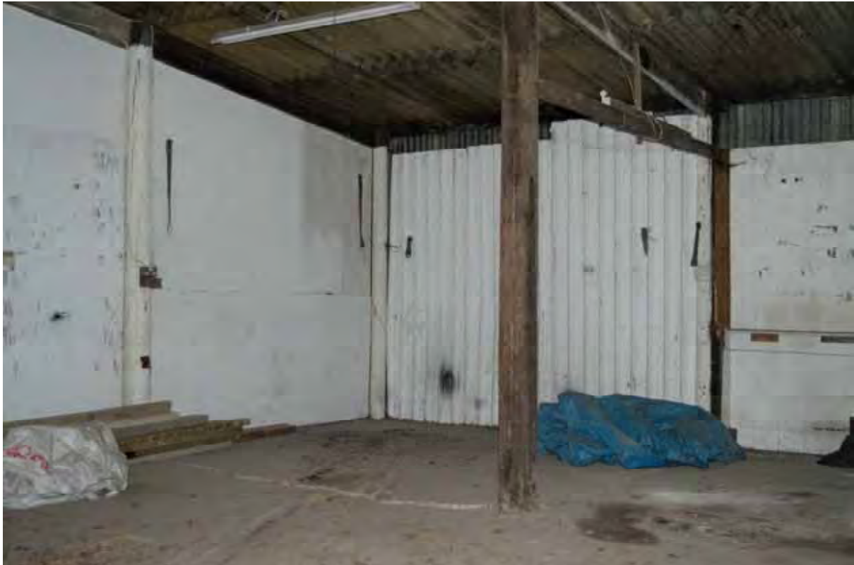
Plate 205: View of Bay 4 within Building 3, facing north-west (556)
