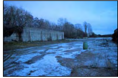
CFB17-0588 Road passing to the west of Stores 5 (foreground) and 6 (2017)
