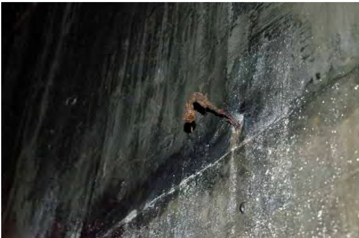
Plate 72: Store 5 – Detail of the brackets formerly securing the timber notice board within the northern end of the western passage, facing south-west (313)
