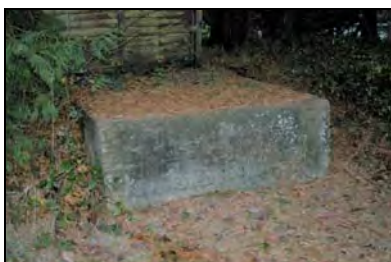
CFB17-0538 Building 10b (2017)
