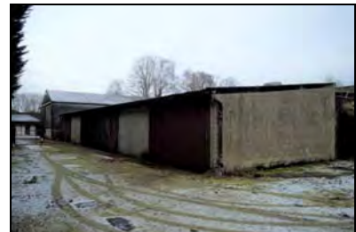
CFB17-0534 Buildings 10b and 10c (2017)
