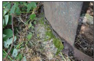
CFB17-0597 South-eastern sentry post
