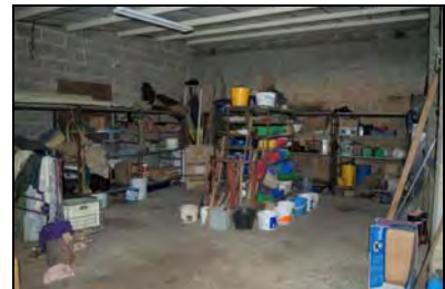
CFB17-0537 Building 10b (2017)
