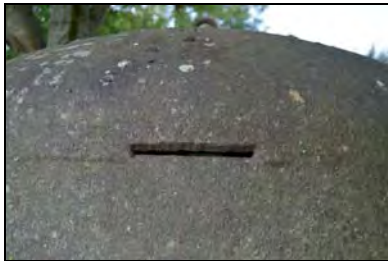
CFB17-0593 South-eastern sentry post
