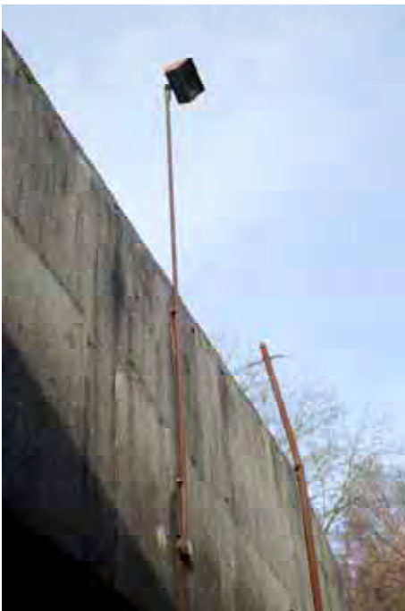
Plate 24: Store 4 – View of the light fittings serving each loading bay (south-east elevation), facing north-east (299)
