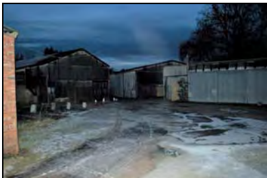
CFB17-0583 Store 10 (centre) / Buildings 10d (right) and 10e (left) (2017)
