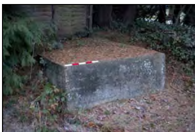
CFB17-0539 Building 10b (2017)
