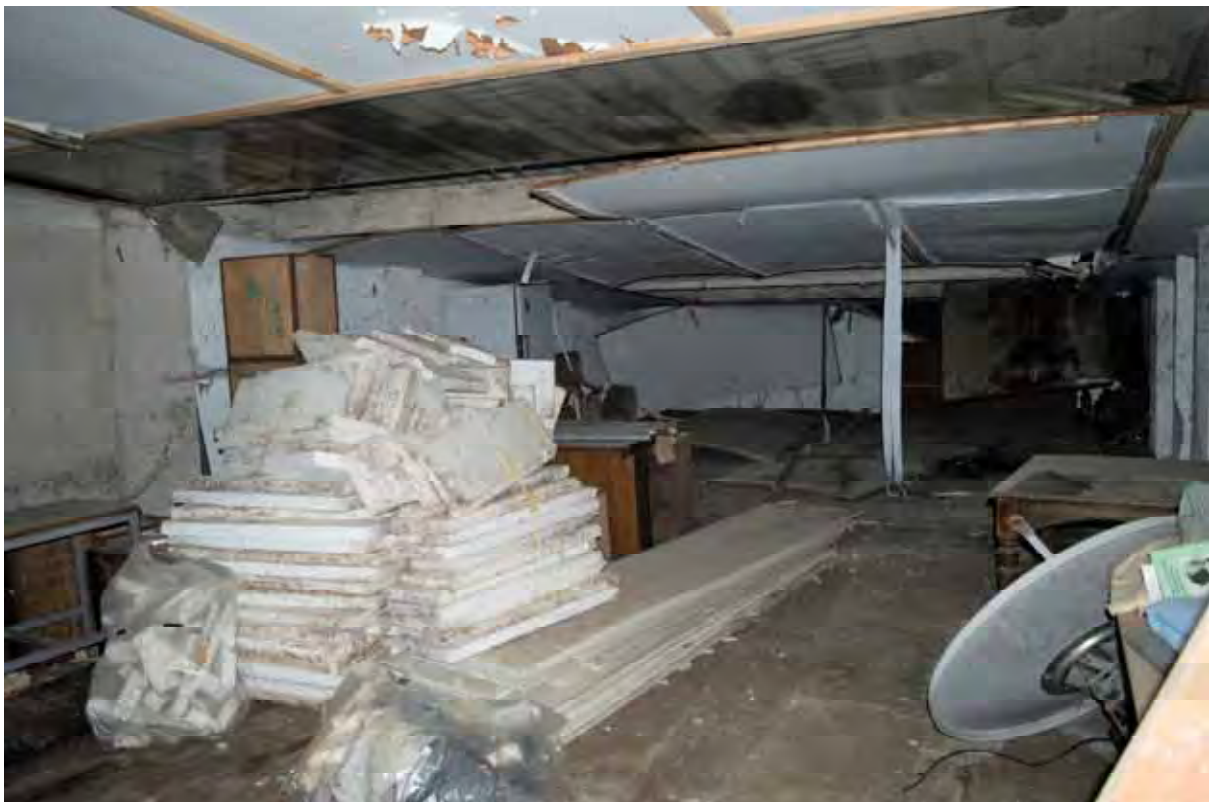
Plate 208: View of an internal bay within Building 7 (northern end), facing north-east (582)
