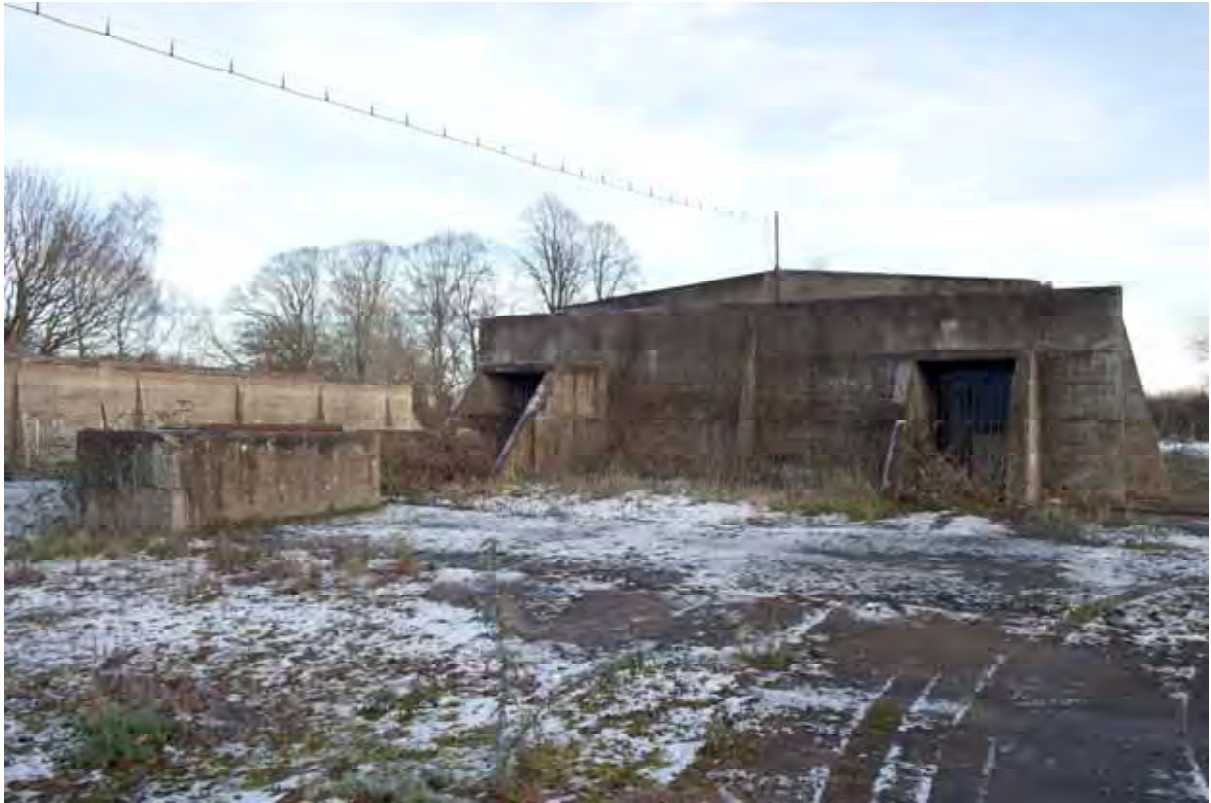
Plate 111: Store 9 – View of the northern loading bay, facing south-east (400)
