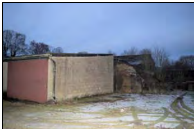
CFB17-0532 Store 10 / Buildings 10b (2017)
