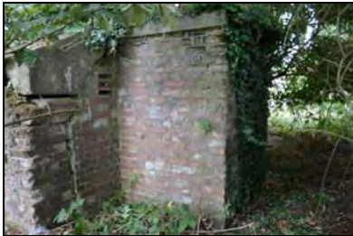
CFB17-0610 Air-raid shelter
