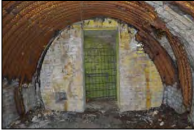
CFB17-0604 Air-raid shelter
