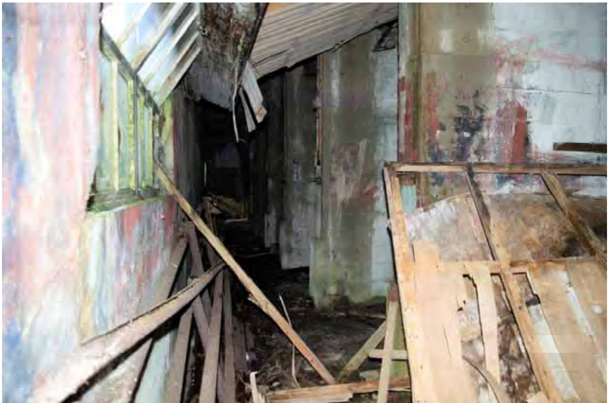
Plate 162: Store 14 – View of the western passage, facing north-west (479)
