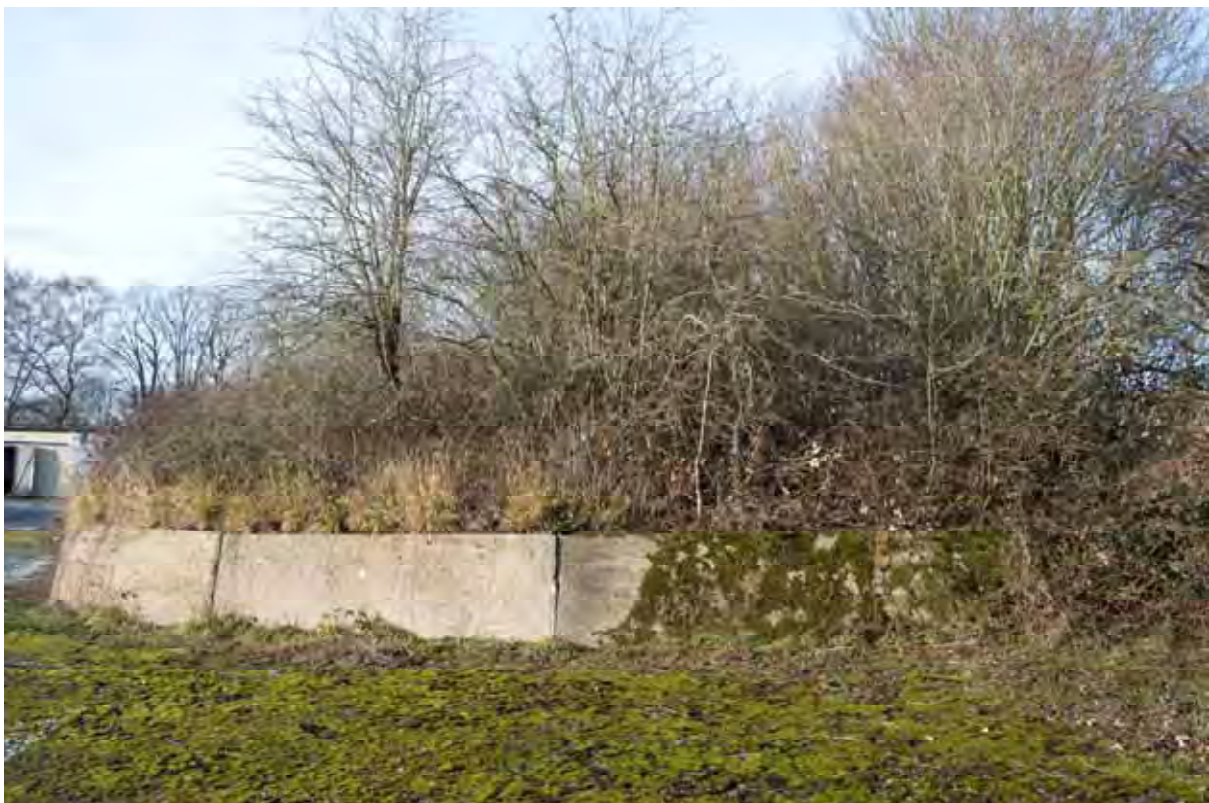
Plate 56: Bund separating Stores 4 and 5, facing north-west (289)
