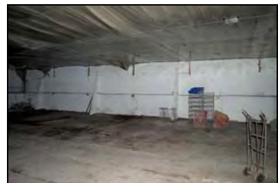
CFB17-0567 Building 10e (2017)
