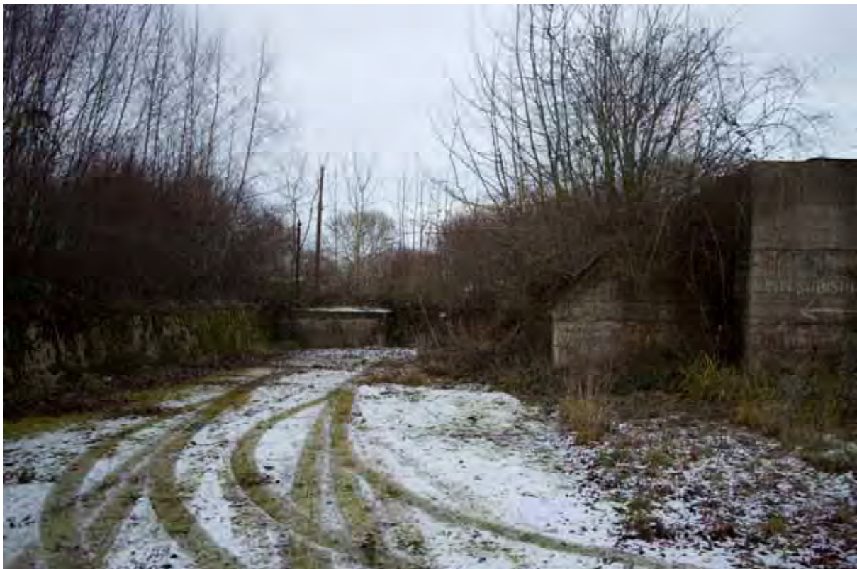
Plate 144: Store 12 – View of the northern loading bay, facing north-east (505)
