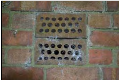
CFB17-0608 Air-raid shelter
