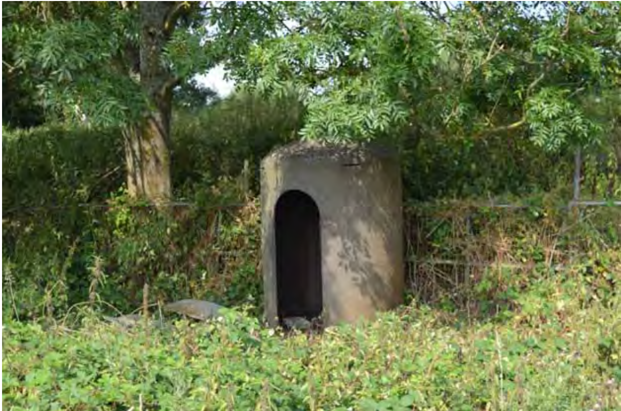
Plate 169: View of the south-eastern sentry post, facing north-west (590)
