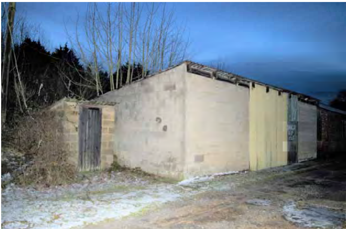
Plate 218: View of the north-east and south-east elevations of Building 11, facing north (572)
