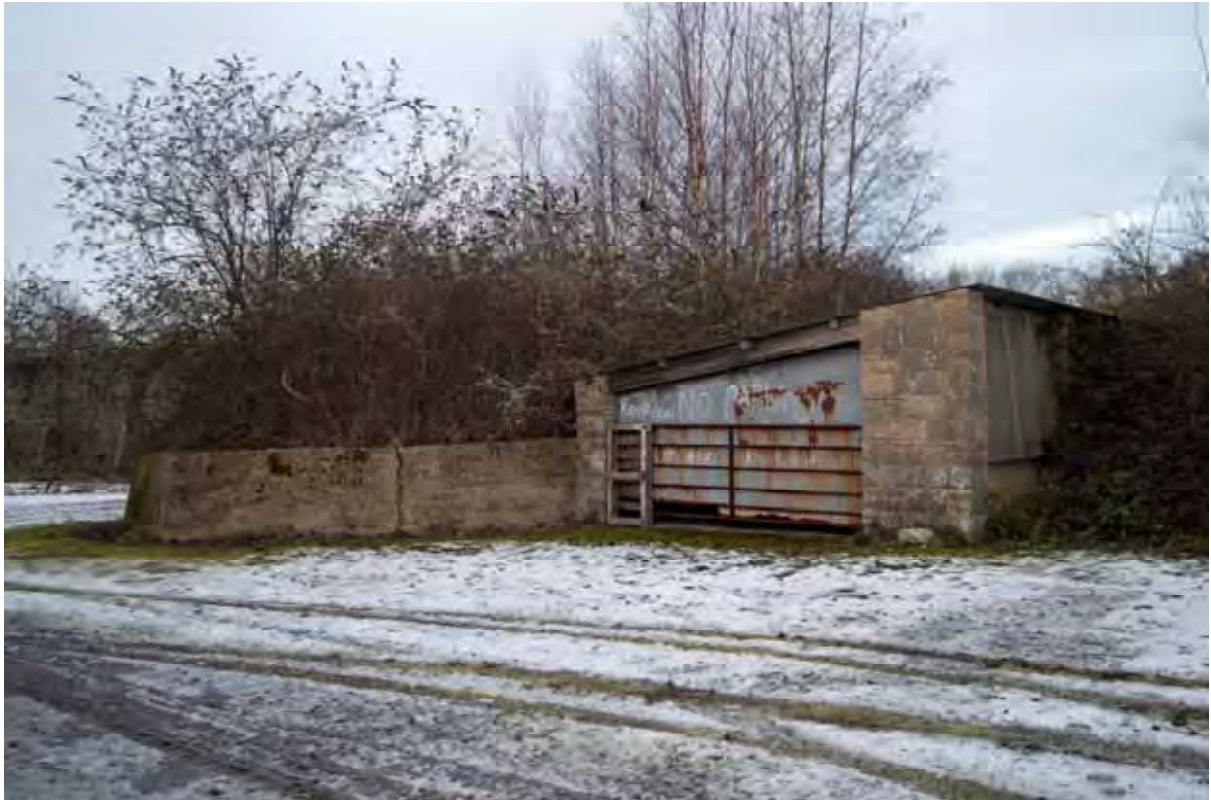
Plate 219: View of the south-west elevation of Building 13, facing north (484)
