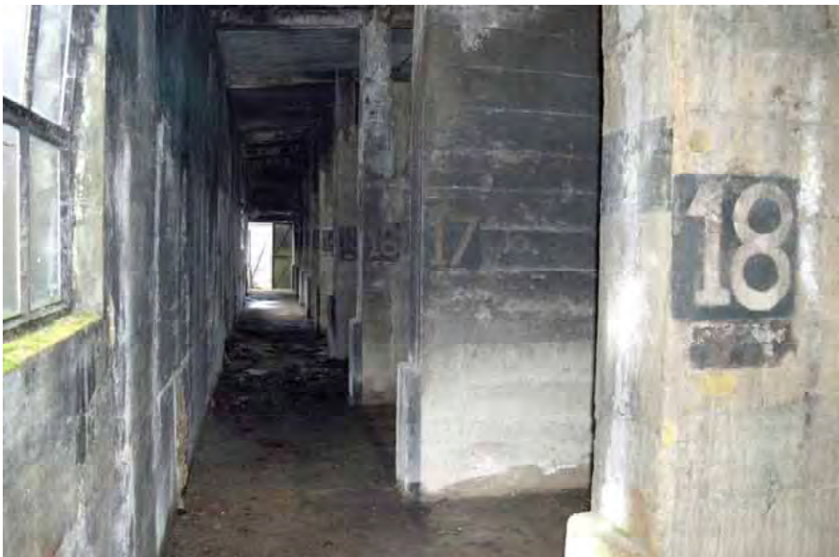
Plate 100: Store 8 – View of the western passage, facing north-west (434)
