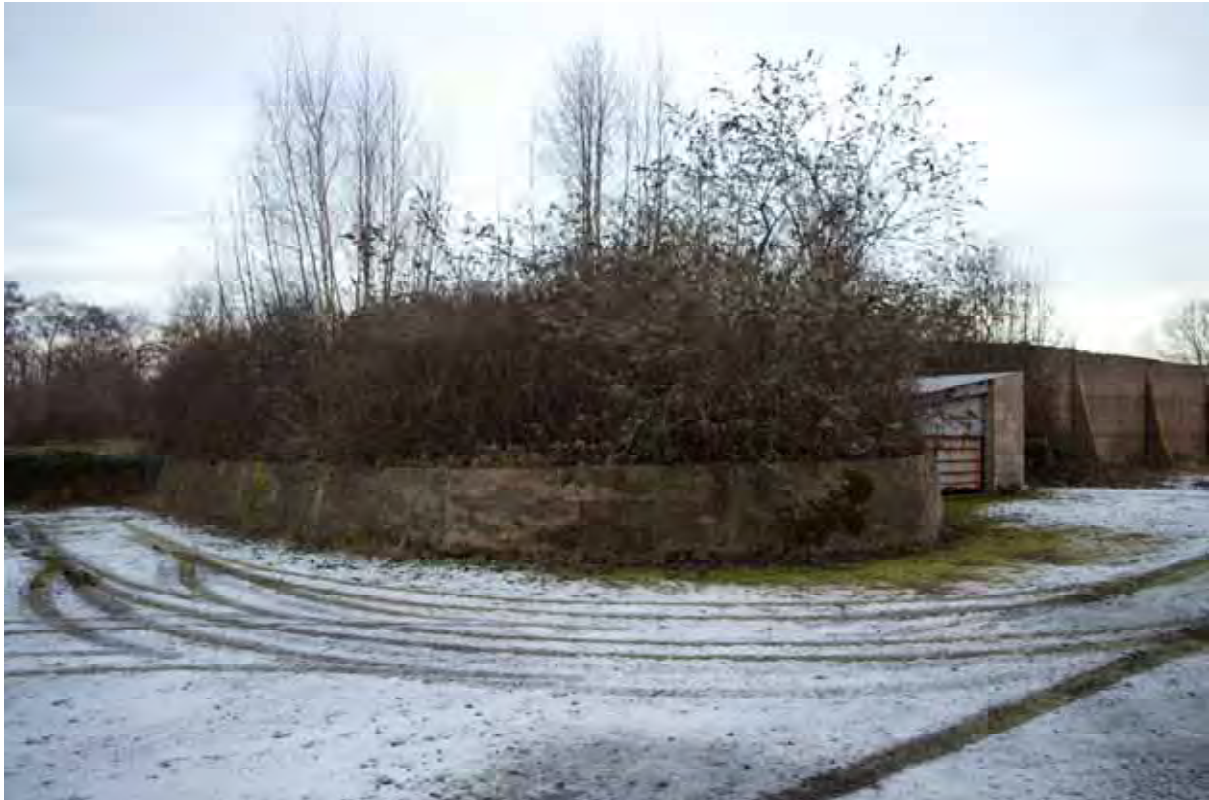
Plate 157: View of the bund separating Store 12 and 14, facing east (485)
