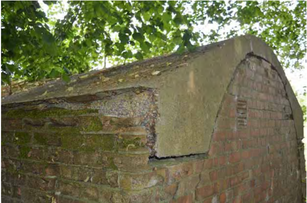
Plate 187: Detail of the air-raid shelter concrete roof cap, facing east (611)
