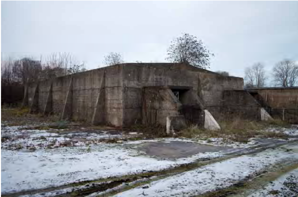
Plate 143: Store 12 – View of the south-east and south-west elevations, facing north (487)
