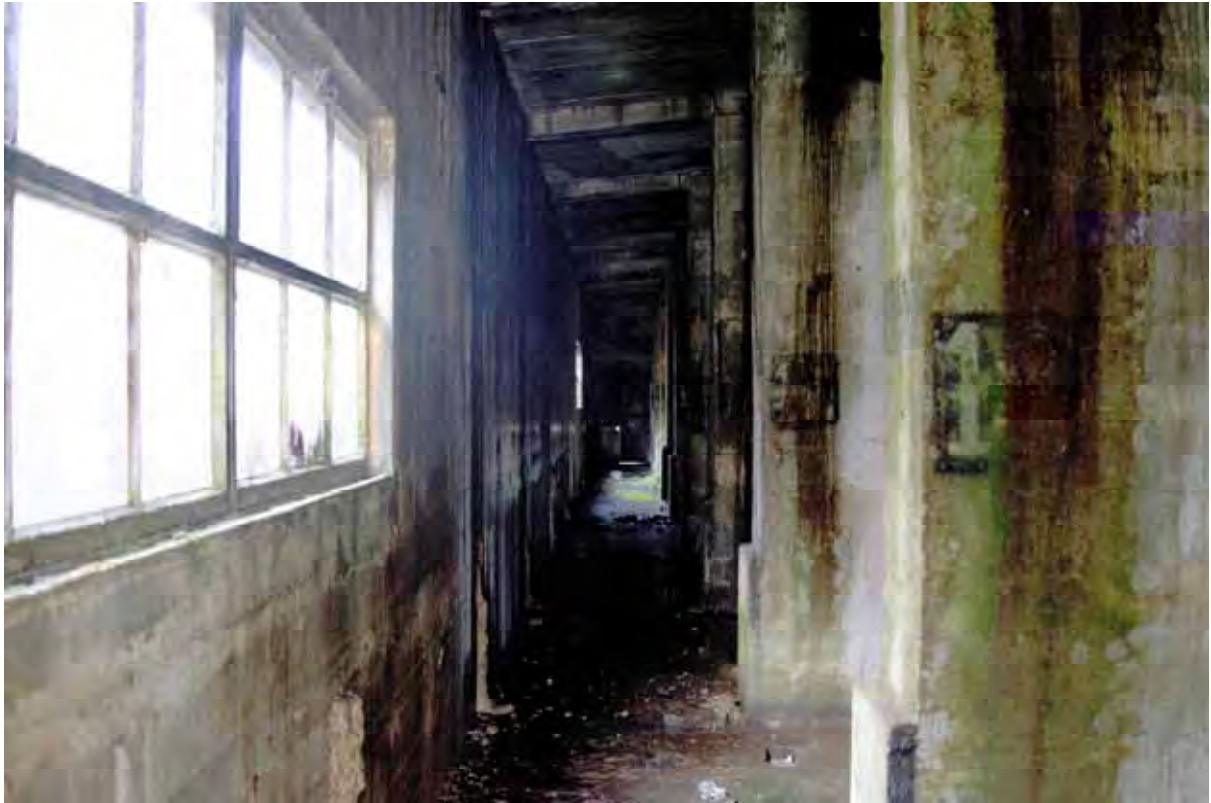
Plate 83: Store 6 – View of the western passage, facing north-west (338)
