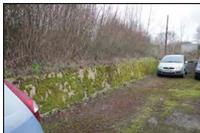
CFB17-0144 Bund separating Stores 12 and 10 (2015)
