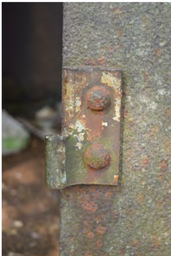
Plate 176: Detail of a door hinge serving the doorway on the south-eastern sentry post (592)
