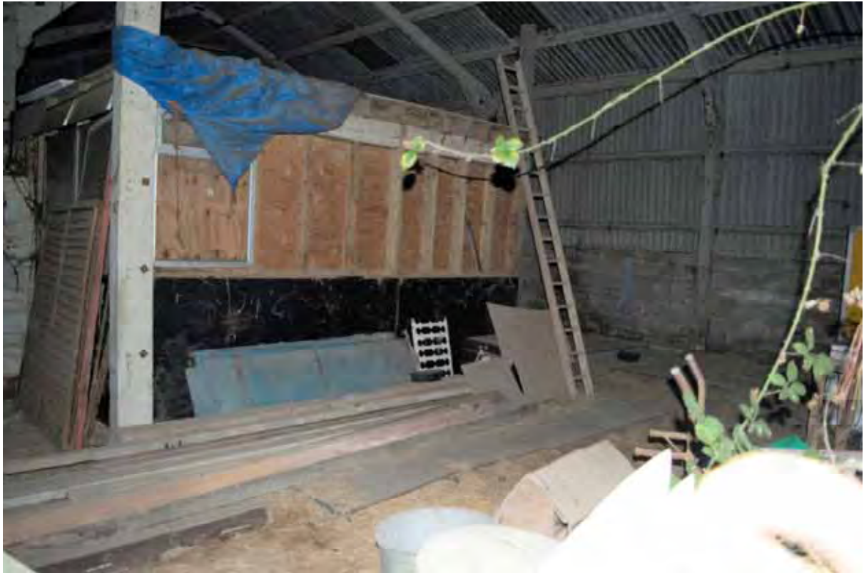
Plate 213: View of the interior of Building 10d, facing north (563)
