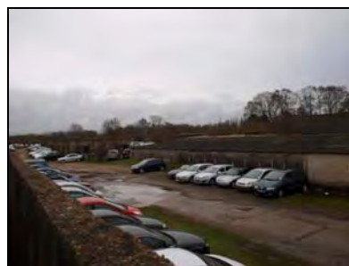
CFB17-0189 Store 4 - looking south-west across the site, Build 7 in foreground (2015)
