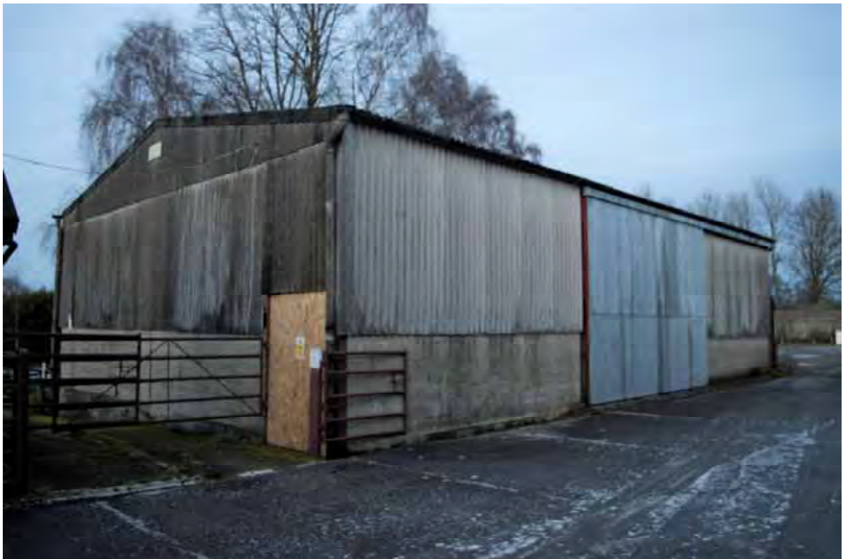
Plate 198: View of Building 2, facing north (545)
