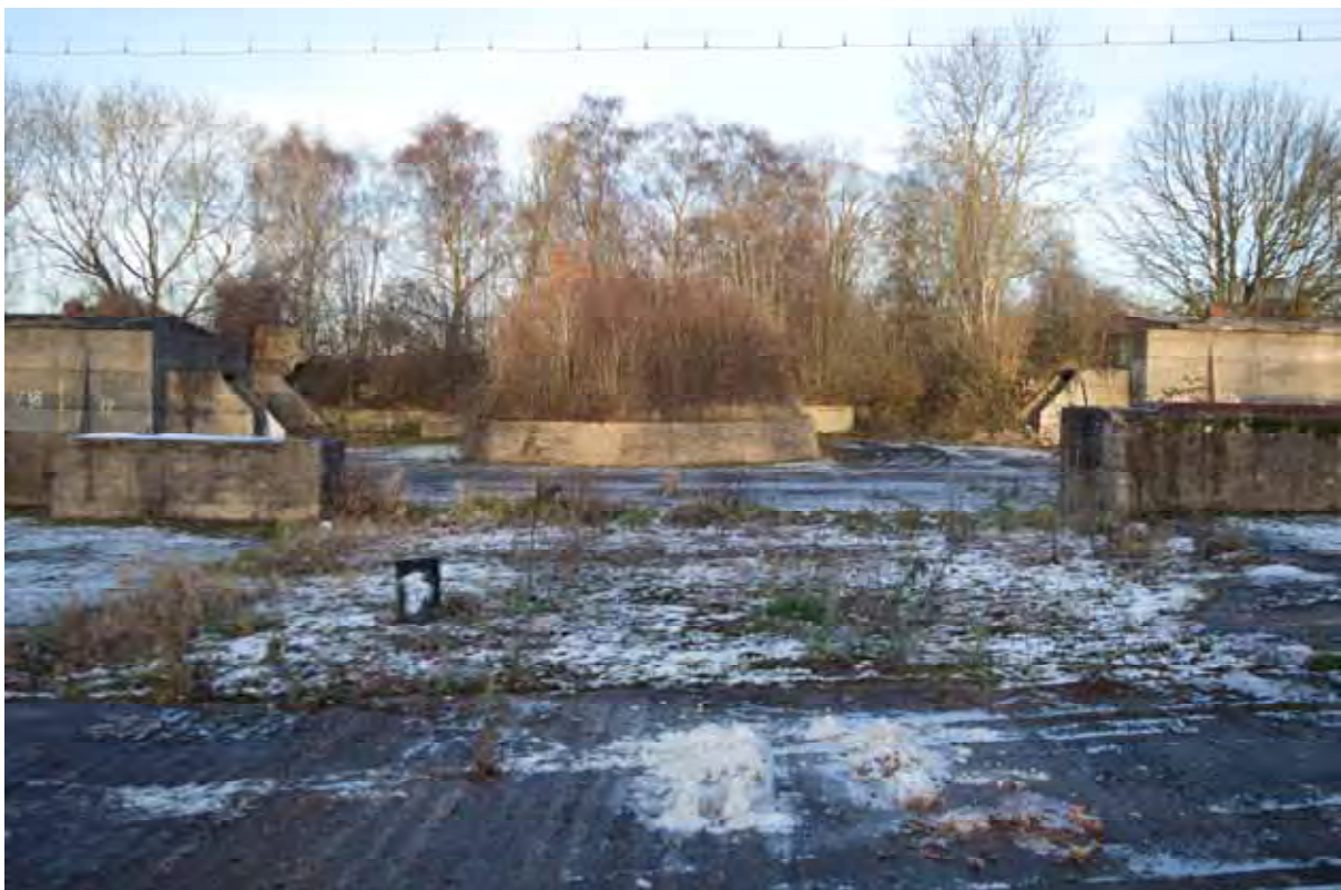
Plate 90: View of the area formerly occupied by the bund separating Stores 8 and 9 (removed after 1990), facing north-east (412)
