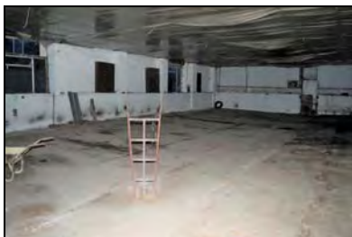
CFB17-0566 Building 10e (2017)
