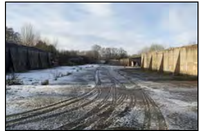
CFB17-0369 Road between Stores 9 (right) and 14 (left) (2017)
