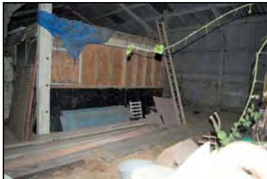
CFB17-0563 Buildings 10c and 10d (2017)
