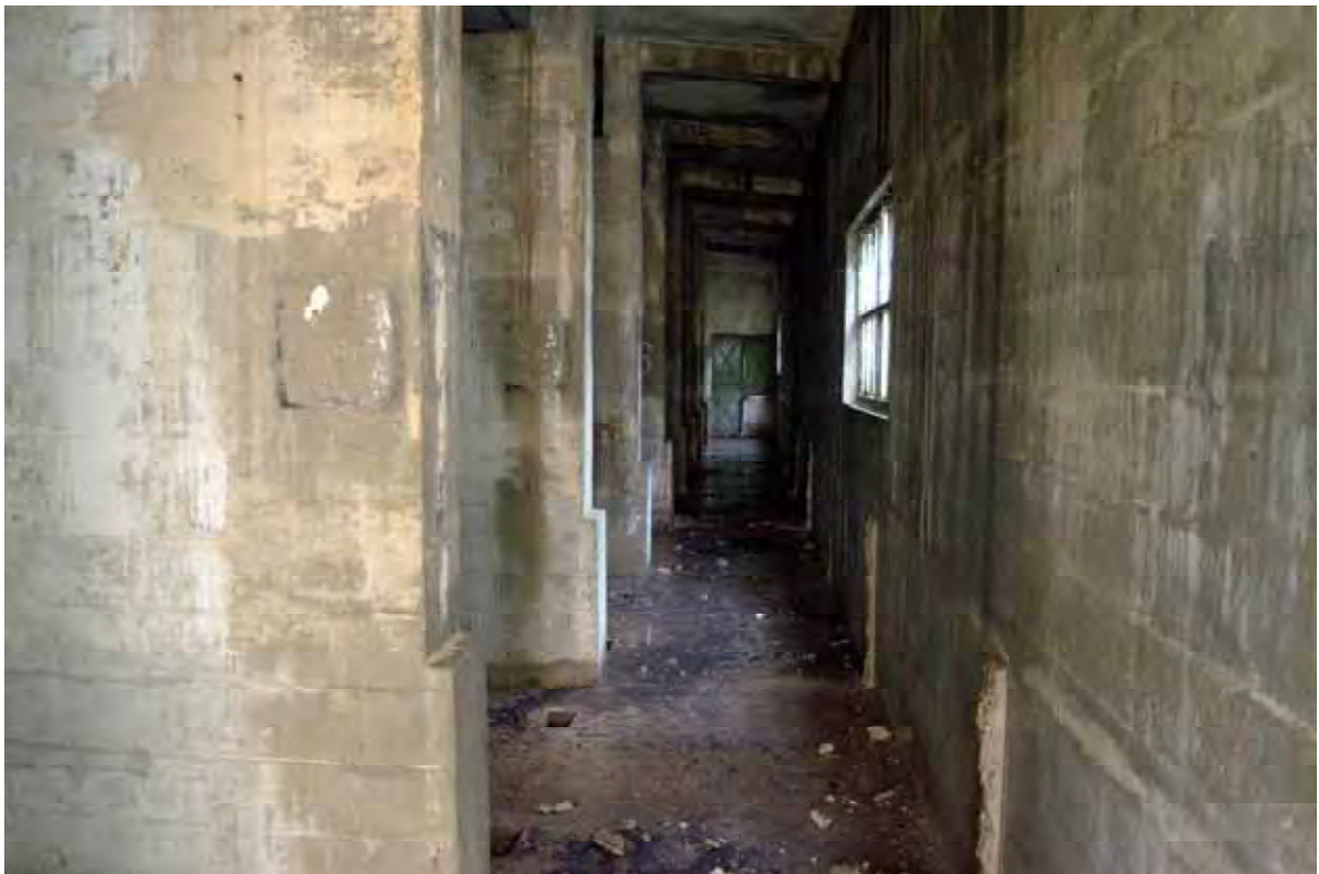
Plate 84: Store 6 – View of the eastern passage, facing north-west (349)
