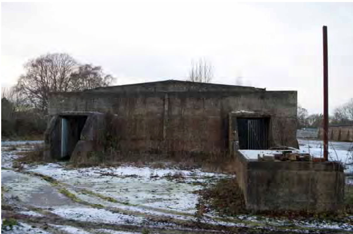
Plate 156: Store 14 – View of the southern loading bay, facing north-west (454)
