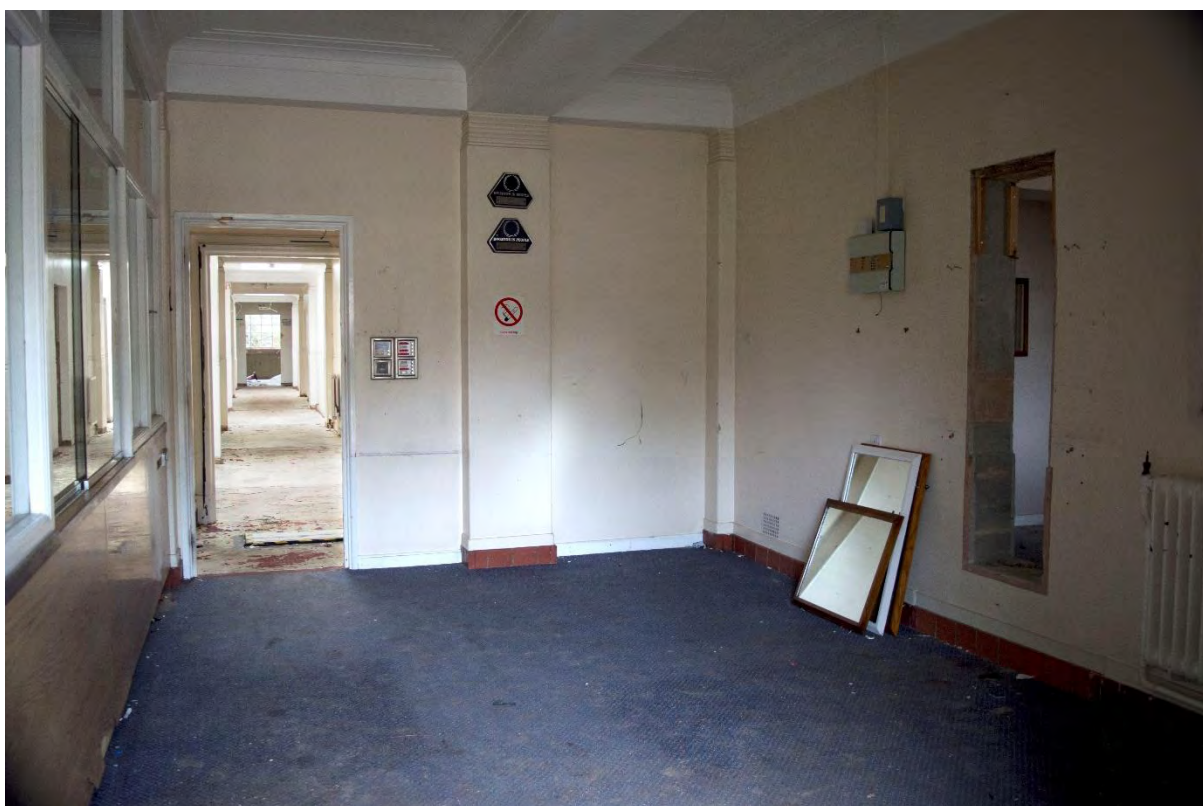
Plate 10 Building 1, entrance/administrative block, main entrance hallway, facing south (FHH17-0994)
