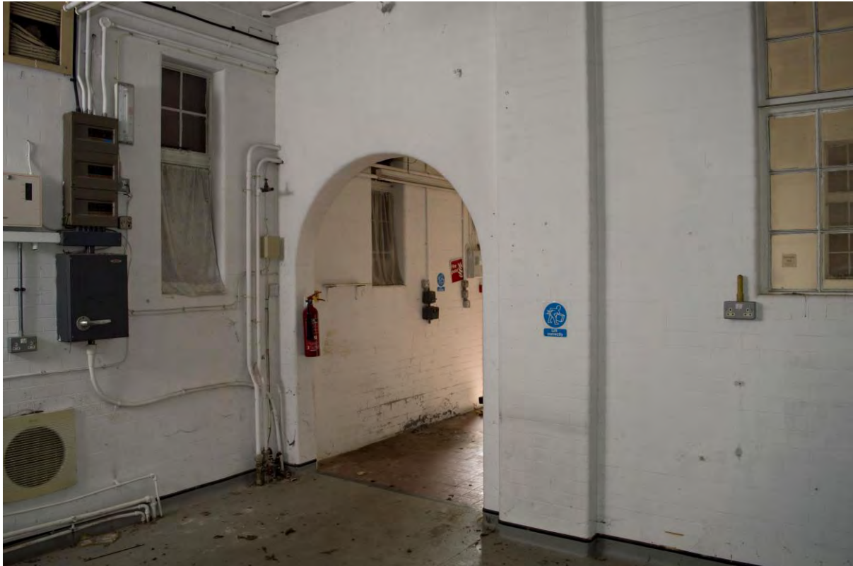
Plate 103 Building 12, disinfectant block, interior of west room, facing north-east (FHH17-0230)
