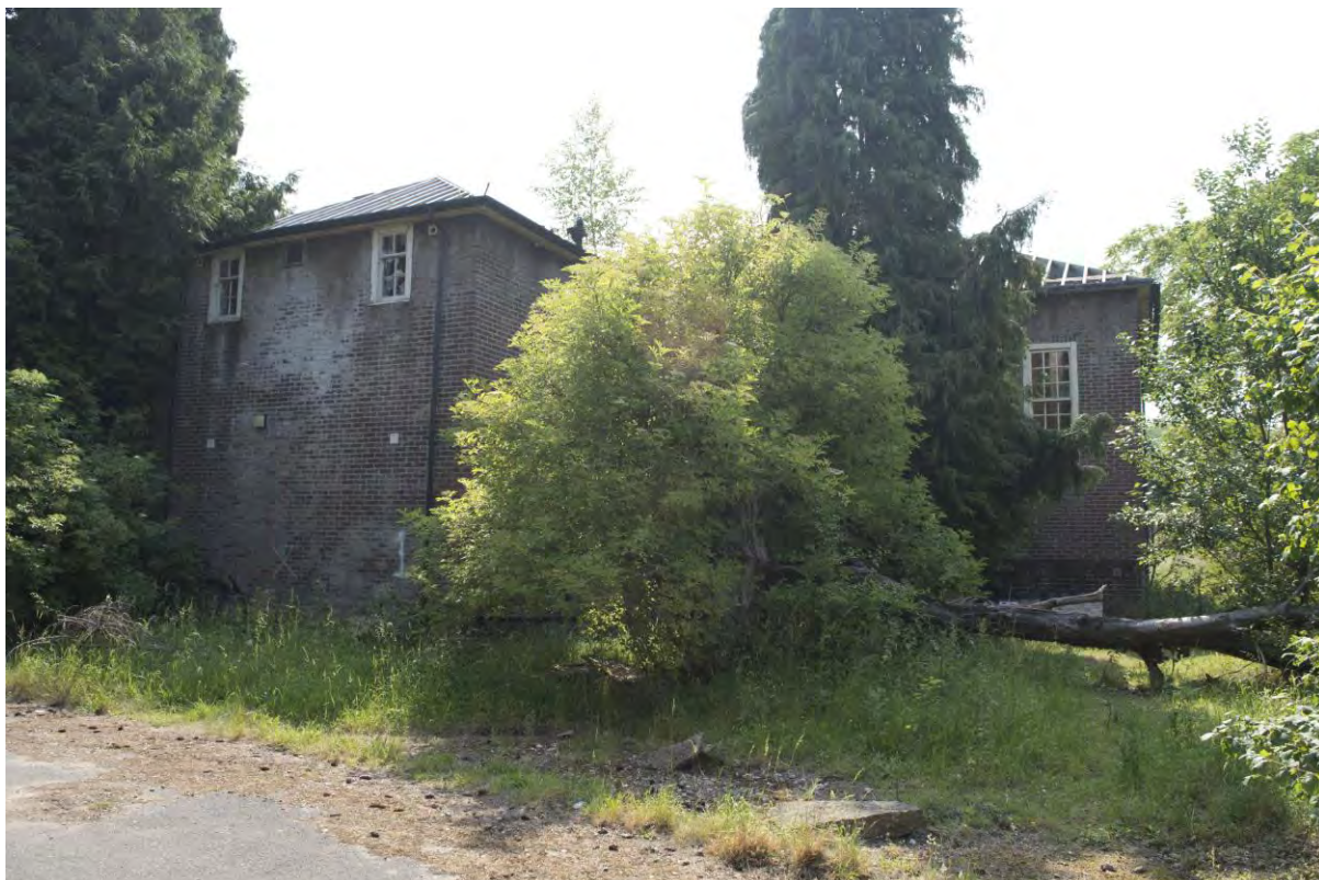
Plate 191 Building 40, male villa, rear (north-west) elevation, showing sanitary annexe (FHH17-0335)
