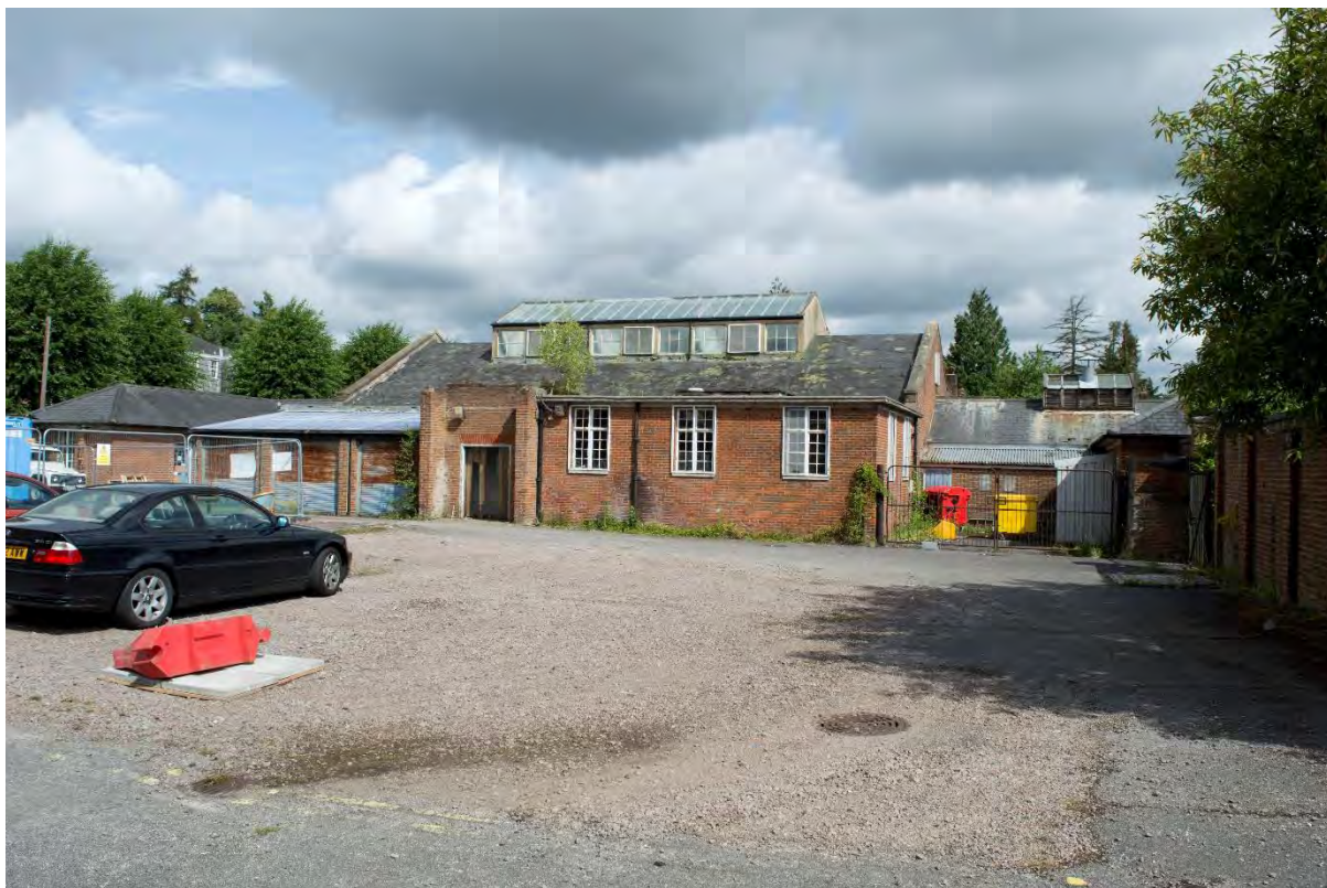
Plate 9 Building 1, central kitchen, facing north-north-west (FHH17-460)
