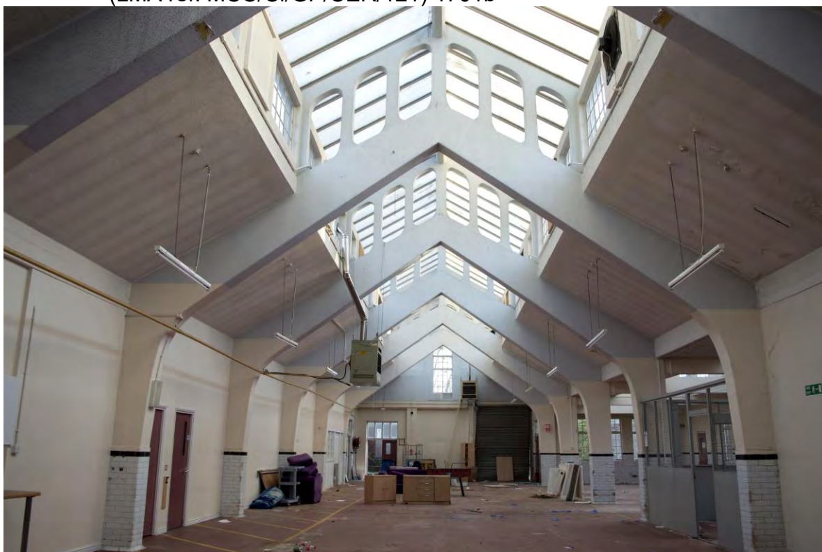
Plate 92 Building 11, general laundry, interior of main range, facing south (FHH17-0701)
