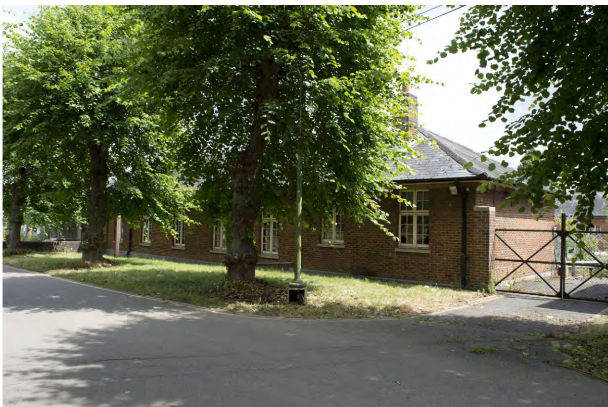
Plate 51 Building 5, workshop on west side of boiler house, west elevation, facing north-west (FHH17-0524)
