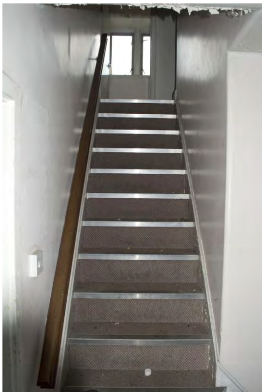
Plate 166 Building 29, gate lodge, front entrance lobby and stairs, facing west (FHH17-0259)
