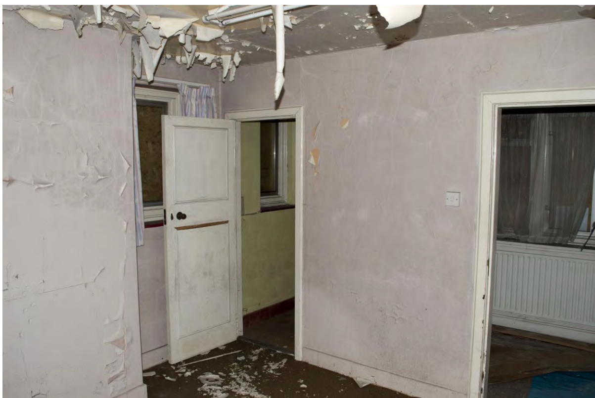
Plate 167 Building 29, gate lodge, north-west room, facing north-east (FHH17-0262)
