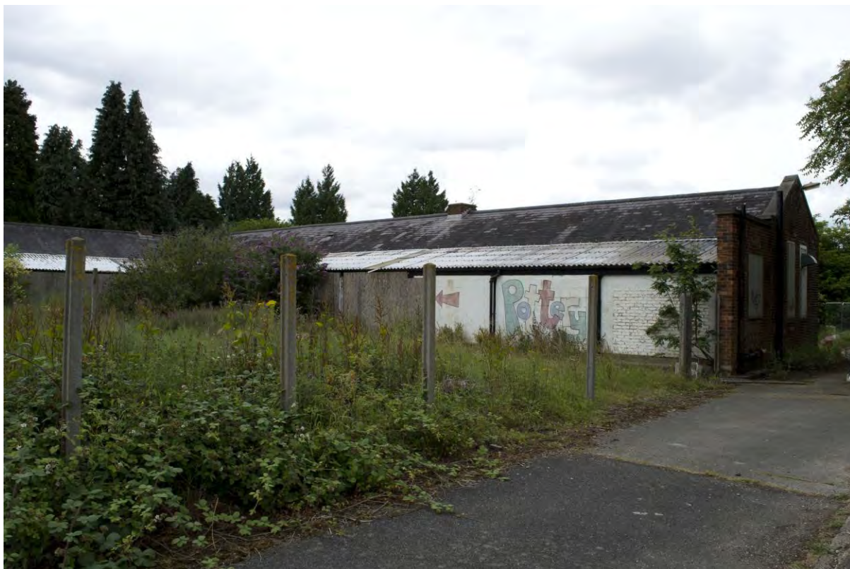
Plate 182 Building 35, workshops, yard elevation of north range, facing north-west (FHH17-0643)
