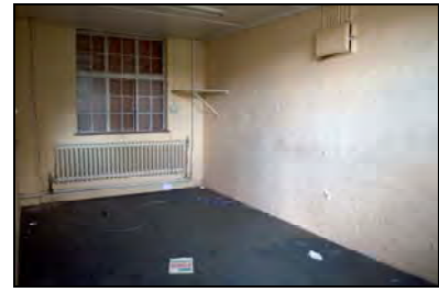
FHH17-0666 Building 07 interior start
