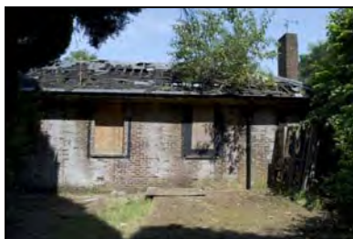
FHH17-0410 Buildings 40 to 53 end
