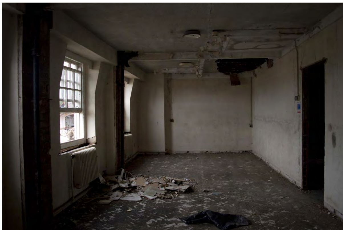
Plate 126 Building 28, nurses' home, nurses' lounge on second floor, facing south (FHH17-1405)
