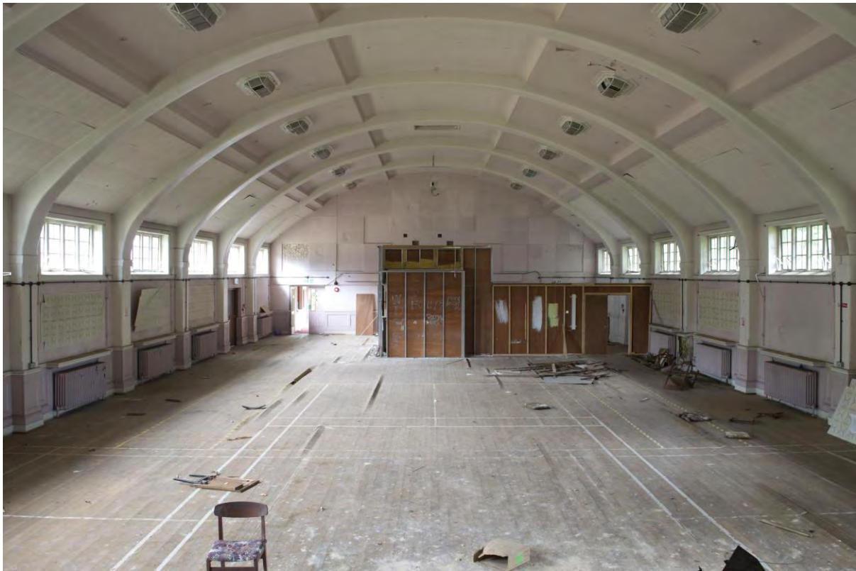
Plate 44 Building 4, recreation hall, facing north (FHH17-0107)
