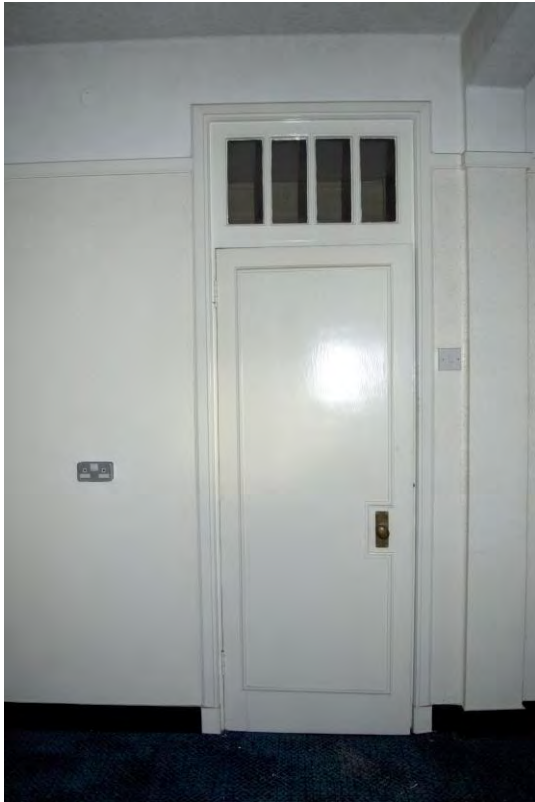
Plate 157 Building 27, nurses' home, typical door, ground floor (FHH17-0956)
