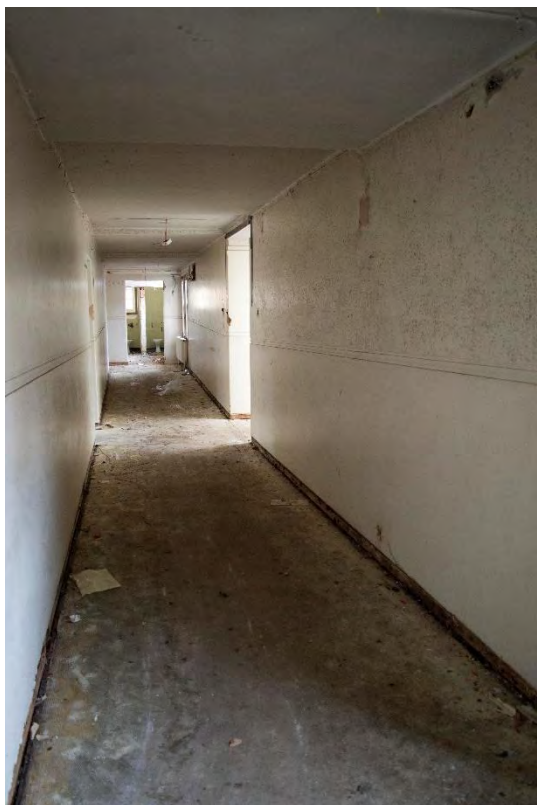
Plate 17 Building 1, dispensary block, corridor to north of dispensary, facing west (FHH17-1091)
