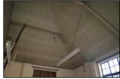
FHH17-0687 Building 09 interior end
