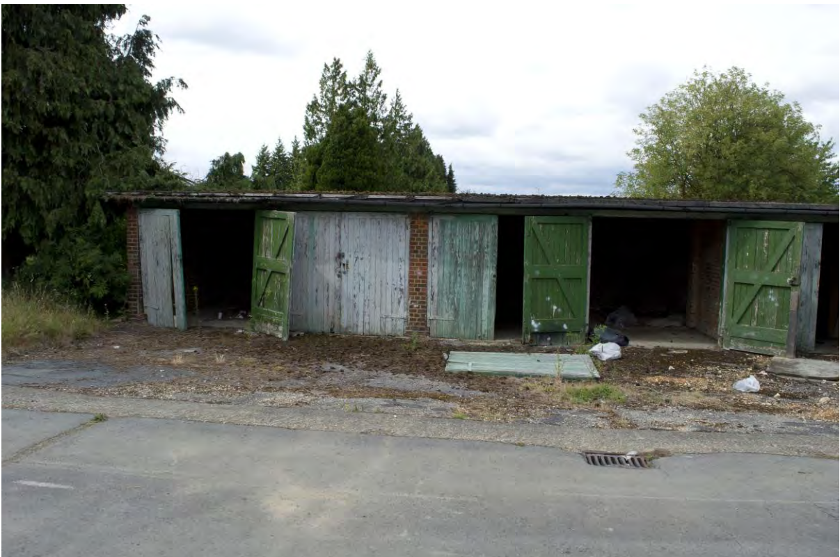
Plate 185 Building 36, south range of larger garages, facing north (FHH17-0316)
