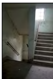
FHH17-0982 Building 28 stairs start
