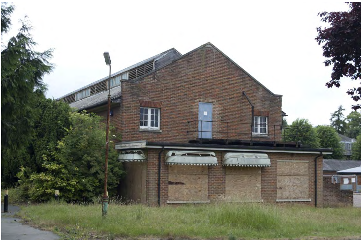
Plate 27 Building 3, main stores, east elevation (FHH17-0007)
