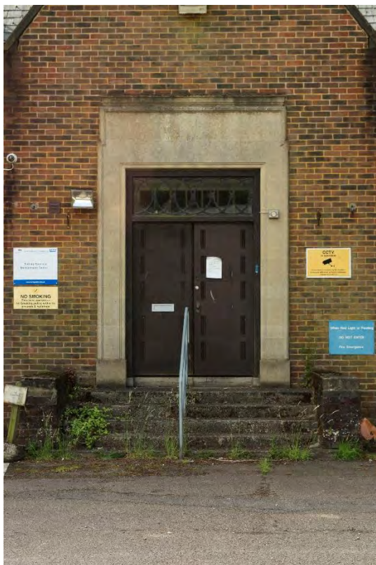
Plate 3 Building 1, detail of principal entrance (FHH17-447)
