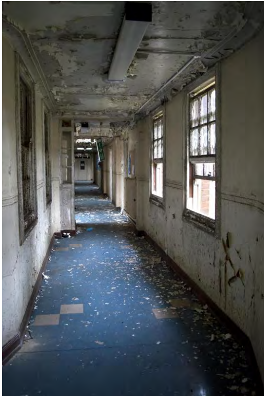
Plate 139 Building 26, nurses' home, corridor, facing north (FHH17-1180)
