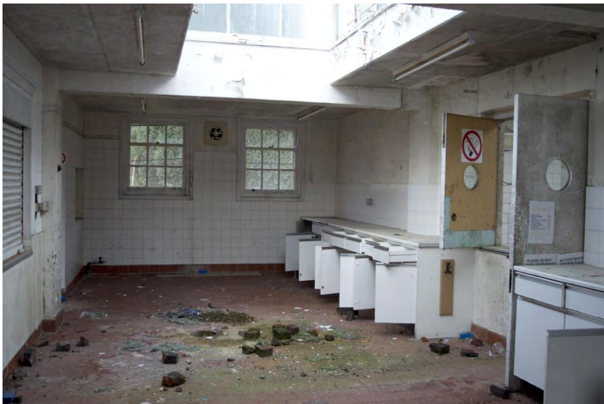
Plate 149 Building 26, nurses' home, scullery and servery, facing north (FHH17-1223)
