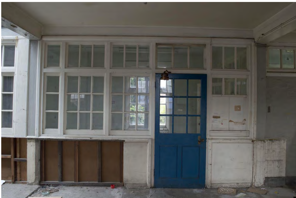
Plate 32: Building 3, main stores, ground floor partition, facing south (FHH17-0026)
