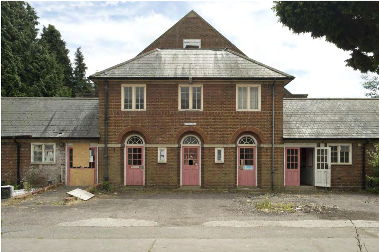
Plate 36 Building 4, recreation hall, north elevation (FHH17-0077)
