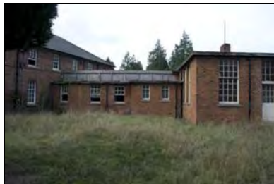
FHH17-0743 Building 26 courtyard external start
