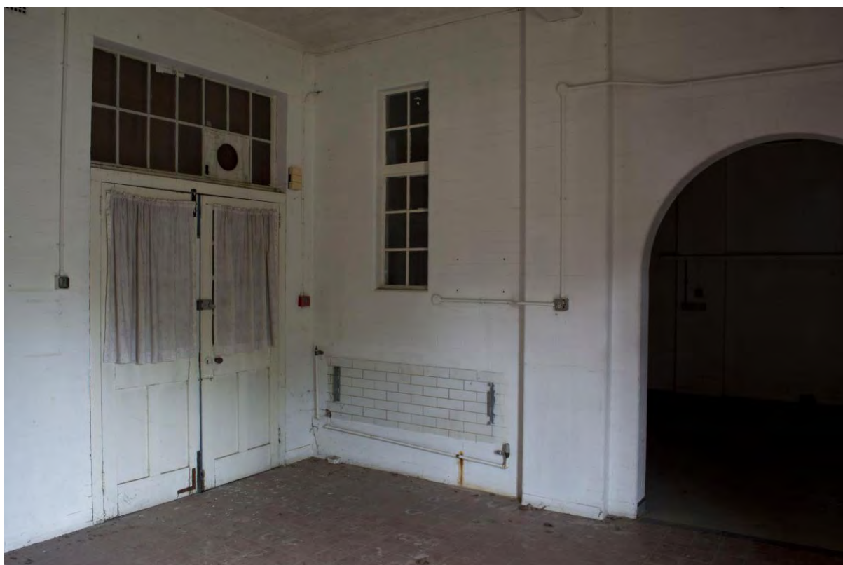
Plate 102 Building 12, disinfector block, interior of east room, facing south-west (FHH17-0226)
