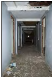
FHH17-1387 Building 28 internal start
