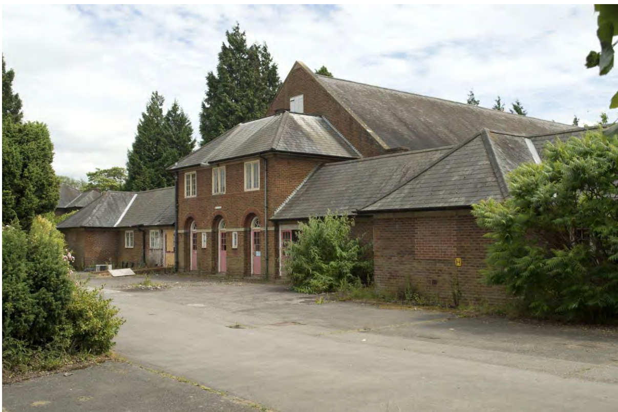
Plate 37 Building 4, recreation hall, north elevation, facing south-east (FHH17-0081)
