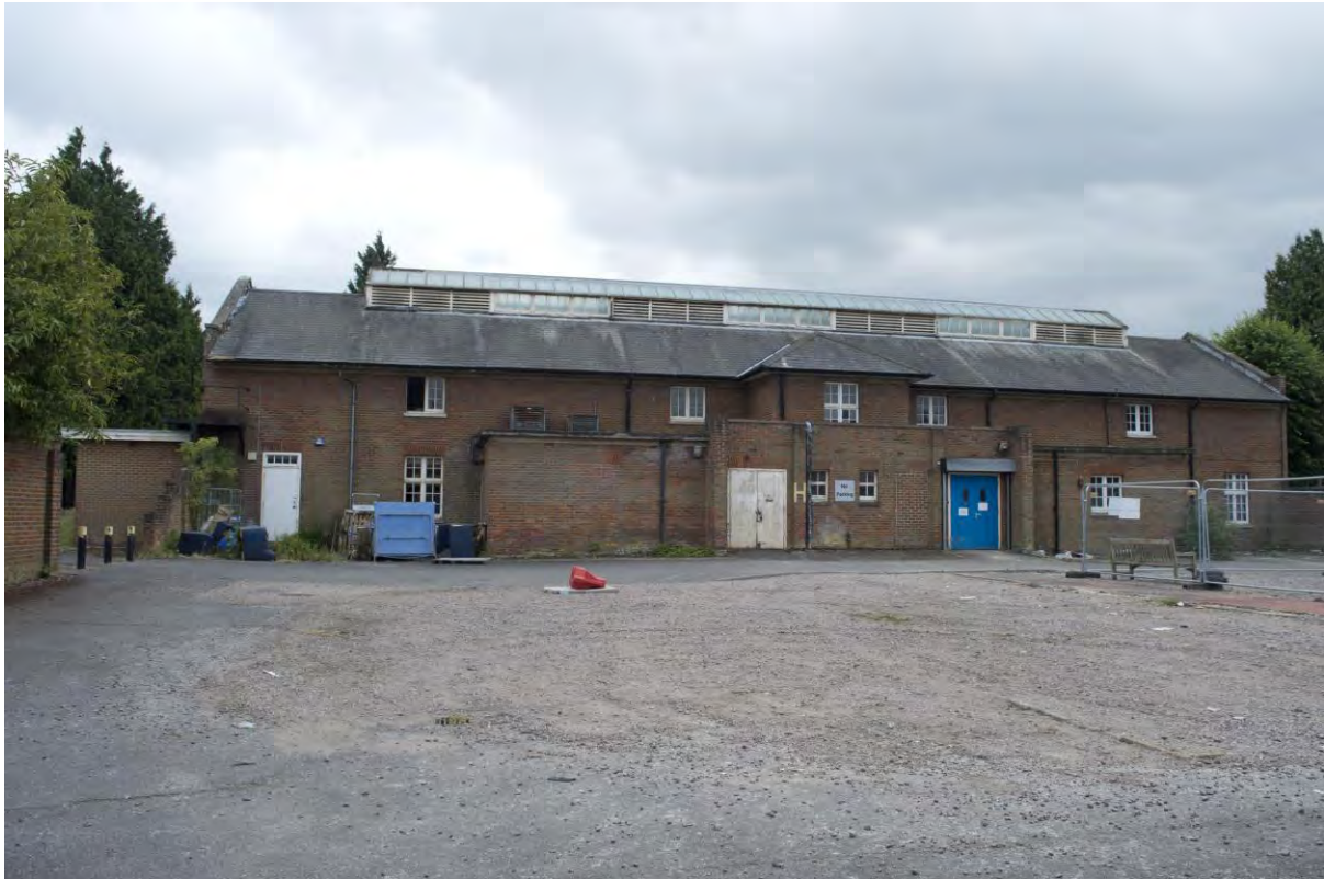
Plate 28 Building 3, main stores, north elevation (FHH17-0010)
