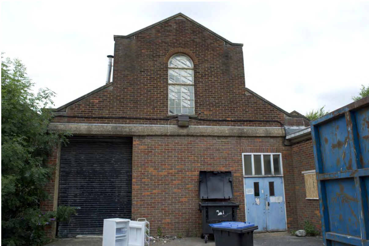
Plate 89 Building 11, general laundry, detail of south elevation of main range (FHH17-0540)
