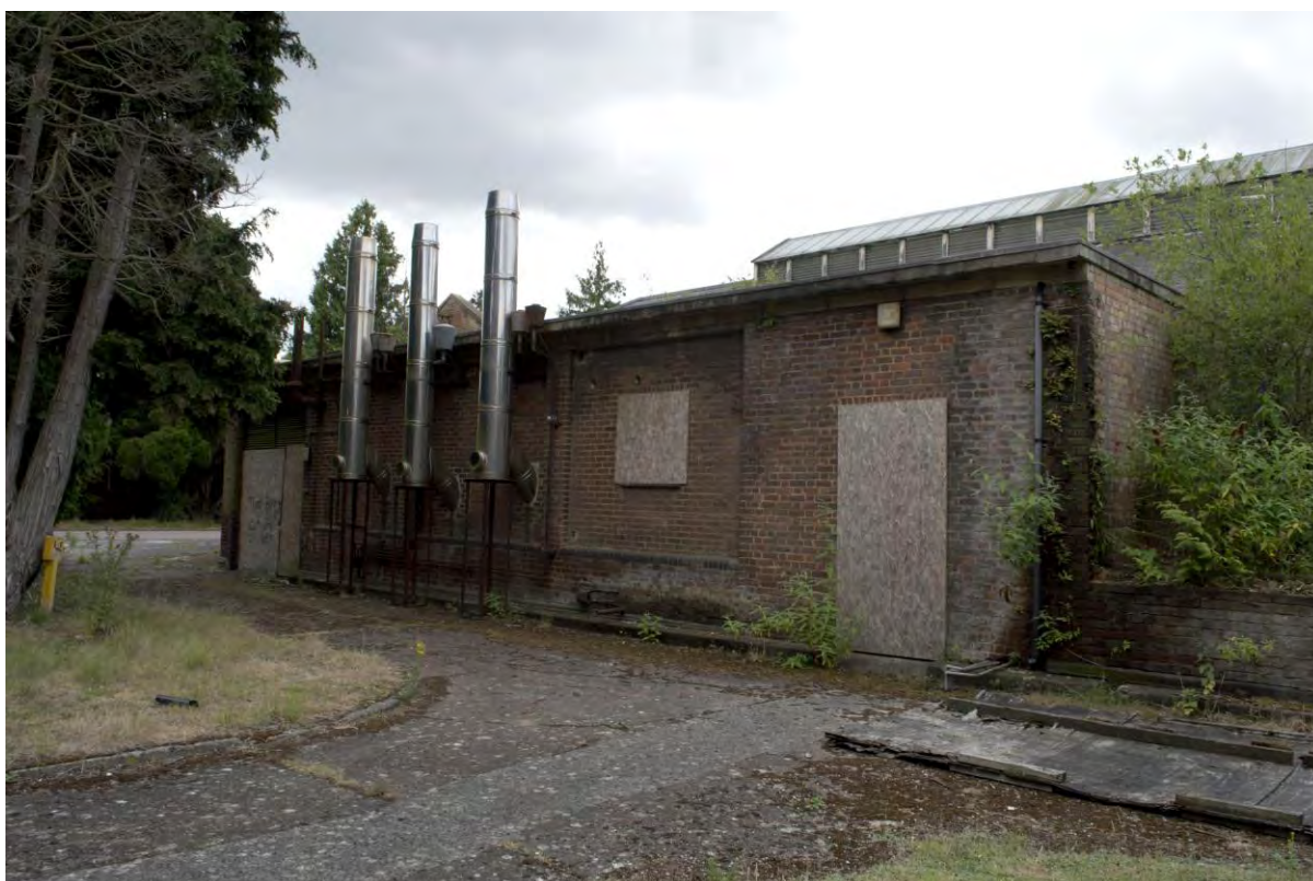
Plate 49 Building 5, boiler house, north elevation of block to north, facing south-east (FHH17-0478)
