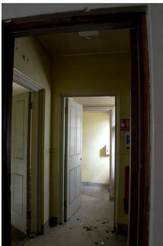
Plate 47 Building 4, recreation hall, side wing to east of stage, facing east (FHH17-0126)
