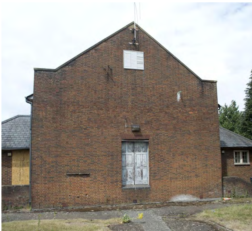
Plate 39 Building 4, recreation hall, south elevation (FHH17-0092/0093)
