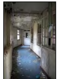
FHH17-1176 Building 26 internal start
