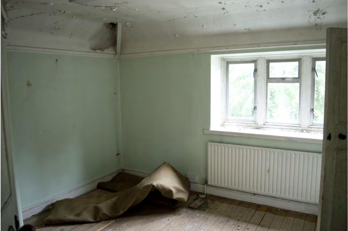
Plate 168 Building 29, gate lodge, first floor north-east room, facing north-east (FHH17-0270)
