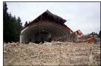
FHH17-1431 Building 4 during demolition
