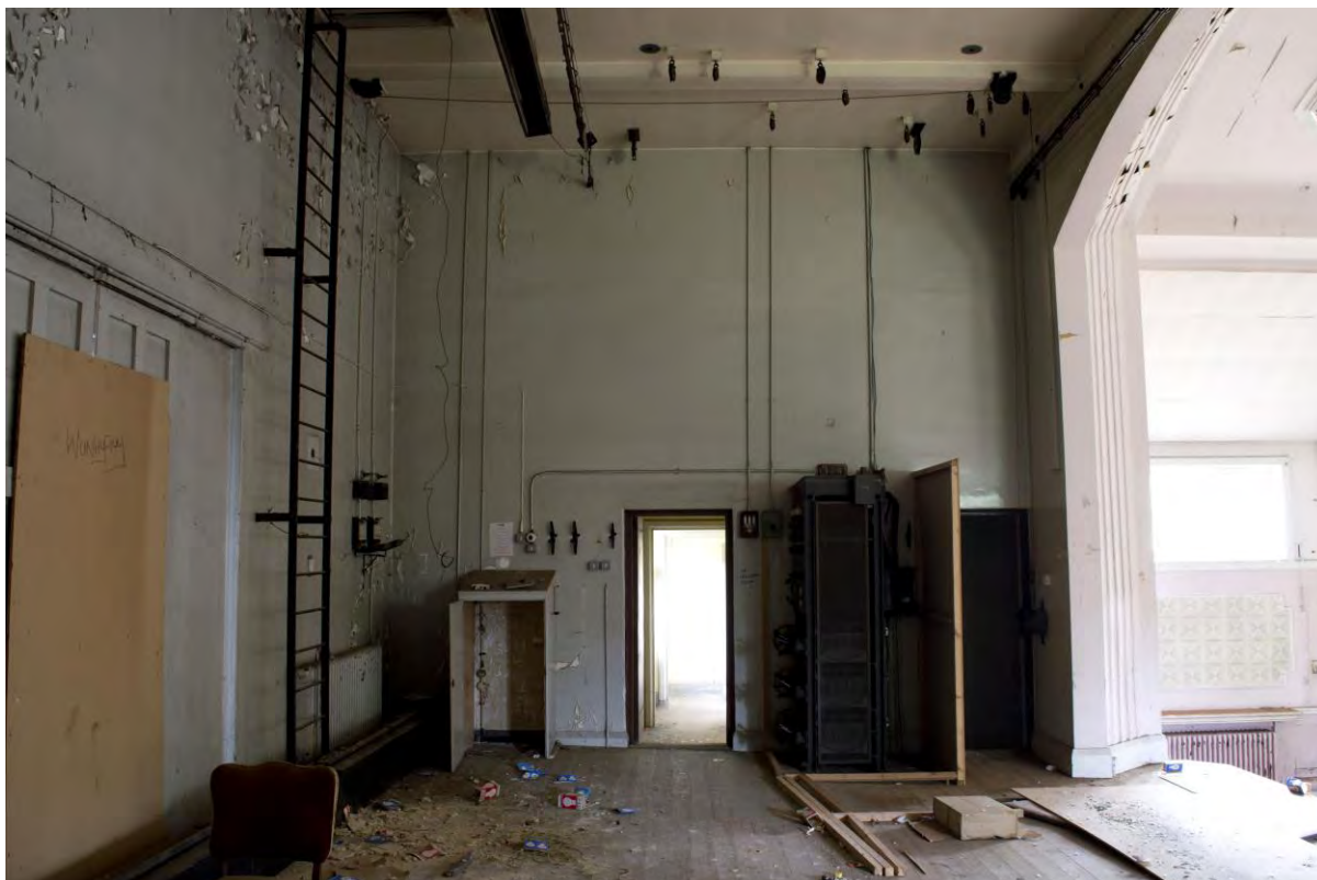
Plate 46 Building 4, recreation hall, stage, facing west (FHH17-0121)
