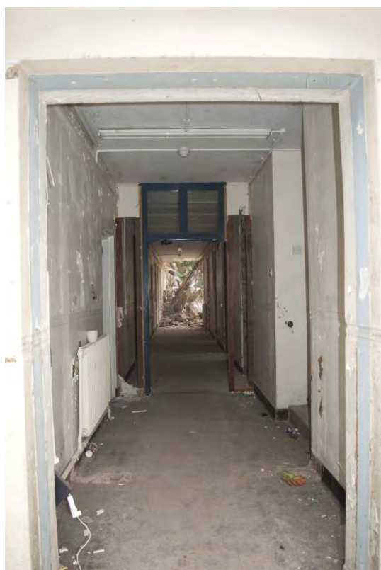
Plate 132 Building 25, nurses' home, ground floor corridor, facing west (FHH17-1281)
