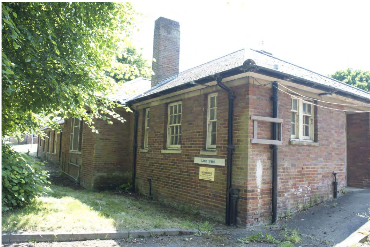
Plate 105 Building 13, fire training building, north and east elevation, facing south-west (FHH17-0248)
