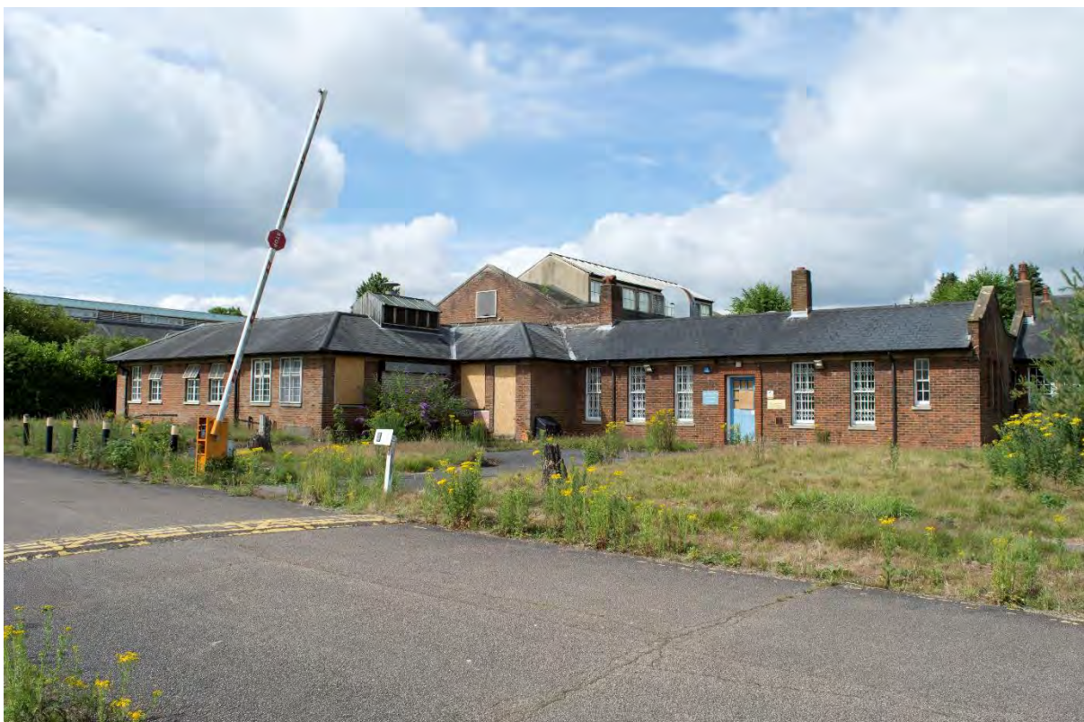
Plate 6 Building 1, dispensary and kitchen blocks, facing south-west (FHH17-456)
