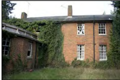
FHH17-0758 Building 27 courtyard external start
