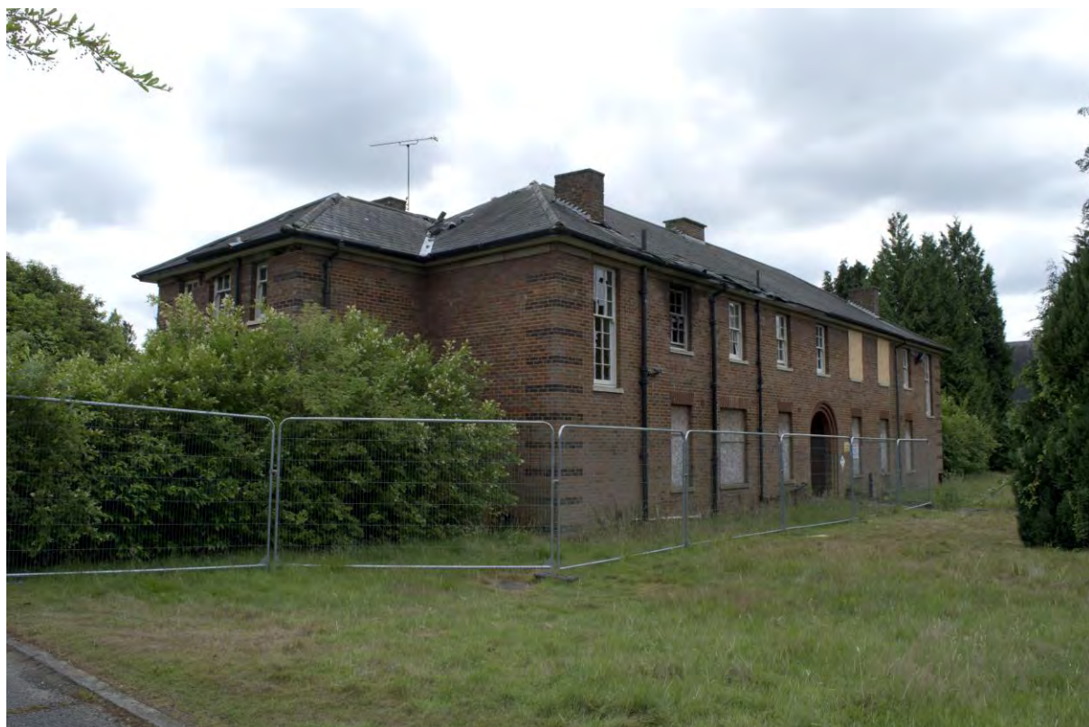
Plate 174 Building 34, male nurses' quarters, north and east elevations, facing south-west (FHH17-0612)
