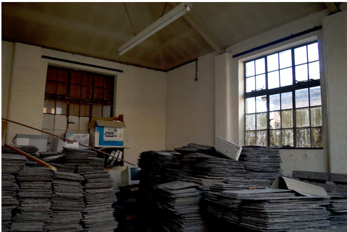
Plate 80 Building 9, workshop, former repair garage at north end of range, facing north-east (FHH17-0686)
