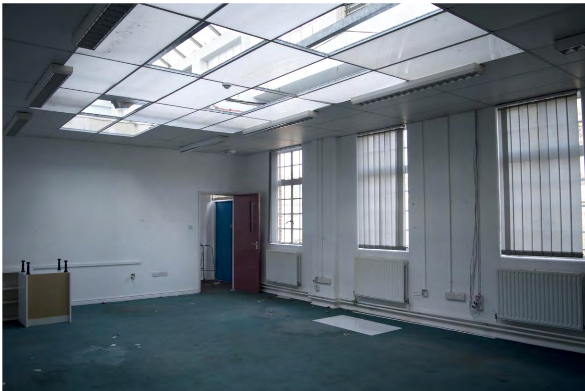
Plate 97 Building 11, general laundry, modernised interior of east flanking range, facing north-east (FHH17-0692)
