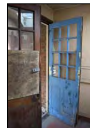
FHH17-1269 Building 26 internal end
