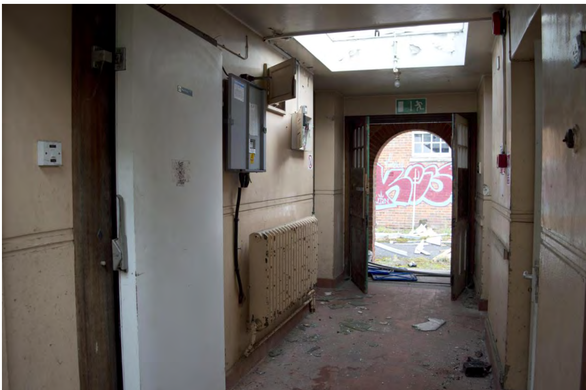
Plate 152 Building 26, nurses' home, corridor to east of kitchens, facing east (FHH17-1245)
