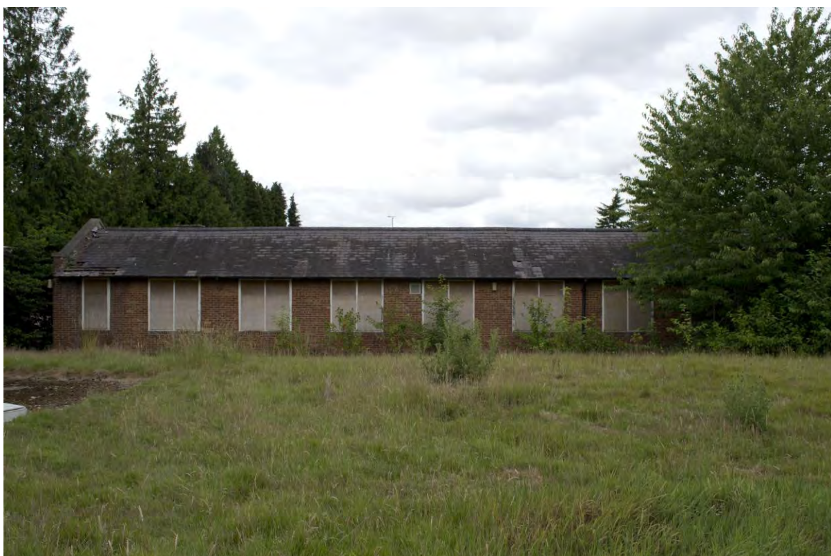
Plate 179 Building 35, workshops, south elevation of south range (FHH17-0630)
