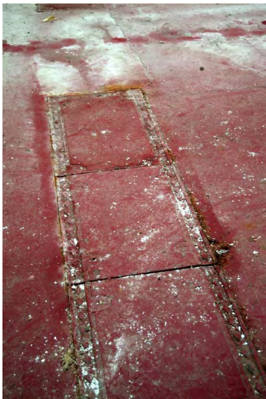
Plate 93 Building 11, general laundry, floor ducts in main range (FHH17-0704)
