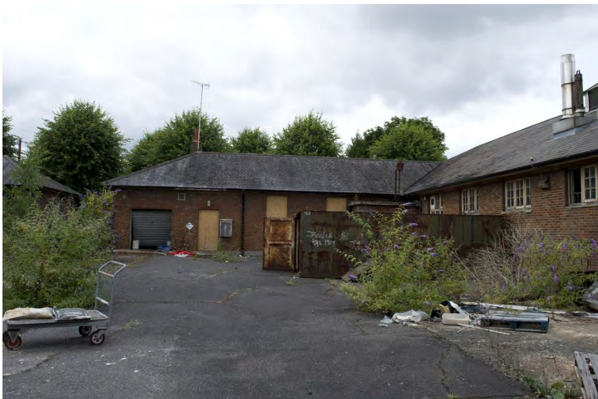
Plate 53 Building 5, boiler house and workshop, facing west across the yard (FHH17-0497)
