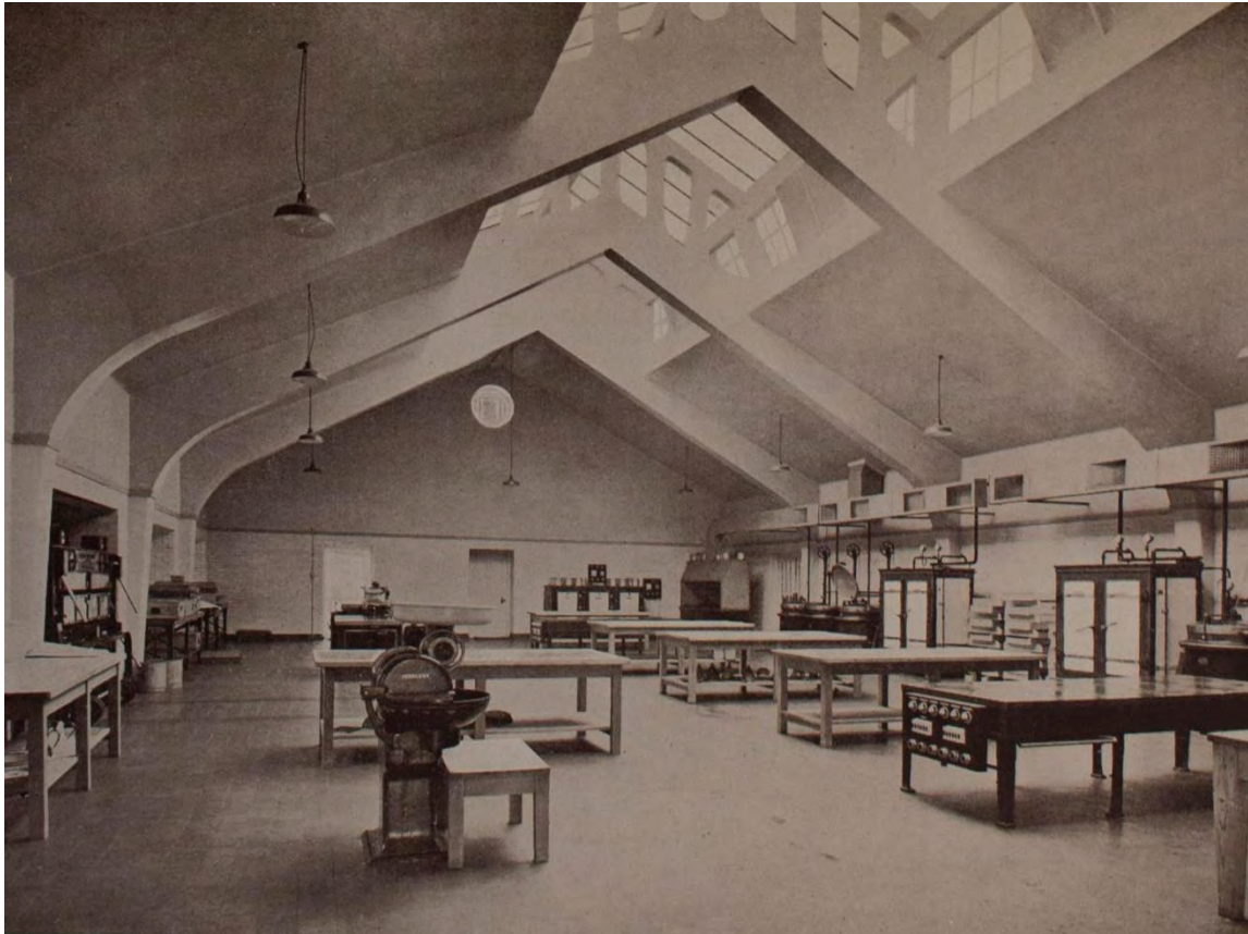
Plate 21 Building 1, central kitchen, 1936, facing north-west (LMA ref. MCC/CI/GP/CER/121) 1696b
