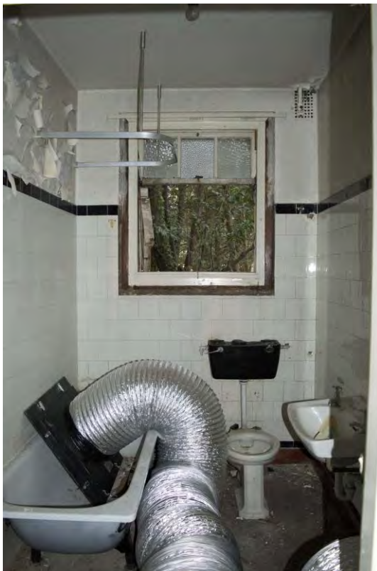
Plate 160 Building 27, nurses' home, bathroom within ground floor flat, facing west (FHH17-1337)
