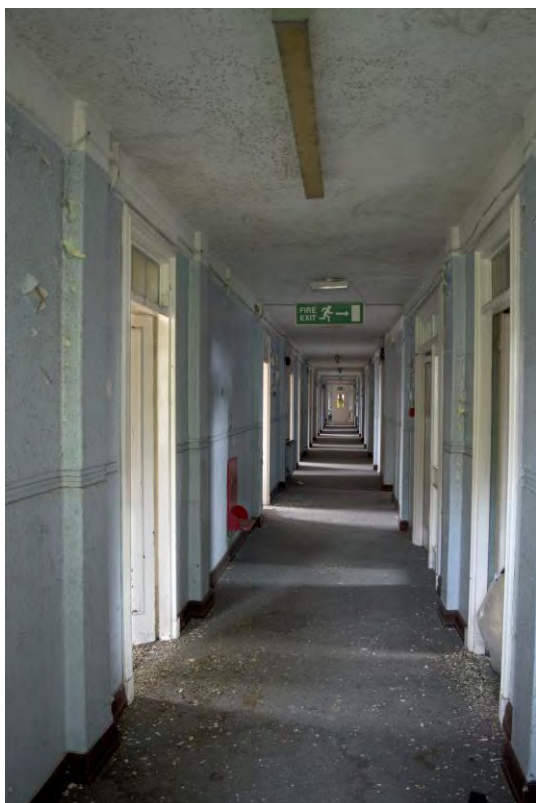
Plate 116 Building 28, nurses' home, first floor corridor, facing south (FHH17-0783)
