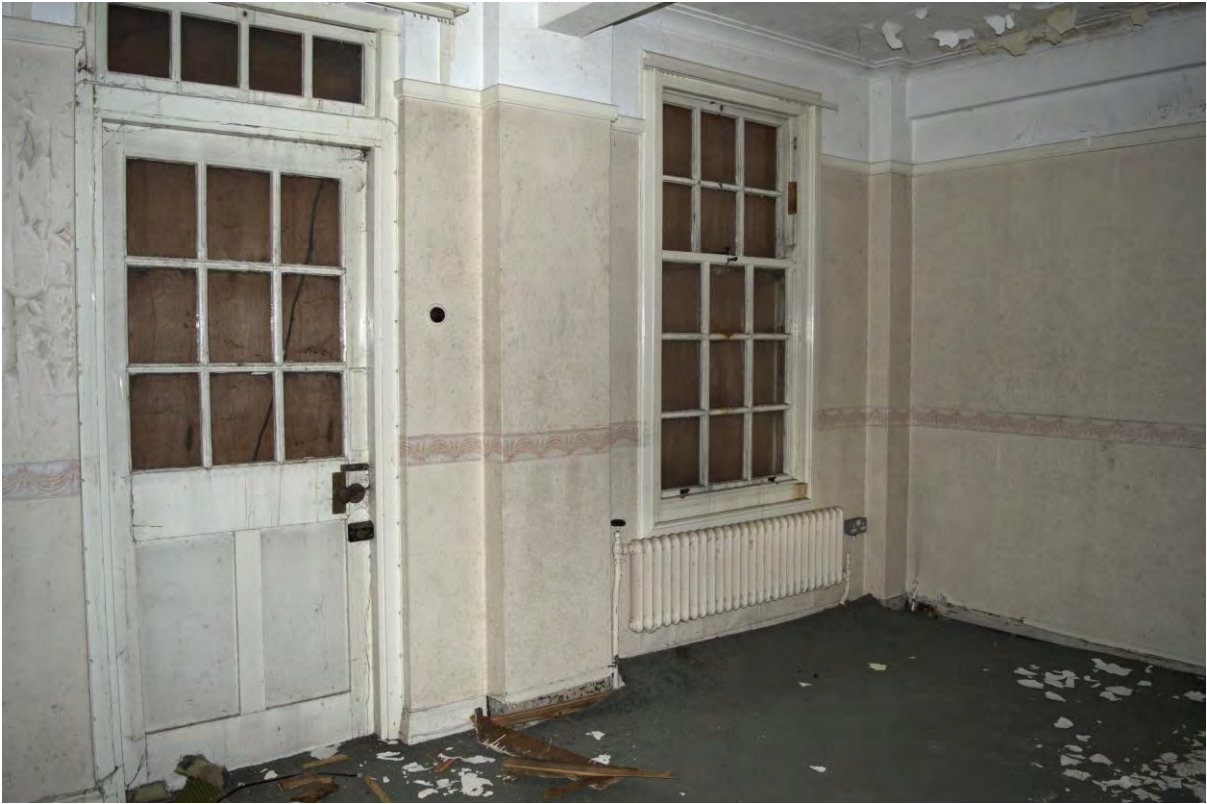
Plate 163 Building 27, nurses' home, dining room, facing north-east (FHH17-0968)
