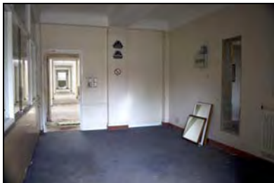
FHH17-0994 Building 1 interior start
