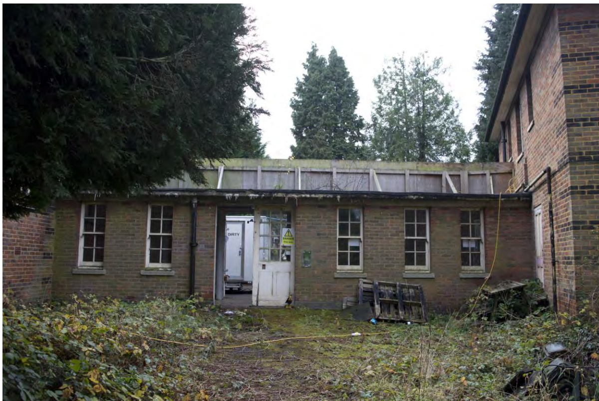
Plate 115 Building 28, nurses' home, corridor linking Buildings 28 and 25, facing south (FHH17-0733)
