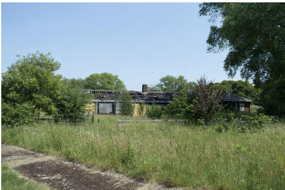
Plate 202 Building 48, male pavilion, south-south-west elevation (FHH17-0377)
