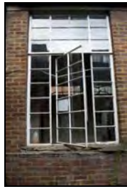
FHH17-0986 Building 1 courtyard start
