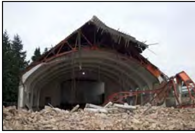
FHH17-1432 Building 4 during demolition
