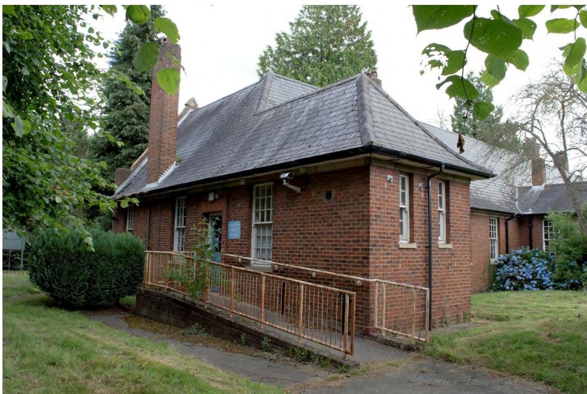
Plate 4 Building 1, entrance/administrative block, facing north-east (FHH17-474)
