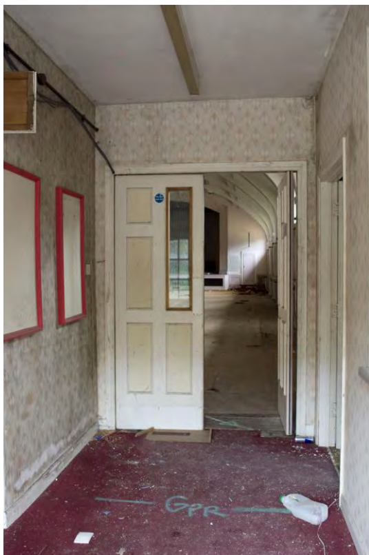
Plate 42 Building 4, recreation hall, entrance lobby in north-west wing, facing south (FHH17-0137)
