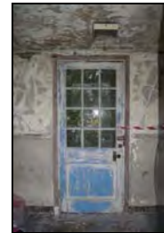
FHH17-1386 Building 27 internal end
