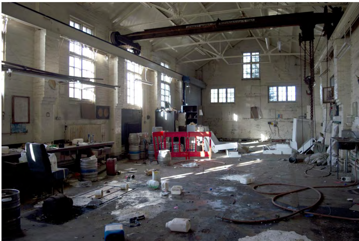
Plate 58 Building 5, workshop on west side of boiler house, facing north (FHH17-0923)
