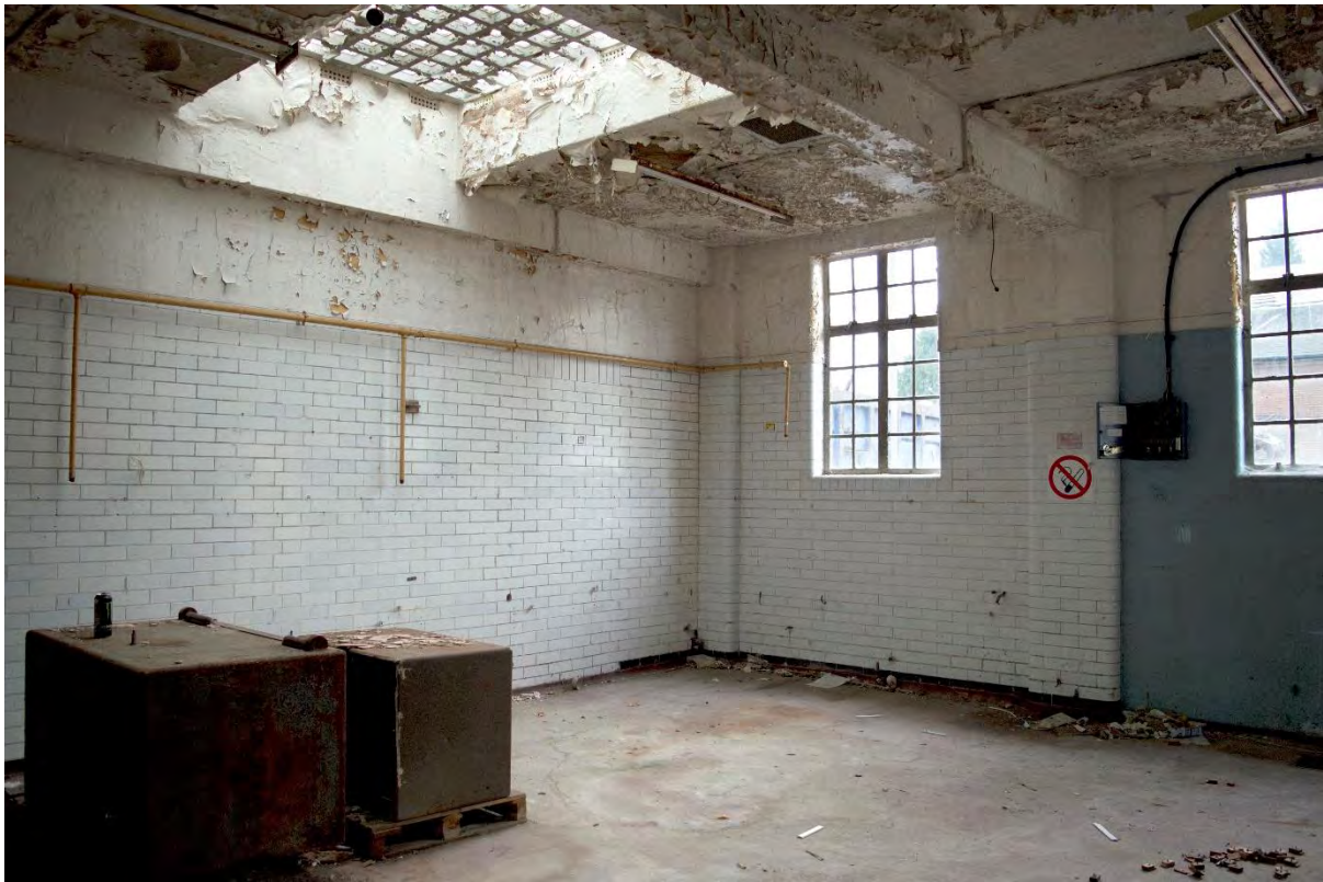
Plate 23 Building 1, central kitchen, scullery, facing south-east (FHH17-1153)
