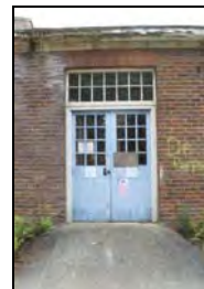
FHH17-0555 Building 11 external end
