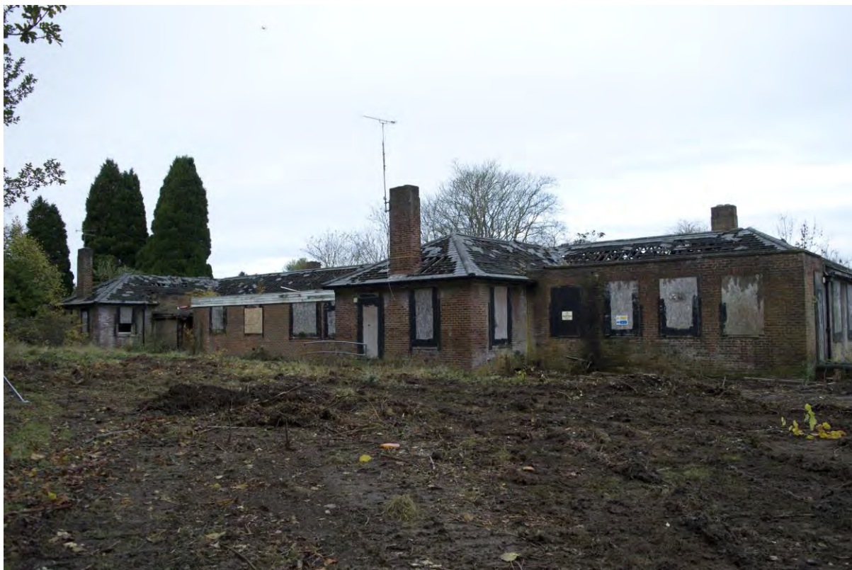
Plate 205 Building 53, male pavilion, principal elevation, facing west (FHH17-0874)
