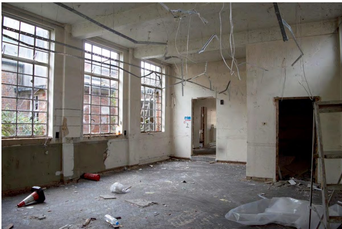
Plate 18 Building 1, dispensary, facing south-west (FHH17-1094)
