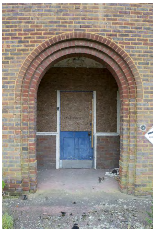
Plate 175 Building 34, male nurses' quarters, principal entrance to north elevation (FHH17-0609)
