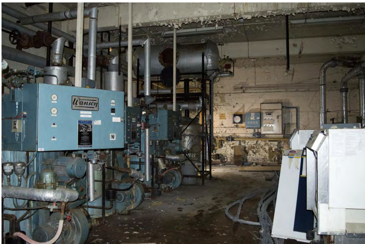
Plate 57 Building 5, boiler house, interior of north block, facing south-east (FHH17-0903)
