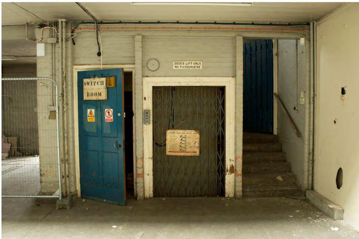
Plate 34: Building 3, main stores, stair and goods lift on north side (FHH17-0036)
