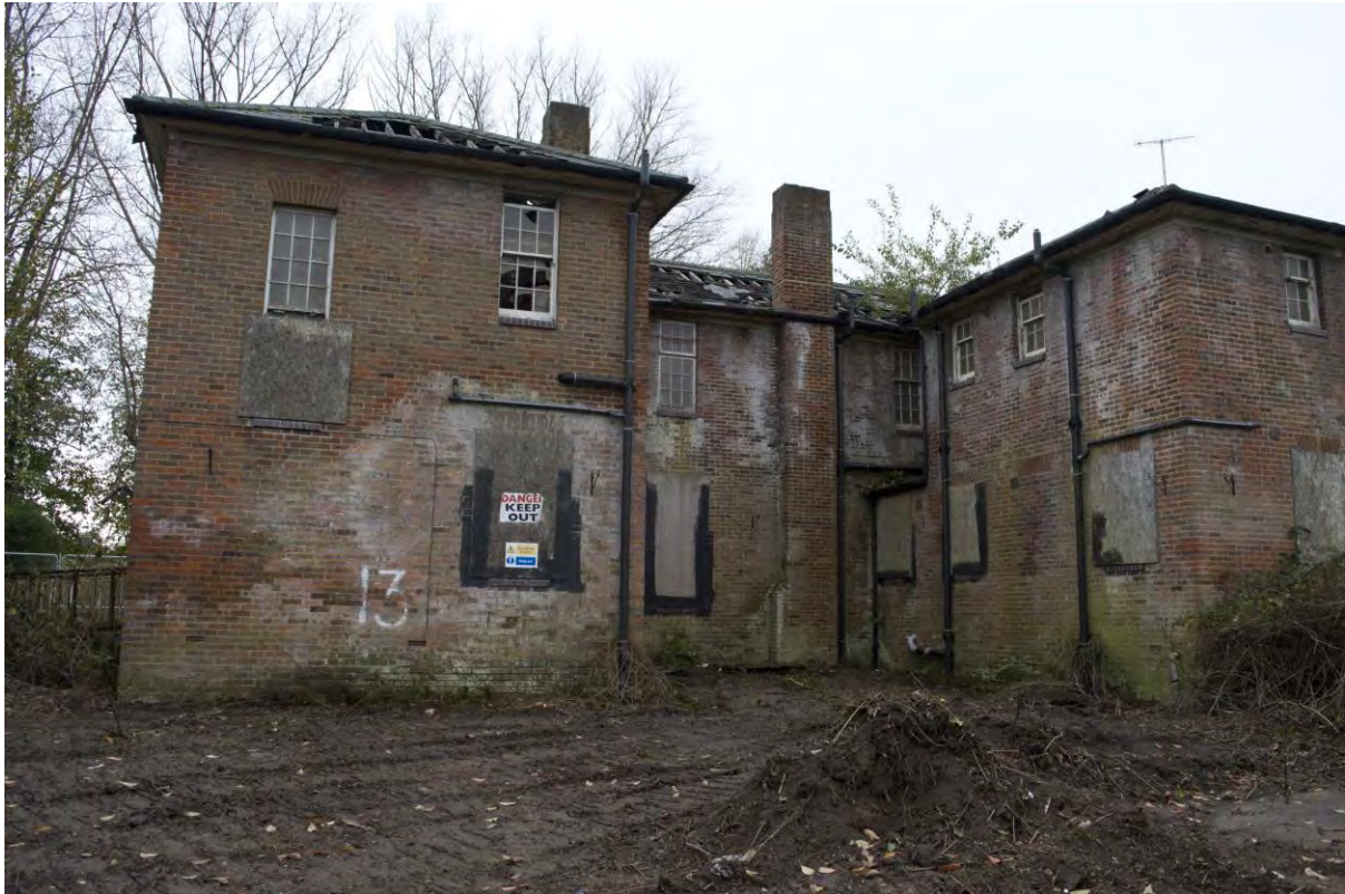
Plate 197 Building 52, male villa, part north elevation (FHH17-0873)
