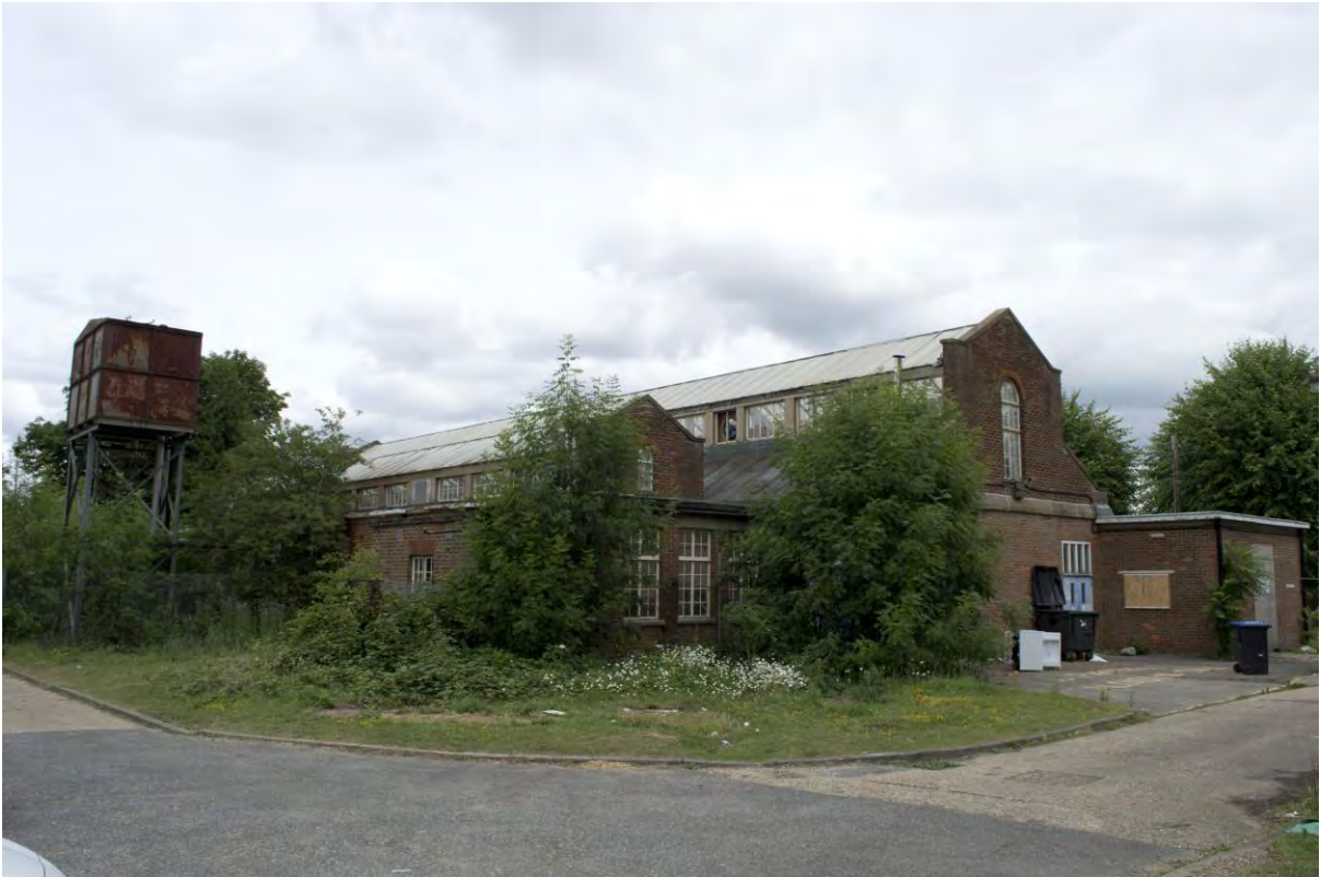
Plate 87 Building 11, general laundry, facing north-east (FHH17-0543)
