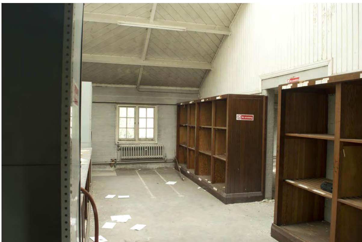
Plate 35: Building 3, main stores, wooden shelving on first floor, facing north (FHH17-0055)
