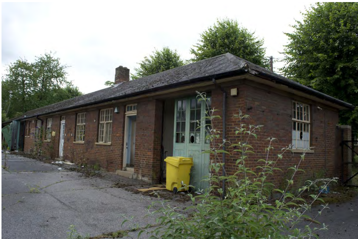
Plate 74 Building 9, workshop, north and east elevations, facing south-west (FHH17-0519)
