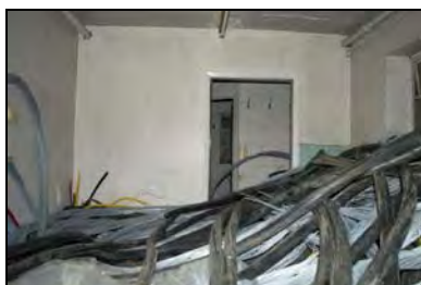
FHH17-0890 Building 05 internal start
