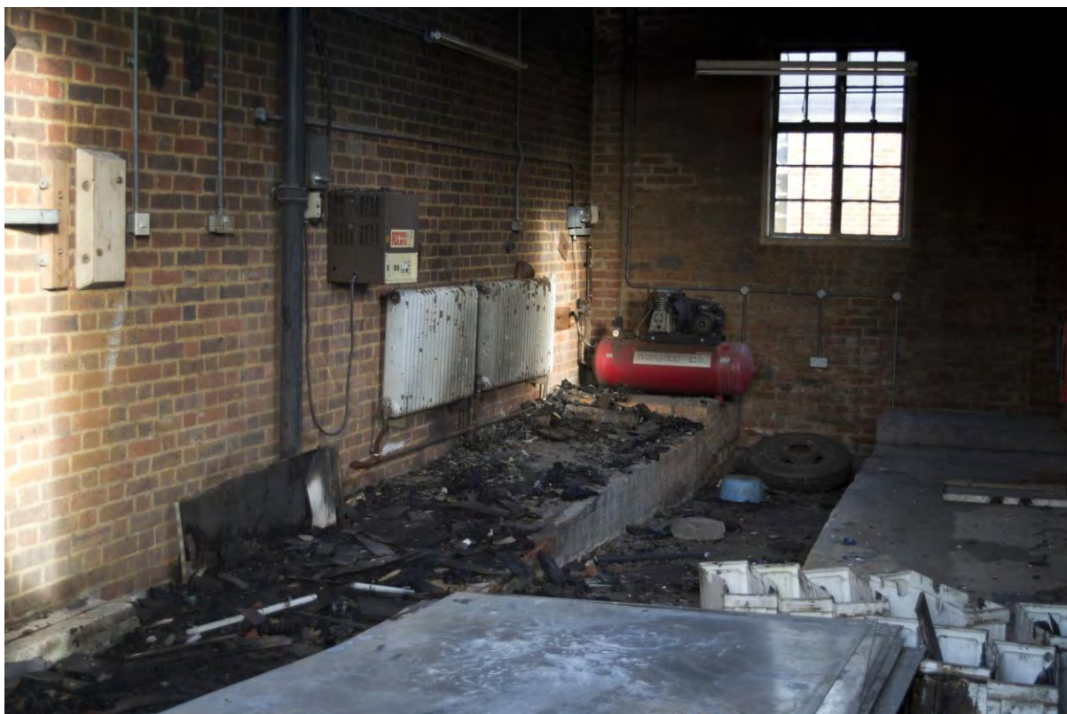
Plate 67 Building 6, fuel store, interior of addition to south, facing east (FHH17-0665)
