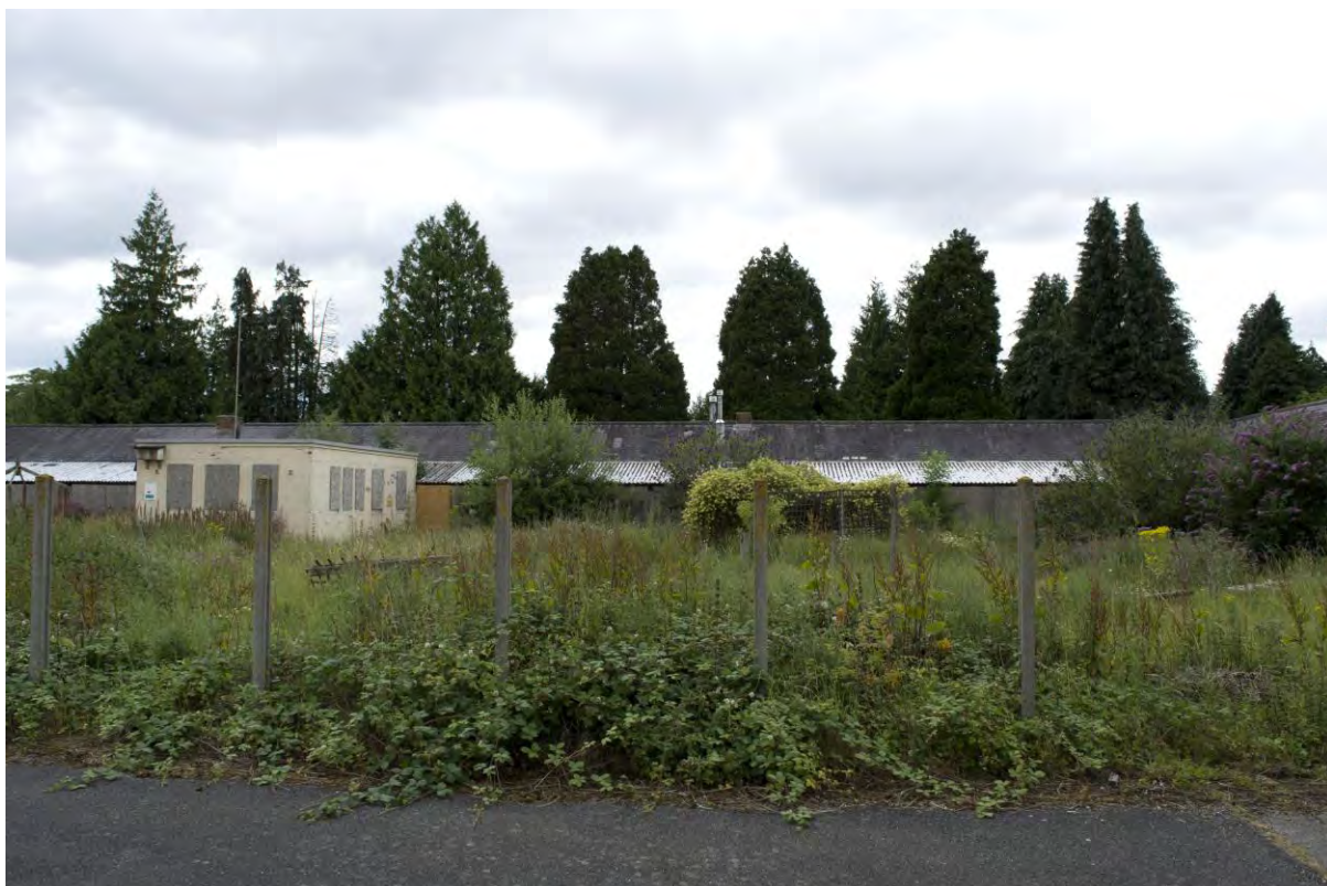
Plate 183 Building 35, workshops, east elevation of west range, showing WC block within yard (FHH17-0642)
