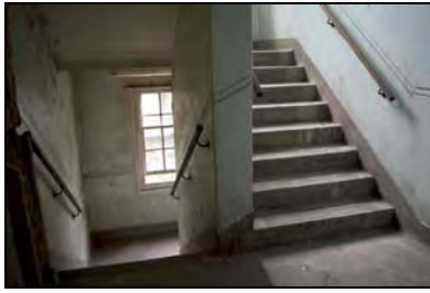
FHH17-0985 Building 28 stairs end
