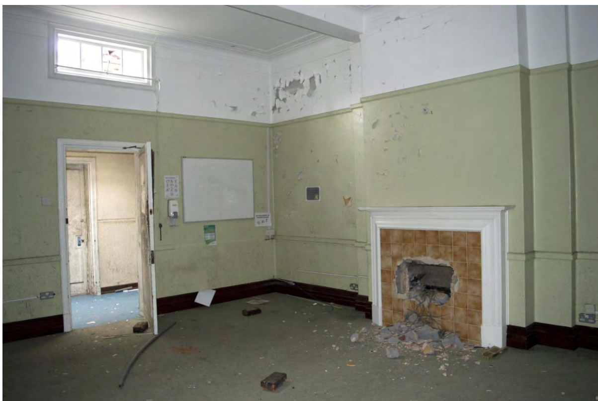
Plate 144 Building 26, nurses' home, Green Room, facing south-east (FHH17-1202)
