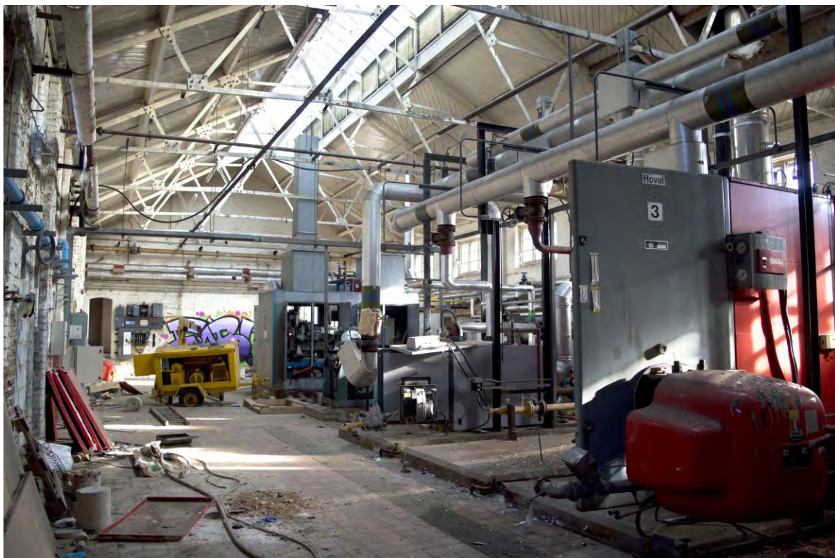
Plate 54 Building 5, boiler house, interior, facing south-east (FHH17-0910)
