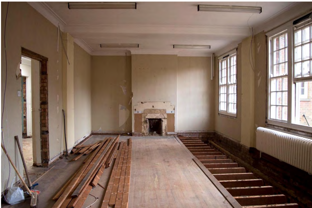
Plate 14 Building 1, entrance/administrative block, probable visiting room, facing south (FHH17-1073)
