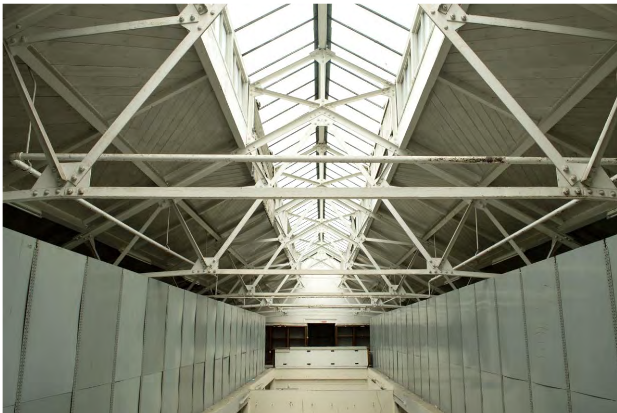
Plate 30 Building 3, main stores, roof, facing east (FHH17-0058)
