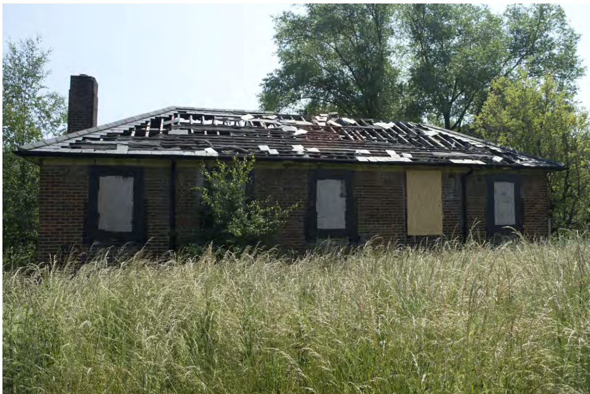
Plate 203 Building 48, male pavilion, west-north-west elevation (FHH17-0380)
