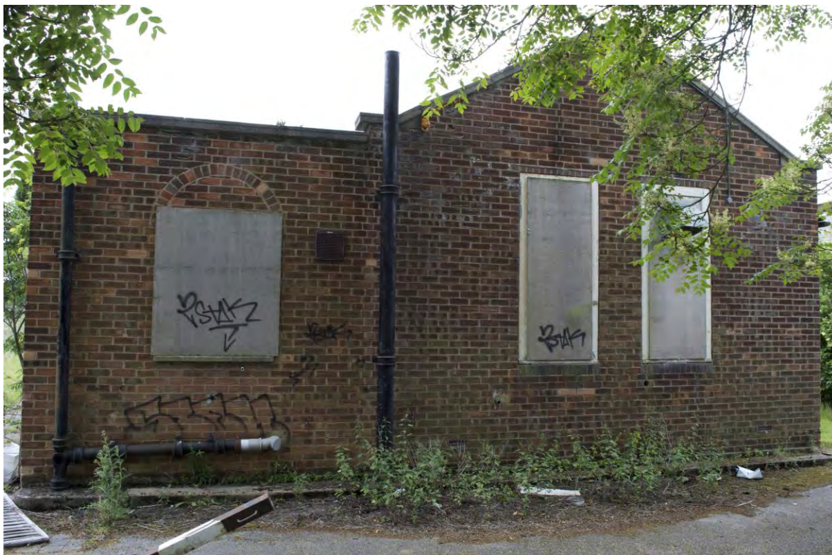
Plate 178 Building 35, workshops, east gable end of north range (FHH17-0644)
