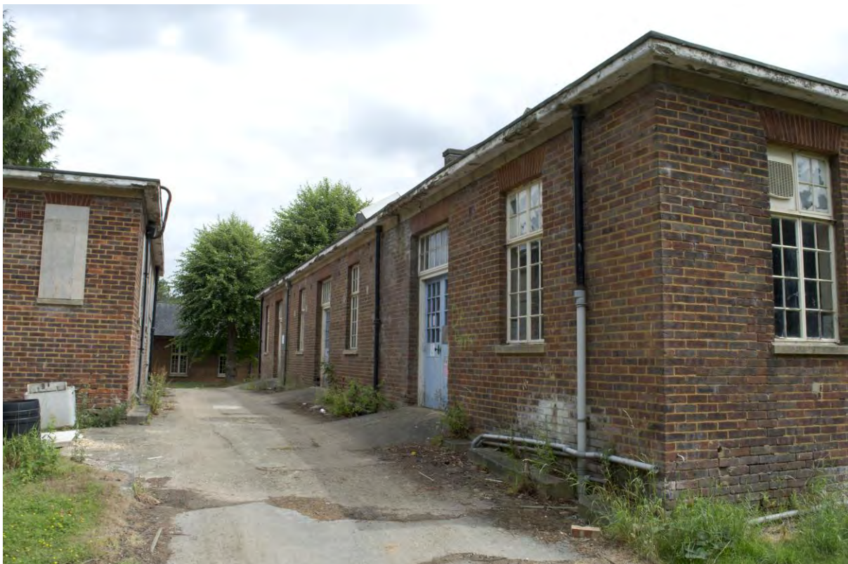
Plate 90 Building 11, general laundry, north elevation, facing east (FHH17-0553)
