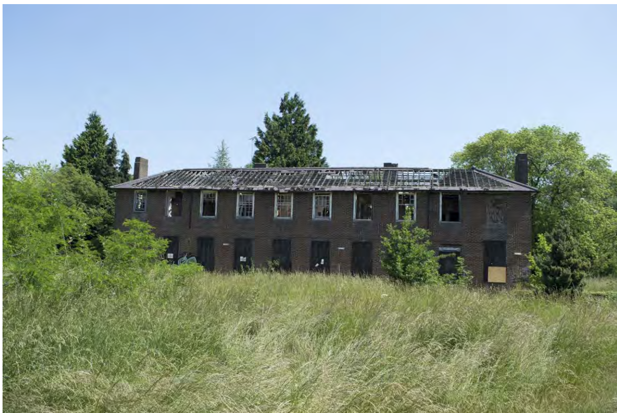
Plate 200 Building 47, male villa, south-west elevation (FHH17-0363)
