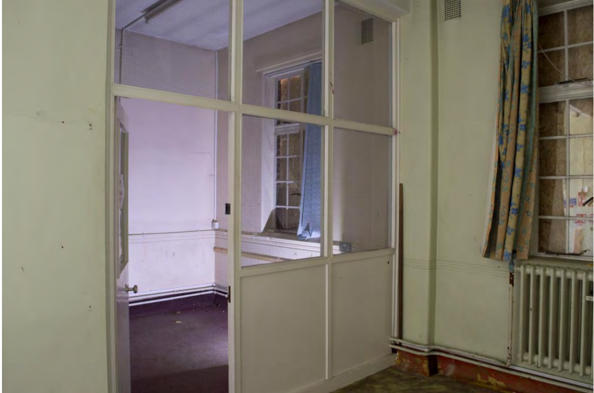
Plate 85 Building 10, staff laundry, modified interior of original laundry distribution room, facing north-east (FHH17-0189)
