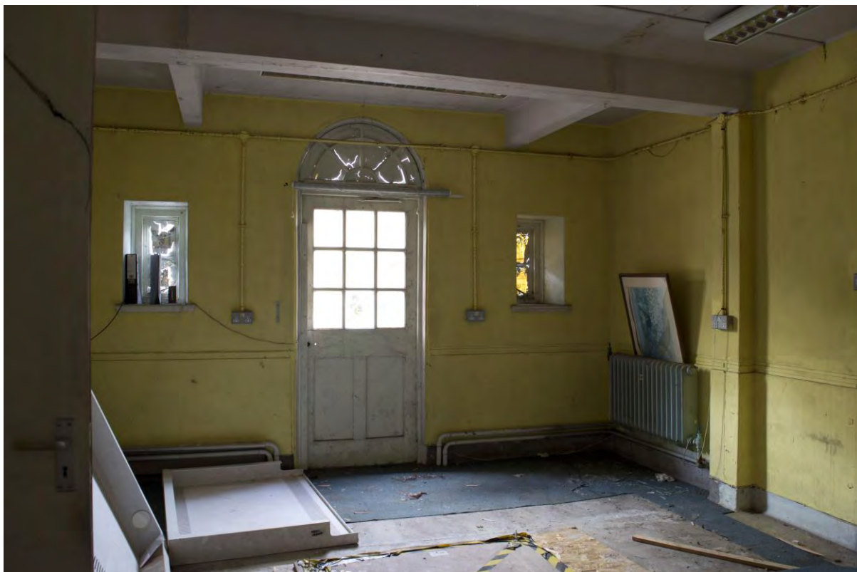
Plate 40 Building 4, recreation hall, entrance hall in entrance block, facing north (FHH17-0155)
