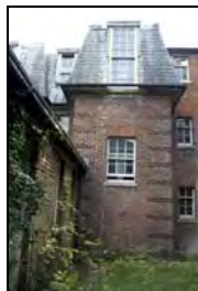
FHH17-0763 Building 28 courtyard external start
