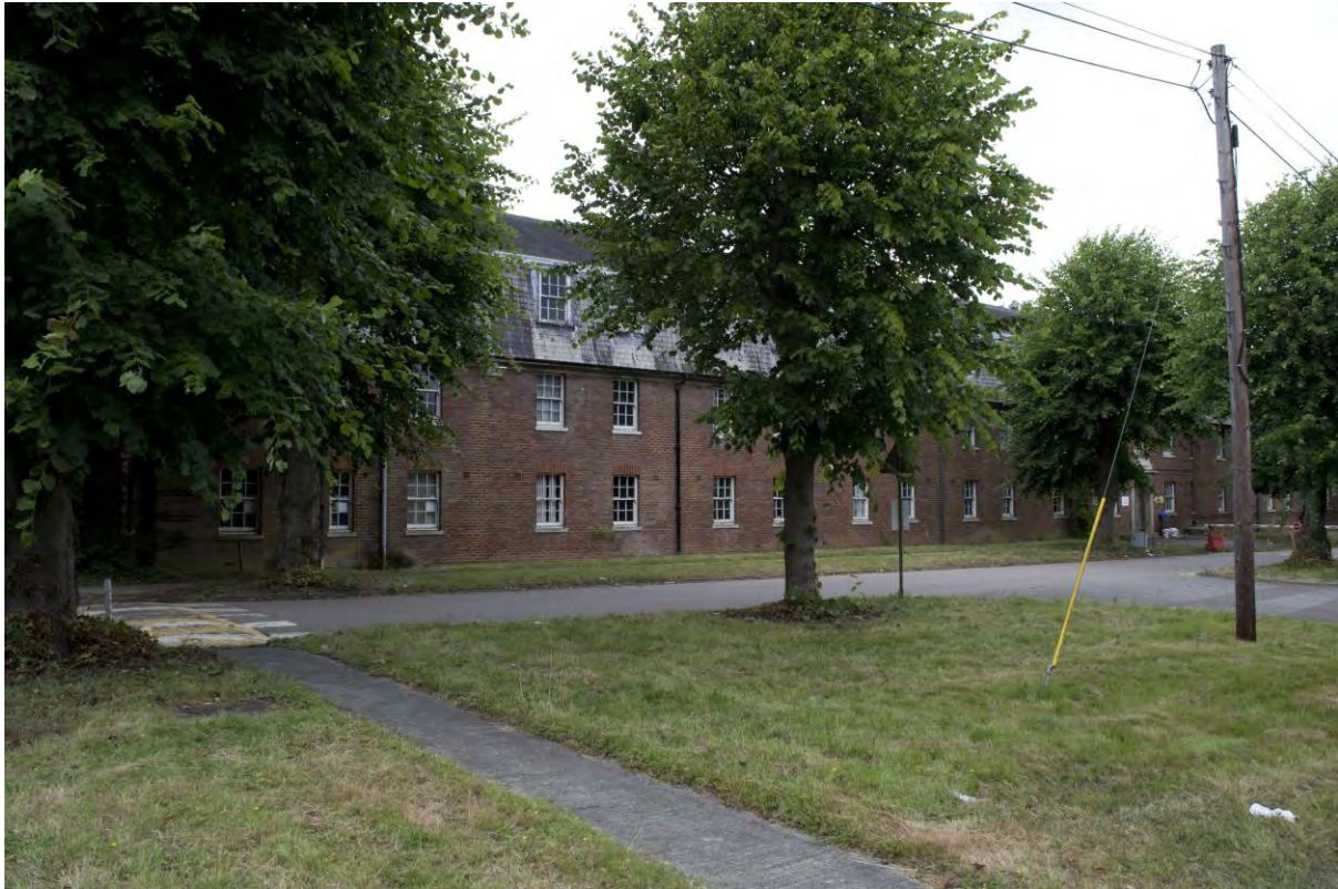
Plate 107 Building 28, nurses' home, east elevation, facing west-north-west (FHH17-0556)
