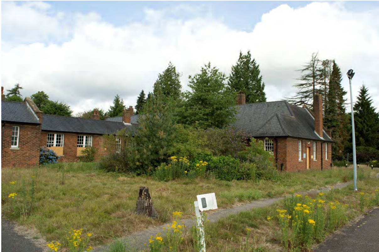
Plate 5 Building 1, entrance/administrative block, facing north-west (FHH17-0451)
