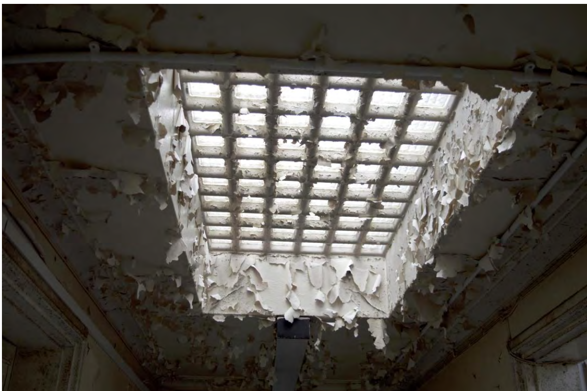
Plate 140 Building 26, nurses' home, roof light in corridor (FHH17-1182)
