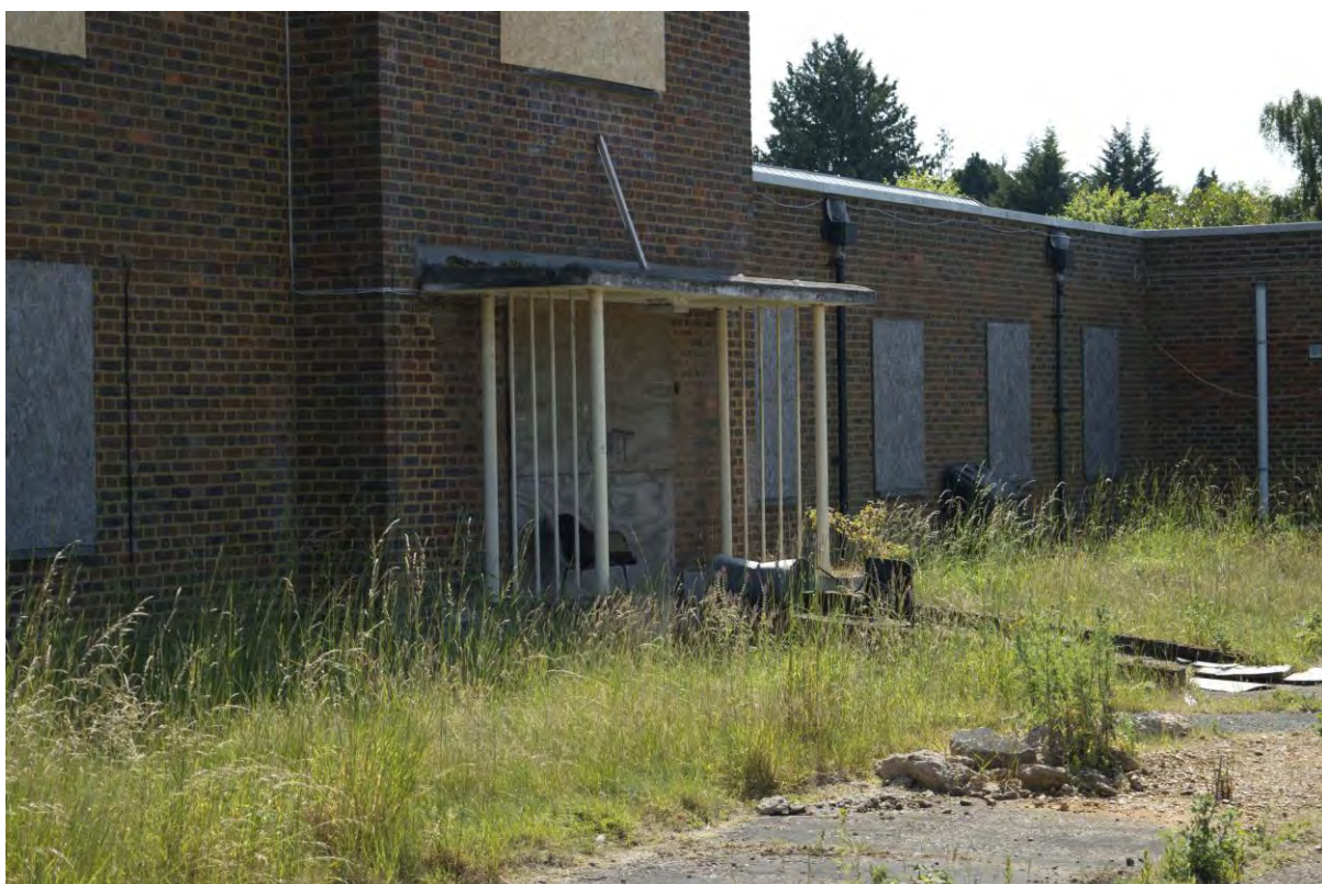
Plate 171 Building 33, nurses' library and postgraduate centre, main entrance, facing south-west (FHH17-0292)
