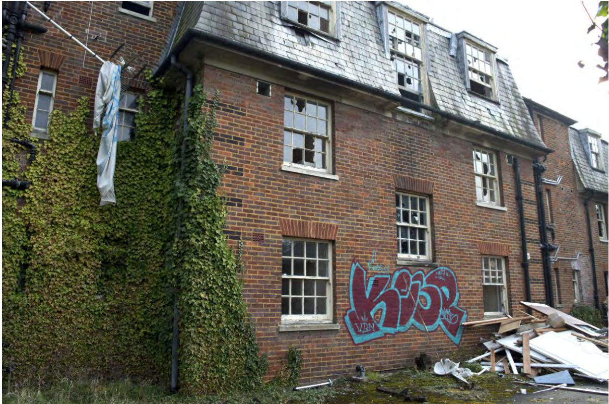
Plate 113 Building 28, nurses' home, west elevation of central part of building (FHH17-0769)
