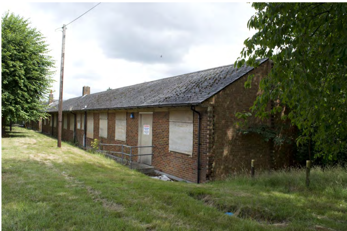
Plate 75 Building 9, workshop, south and west elevations, facing north-east (FHH17-0521)
