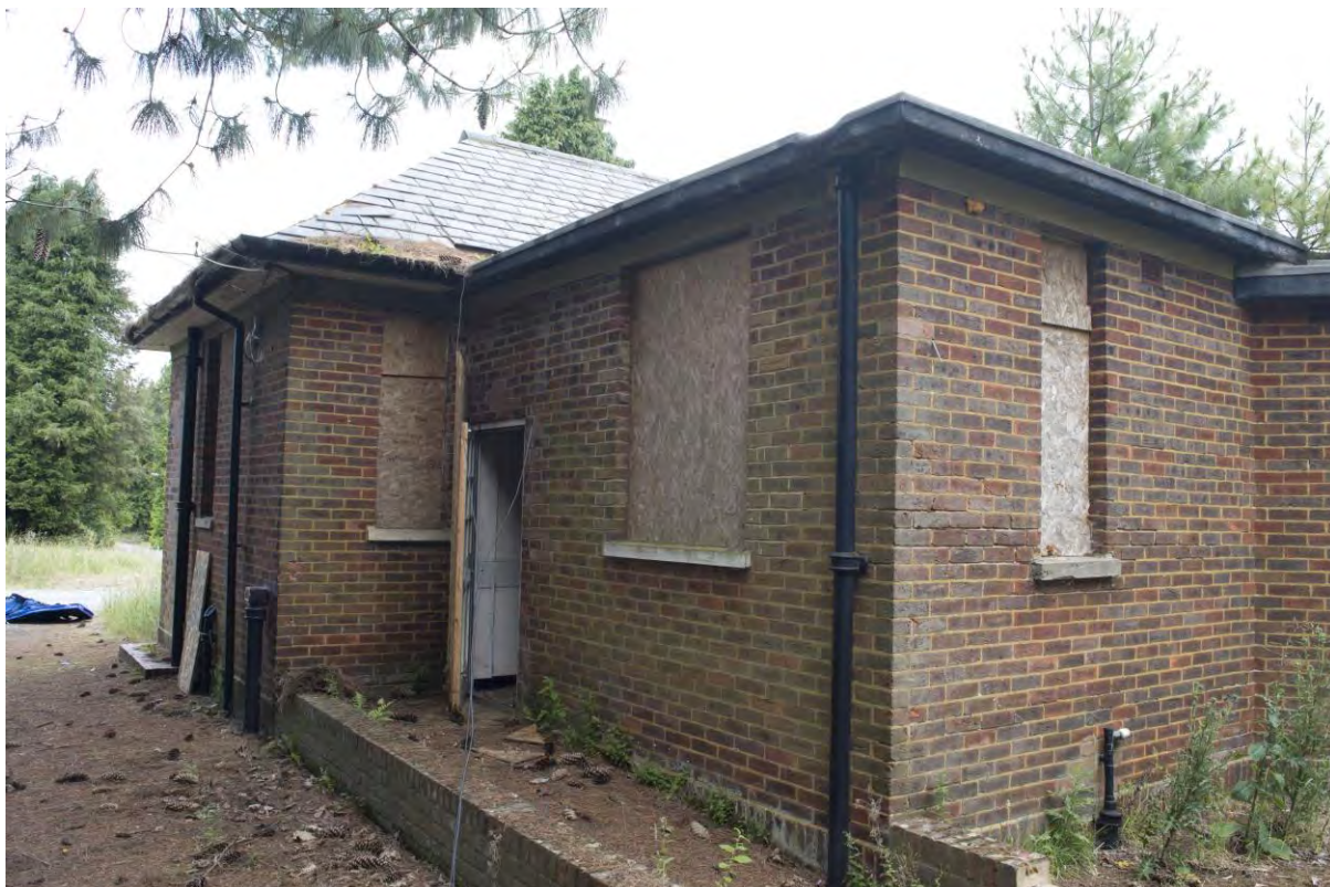
Plate 213 Building 56, mortuary, west elevation (FHH17-0415)
