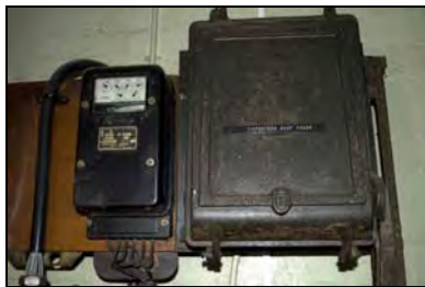
FHH17-0944 Building 05 internal end
