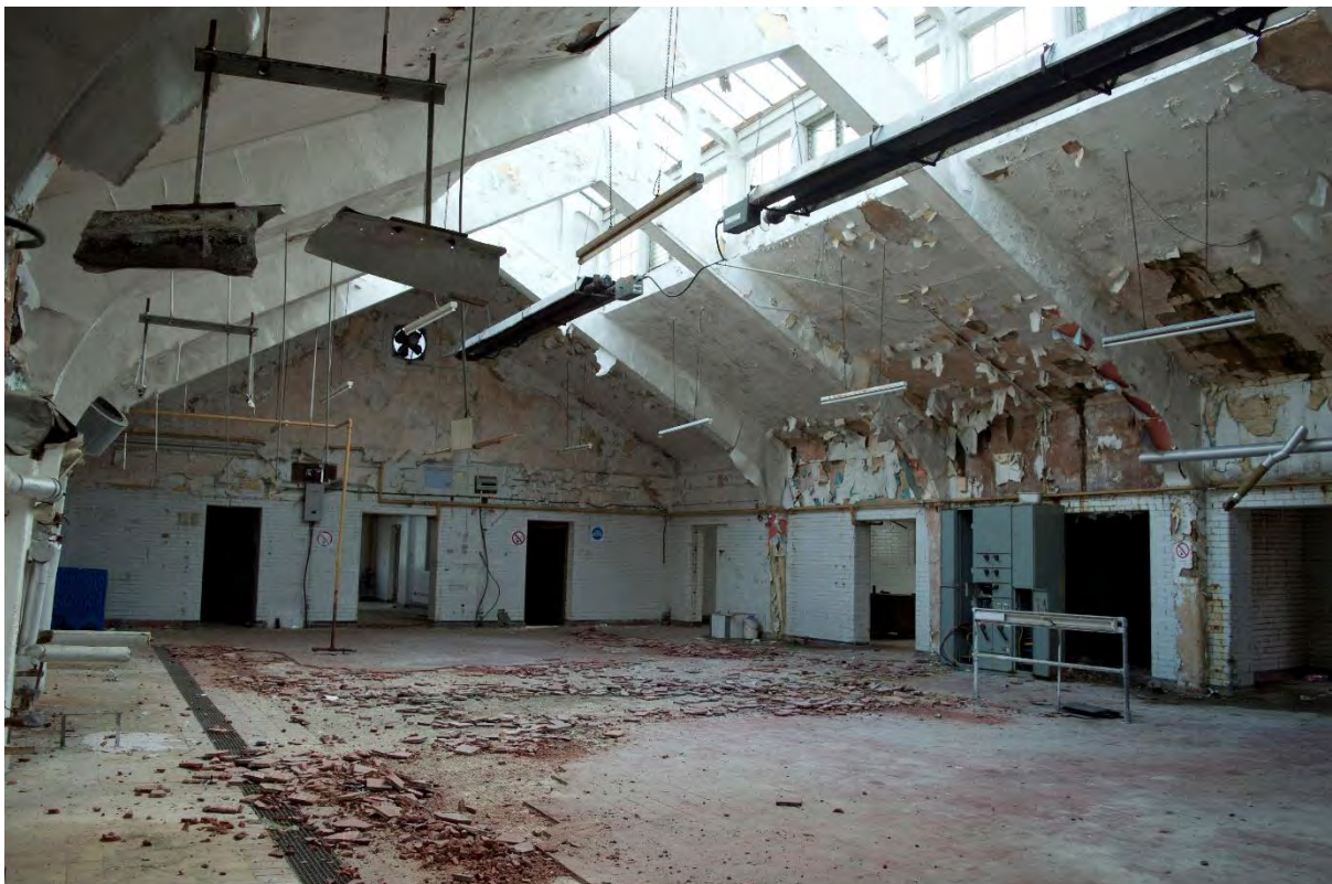
Plate 20 Building 1, central kitchen, facing south-east (FHH17-1164)
