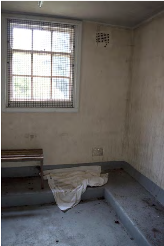
Plate 153 Building 26, nurses' home, vegetable store, facing south (FHH17-1249)
