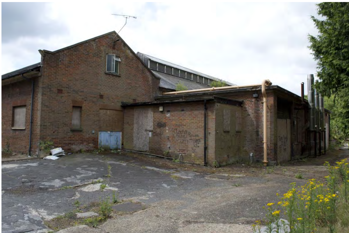
Plate 48 Building 5, boiler house and bakery, north-elevation, facing south-west (FHH17-0479)
