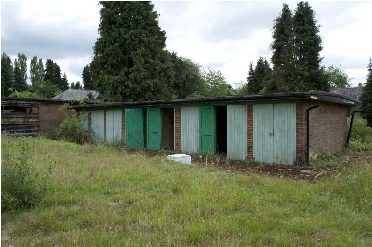
Plate 184 Building 36, north range of smaller garages, facing south-west (FHH17-0299)
