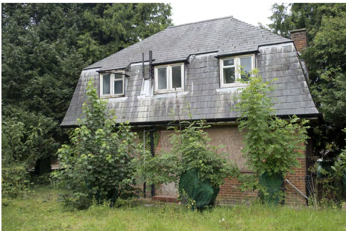
Plate 165 Building 29, gate lodge, west elevation (FHH17-0254)
