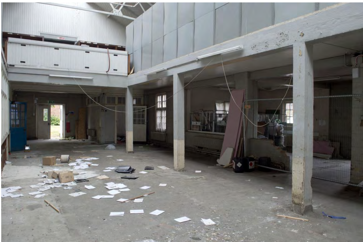
Plate 29 Building 3, main stores, interior, facing west (FHH17-0019)
