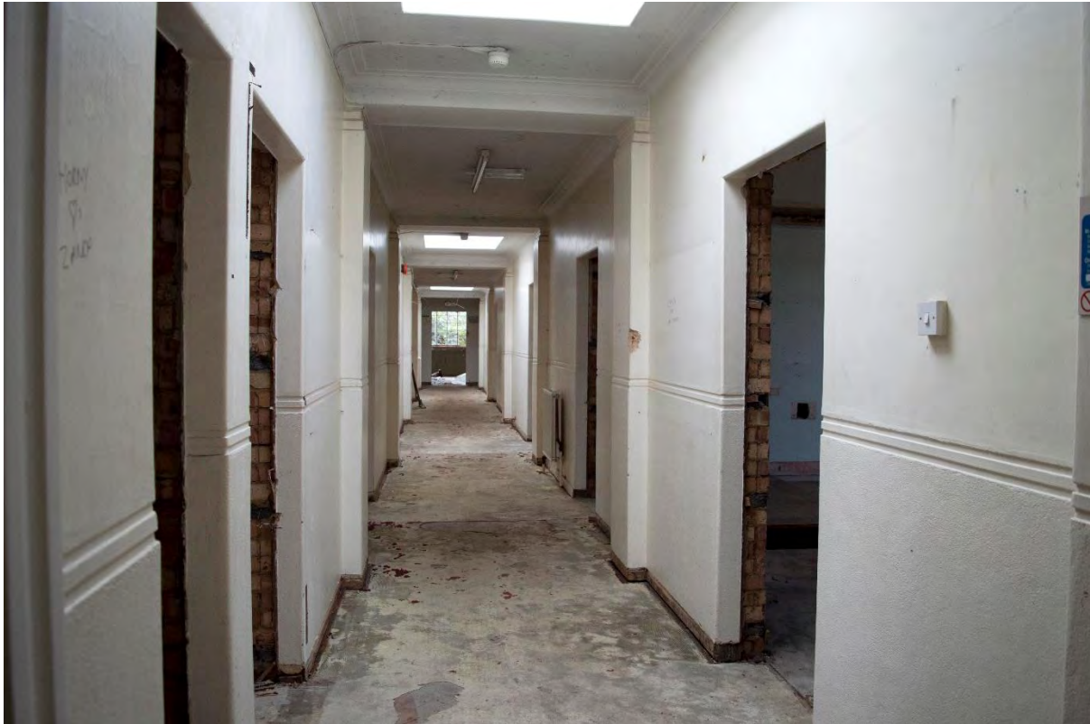
Plate 13 Building 1, entrance/administrative block, south corridor, facing south (FHH17-1047)
