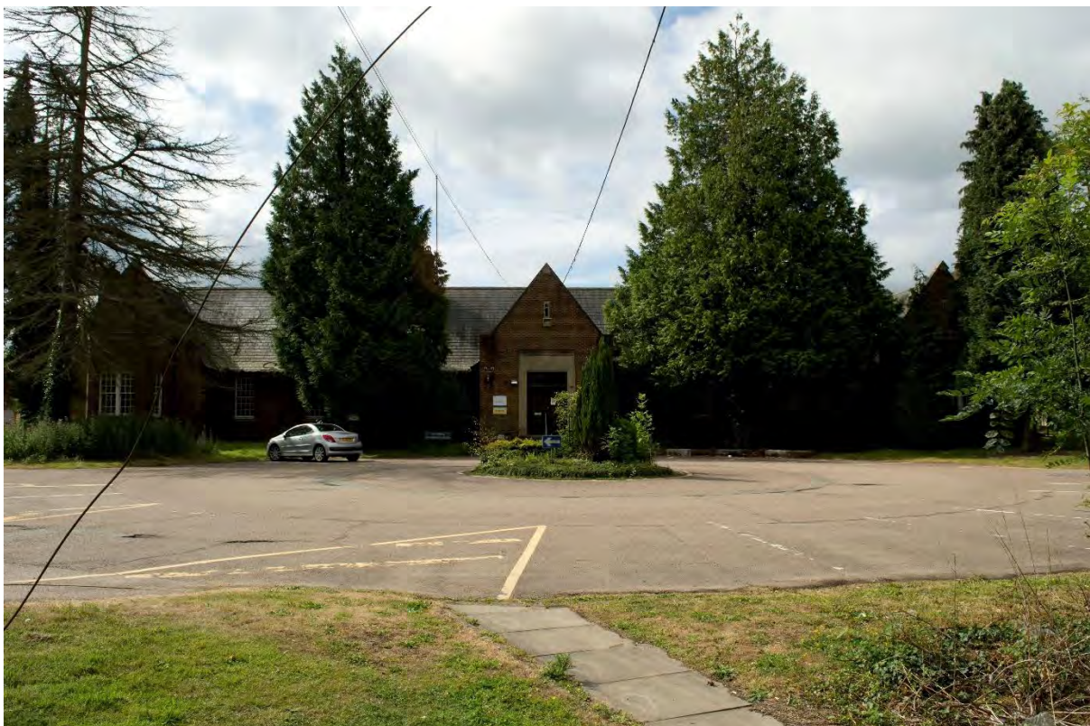
Plate 2 Building 1, principal (north) elevation of the entrance/administrative block (FHH17-0443)
