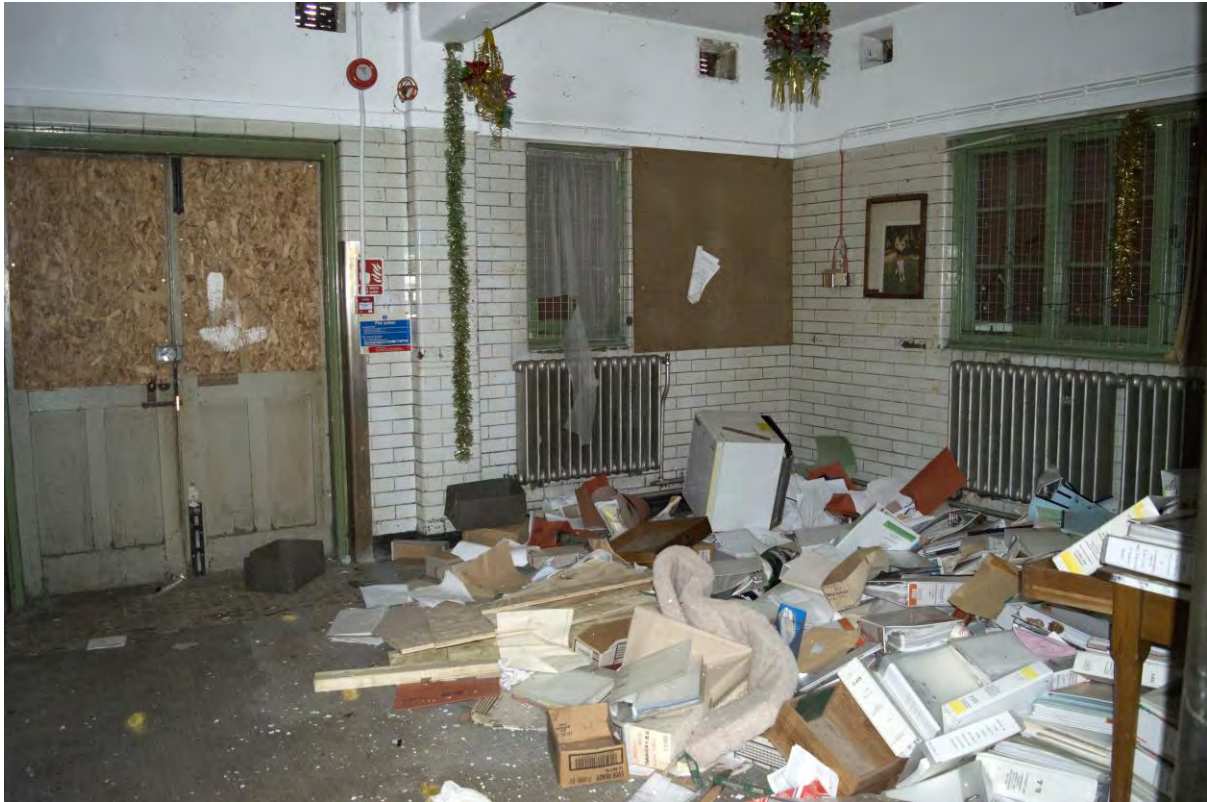
Plate 62 Building 5, bakery, cooling room, facing north-east (FHH17-0931)
