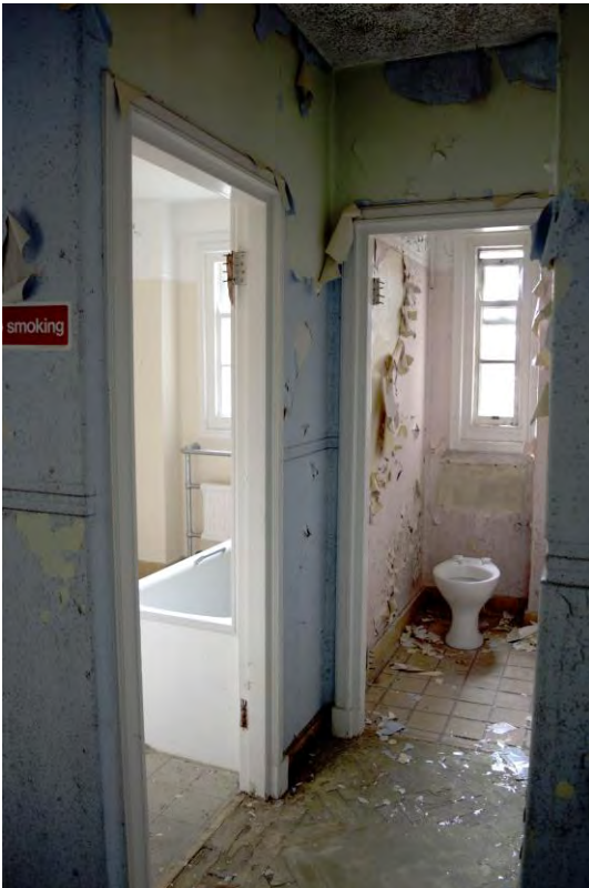
Plate 120 Building 28, nurses' home, typical bathroom arrangement, first floor (FHH17-0781)
