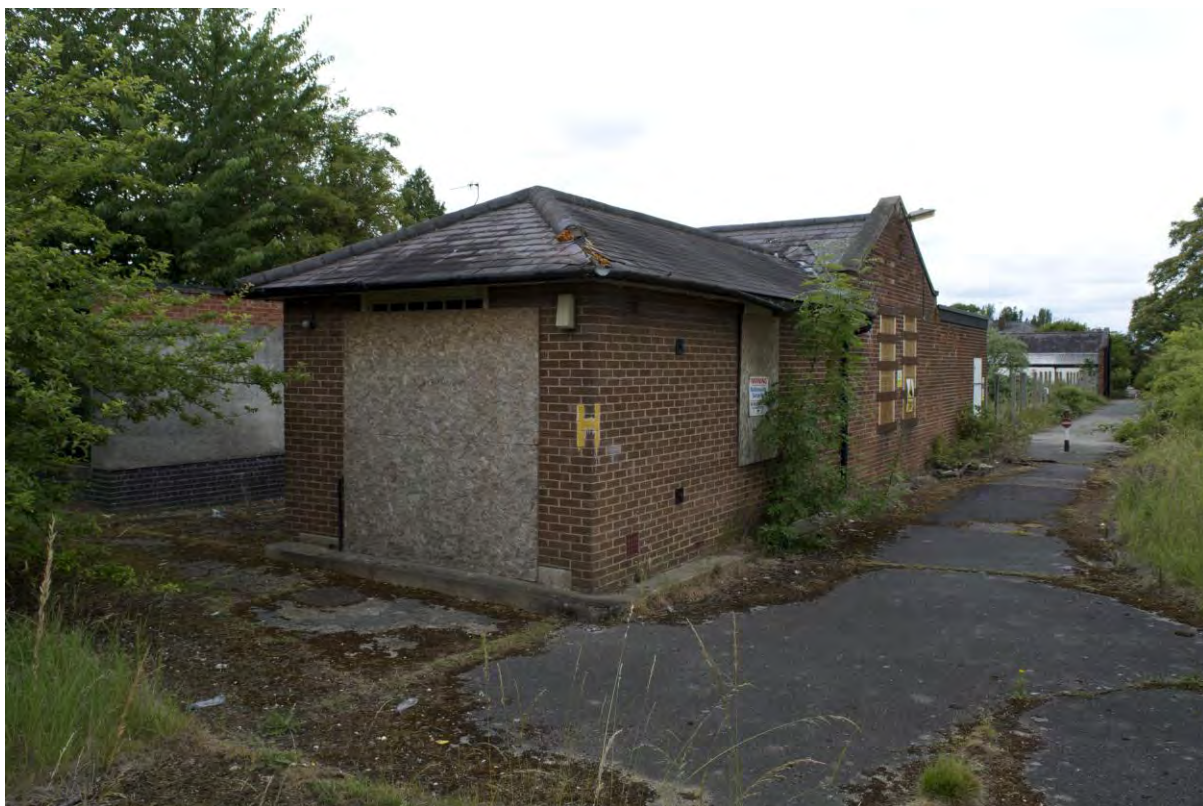
Plate 181 Building 35, workshops, extensions to east end of south range, facing north-west (FHH17-0634)
