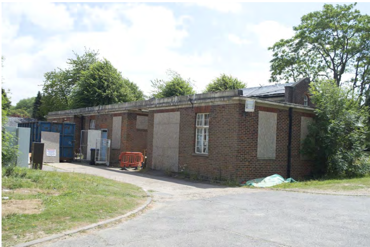
Plate 81 Building 10, staff laundry, facing south-east (FHH17-0182)
