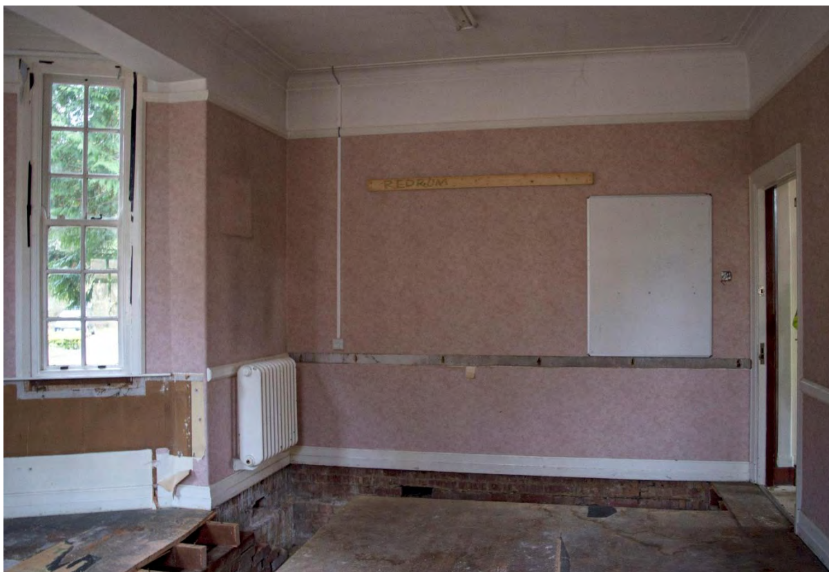
Plate 12 Building 1, entrance/administrative block, typical room in north range (FHH17-1035)
