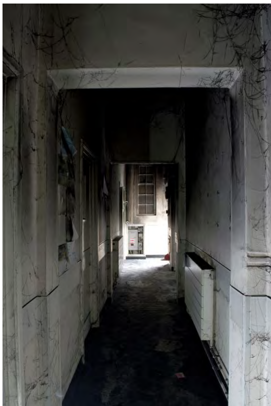
Plate 215 Building 56, mortuary, central corridor, facing east (FHH17-0425)
