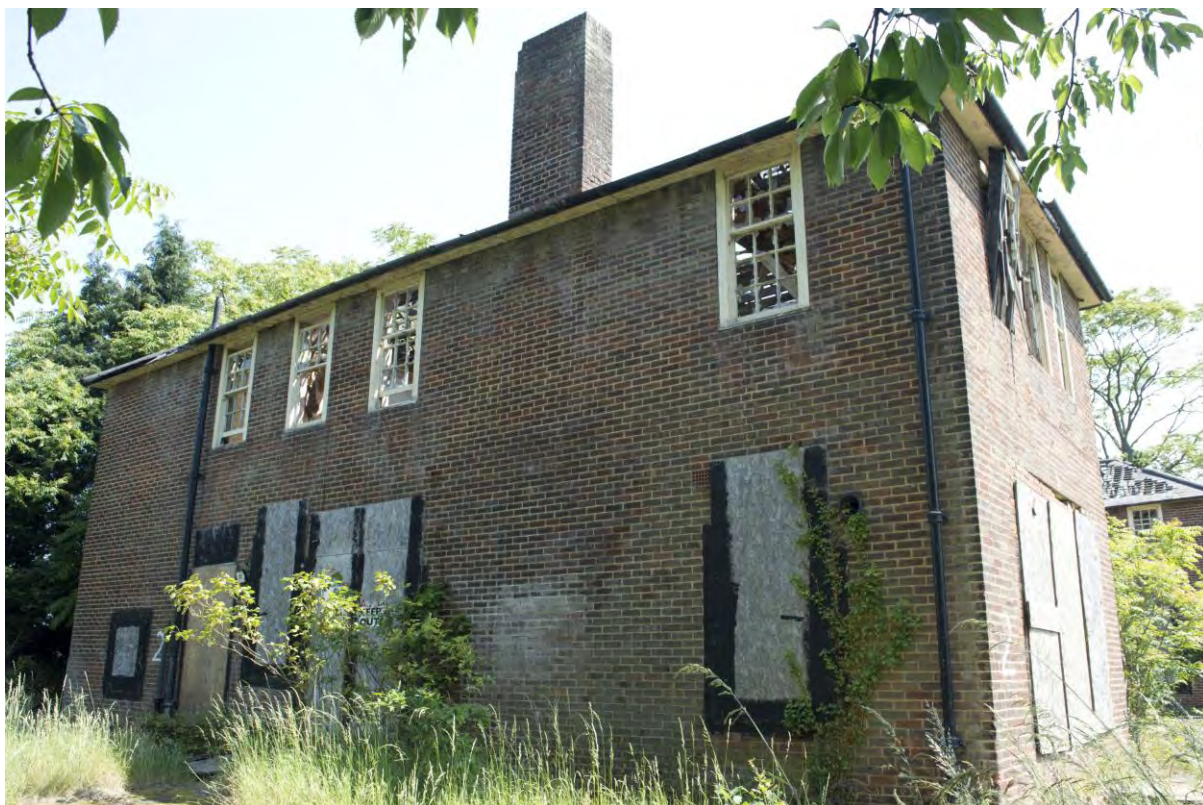
Plate 196 Building 41, male villa, west elevation (FHH17-0354)
