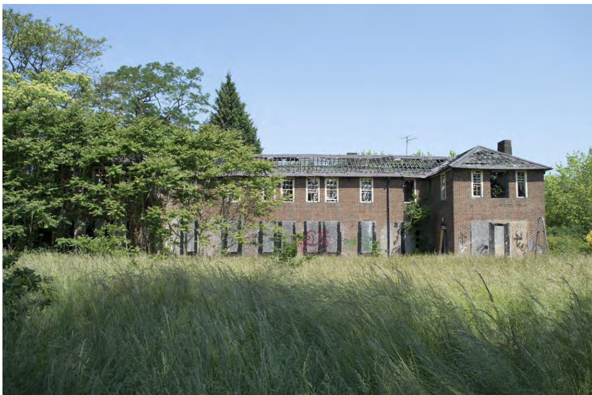
Plate 194 Building 42, male villa, south elevation (FHH17-0362)
