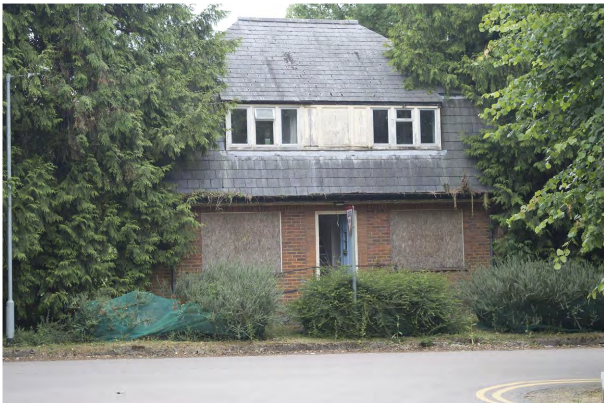
Plate 164 Building 29, gate lodge, east elevation (FHH17-0251)
