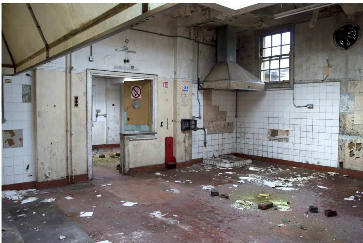
Plate 150 Building 26, nurses' home, main kitchen, facing north-east (FHH17-1236)
