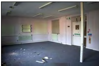
FHH17-0676 Building 09 interior start
