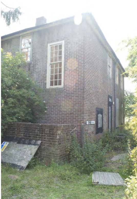
Plate 190 Building 40, male villa, south-west and part north-west elevations, facing east (FHH17-0336)
