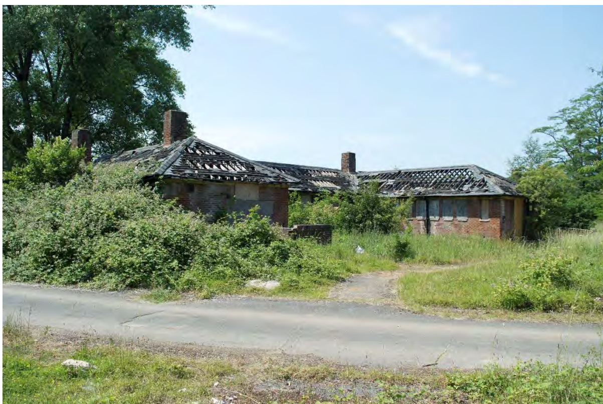
Plate 204 Building 48, male pavilion, rear (east-north-east) elevation, facing west (FHH17-0388)
