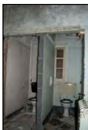
FHH17-1303 Building 27 internal start
