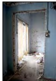
FHH17-1175 Building 1 interior end
