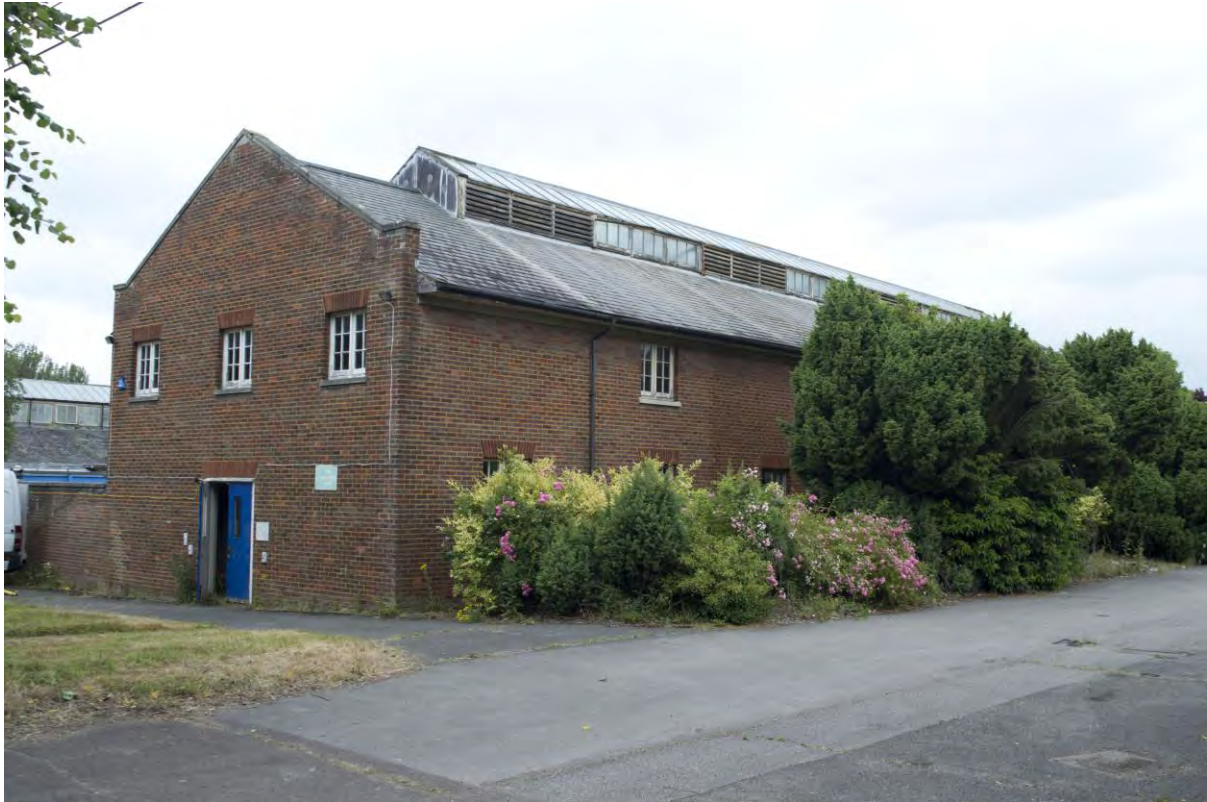
Plate 26 Building 3, main stores, south and west elevations, facing north-east (FHH17-0003)
