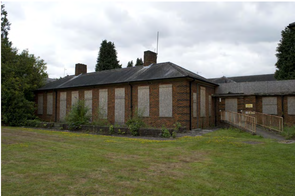
Plate 134 Building 26, nurses' home, facing north-east (FHH17-0583)
