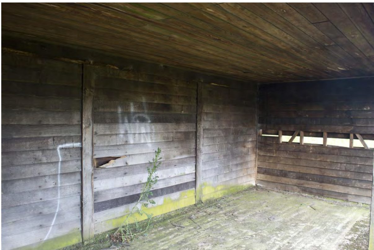
Plate 210 Western football field shelter, interior, facing south-west (FHH17-0329)
