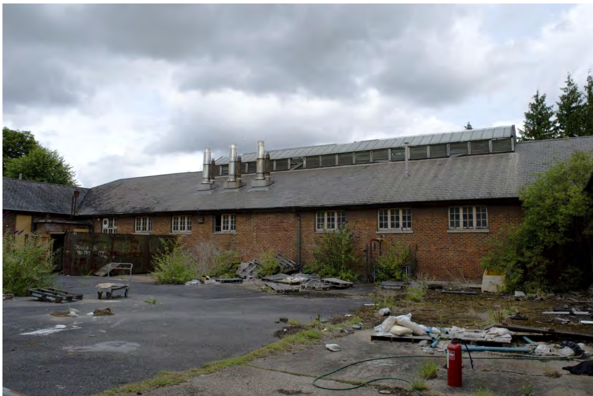
Plate 50 Building 5, boiler house, south elevation, facing north-north-west (FHH17-0496)
