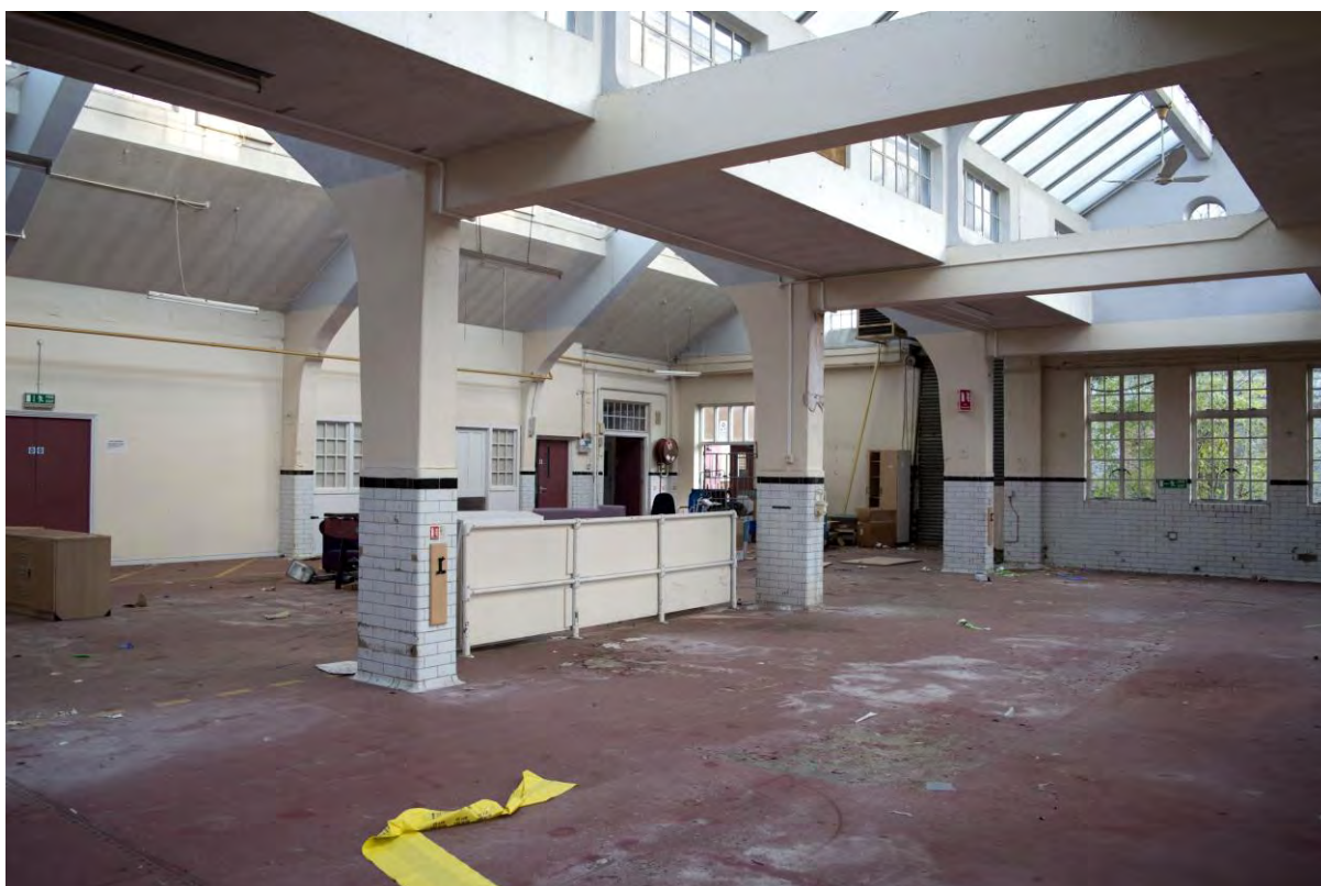
Plate 94 Building 11, general laundry, interior of west flanking range, facing south-east (FHH17-0708)
