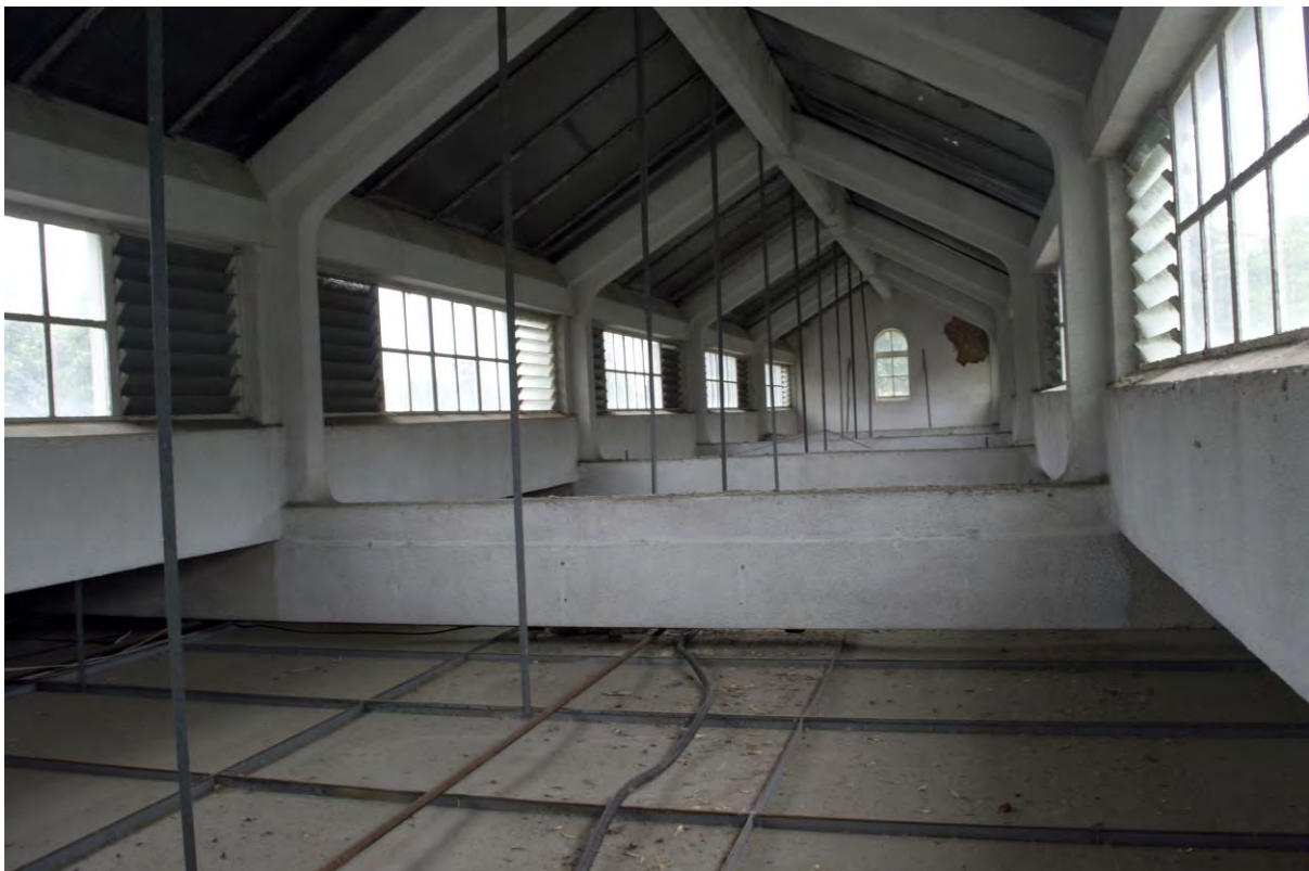
Plate 84 Building 10, staff laundry, roof of main range, facing east (FHH17-0212)
