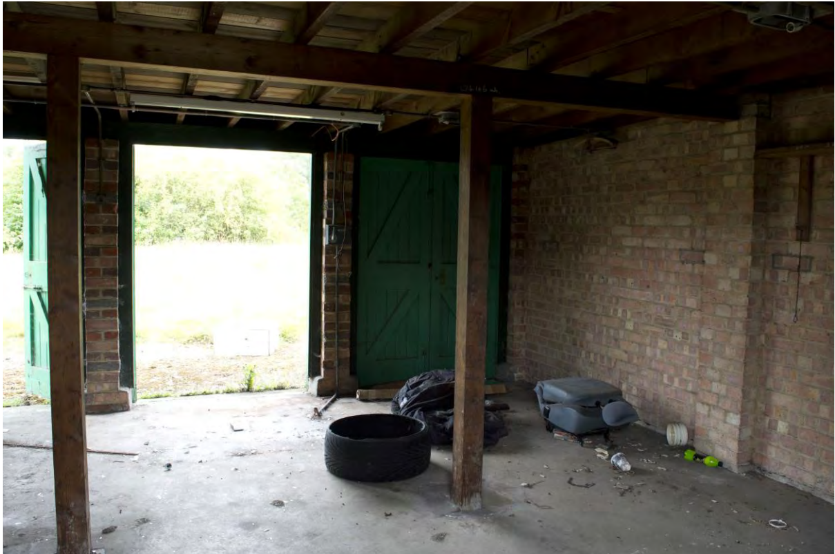
Plate 186 Building 36, interior of north range, facing south-east (FHH17-0313)
