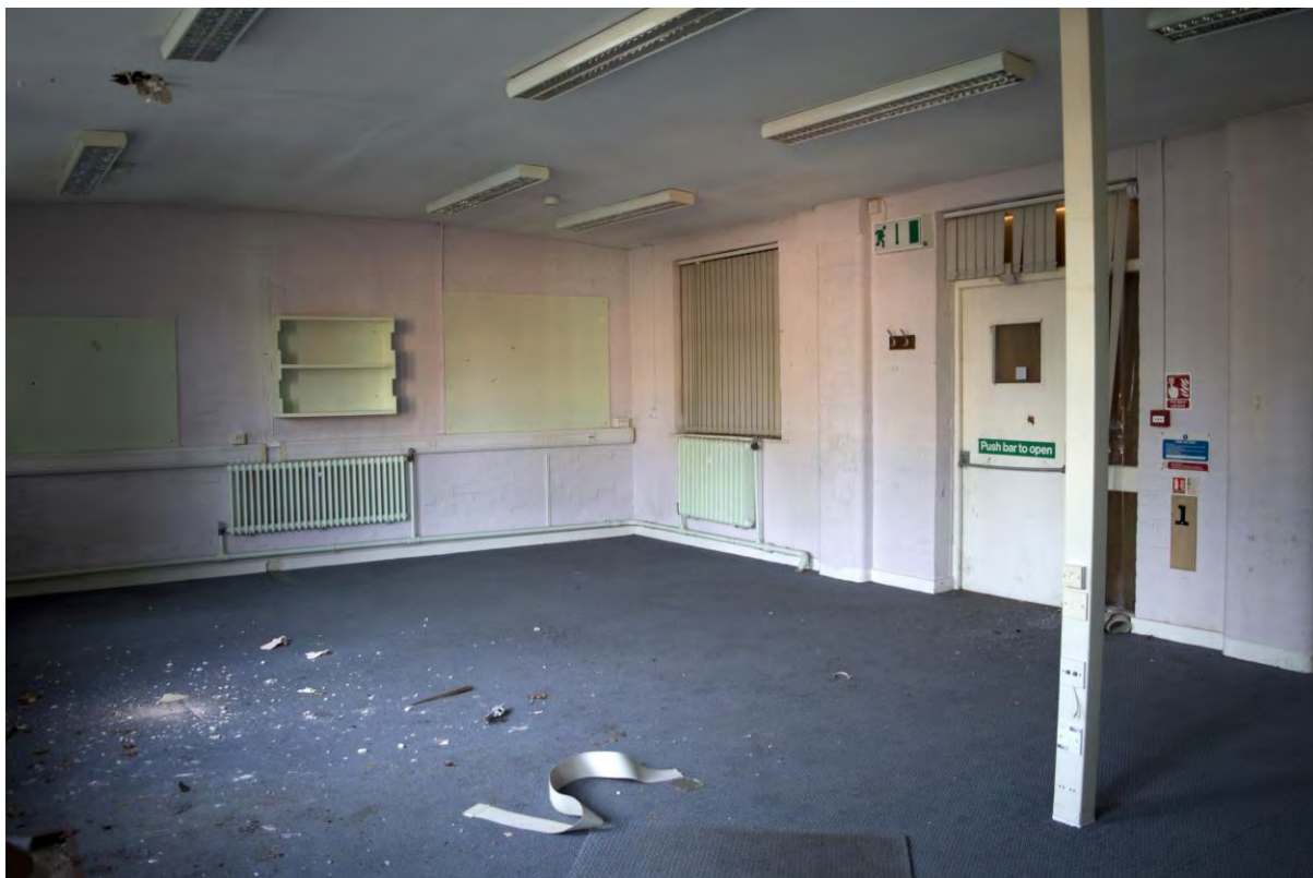
Plate 76 Building 9, workshop, interior of southern part of range, facing south-west (FHH17-0676)
