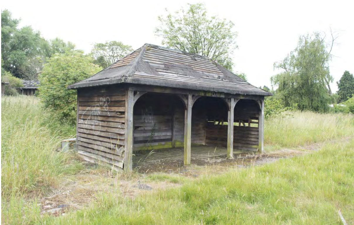
Plate 209 Western football field shelter, facing south-west (FHH17-0328)
