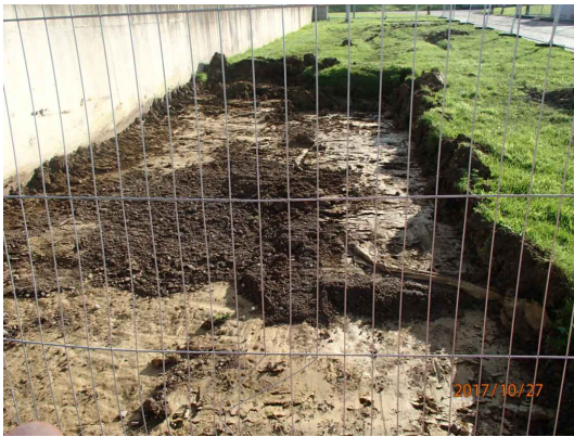
Area 3 looking south
