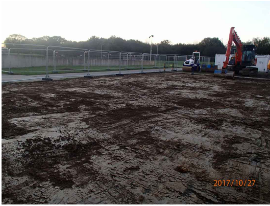
Area 1 looking south-west
