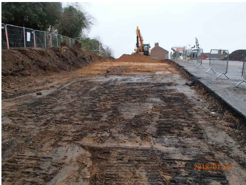
Mechanical ground reduction looking west
