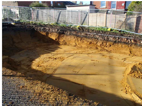
Mechanical ground reduction looking south west
