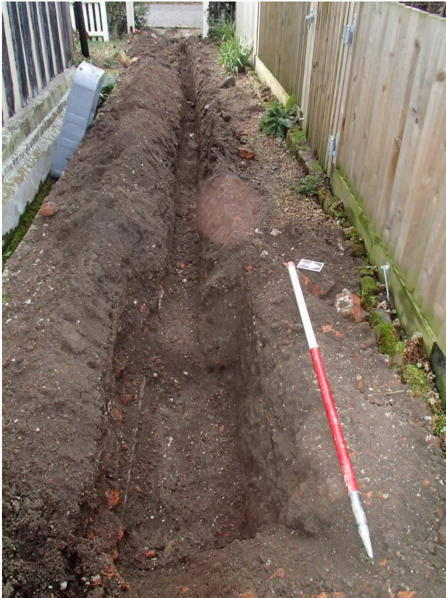
Trench through garden adjacent to the house
