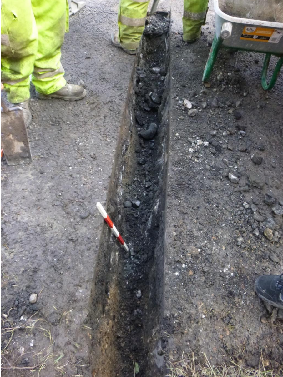
Trench through road
